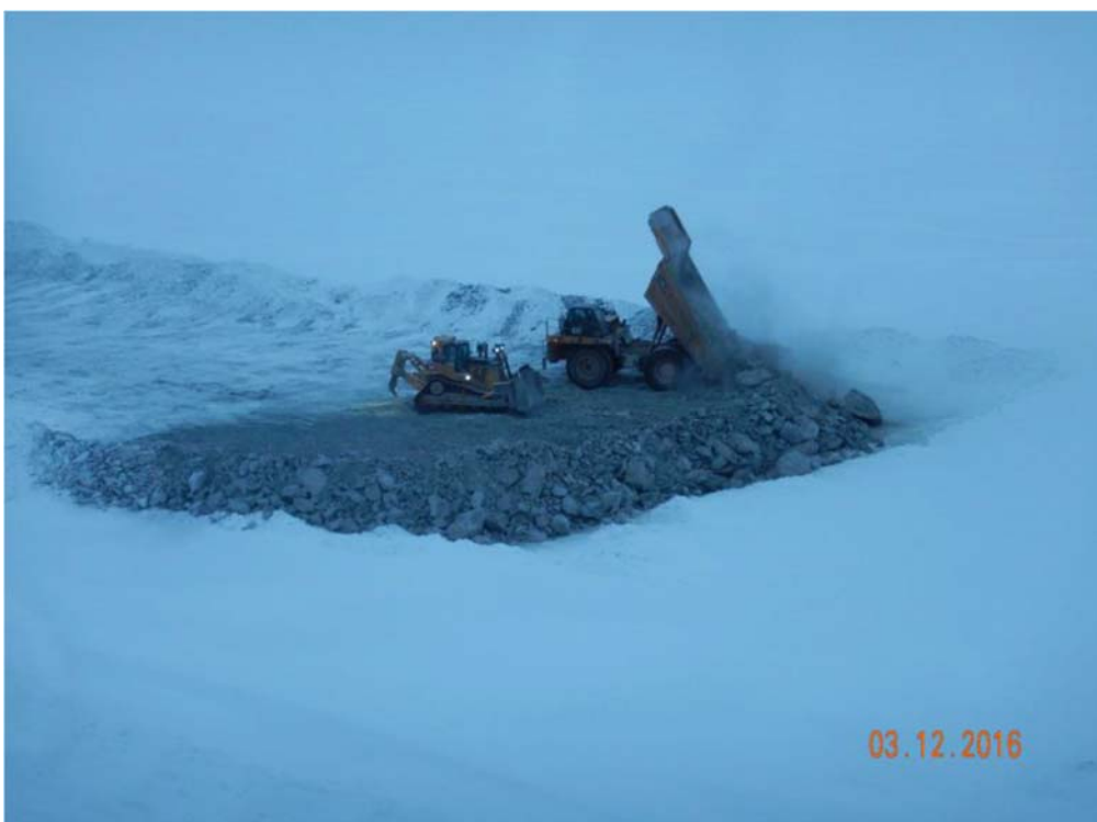
Photo 9: TSF North Cell, NPAG Cover construction, winter 2016
