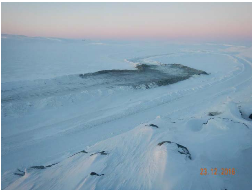
Photo 8: TSF North Cell, NPAG Cover construction, winter 2016
