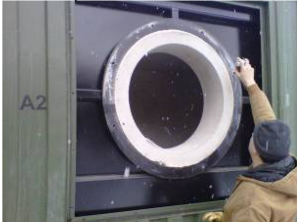
Gasket adhesive spray being applied
