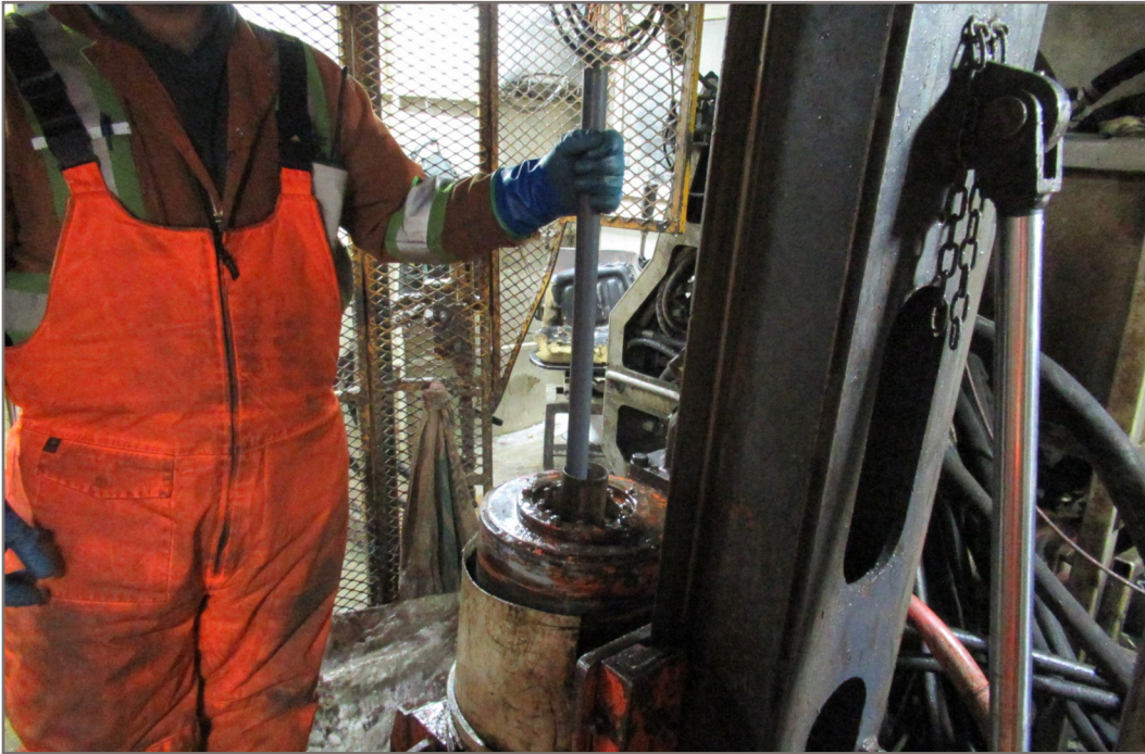
Photo 18: GT21-61 (36) multi-bead GTC installation; depth 10.95 m
