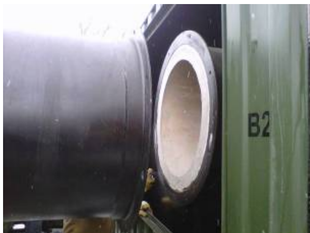
Gasket NOT installed
