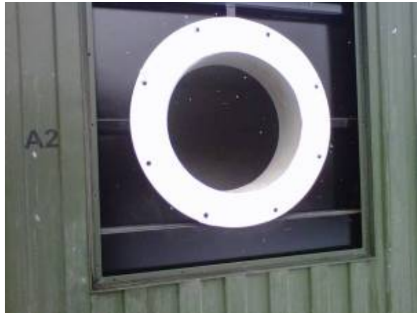
Correctly Installed Gasket
