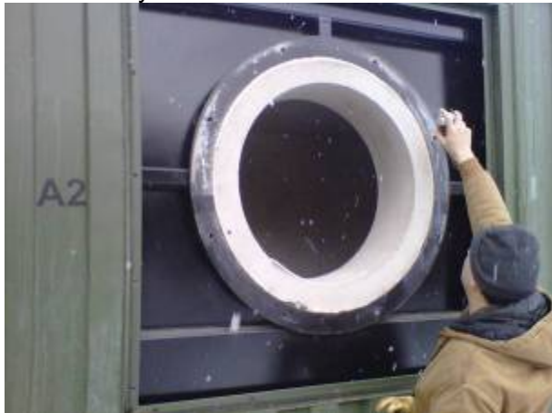
Gasket adhesive spray being applied
