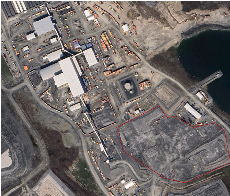
Figure 3.3-2: Transit Pad for Tailings to be Back-Hauled Underground Located within the Confines of the Portal 2 Ore Pad
