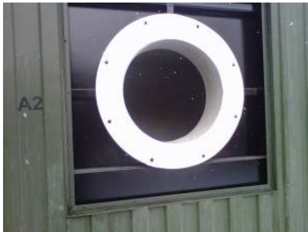
Correctly Installed Gasket
