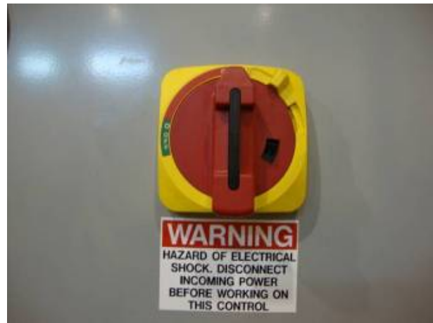
Power is ON in this position
