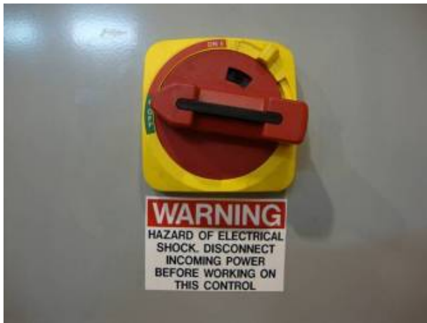
Power is OFF in this position
