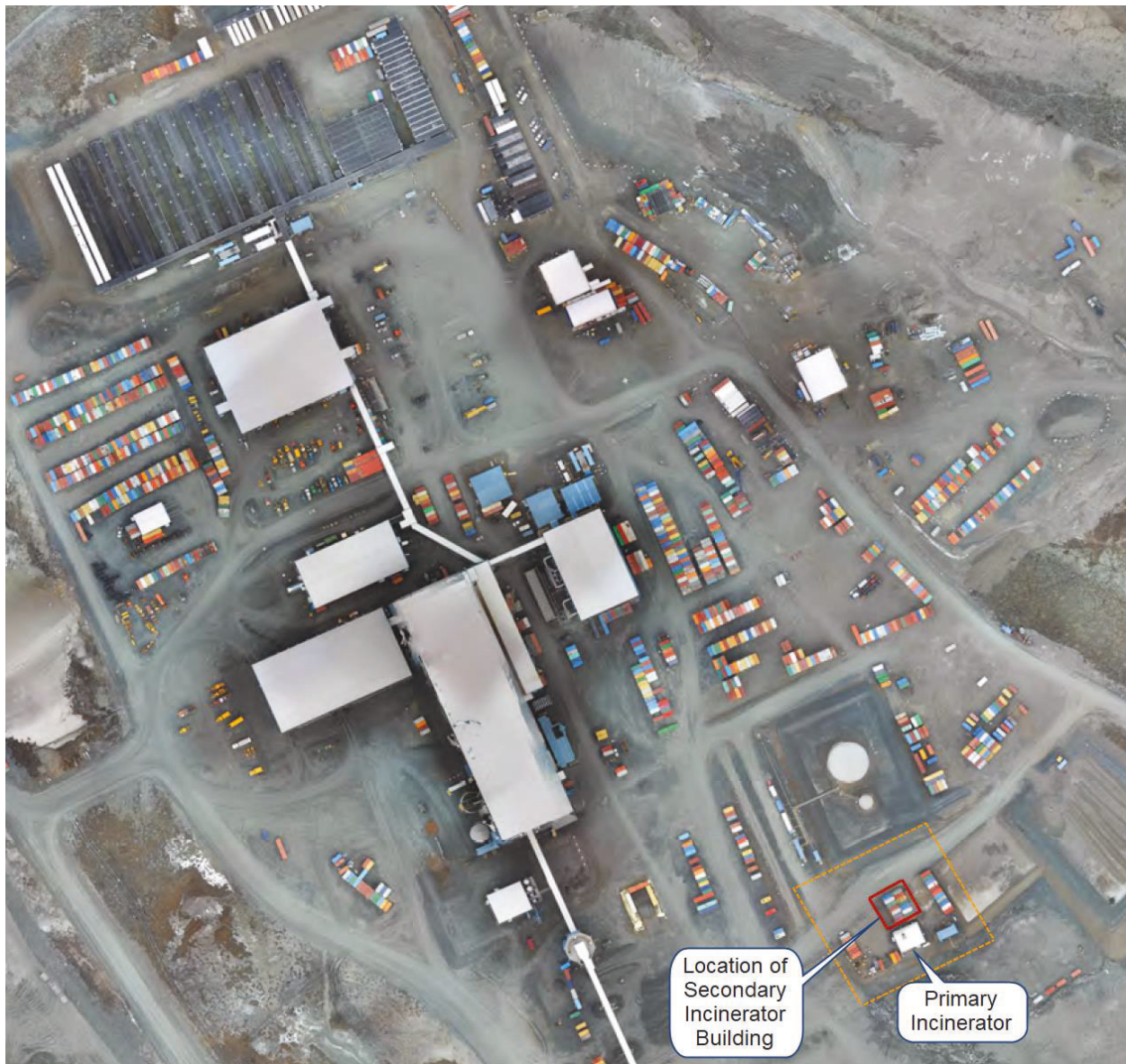
Figure 1 Site View – Location of Secondary Meliadine Incinerator
