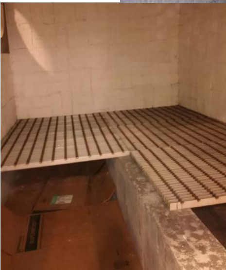
Floor and grate detail
