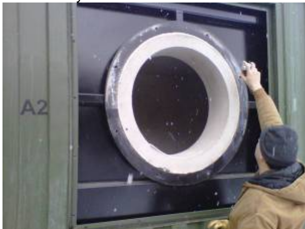
Gasket adhesive spray being applied
