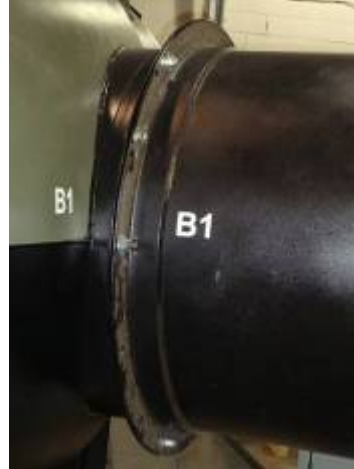
Correctly installed Breech on Secondary Chamber
