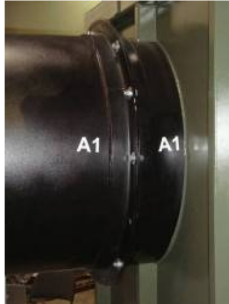
Correctly Installed Breech on Primary Chamber
