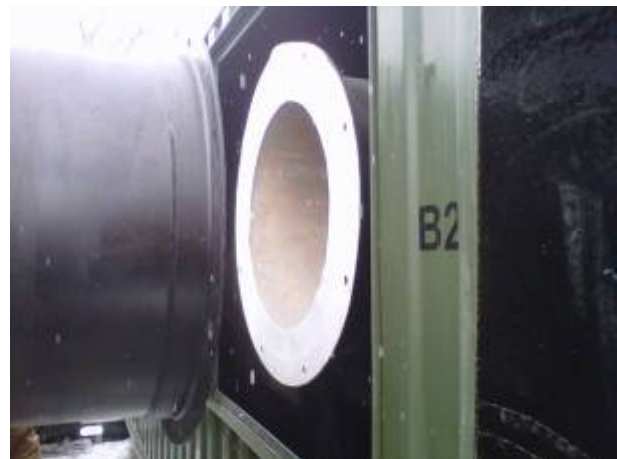
Correctly Installed Gasket
