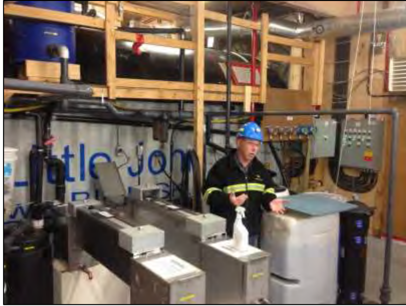
Photo 9: Wastewater treatment system – ultraviolet stage
