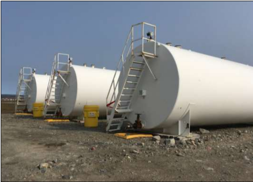
Figure 15. Temporary fuel farm at the main mine site. No secondary containment was evident here.
