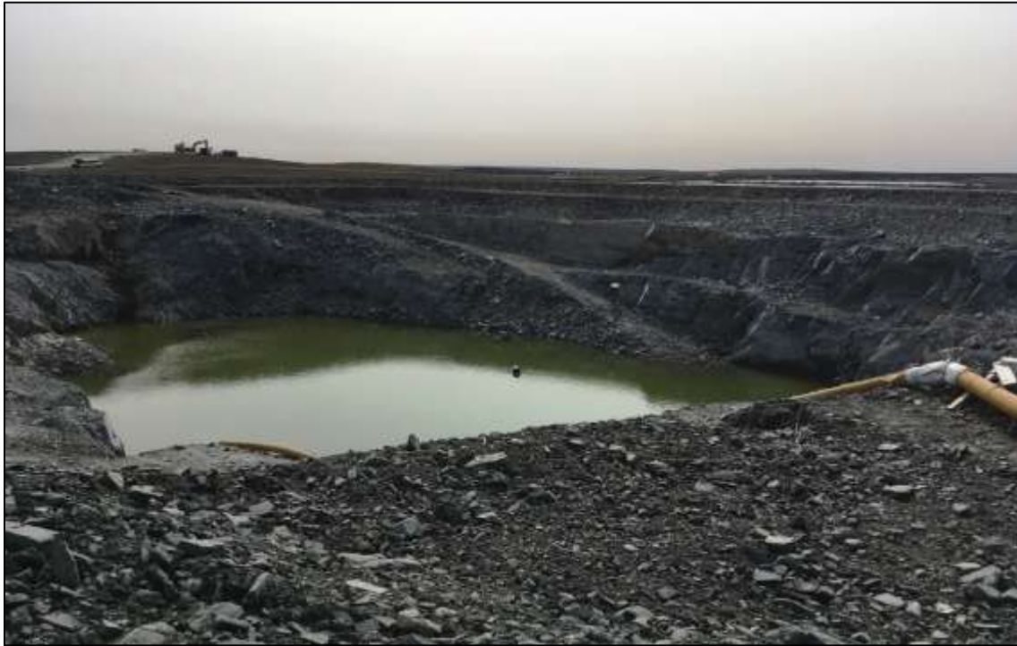
Figure 11. Saline water pond, which temporarily stores saline water from underground operations the Meliadine Gold Mine Project.
