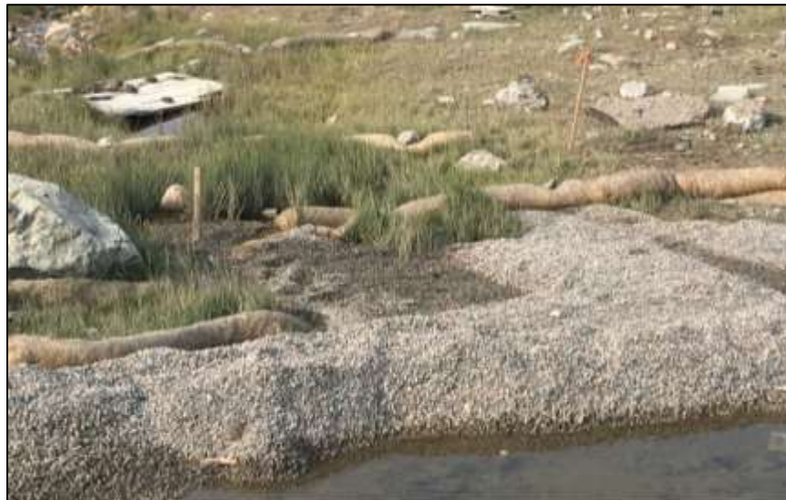
Figure 5. Saw logs and gravel berm used to control sediment loading to the terrestrial environment during freshet.
