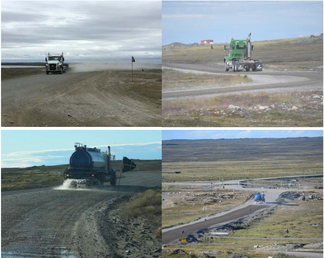
Figure 1: Assessment of the effectiveness of dust suppression. Top left – untreated road and fugitive dust, bottom left, bottom right – application of the dust suppressant, top right – after the application of the dust suppressant.
