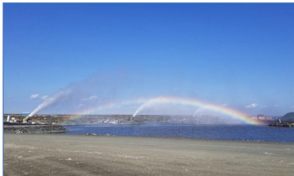
Photo 12. Three (3) evaporators used at a containment pond to maintain capacity within the main camp.
