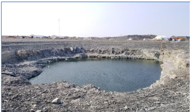
Photo 11. Saline water pond, which stores saline water from underground operations at the Meliadine Gold Mine Project.
