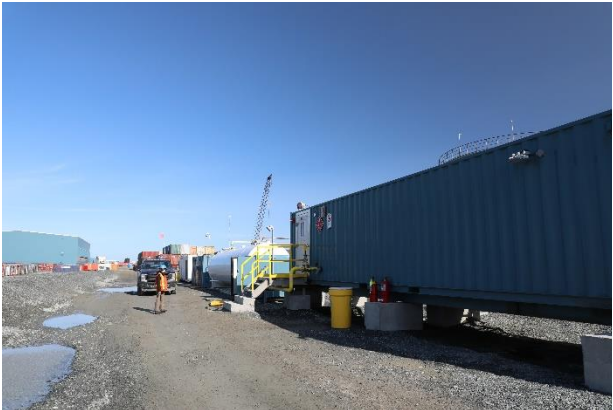
Photo 21. Fuel Tank Farm #1 transfer station
