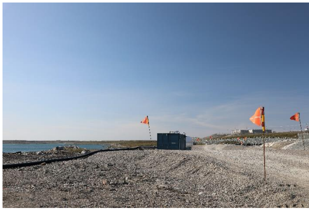
Photo 6: Saline Water Discharge tank
