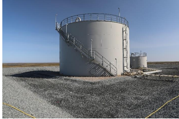
Photo 24. Fuel tank farm #2.
