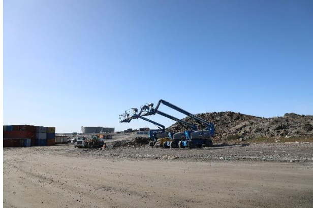
Photo 4. Equipment at the laydown area
