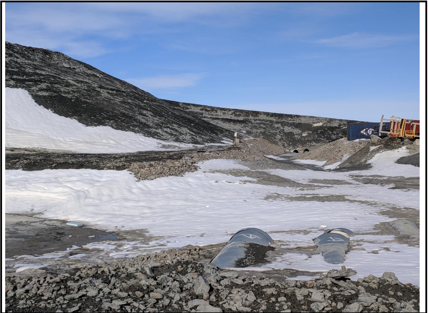
Picture 8: Culvert 2 not flowing – blocked by snow.
