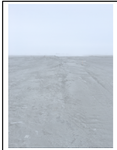
Photo 4: Line of uncompacted material between sub-cells 4/5 and the center cell; view facing north
