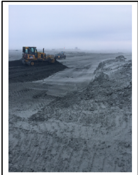
Photo 3: Pushing unfrozen tailings in the center cell; view facing southeast
