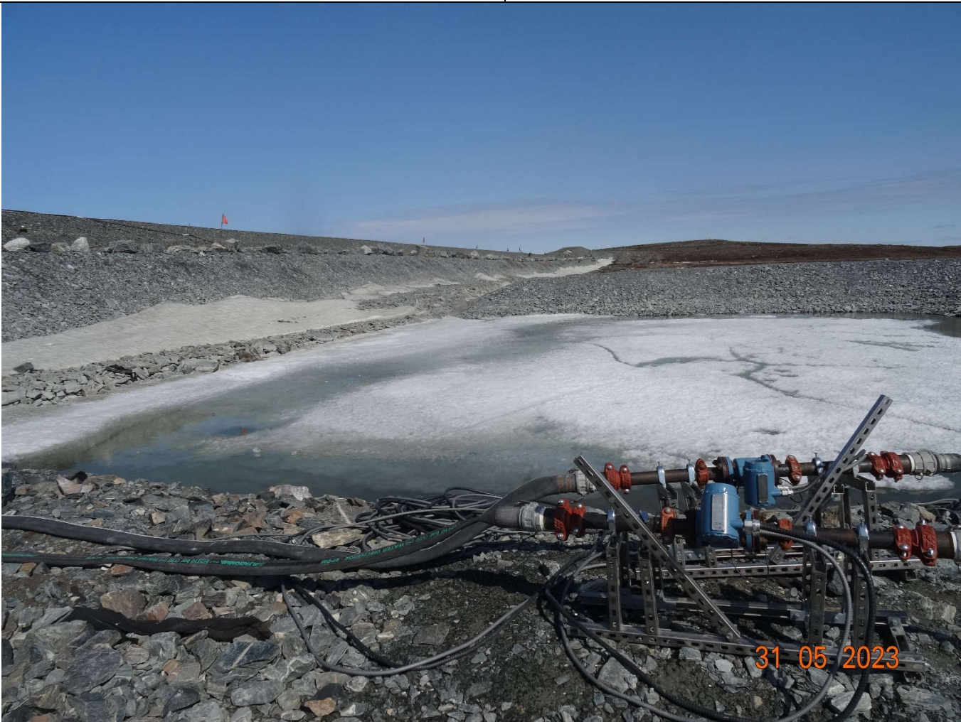
Description: Dyke for Containment Pond 1. Photo from toe of structure with sump in foreground.
