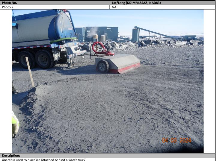
Aparatus used to place ice attached behind a water truck.
