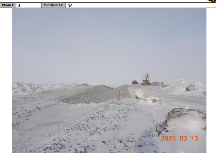
Channel 11 under construction. Flow is to background of photo to future CP9. Note that although this appears uphill surveyors are onsite and confirm correct direction of gradient.
