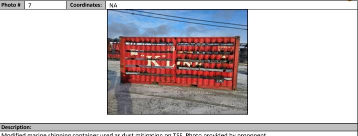
Modified marine shipping container used as dust mitigation on TSF. Photo provided by proponent.
