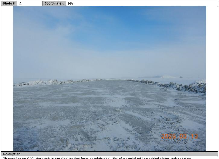
Thermal berm CP9. Note this is not final design form as additional lifts of material will be added along with capping.
