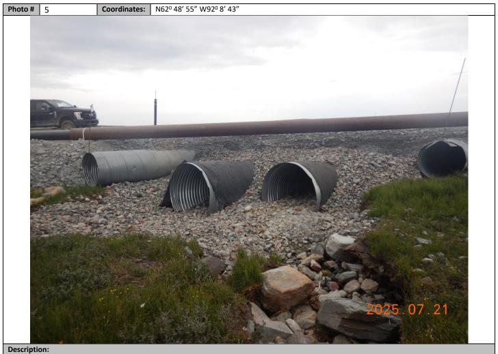
Culvert 11 on bypass road. Note clean gravel was used in construction to minimize sedimentation with new infrastructure and no markers were used. Culvert markers aid heavy equipment operators from damaging infrastructure during freshet preparation.
