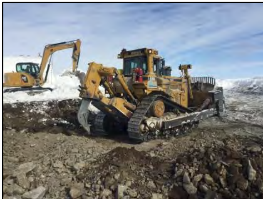
April 15: Using D9 dozer with ripper and 308 excavator for remediation efforts.
