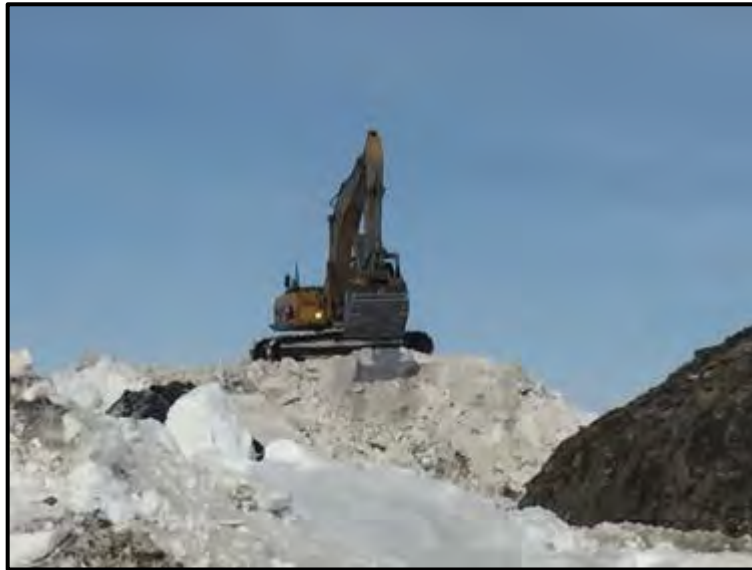
April 16: Excavator leveling snow pile in preparation for liner.
