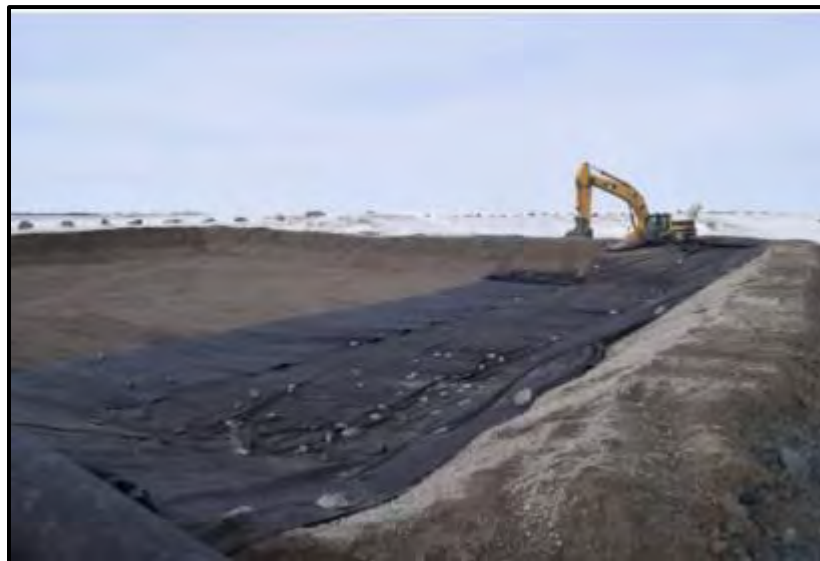
May 6: Installing liner at P1 cell.
