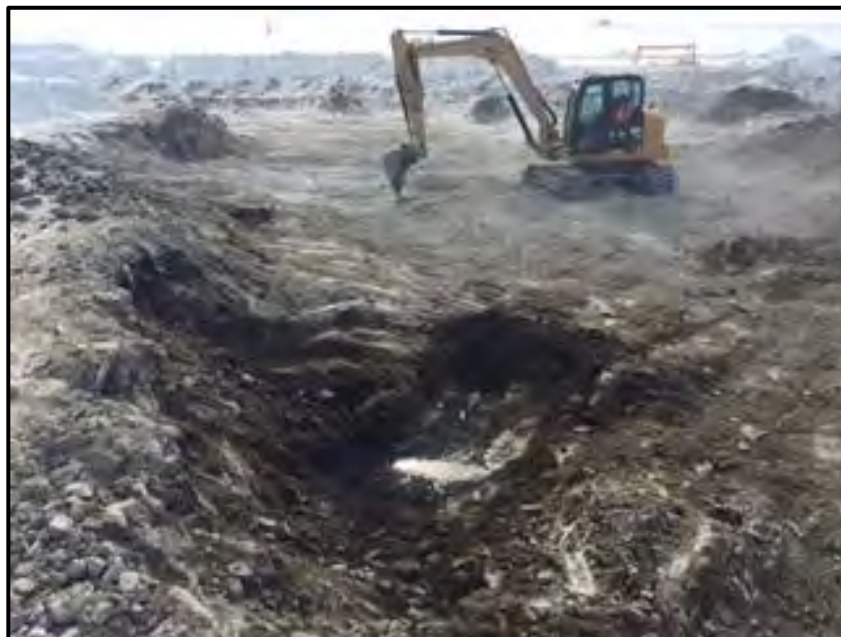
April 16: Free product accumulating in a small bellhole on the north side of the south excavation in the former tank 18 area.
