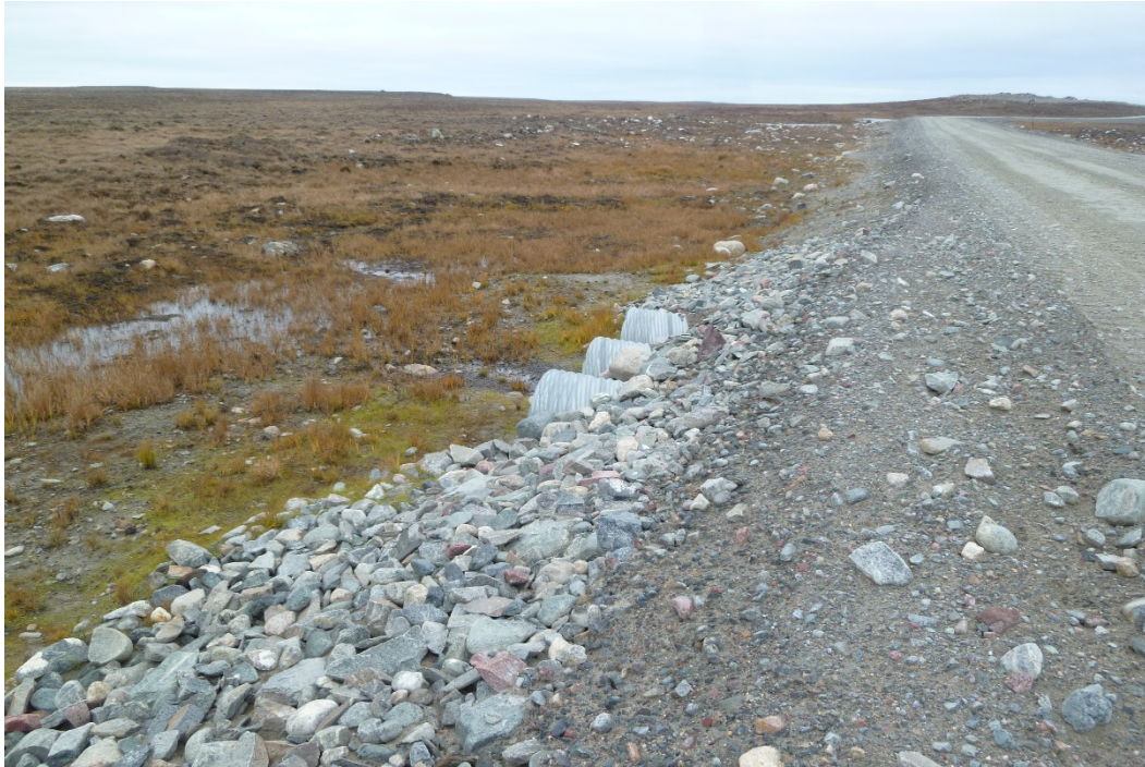
Photograph 37: 3x700mm Ø CSP at KM26.5. Upstream Ends of the Culverts (20 September 2017)
