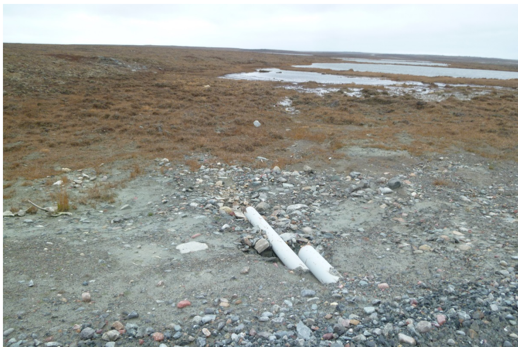
Photograph 42: 2 vertically Offset 160 mm Ø Steel Pipes, Looking Downstream at Outlet of the Steel Pipes, At KM26.8 (20 September 2017)
