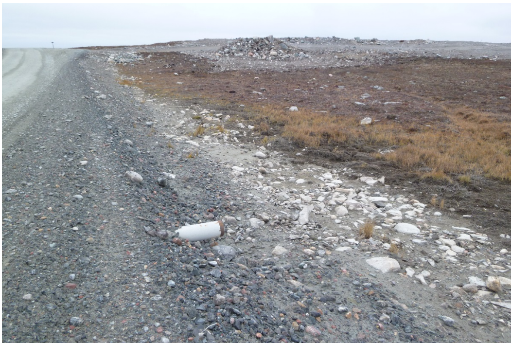
Photograph 40: 2 Vertically Offset 160mm Ø Steel Pipes, Clear, no Flow, Upstream View – at KM26.8 (20 September 2017)
