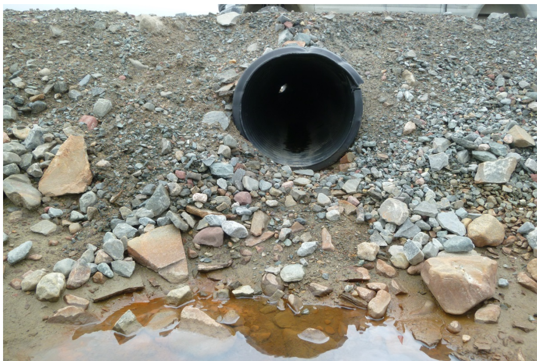
Photograph 52: 500 mm Ø HDPE Corrugated Culvert, View Through Culvert from Downstream to Upstream, Clear, No Flow, Some Dents of Side Wall at KM29.6 (22 September 2017)
