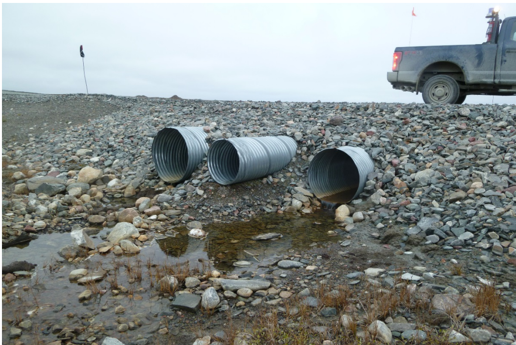
Photograph 46: Downstream Ends Of 3 CSP Culverts, Left to Right: 1000 mm, 700 mm, 900 mm \varnothing at KM27.1 (20 September 2017)
