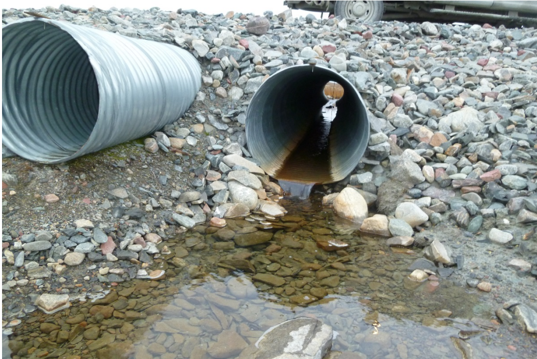
Photograph 45: Photo through the 900mm \varnothing culvert from Downstream to Upstream, Small Flow – KM27.1 (20 September 2017)
