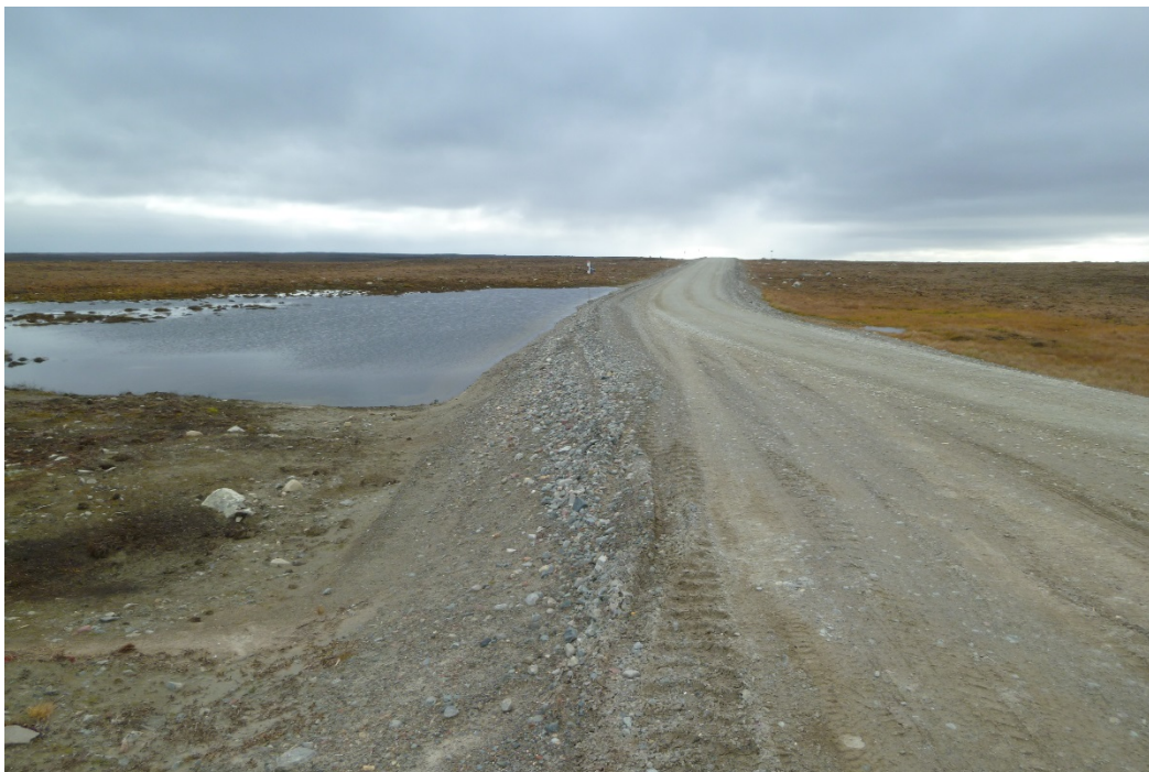
Photograph 48: KM28.7, Water Ponded on East Side of Road. AEM Reports that the Road is Wet for Most of the Open Water Season in this Area, Indicating Seepage through the Road. (22 September 2017)
