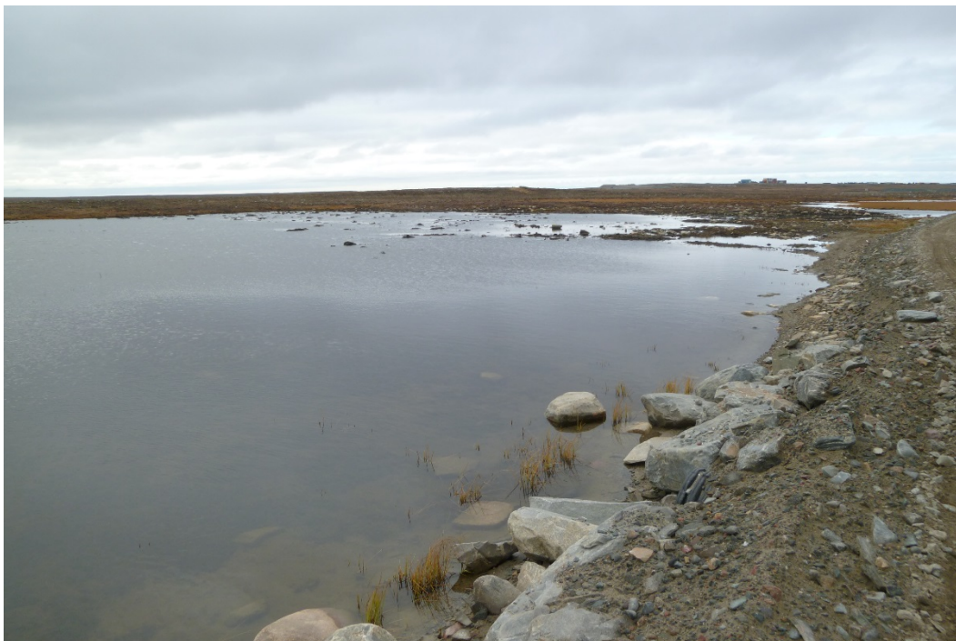
Photograph 50: Water Ponded on West Side of Road Upstream Of 500 mm Ø Corrugated HDPE Culvert at KM29.6, Looking North (22 September 2017)
