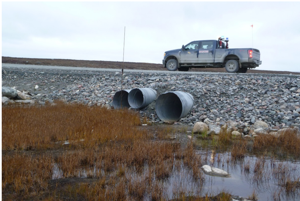
Photograph 44: Upstream Ends of Three Culverts at KM27.1. From left to right, 1000 mm, 700 mm, and 900 mm Ø CSP (20 September 2017)
