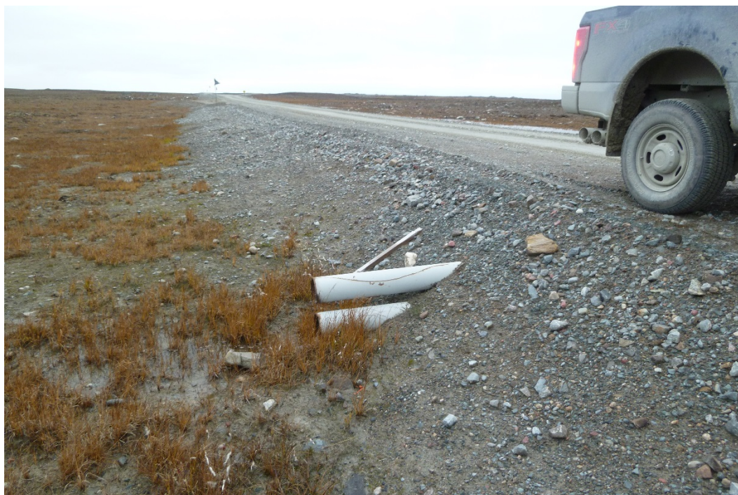
Photograph 34: Two Vertically Offset, 160 mm Ø steel pipes. Downstream Ends of the Pipes, at KM26.2 (20 September 2017)
