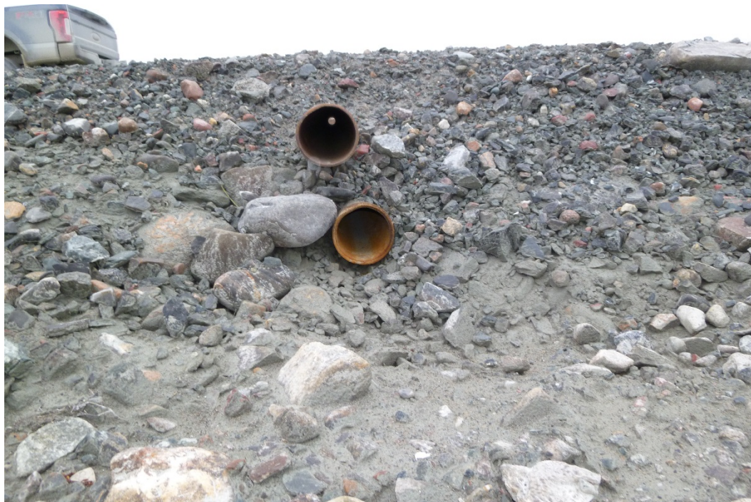
Photograph 41: 2 Vertically Offset 160 mm Ø Steel Pipes, Looking from Upstream to Downstream at Inlet of The Steel Pipes, At KM26.8. Pipes Showing More Oxidation Since 2016 Inspection (20 September 2017)
