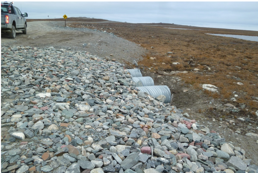
Photograph 38: 3x700mm Ø CSP at KM26.5. Downstream Ends of the Culverts (20 September 2017)
