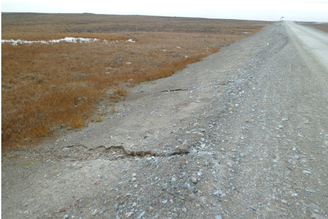
Photograph 32: Erosion of Road Embankment Near 600mm Ø HDPE culvert at KM25.8 (22 September 2017)
