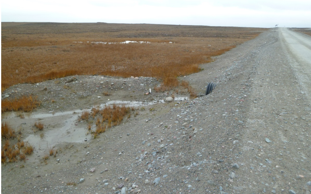
Photograph 31: Downstream end of 600 mm Ø HDPE Culvert at KM25.8. Some Sediment Erosion and Deposition Evident (22 September 2017)
