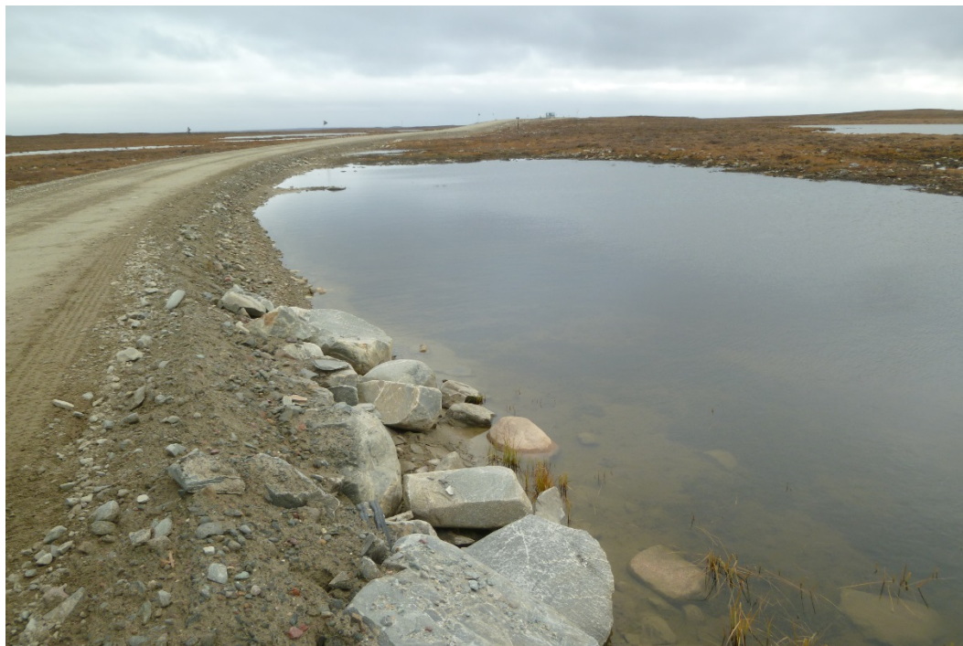
Photograph 51: 500mm Ø HDPE Corrugated Culvert Upstream Inlet (Between Rocks), At KM29.6, Looking South (22 September 2017)
