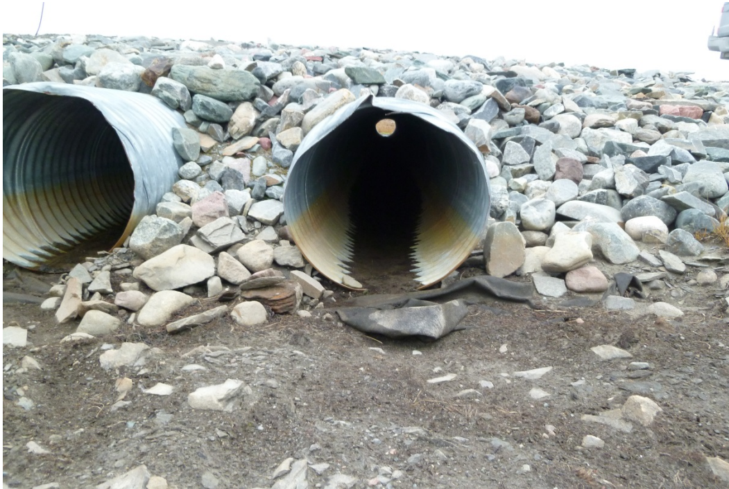
Photograph 39: 3x700mm Ø CSP at KM26.5. This Photo Showing the Inside of the North Culvert from Downstream Looking Upstream (20 September 2017)
