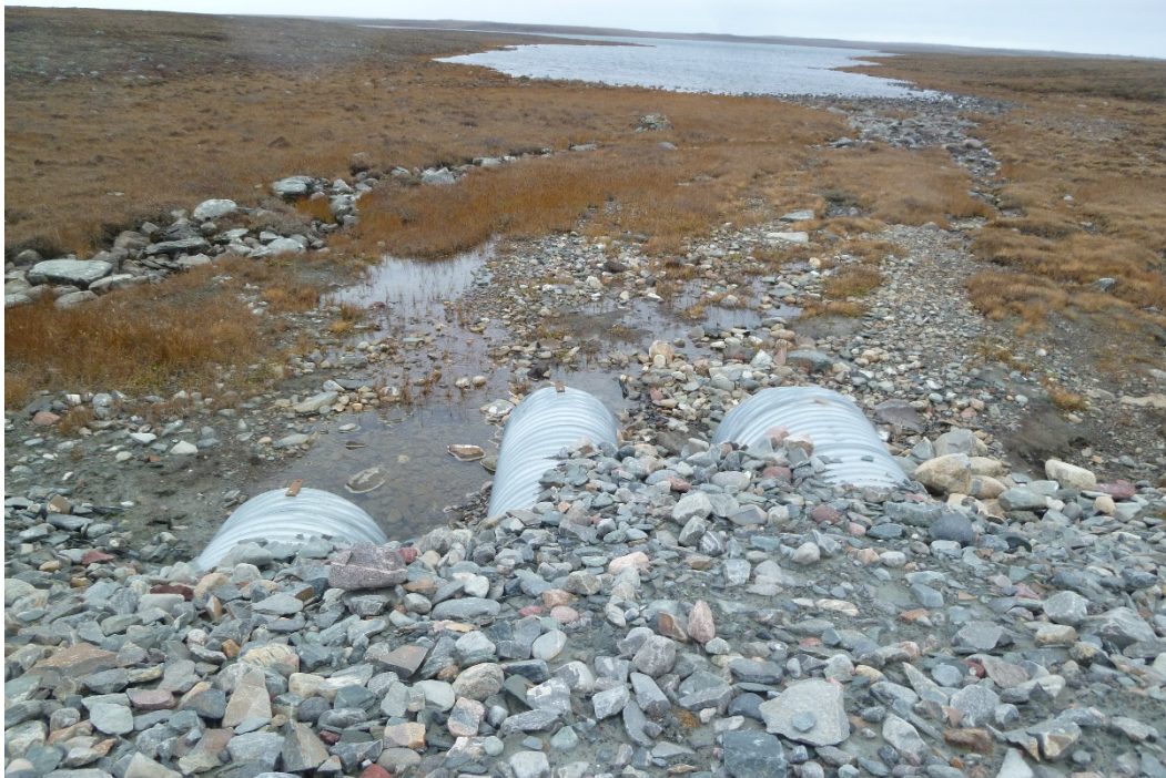
Photograph 47: Looking Downstream At 3 CSP, Left to Right: 900 mm, 700 mm, 1000 mm Ø at KM27.1 (20 September 2017)
