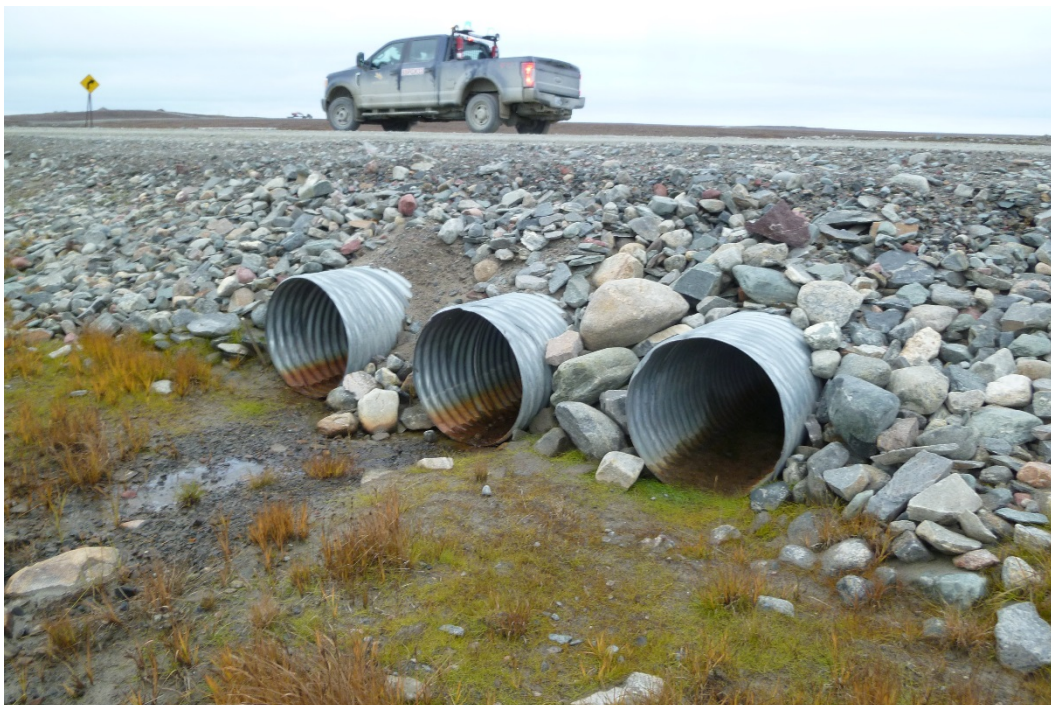
Photograph 36: 3x700mm Ø CSP at KM26.5. Inverts from Upstream Side (20 September 2017)
