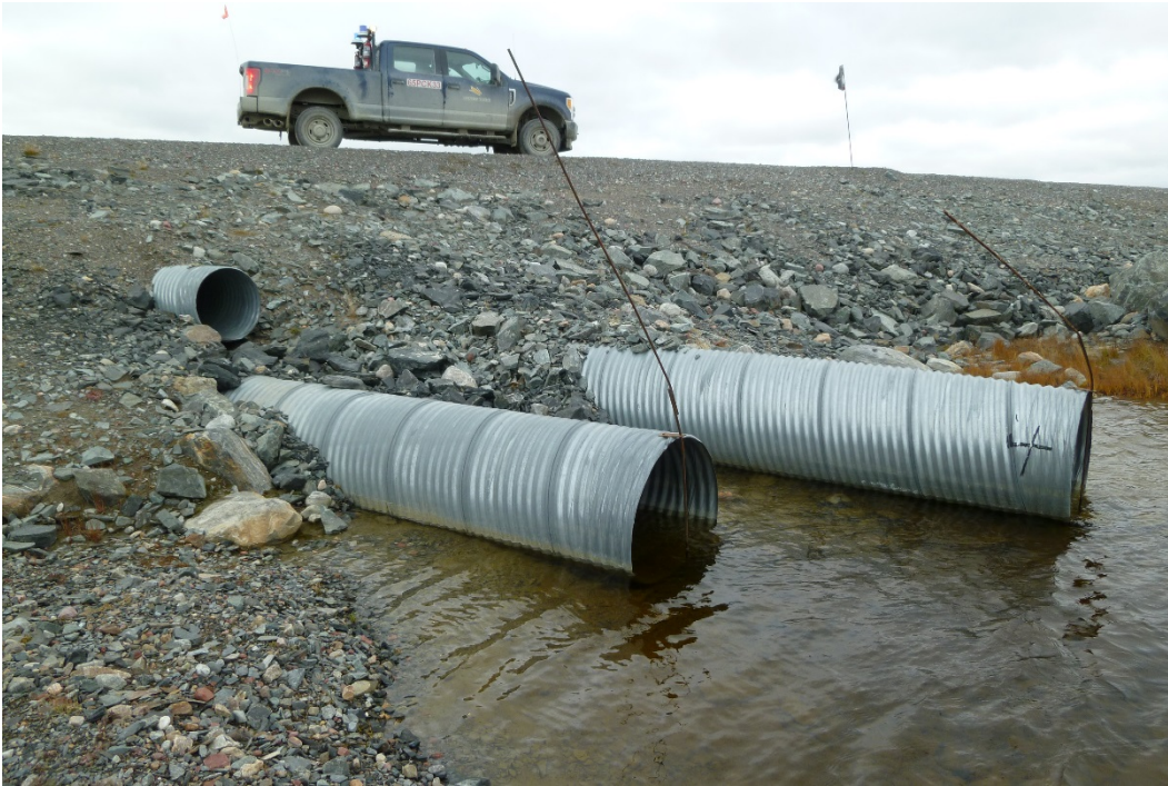
Photograph 79: Downstream Ends of 3 CSP Culverts at KM7.4. Middle, (700 mm Diameter) Culvert Should be Extended and Additional Armouring Added to Reduce Erosion Potential (20 September 2017)
