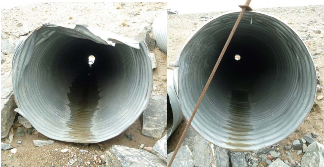
Photograph 75 And 76: At KM7.4, Upstream to Downstream View Through Damaged 900 mm Diameter Culvert Inlet, Likely Crushed by Rocks (On Left). Upstream to Downstream View Through 700 mm Diameter Culvert (on right) (20 September 2017)
