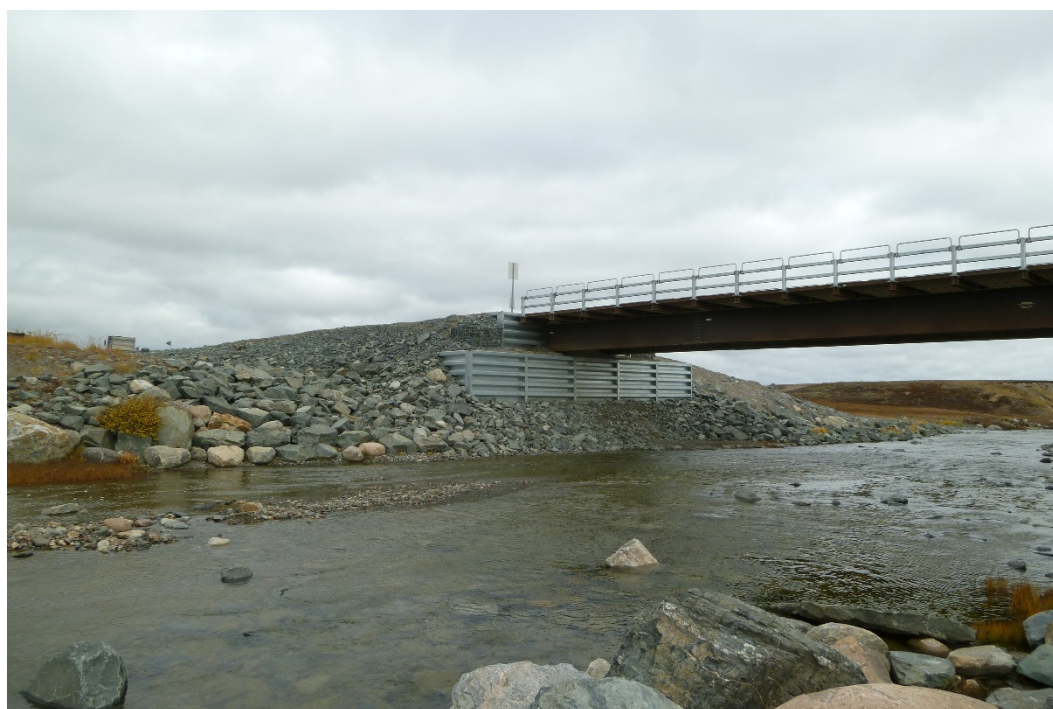
Photograph 55: Char River Bridge, Left (north) Abutment Armouring from the Upstream Side (20 September 2017)
