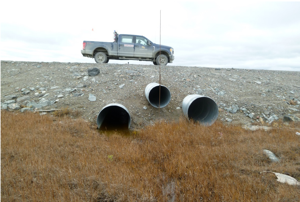
Photograph 69: Downstream Ends of 3 CSP Culverts at KM7.0 (20 September 2017)
