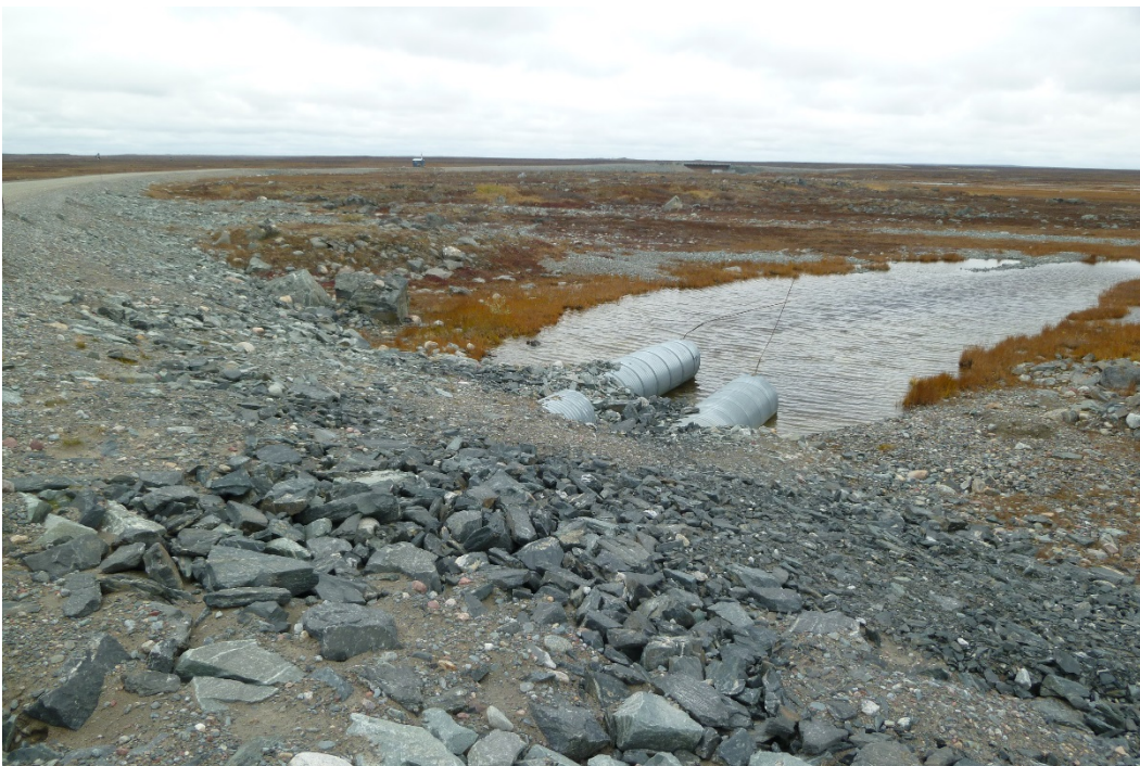
Photograph 78: At KM7.4, Looking at Downstream Ends of 3 CSP Culverts (20 September 2017)
