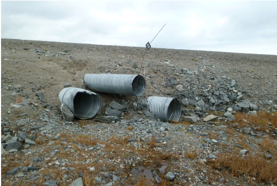
Photograph 74: At KM7.4, Upstream Ends of 3 CSP Culverts. Culvert Diameters are from Right to Left, 1000 mm, 700 mm, and 900 mm. Inlet of the 900 mm has been Partially Crushed (20 September 2017)
