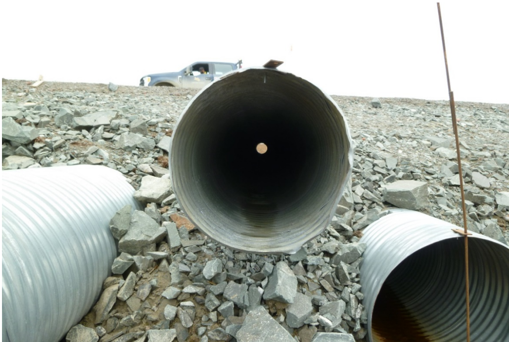
Photograph 71: Upstream to Downstream View Through 700 mm Diameter CSP Culvert at KM7.1 (20 September 2017)
