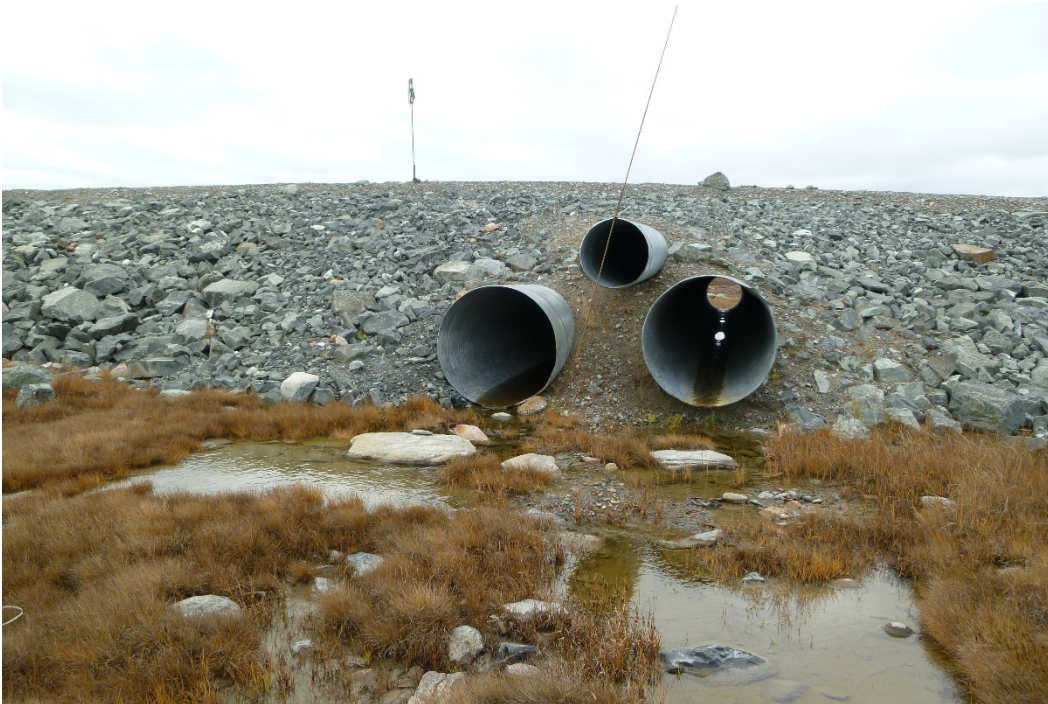
Photograph 63: Downstream Ends of 3 CSP Culverts at KM6.2 (20 September 2017)
