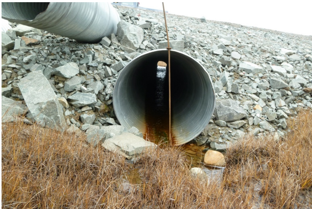
Photograph 72: Upstream to Downstream View Through Right 1000 mm Diameter CSP Culvert at KM7.1 (20 September 2017)
