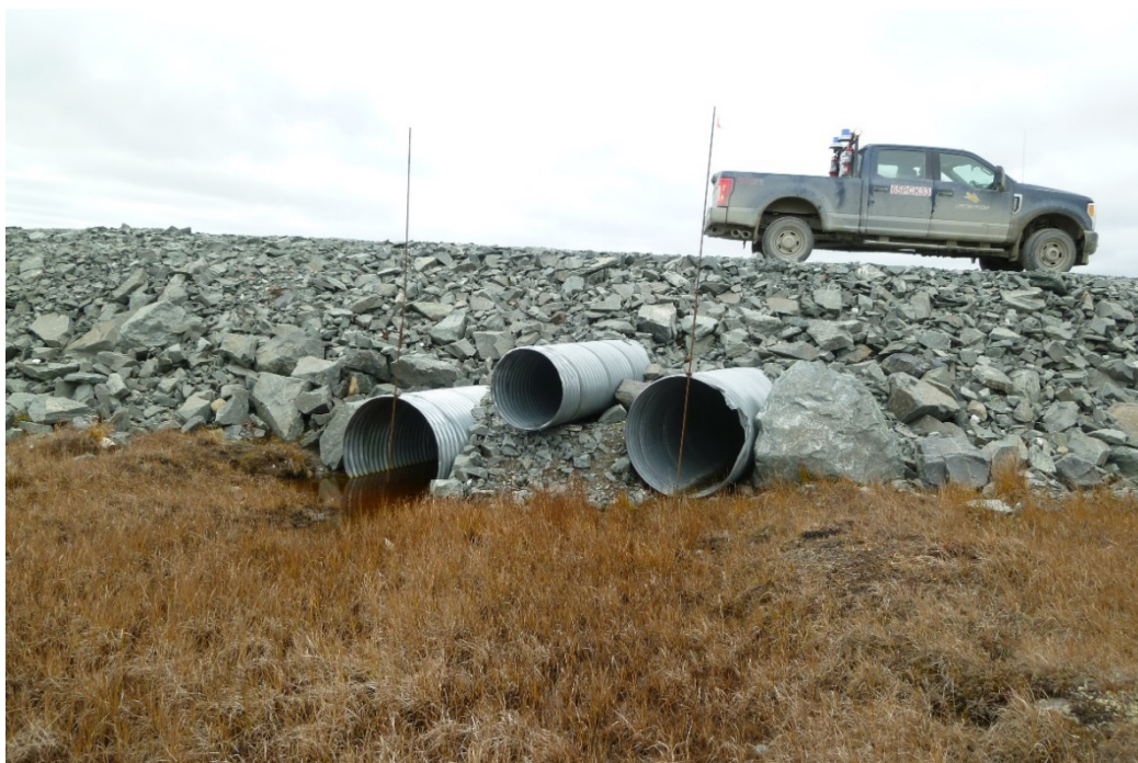
Photograph 73: Downstream Ends of 3 CSP Culverts at KM7.1 (20 September 2017)
