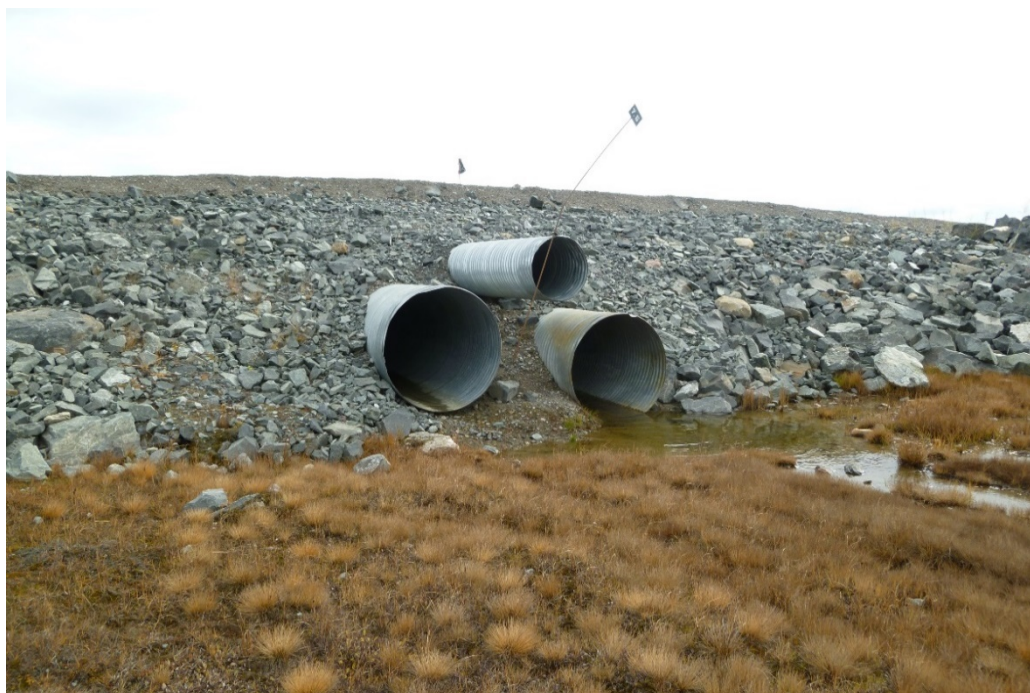
Photograph 59: At KM6.2, Upstream Ends Of 3 CSP Culverts. Lower Two Culverts Are 1300 mm in Diameter, Upper Culvert Is 700 mm in Diameter. All are in Good Condition (20 September 2017)
