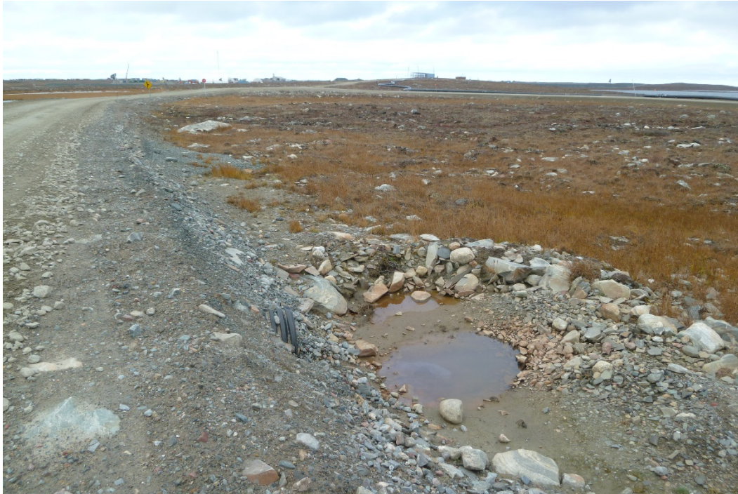
Photograph 53: 500 mm Ø HDPE Corrugated Culvert, Downstream Inlet of Culvert at KM29.6. Small Erosion Evident Upstream (22 September 2017)
