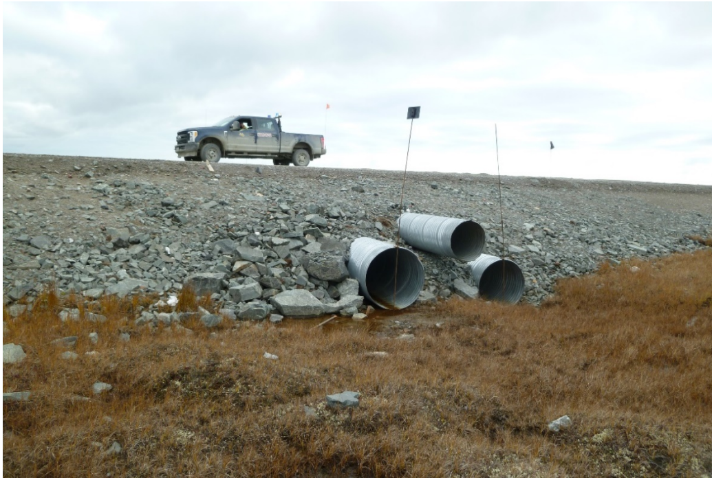
Photograph 70: At KM7.1, Upstream Ends of 3 CSP Culverts. Lower Two Culverts are 1000 mm in Diameter and Upper Culvert Is 700 mm in Diameter. Small Flow Through Culvert on the Right Hand Side, at Time of Inspection, Some Dents in 700 mm (20 September 2017)
