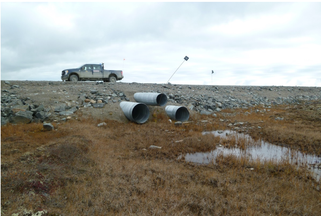
Photograph 65: At KM7.0, Upstream Ends of 3 CSP Culverts. Vertically Offset. Lower Two Culverts are 1000 mm in Diameter and Upper Culvert is 700 mm in Diameter. Some Exposed Esker Sand, Additional Armouring should be Considered (20 September 2017)
