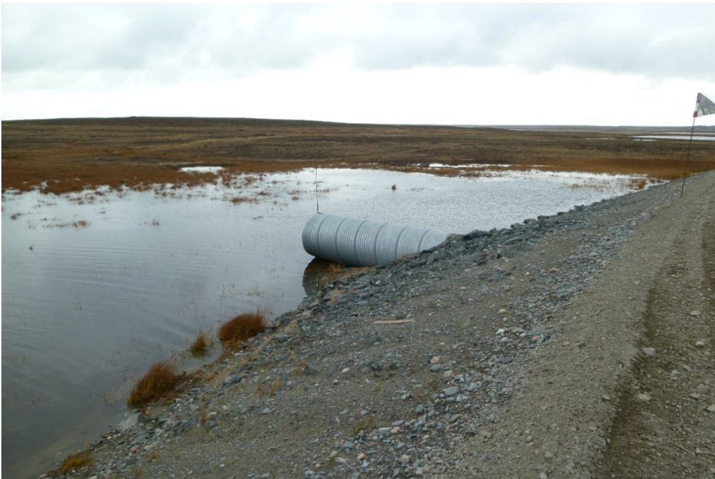
Photograph 96: Upstream End of a Single 1300 mm Diameter CSP Culvert at KM9.5. Good Condition, no Obstructions. Water Ponded on Upstream with very Low Flow Due to Elevated Inlet of CSP (20 September 2017)
