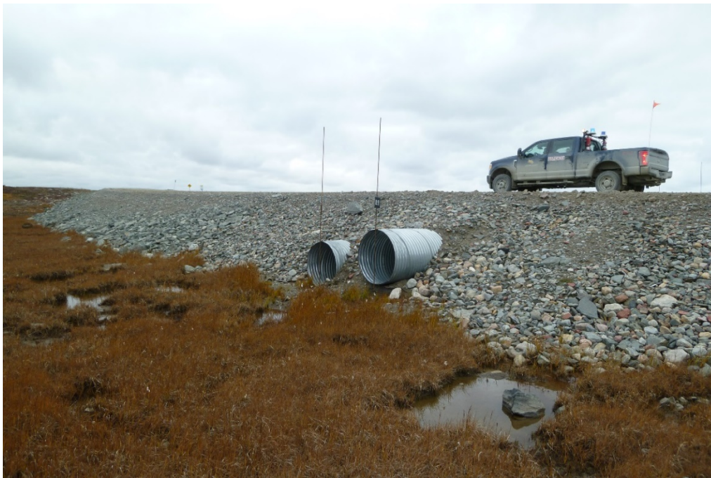
Photograph 90: Upstream Ends of Two 1000 mm Diameter CSP Culverts at KM9.1 Looking North (20 September 2017)
