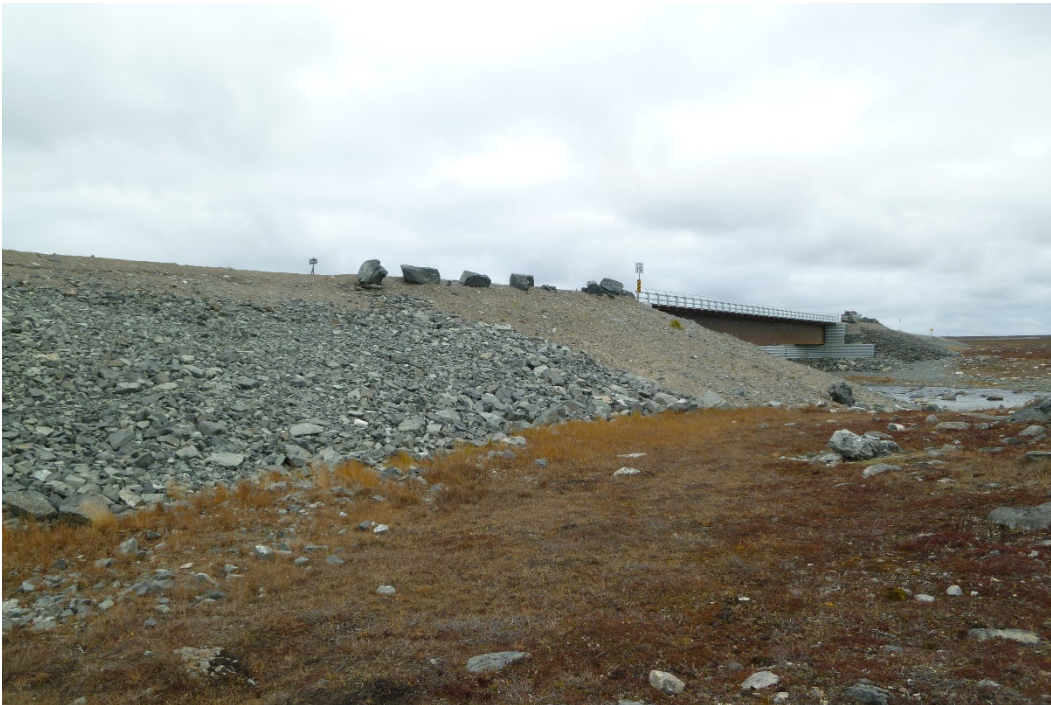
Photograph 88: Meliadine River Bridge at KM8.0. Slope of Right (South) Abutment, Esker Sand Exposed. Consider Adding Armouring with Coarser Grained Material to Reduce Erosion Potential (20 September 2017)
