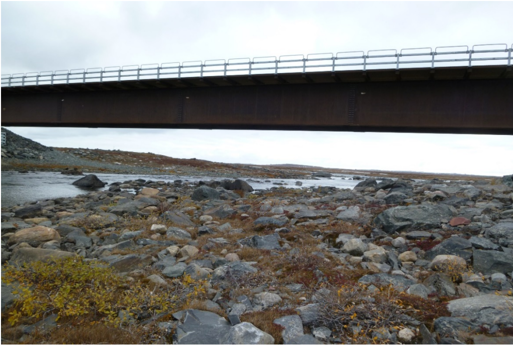
Photograph 89: Meliadine River Bridge View from Upstream to Downstream Beneath Bridge Deck. Low Flow at Time of Inspection Gravel and Cobble Bedding (20 September 2017)
