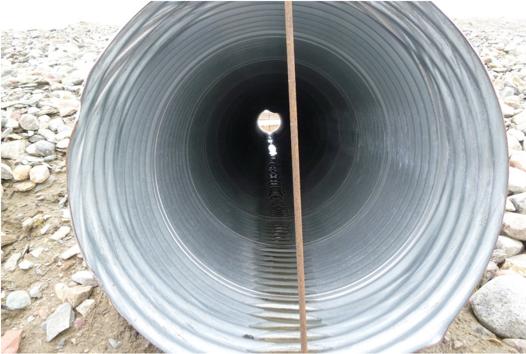
Photograph 91: View through North CSP Culvert at KM9.1 from Upstream to Downstream. Some Deformation of Culvert below Road (20 September 2017)
