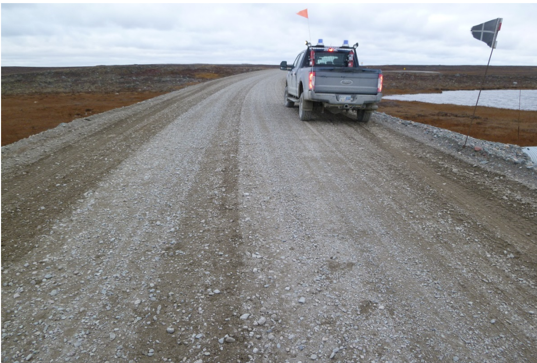
Photograph 94: Road Surface Over Two CSP Culverts at KM9.1 (20 September 2017)
