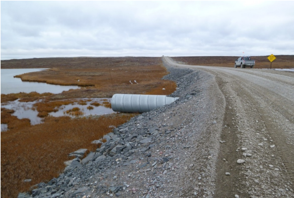
Photograph 97: Downstream End of a Single 1300 mm Diameter CSP Culvert at KM9.5 (20 September 2017)
