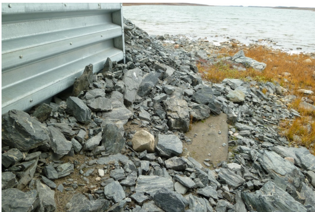
Photograph 1022: M-5 Bridge at KM10.5, Exposed Fabric on Downstream End of Left (North) Abutment Indicating Possible Erosion (20 September 2017)
