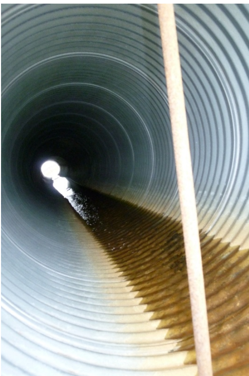
Photograph 98: KM9.5, Looking from Downstream to Upstream Through the 1300 mm Diameter Culvert (20 September 2017)
