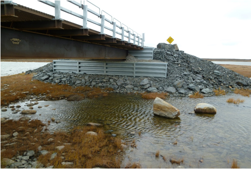
Photograph 103: M-5 Bridge at KM10.5 Right (South) Abutment, Upstream Side. Area of Possible Erosion or Settlement Identified During 2016 Inspection Shows no Signs of Change (20 September 2017)
