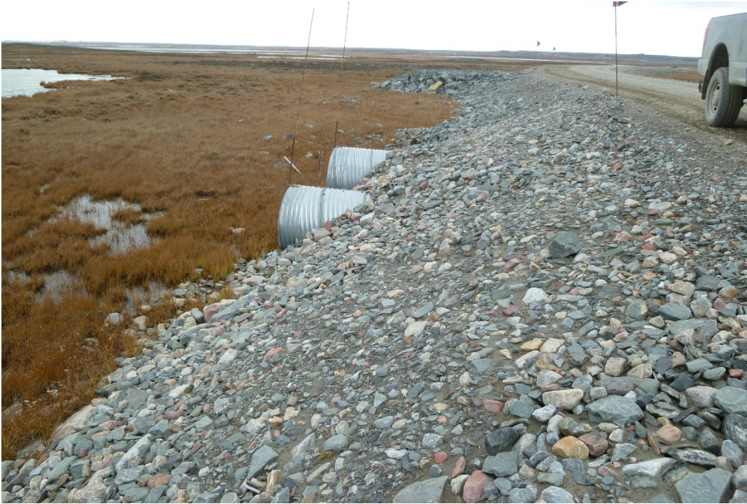
Photograph 93: Downstream Ends of Two CSP Culverts at KM9.1 (20 September 2017)
