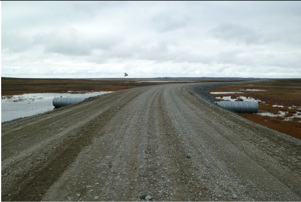
Photograph 95: Road Surface Over a Single 1300 mm Diameter CSP Culvert at KM9.5 (20 September 2017)
