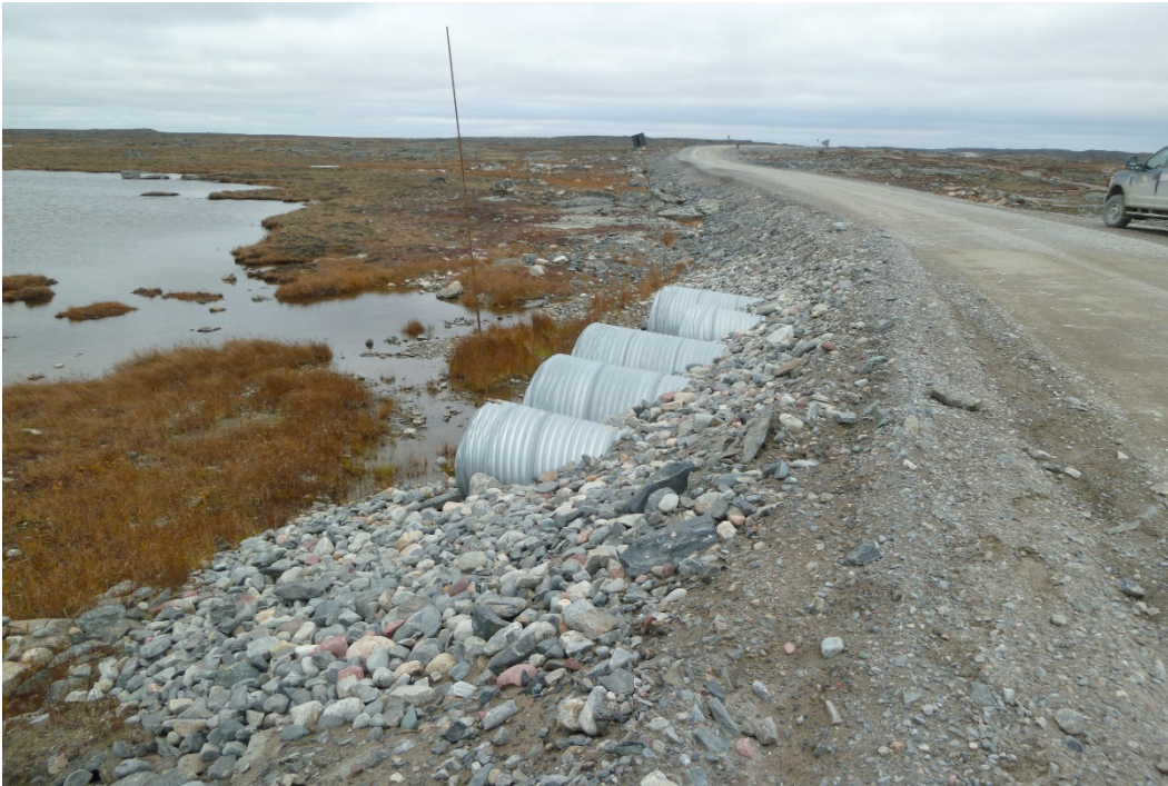
Photograph 119: Downstream View of 5 CSP Culverts at KM13.5 (20 September 2017)
