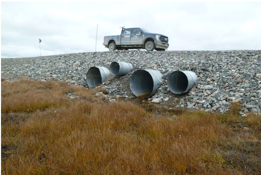
Photograph 108: Downstream Ends of Four CSP Culverts at KM12.1. From Left to Right Diameters are 1300 mm, 700 mm, 1300 mm, 900 mm (20 September 2017)
