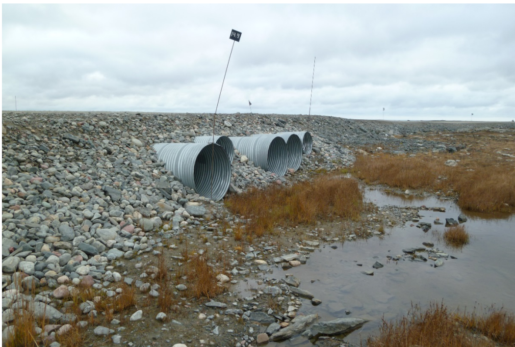
Photograph 118: At KM13.5, There are 5 CSP Culverts (3×1300 mm Ø; 2×900mm Ø). View of Upstream Ends of the Culverts. 900 mm Culverts are Vertically Elevated (20 September 2017)
