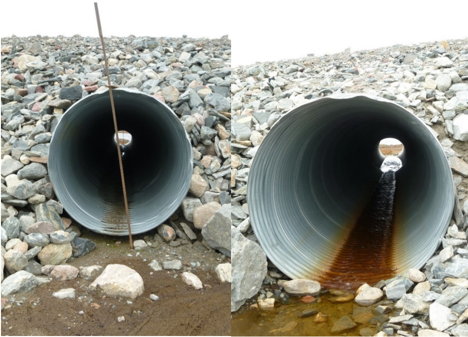
Photographs 111 and 112: Upstream to Downstream View Through Two Northern CSP Culverts at Km12.1. 900 mm Ø on Left and 1300 mm Ø On Right (20 September 2017)
