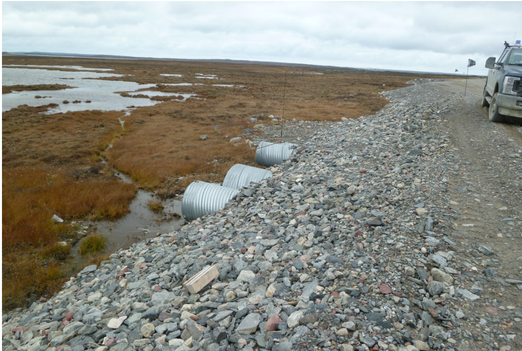
Photograph 107: Downstream Ends of Four CSP Culverts at KM12.1 (20 September 2017)
