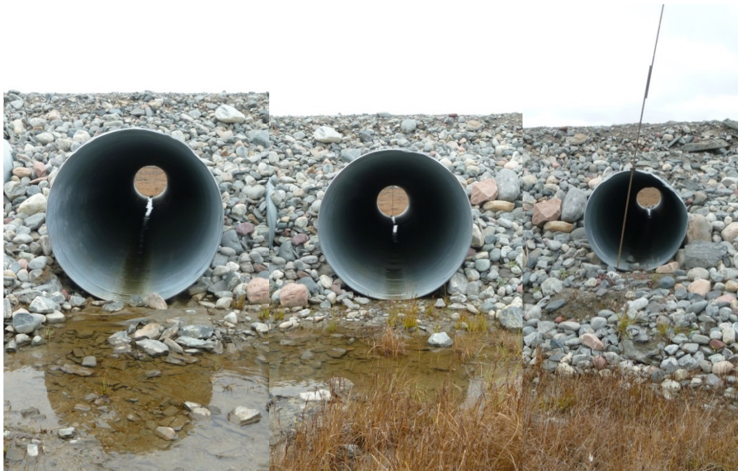
Photographs 122, 123 And 124: Upstream to Downstream Views Through Middle and South 1300 mm Ø CSP Culverts (Left and Middle Photographs Respectively) and South 900 mm Ø CSP Culvert (Right Photograph) Located at KM13.5 (20 September 2017)
