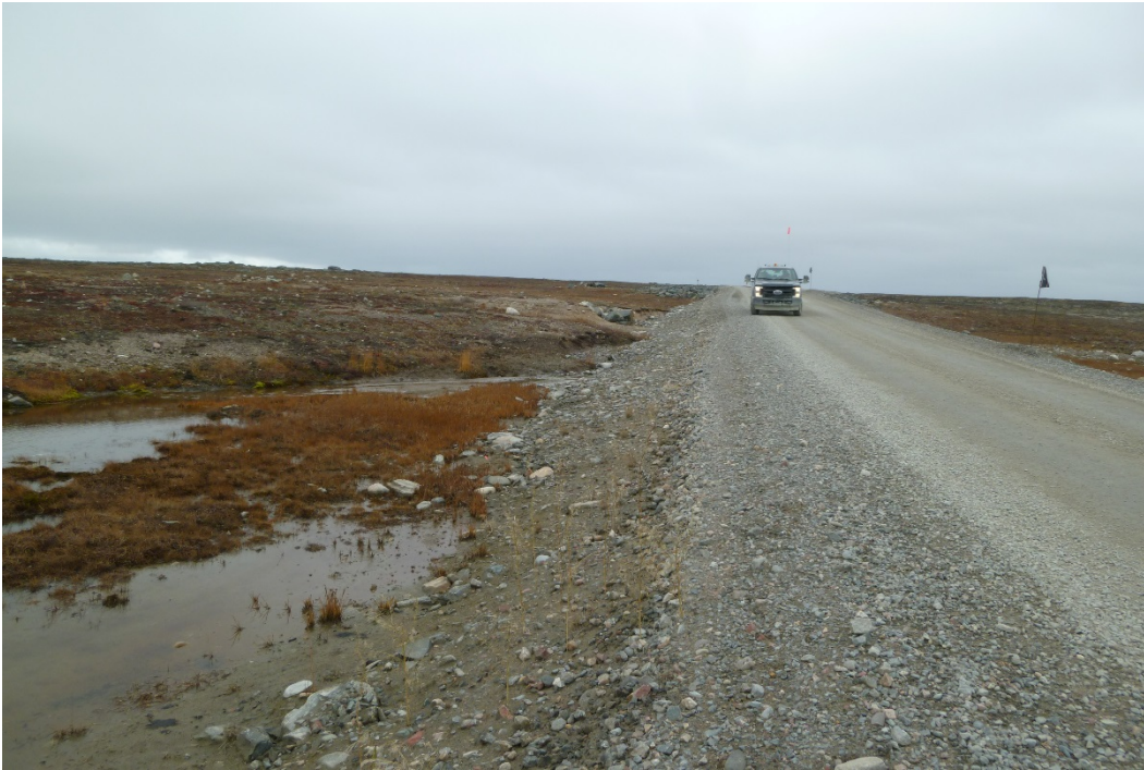
Photograph 117: KM 12.6, Ponded Water and Erosion of Road Embankment Evident (22 September 2017)
