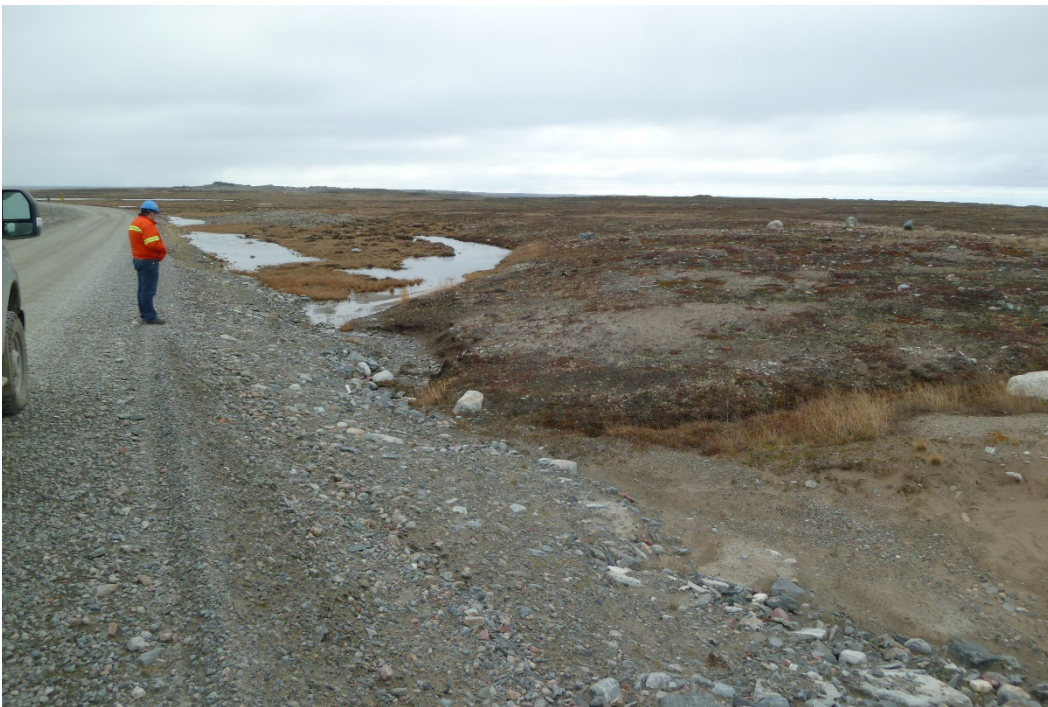
Photograph 116: KM 12.6, Ponded Water and Erosion of Toe Road Embankment Evident (22 September 2017)
