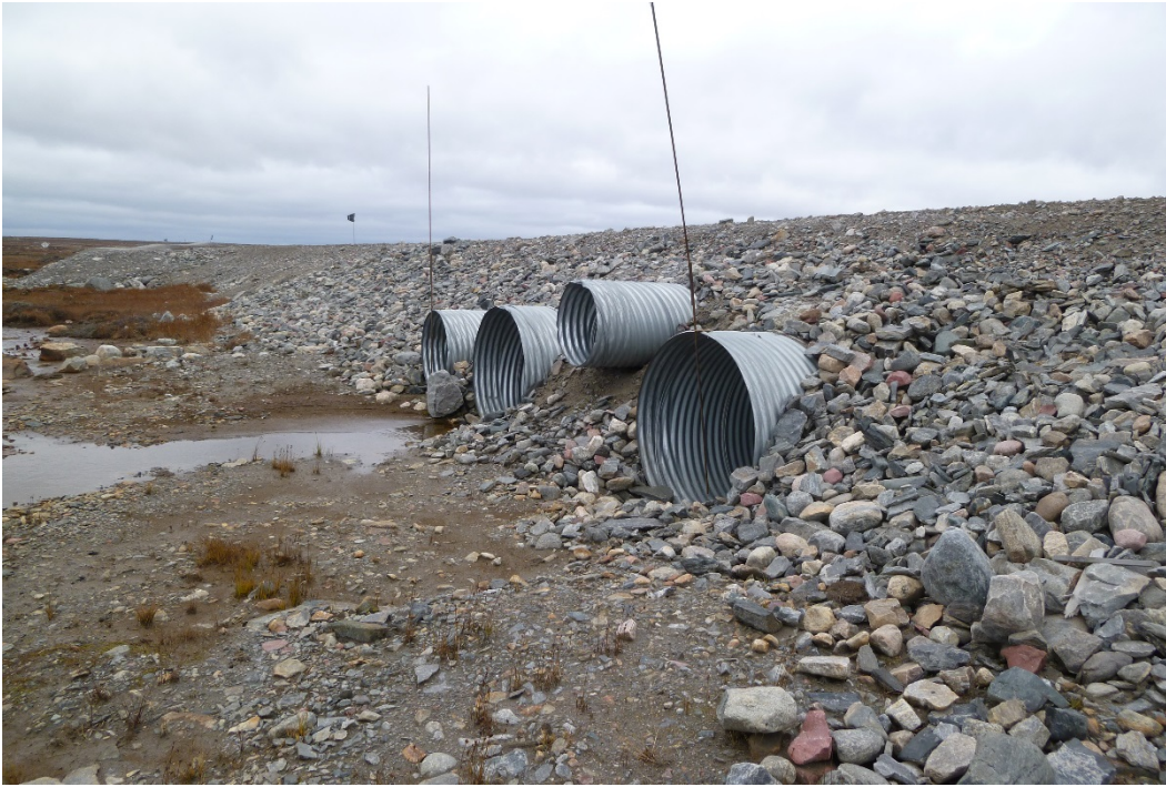
Photograph 109: Upstream Ends of Four CSP Culverts at KM12.1 (20 September 2017)
