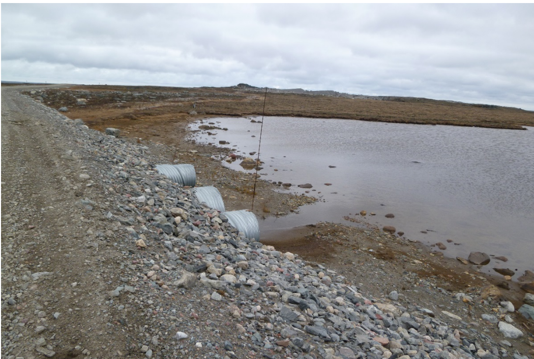
Photograph 110: Upstream Ends of Four CSP Culverts at KM12.1 (20 September 2017)
