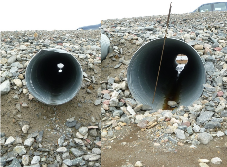
Photographs 113 and 114: Upstream to Downstream View Through Two Southern CSP Culverts at Km12.1. 700 mm Ø On Left and 1300 mm Ø On Right (20 September 2017)
