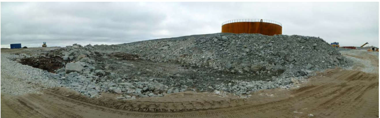
Photograph 5: Itivia Site, Looking North at South Corner of Tank #1 and #2 Containment Berm (22 September 2017)
