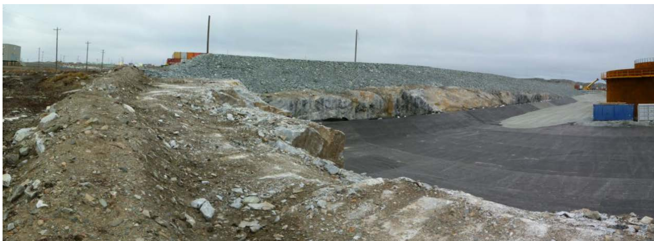
Photograph 7: Itivia Site, South Slope of Upper Pad and South Rock Cut Face, North of Tank #1 and #2 (22 September 2017)
