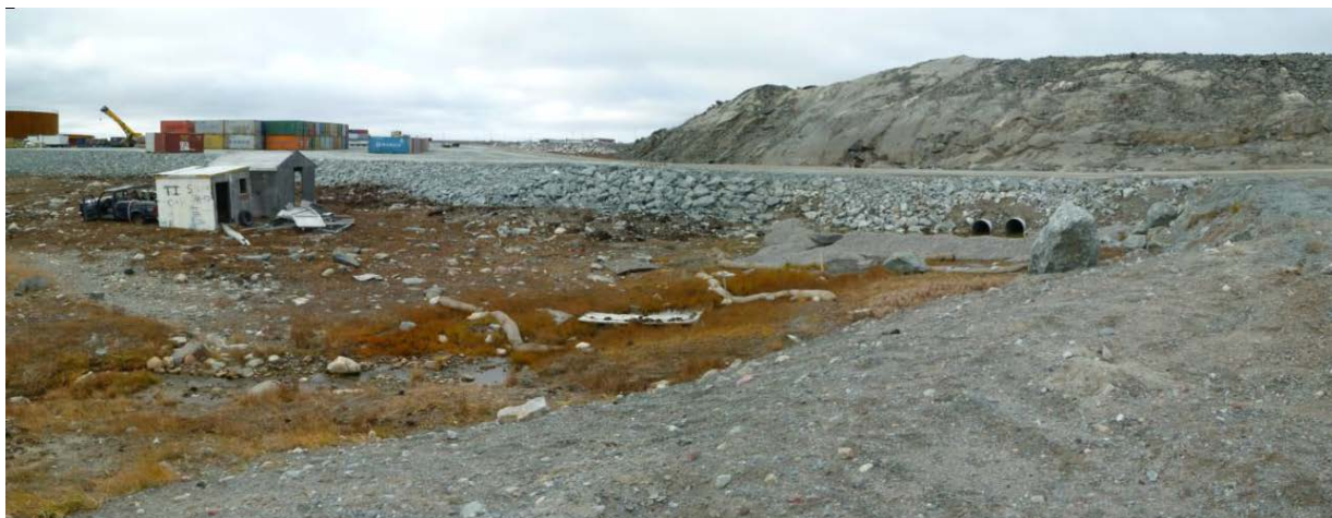
Photograph 14: Itivia Site, Access Road to Site with Culverts (22 September 2017)
