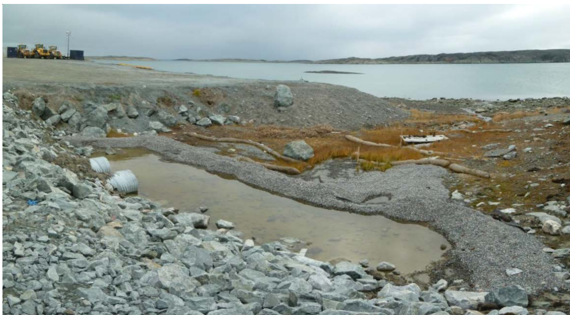
Photograph 15: Itivia Site, View Downstream from Culverts Through Access Road to Site (22 September 2017)
