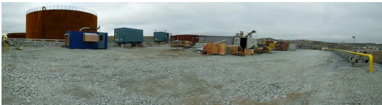
Photograph 9: Itivia Site, Area East of Tank #1 and #2, Looking North (22 September 2017)
