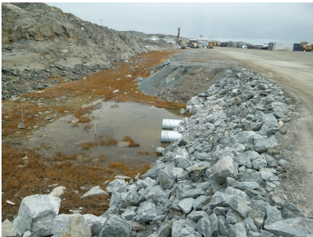
Photograph 13: Itivia Site, Upstream ends of Culverts Through Access Road (22 September 2017)
