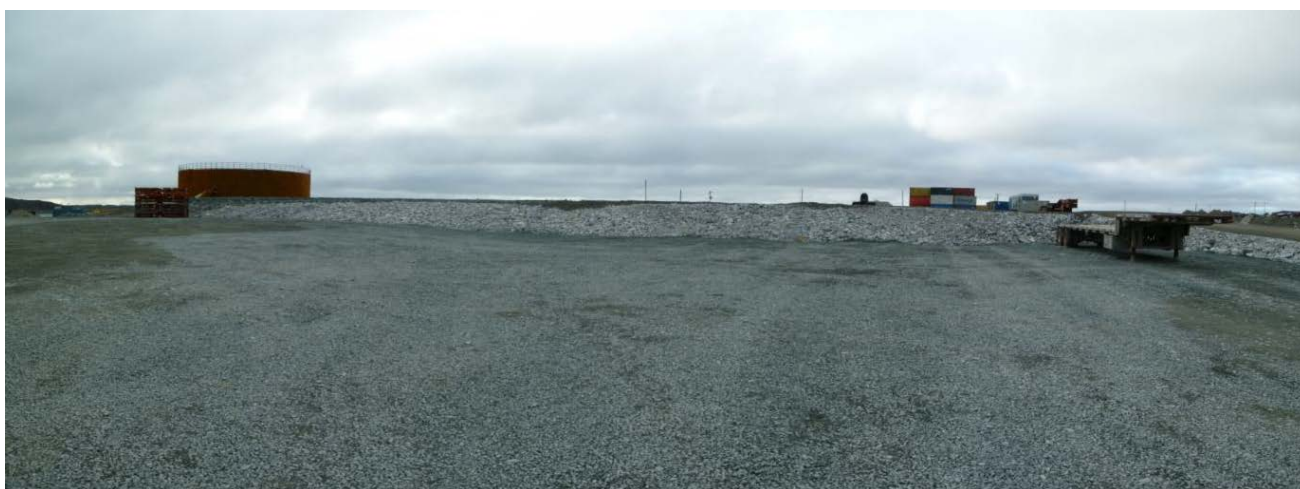
Photograph 10: Itivia Site, Upper East Pad Area, Looking Northwest (22 September 2017)
