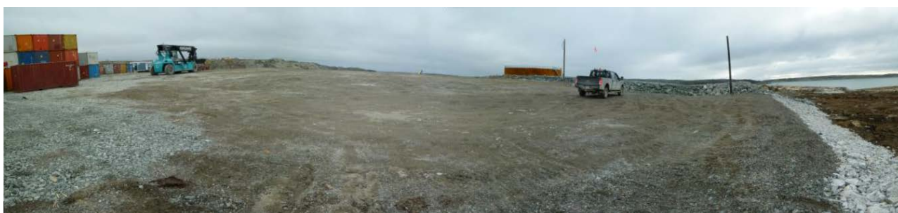
Photograph 11: Itivia Site, Upper North Pad Area, Looking South (22 September 2017)
