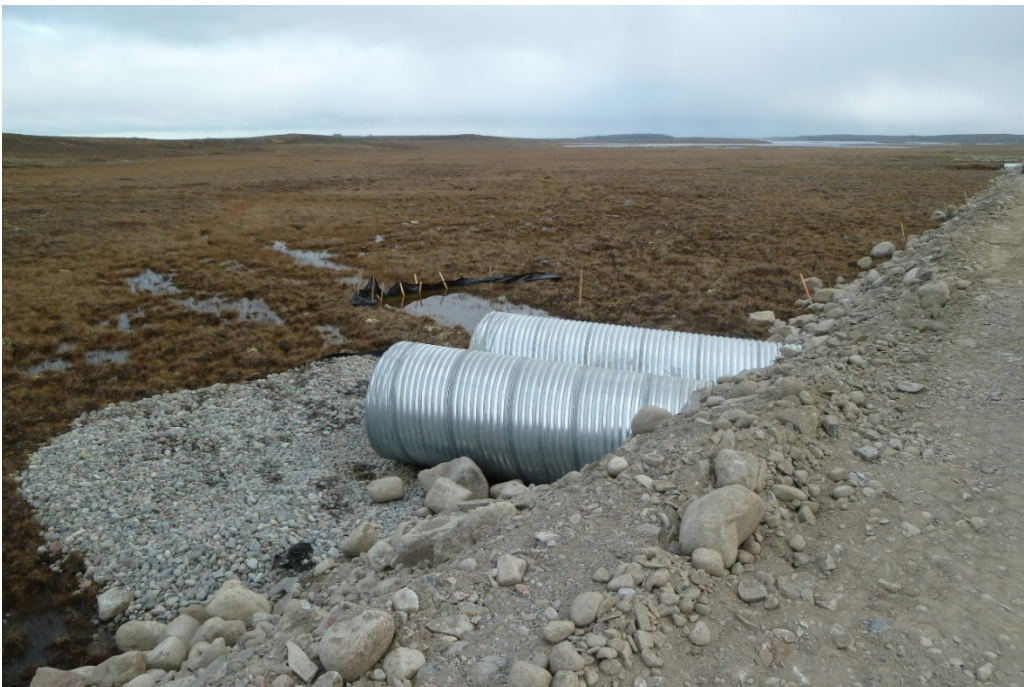
Photograph 28: Itivia Bypass Road, Culverts at 1.4 Kilometers from Intersection with AWAR. View of Culverts on East Side of Road, Looking Southeast (22 September 2017)
