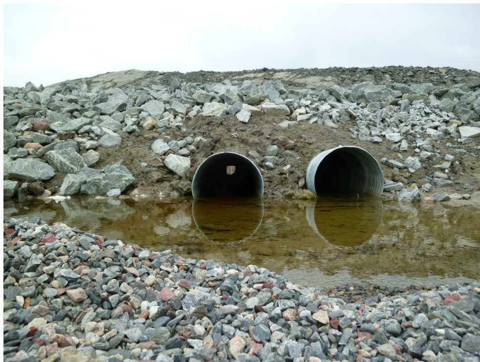
Photograph 16: Itivia Site, Downstream end of Culverts Through Access Road (22 September 2017)
