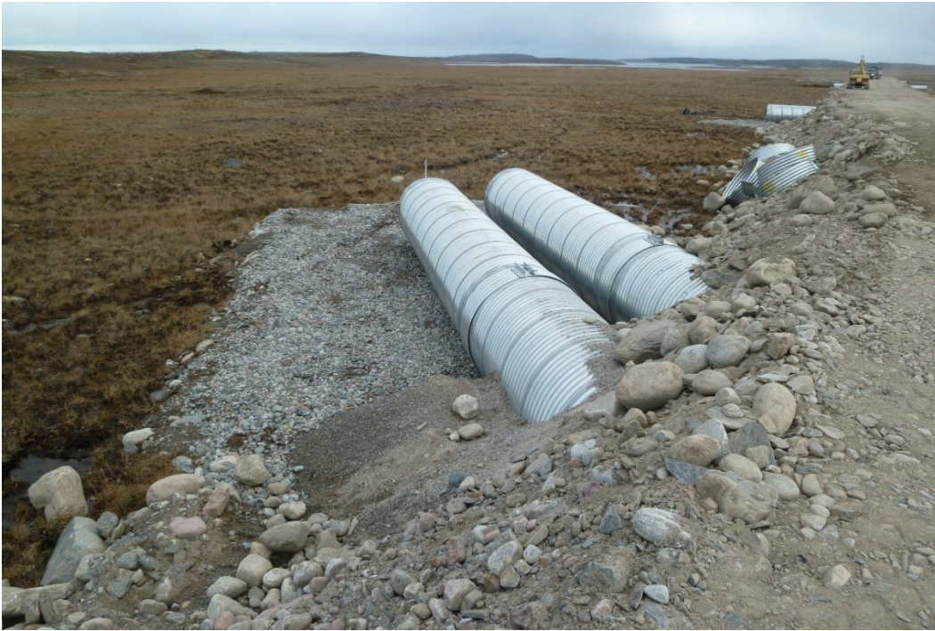
Photograph 25: Itivia Bypass Road, Culverts at 1.3 Kilometers from Intersection with AWAR. View of Culverts on East Side of the Road, Looking South (22 September 2017)
