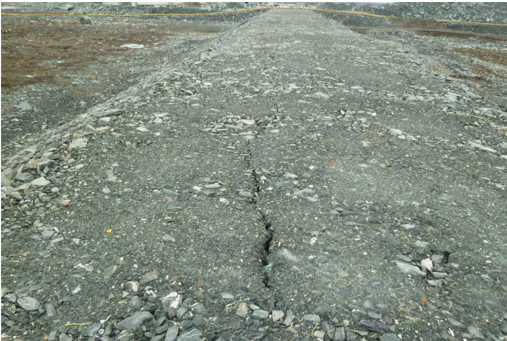
Photograph 4: DP1-A, Cracking Observed On Crest (20 September 2017)
