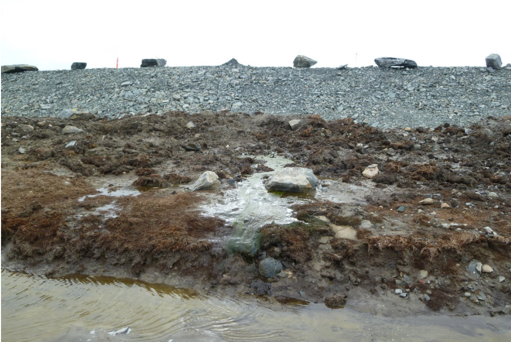
Photograph 15: DP1-B, Seepage Visible from Dike Toe near Station 0+190 (20 September 2017)
