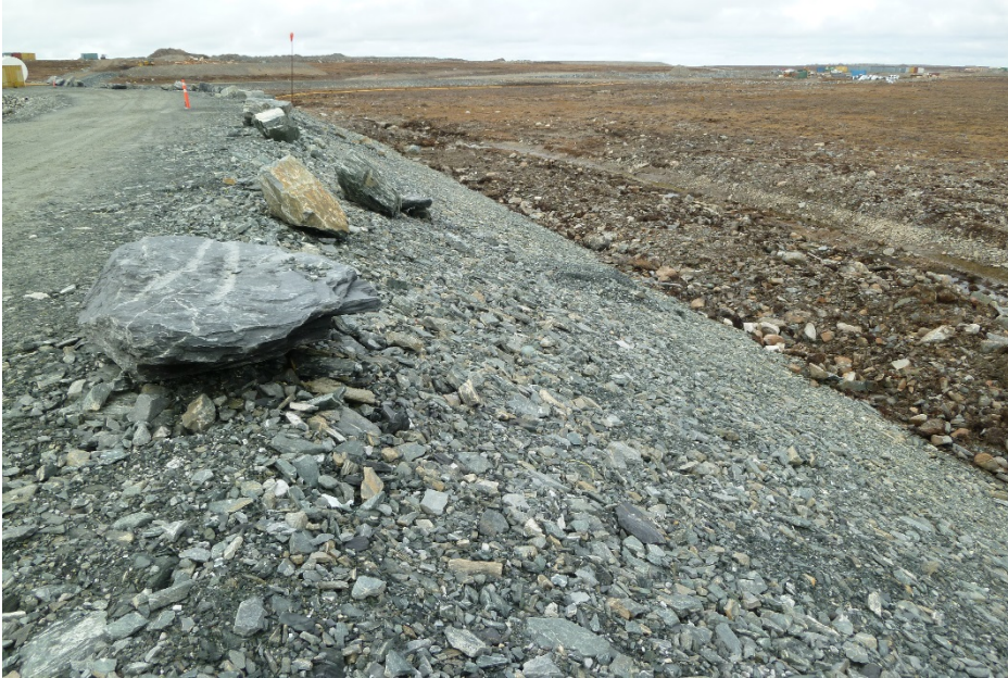
Photograph 11: DP1-B, Downstream Slope near Station 0+240, Looking West. Orange Delineator on Crest Marks Thermistor Location (20 September 2017)
