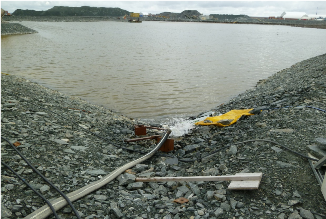
Photograph 17: DP1-B, Seepage Water being Pumped back into P1 from Downstream Sump, East of Snow Melt Pond (20 September 2017)
