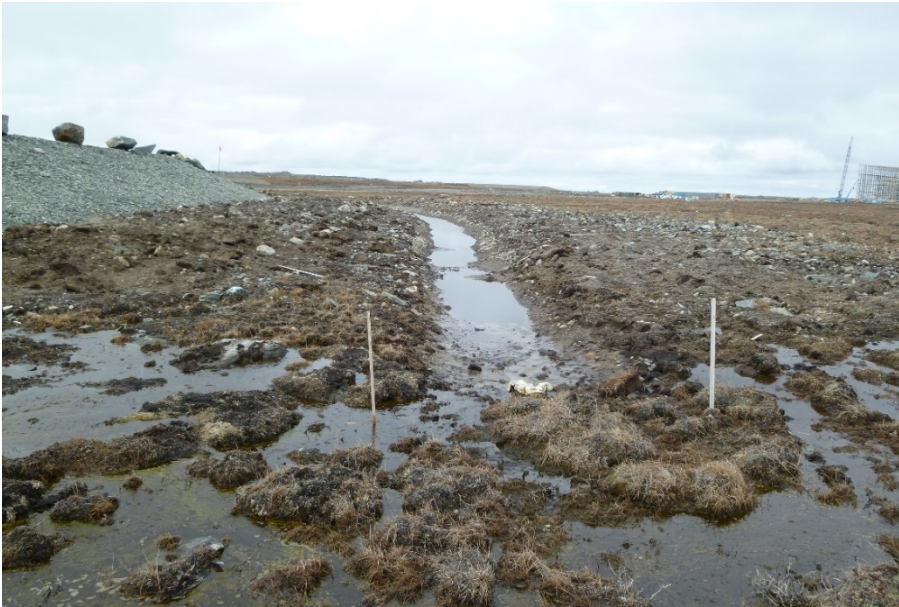
Photograph 13: DP1-B, Run-off and Seepage Collection Channel Downstream of Dike near Station 0+300, Looking West (20 September 2017)
