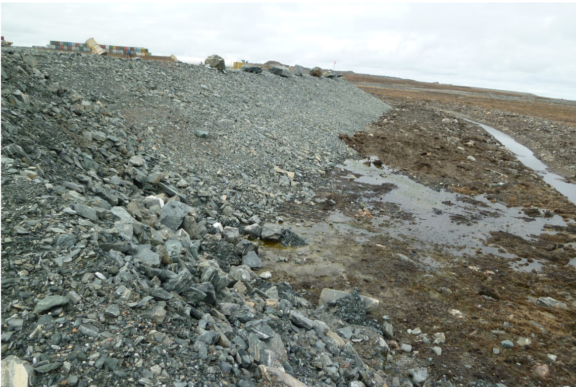
Photograph 12: DP1-B, Downstream Slope near Station 0+300, Looking West from Access Ramp. Some Seepage from Downstream Toe. Run-off and Seepage Collection Channel to Right of Photograph (20 September 2017)
