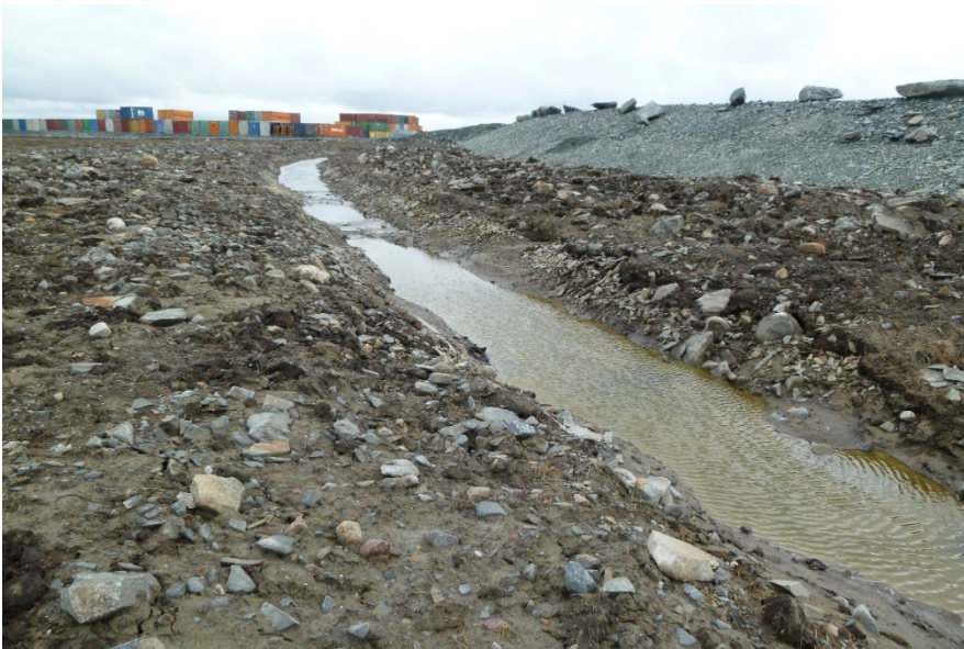
Photograph 14: DP1-B, Run-off and Seepage Collection Channel Downstream of Dike near Station 0+200, Looking East. Visible Flow towards Sump (20 September 2017)
