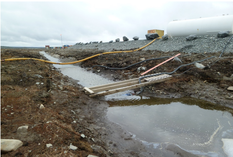
Photograph 16: DP1-B, Downstream Channel and Sump near Station 0+120, Looking East. Active Pumping at Time of Site Visit (20 September 2017)
