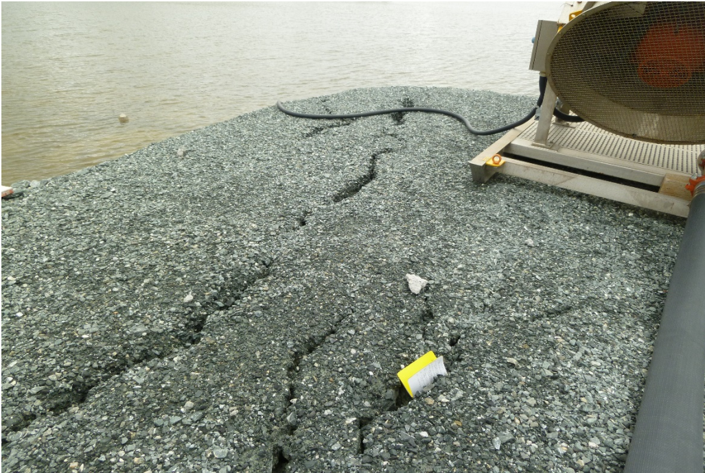
Photograph 25: DP1-B, Cracking Observed (3 to 10 cm wide) in Jetty for Evaporator #1
