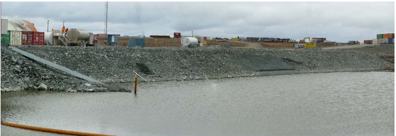
Photograph 36: DP2-A, Upstream Face of West End of Dike, Looking South. Repair of Previous Sloughing of the Slope Visible, near Station 0+065 (20 September 2017)
