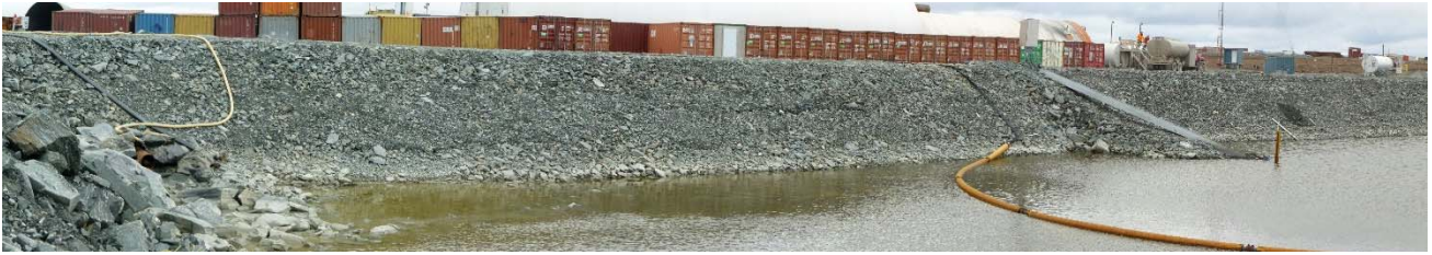
Photograph 35: DP2-A, Upstream Face of East End of Dike, Looking South, some Cracking Visible (20 September 2017)
