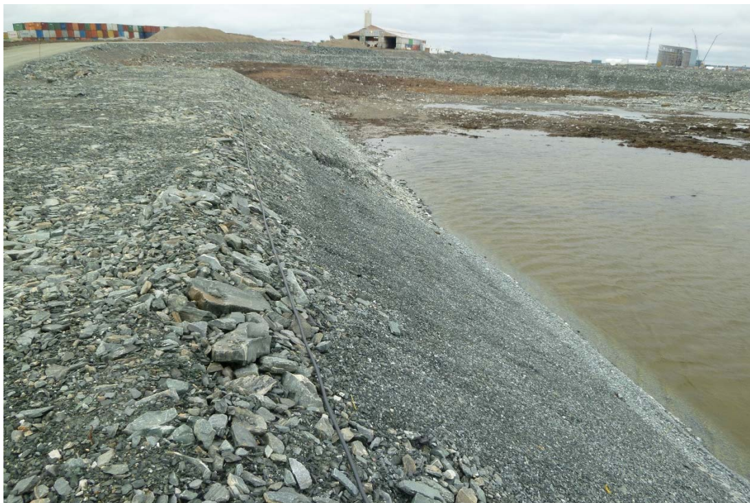
Photograph 31: DP2-A, Upstream Slope near Station 0+065, Looking West. Finer Grained Material on Slope Where Historic Slump was Remediated (20 September 2017)
