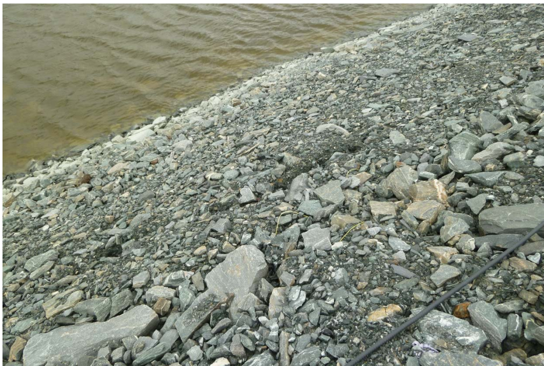
Photograph 32: DP2-A, Cracking on Upstream Slope near Station 0+075 (20 September 2017)
