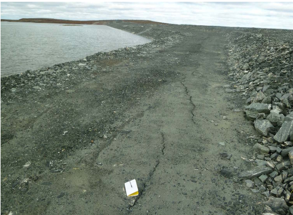
Photograph 4: D-CP1, Cracking on Upstream Bench Crest near Station 1+150, Looking Northeast (19 September 2017)
