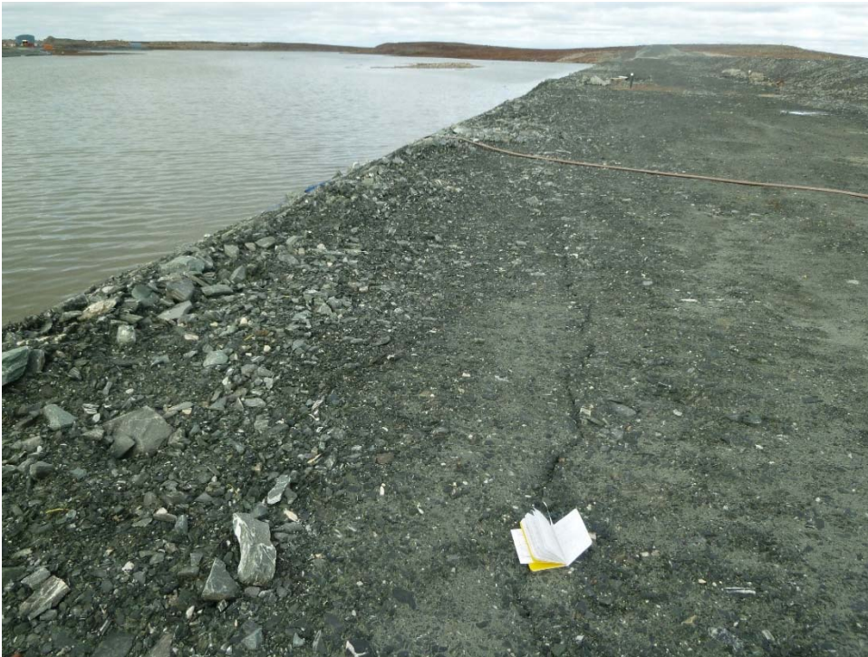
Photograph 5: D-CP1, Cracking along Upstream Bench Crest near Station 1+225, Looking North (19 September 2017)
