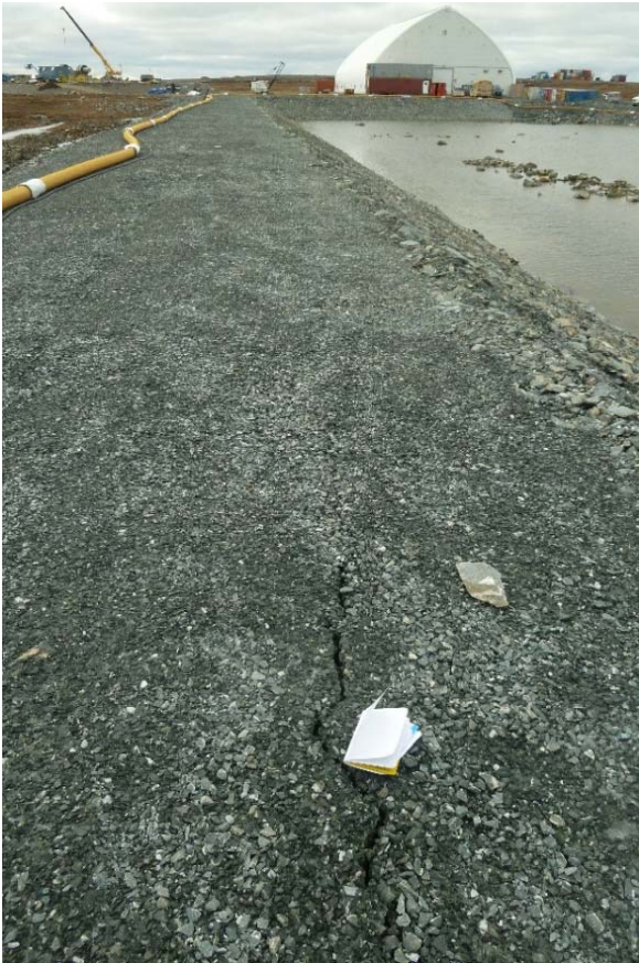
Photograph 47: DP3-A, Cracking Observed on Crest near Station 0+140 (19 September 2017)
