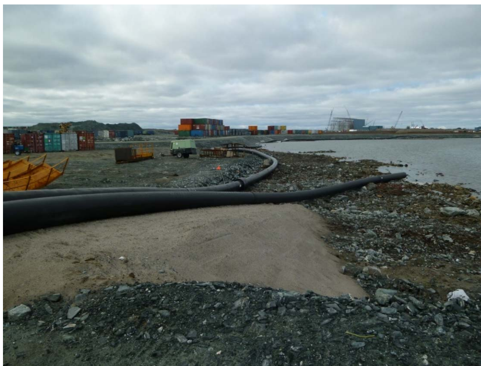
Photograph 2: D-CP1, Water Pipeline Ramp Upstream of the Dike near Station 1+140, Looking West. Sand is Susceptible to Erosion (19 September 2017)
