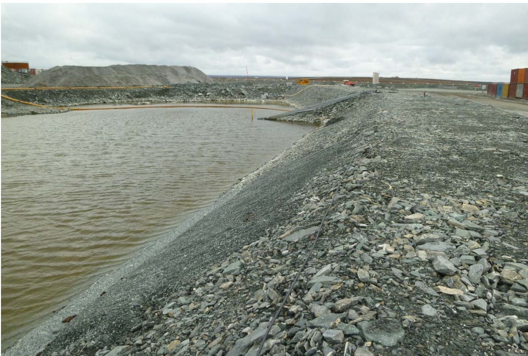
Photograph 30: DP2-A, Upstream Slope near Station 0+025, Looking East. Finer Grained Material on Slope Where Historic Slump was Remediated (20 September 2017)
