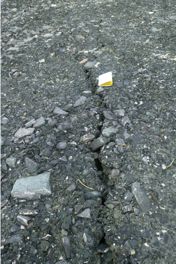
Photograph 9: D-CP1, Crack (approximately 2 to 3 cm wide) on Upstream Bench near Station 1+435 (19 September 2017)
