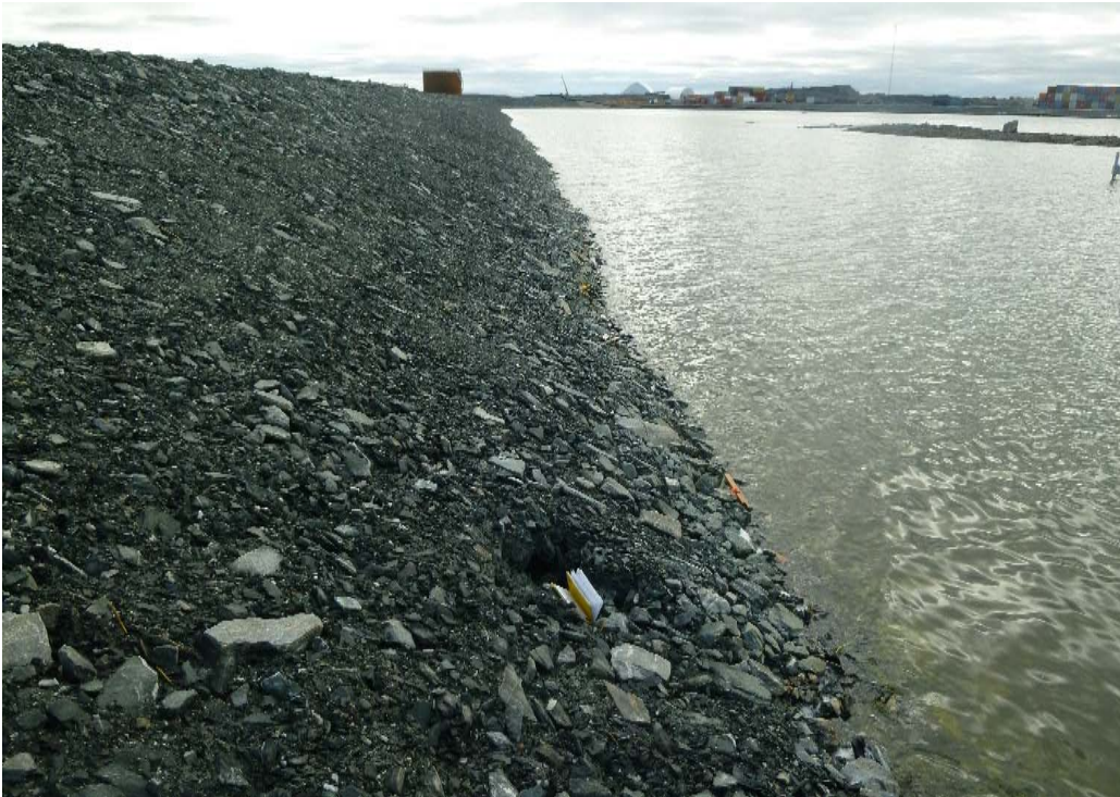
Photograph 10: D-CP1, Small Settlement/depression near Upstream Toe near Station 1+500, Looking South (19 September 2017)
