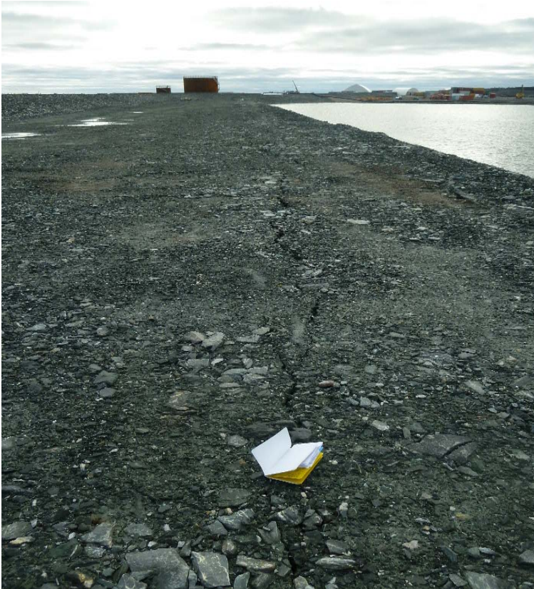
Photograph 8: D-CP1, Cracking along Upstream Bench Crest near Station 1+450, Looking South (19 September 2017)
