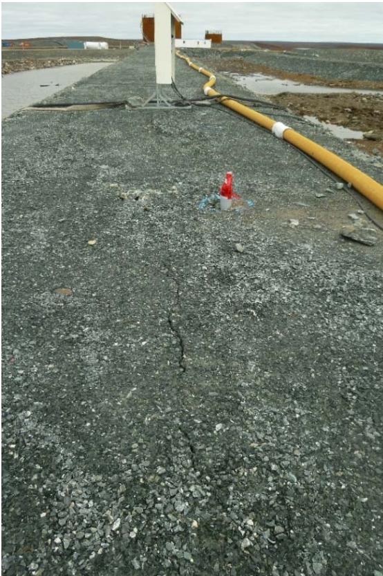
Photograph 46: DP3-A, Cracking Observed on Crest near Station 0+150, Looking Southwest (19 September 2017)
