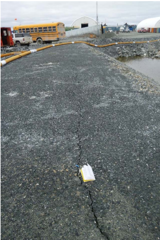
Photograph 50: DP3-A, Cracking Observed on Crest from Station 0+000 to 0+050, Looking West (19 September 2017)
