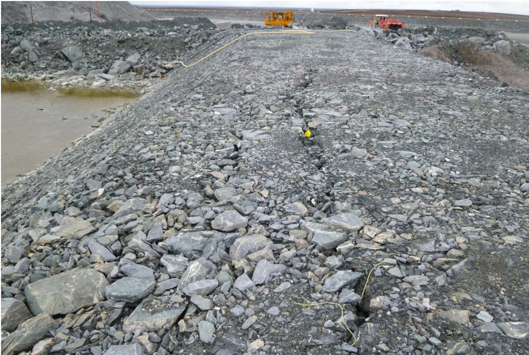
Photograph 33: DP2-A, Cracking on Crest of Dike near Station 0+090, Looking East (20 September 2017)
