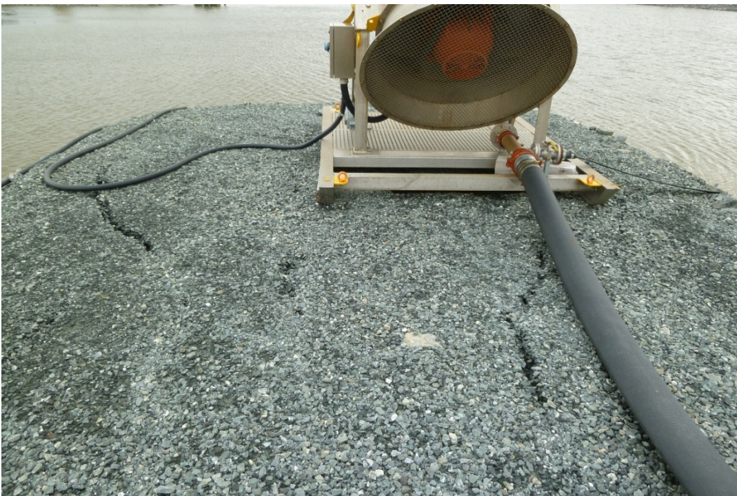
Photograph 24: DP1-B Cracking Observed in Crest of Jetty for Evaporator #2
