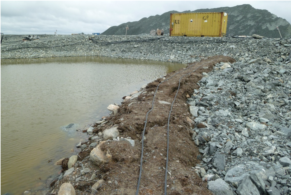
Photograph 27: P1 Till Dividing Berm, Erosion and Cracking Observed, Looking East near Intersection with DP1-B (Station 0+420)
