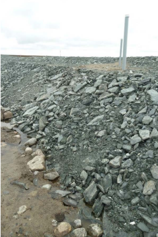
Photograph 38: D-CP5, Ponded Water at Upstream Toe of Dike near Station 1+185. Vertical Temperature Cables (VGTC-1 and 2) in Background (19 September 2017)
