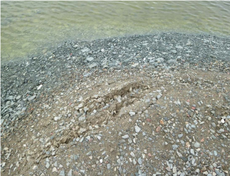
Photograph 47: D-CP5, Jetty 5, Cracking and Settlement of the Southwest Toe of the Jetty (19 September 2017)
