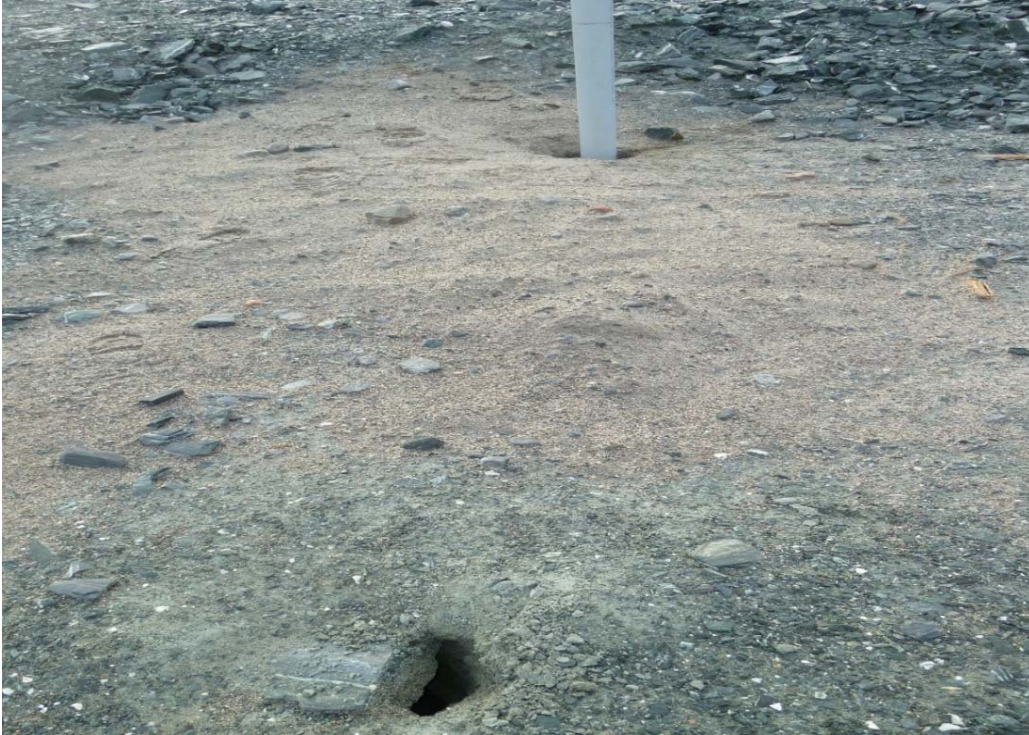
Photograph 35: D-CP5, Small Hole in Upstream Crest near Station 1+185. Vertical Temperature Cable (VGTC-2) in Background (19 September 2017)
