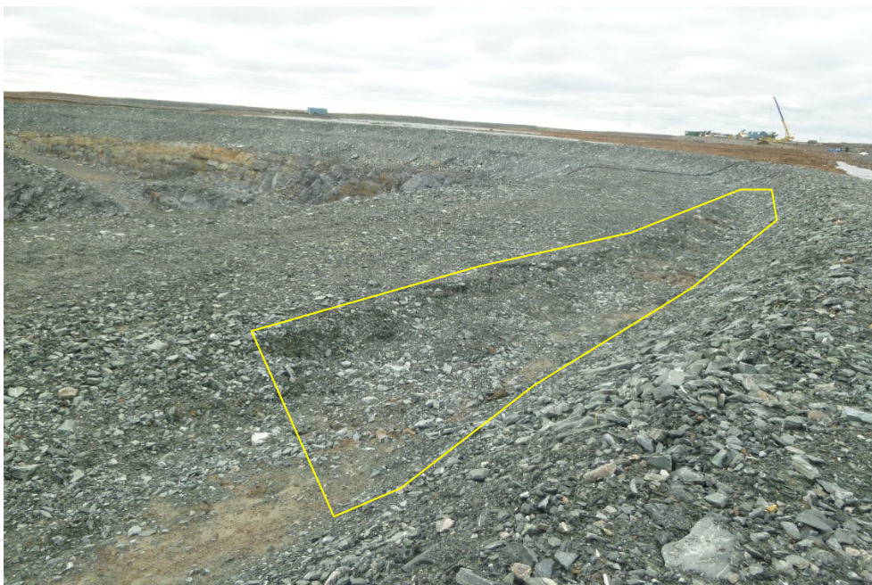
Photograph 62: Saline Pond, Possible Settlement near Toe of Northwest Perimeter Berm (19 September 2017)
