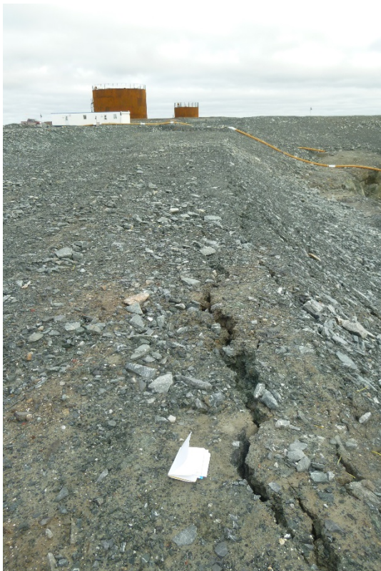
Photograph 61: Saline Pond, Cracking in Perimeter Berm on Northwest Side of Pond (19 September 2017)
