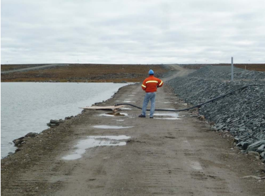
Photograph 37: D-CP5, Pump Back Discharge on Upstream Slope (after being extended) near Station 1+170 (19 September 2017)
