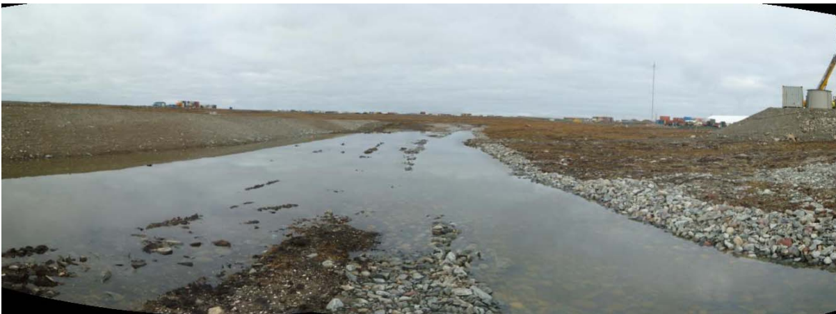
Photograph 51: Channel 5, Looking West near Station 0+145. Water has Overflowed Channel 5 and is Ponding against Berm 3 (19 September 2017)
