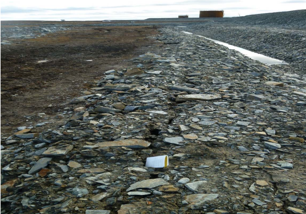
Photograph 22: D-CP1, Cracking Downstream of the Seepage Collection Channel near Station 1+330, Looking South (19 September 2017)
