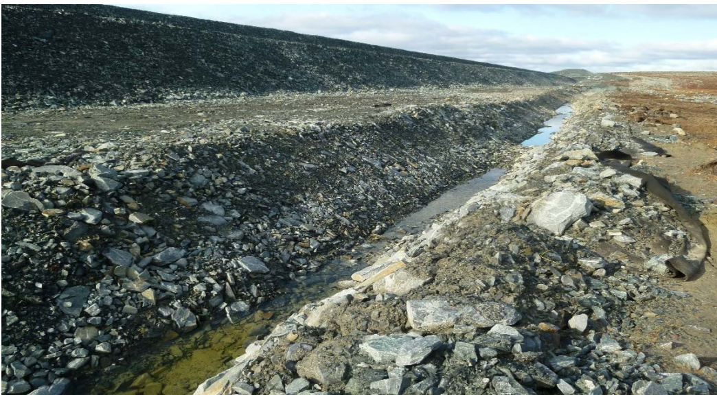
Photograph 23: D-CP1, Downstream Seepage Collection Channel near Station 1+285, and Looking North (19 September 2017)
