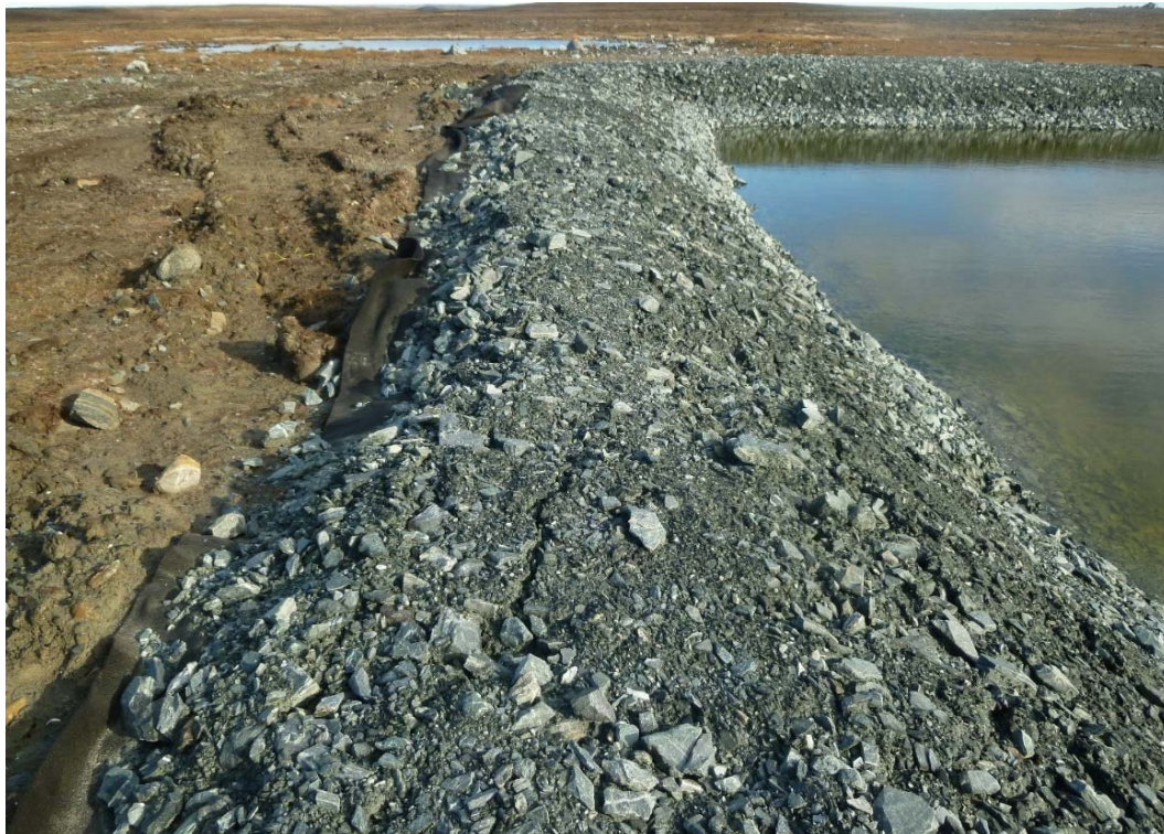
Photograph 24: D-CP1, North Side of Downstream Pond, and Some Cracking/slumping, Looking East (19 September 2017)
