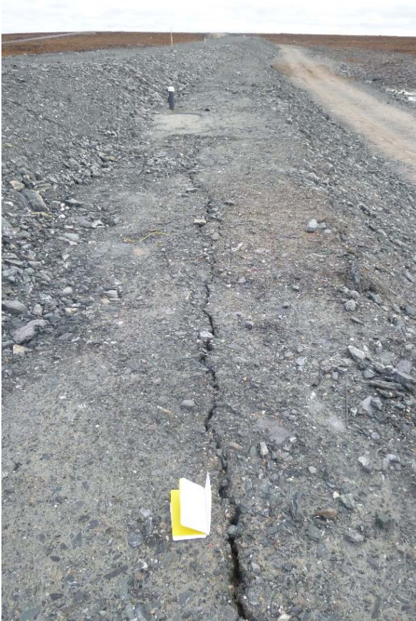
Photograph 44: D-CP5, Cracking on Downstream Berm Crest near 1+ 175, Looking Northeast (19 September 2017)
