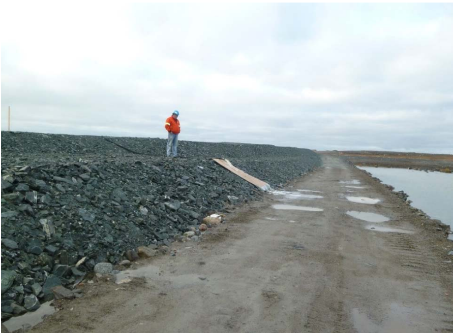
Photograph 36: D-CP5, Pump Back Discharge on Upstream Slope (prior to being extended) near Station 1+170 (19 September 2017)
