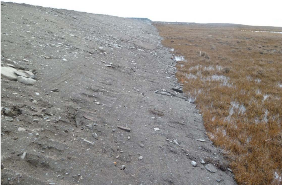
Photograph 57: Berm 3, Downstream Slope near Mid-point of Dike, Water Poned within Vegetation, Looking Southeast (19 September 2017)
