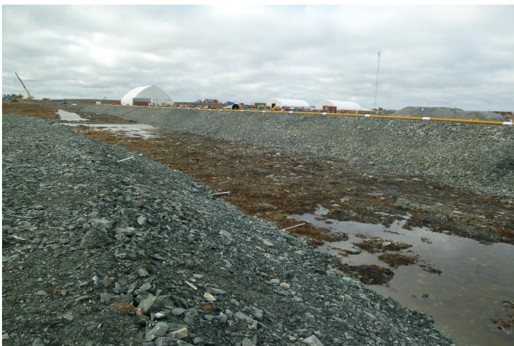
Photograph 66: Saline Pond, Downstream Slope of the Northwest Perimeter Berm and Area between Saline Pond and DCP3-A. Small Amount of Water Ponded Adjacent to the Saline Pond Perimeter Berm (19 September 2017)
