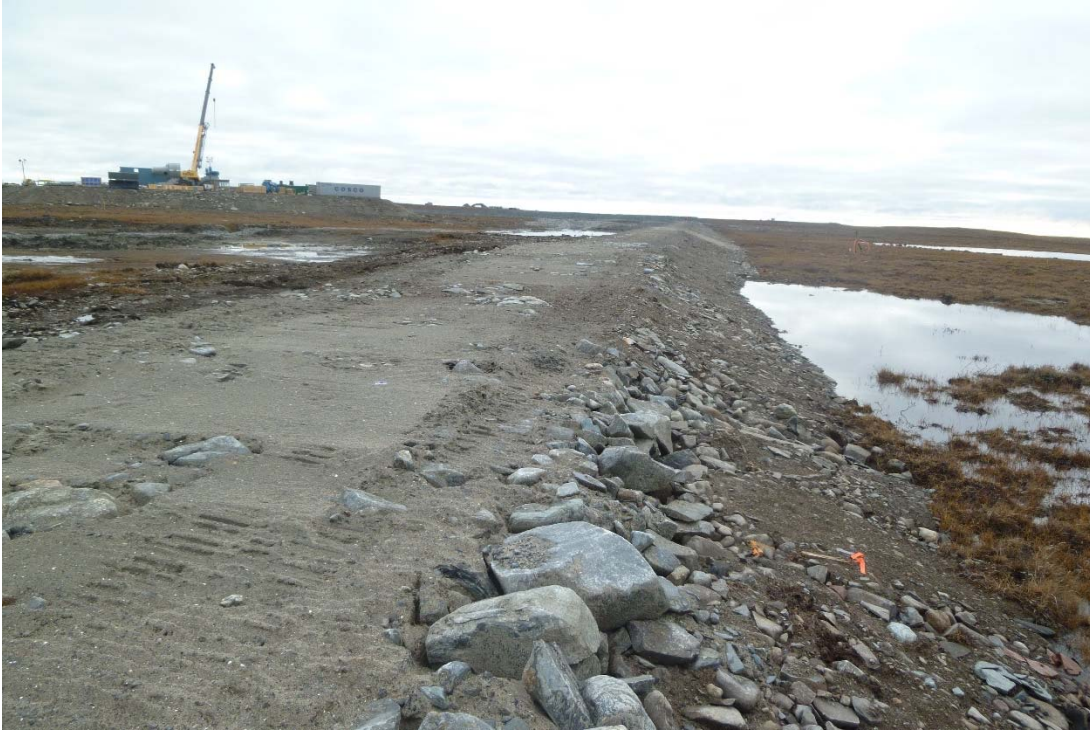
Photograph 56: Berm 3, Downstream Slope and Crest, Small Pond of Water against Downstream Toe near Northwest Abutment, Looking Southeast (19 September 2017)
