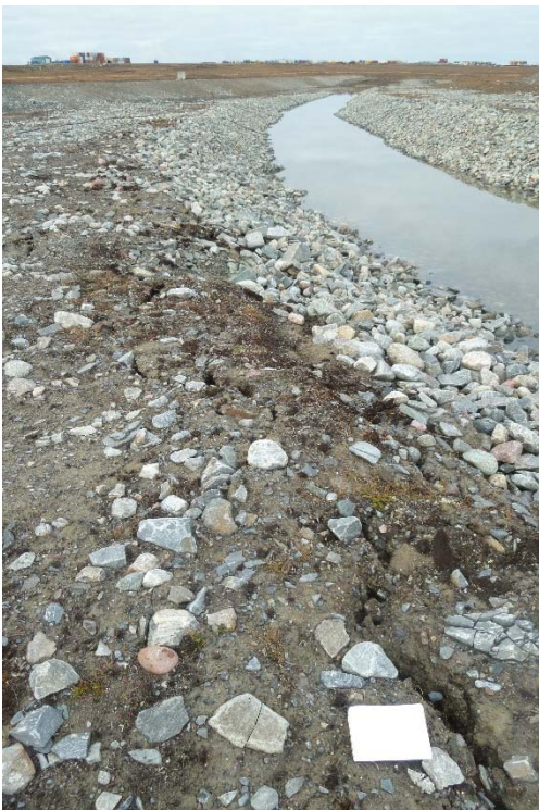
Photograph 49: Channel 5, Looking West from near Station 0+250. Some Cracking Adjacent to Channel (19 September 2017)
