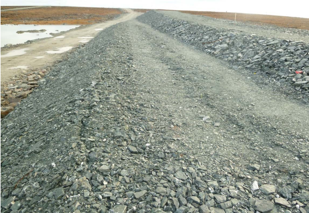
Photograph 31: D-CP5, Minor Settlement and Cracking on Upstream Crest and Slope, near Station 1+210 (19 September 2017)
