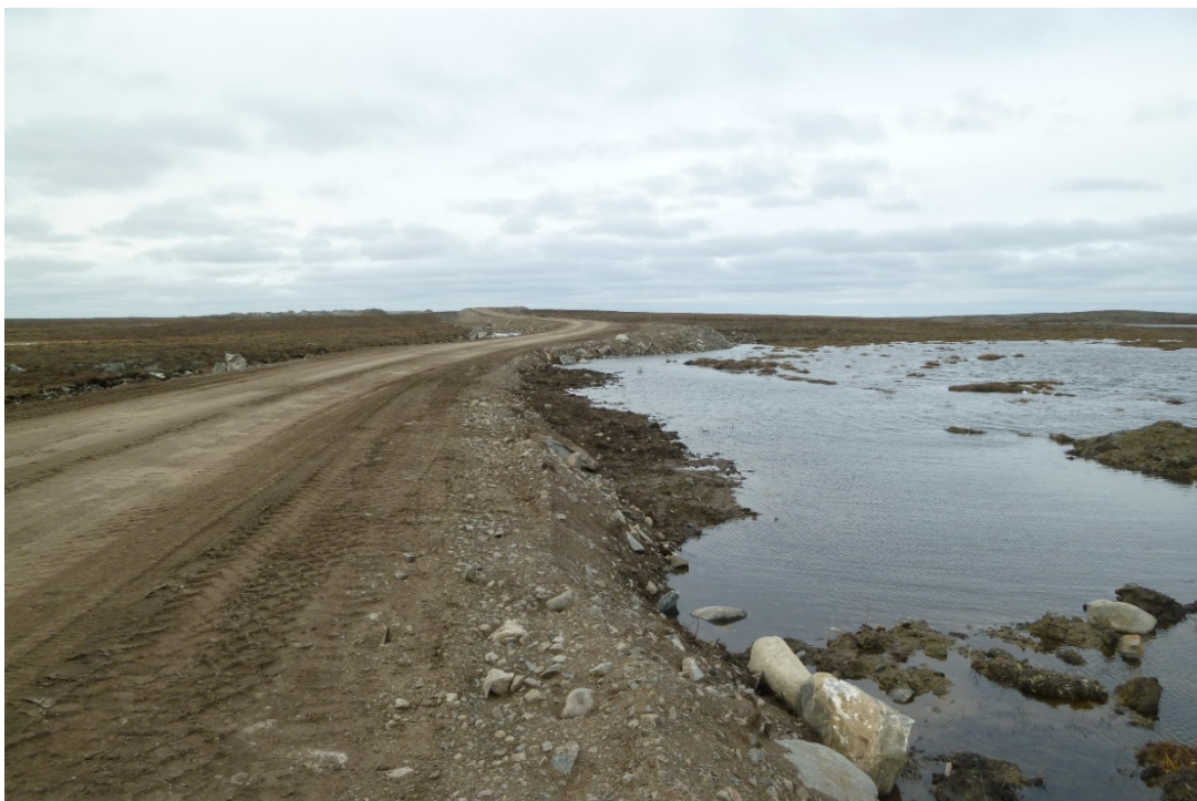
Photograph 30: Emulsion Plant Access Road, Lake H15E Ponding on Northeast Side of the Road near South End of Road. No Culvert Installed (21 September 2017)
