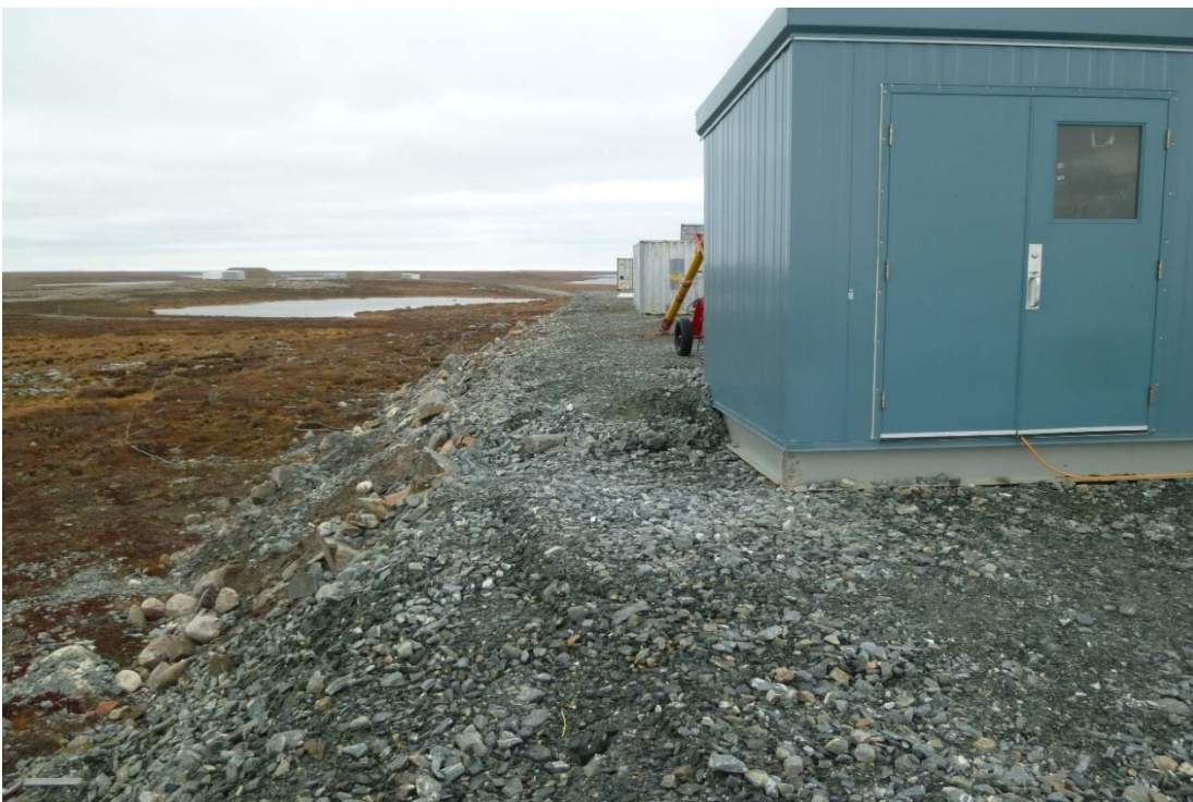
Photograph 24: ANFO Plant Pad, Some Erosion and Settlement on Southwest Slope, Looking Northwest (21 September 2017)
