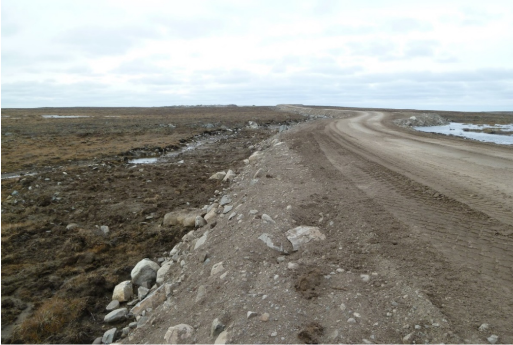
Photograph 31: Emulsion Plant Access Road, Lake H15E in top Right of Photo (Photograph 30), and Minimal Water on Southwest Side of Access Road. No Culvert in Place (21 September 2017)
