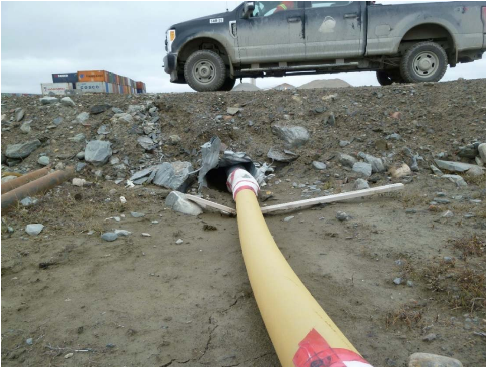
Photograph 9: Road to Tiriganiaq Esker, Culvert for Pipeline Crossing North Side of Road (21 September 2017)
