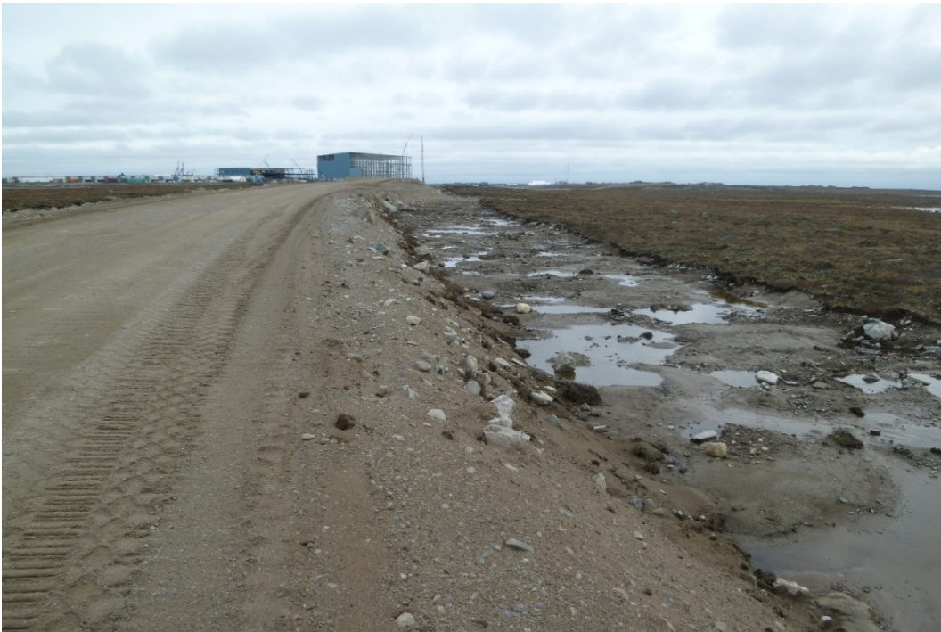
Photograph 32: Emulsion Plant Access Road, Area Stripped Adjacent to the Road with Small Amount of Ponding, Looking Southeast (21 September 2017)
