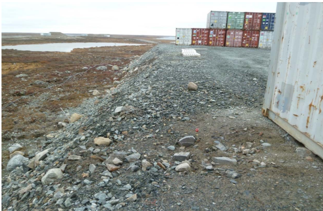
Photograph 25: ANFO Plant Pad, Some Erosion on Southwest Slope, Looking Northwest (21 September 2017)
