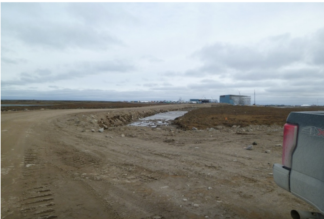
Photograph 39: Emulsion Plant Access Road, Looking South from Emulsion Plant Pad. Water Poned on Southwest Side of Road where Foundation was Stripped (21 September 2017)
