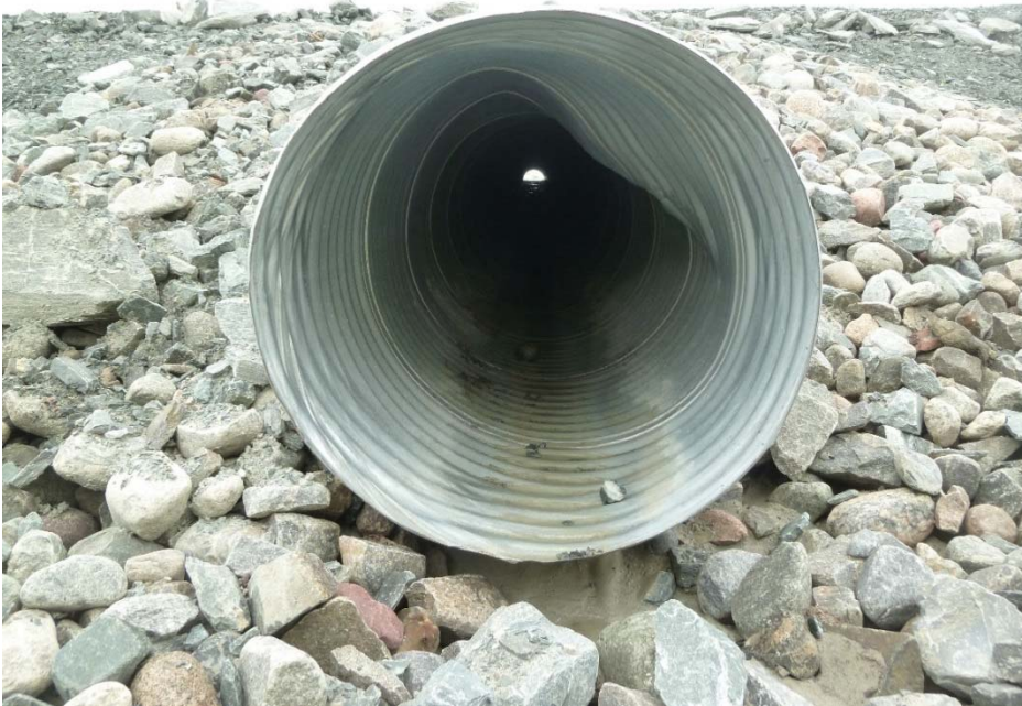
Photograph 5: Culvert #4, Looking Through Upstream End of Culvert. Some Damage Visible (21 September 2017)
