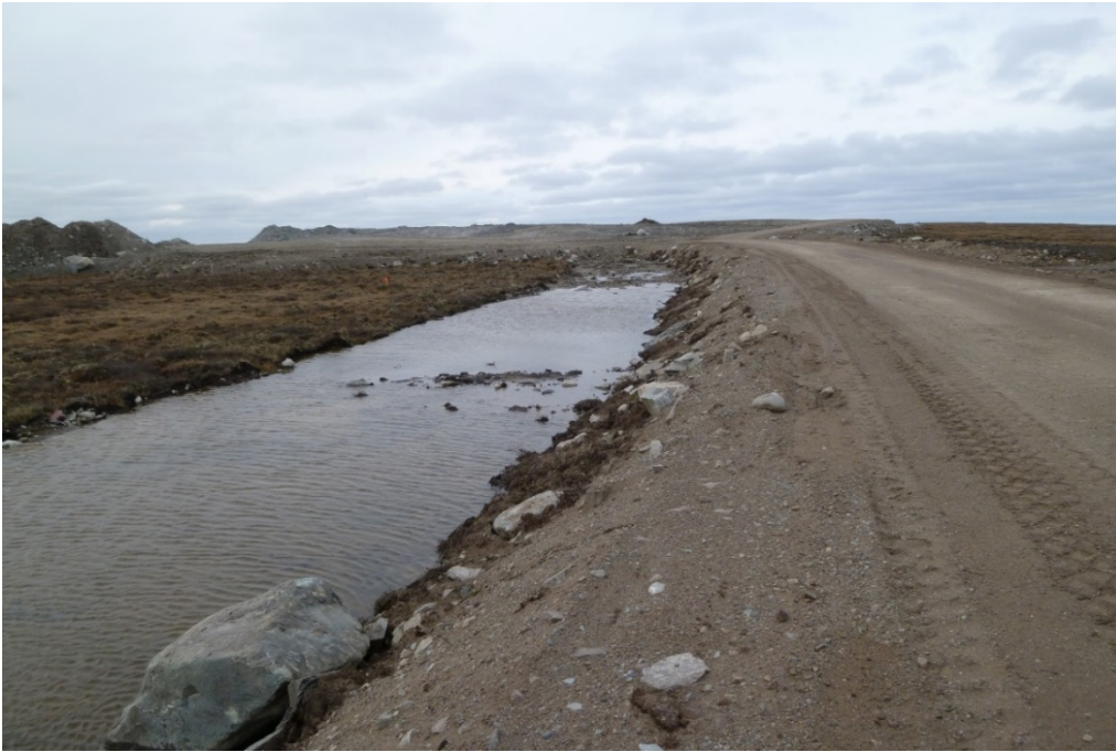
Photograph 33: Emulsion Plant Access Road, Water Poned on Southwest Side of Road where Stripping was Completed, Looking Northwest (21 September 2017)
