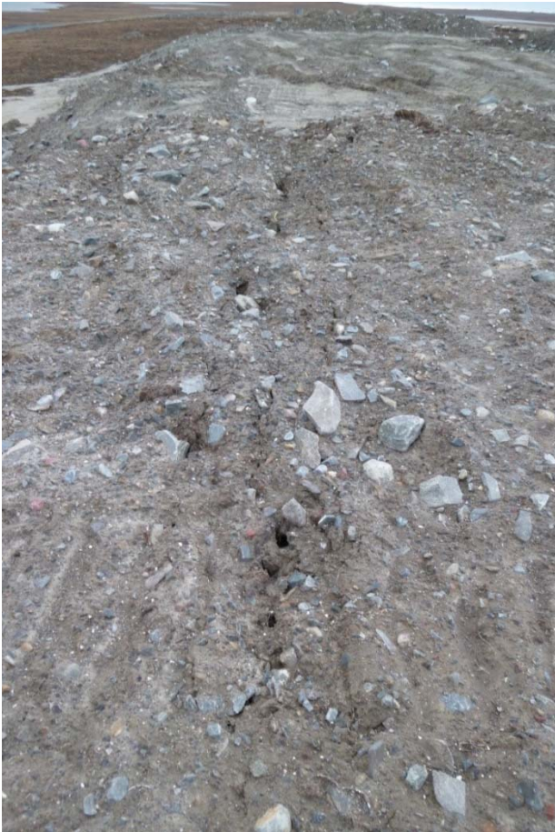
Photograph 17: Wesmeg Borrow Cracking Along Crest of Slope (21 September 2017)
