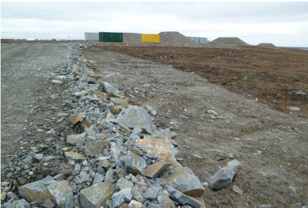
Photograph 14: Road to Wesmeg Borrow, Stripping Along Edge of Road has been Recontoured, Coarser Rockfill Placed on Road Surface, Looking East, Magazine Storage in Background (21 September 2017)
