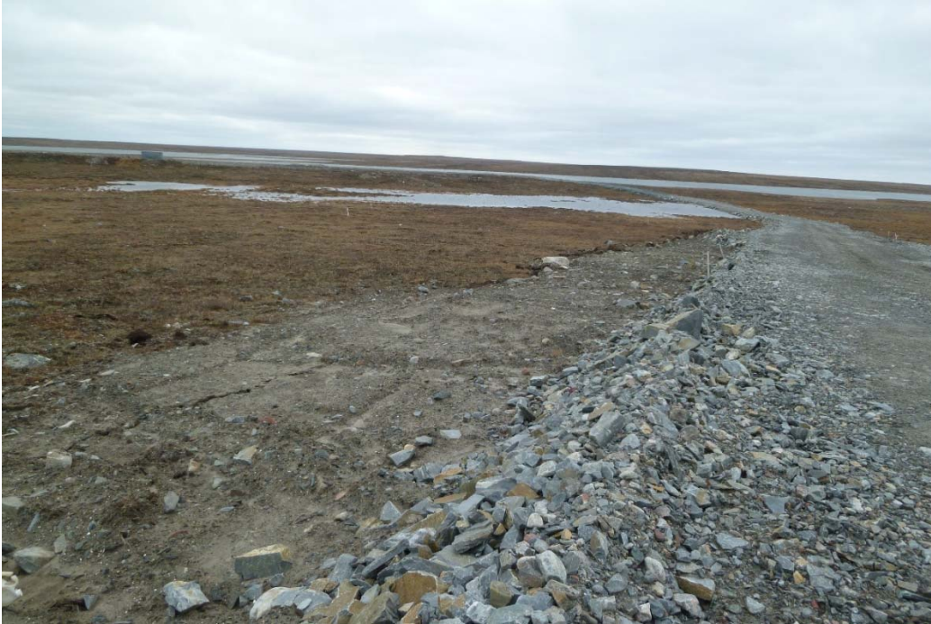
Photograph 13: Road to Wesmeg Borrow, Stripping along Edge of Road has been Recontoured, Water Poned against Road in Low Area in Background, Looking West (21 September 2017)
