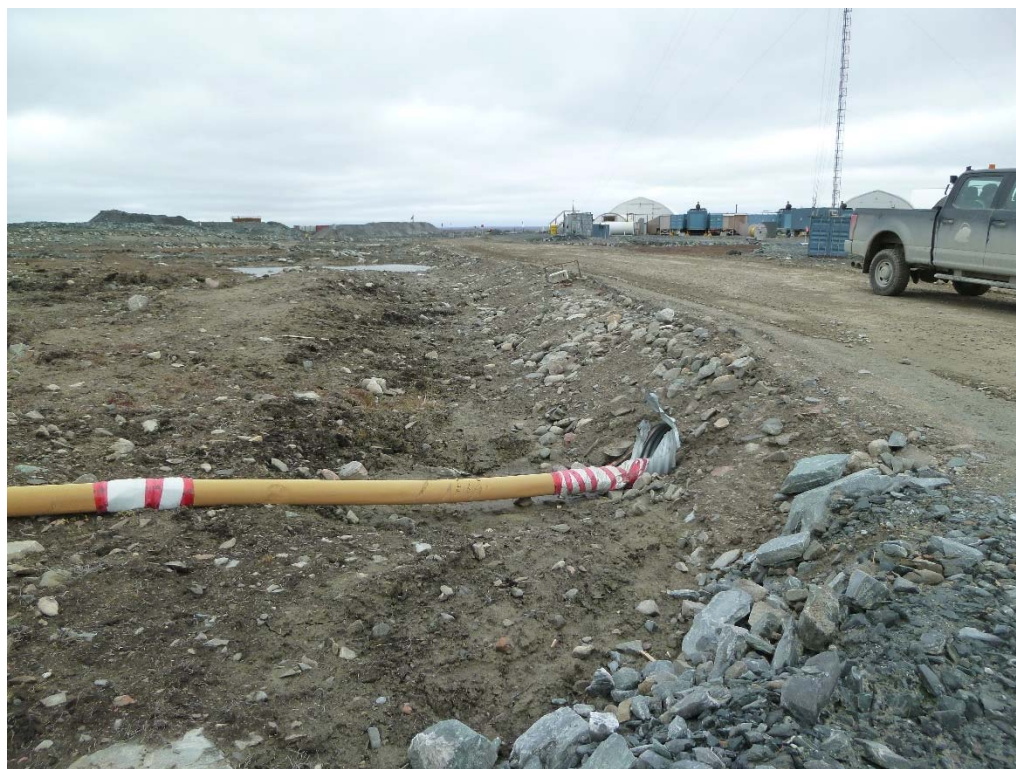
Photograph 8: Road to Tiriganiaq Esker, South Side of Road, Looking West. Culvert for Pipeline Crossing (21 September 2017)
