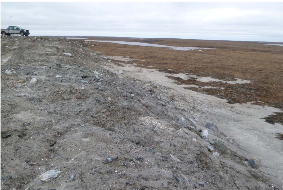
Photograph 16: Wesmeg Borrow, Erosion Downslope, Looking Southeast (21 September 2017)
