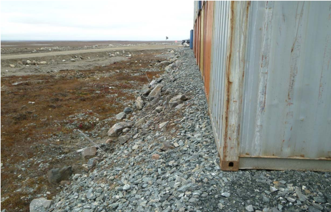
Photograph 27: ANFO Plant Pad, East Slope, Looking North. Sea-containers are Located Very Close to Crest (21 September 2017)
