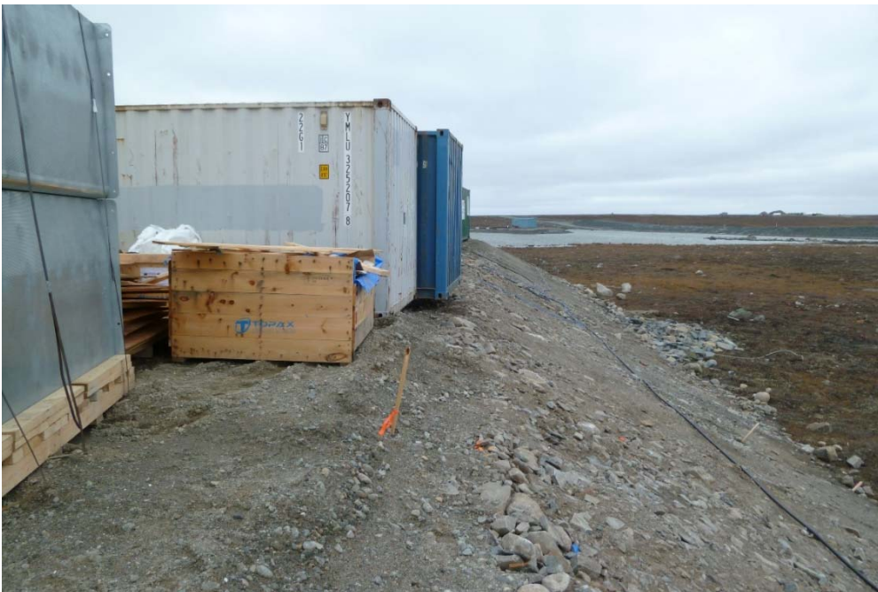
Photograph 58: Ventilation Intake Pad, Southwest Crest and Slope, Looking Southeast. Sea-containers are Located Very Close to Crest (21 September 2017)
