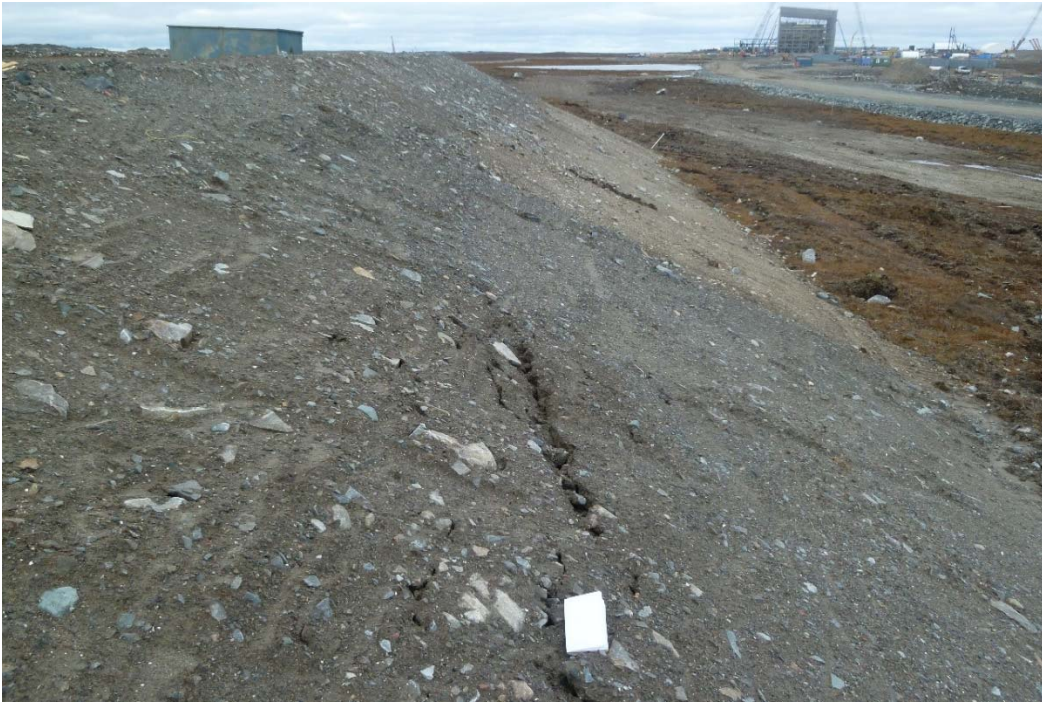
Photograph 65: Exploration Landfill, Cracking Mid Slope of East Berm, Looking North (19 September 2017)
