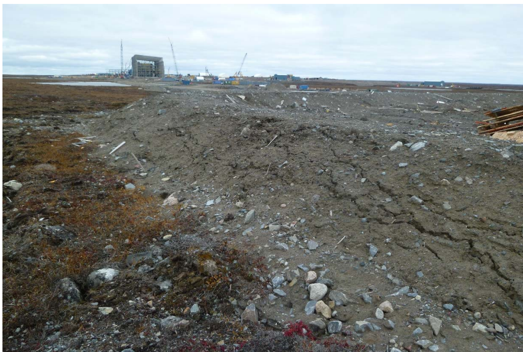
Photograph 62: Exploration Landfill, Downstream Slope of North End of West Berm, Cracking Visible (19 September 2017)
