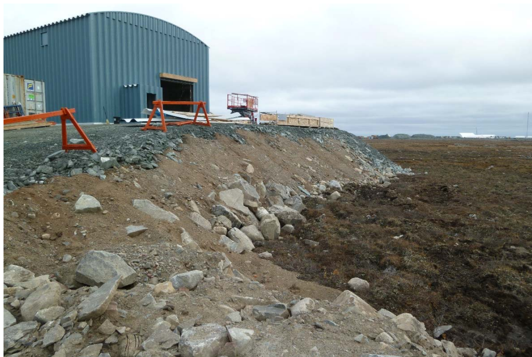
Photograph 14: Incinerator Pad, West Slope, Looking South. Variable Material Used for Pad Construction (21 September 2017)
