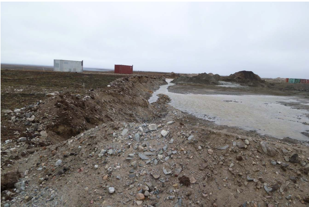
Photograph 10: Industrial Pad, Quarry Area East of Industrial Pad, Water Ponding and Ditching for Water Management, Looking South (21 September 2017)
