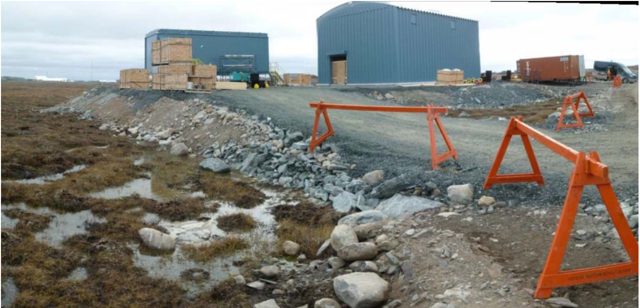
Photograph 15: Incinerator Pad, East Slope Looking South. Variable Material Used for Pad Construction. No Culvert Installed Through Access Road to Incinerator (21 September 2017)
