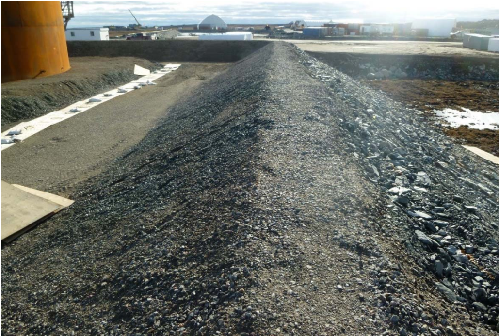
Photograph 52: New Fuel Tank Storage Area, Crest and Inside Slope of Northwest Berm, Looking Southwest (19 September 2017)
