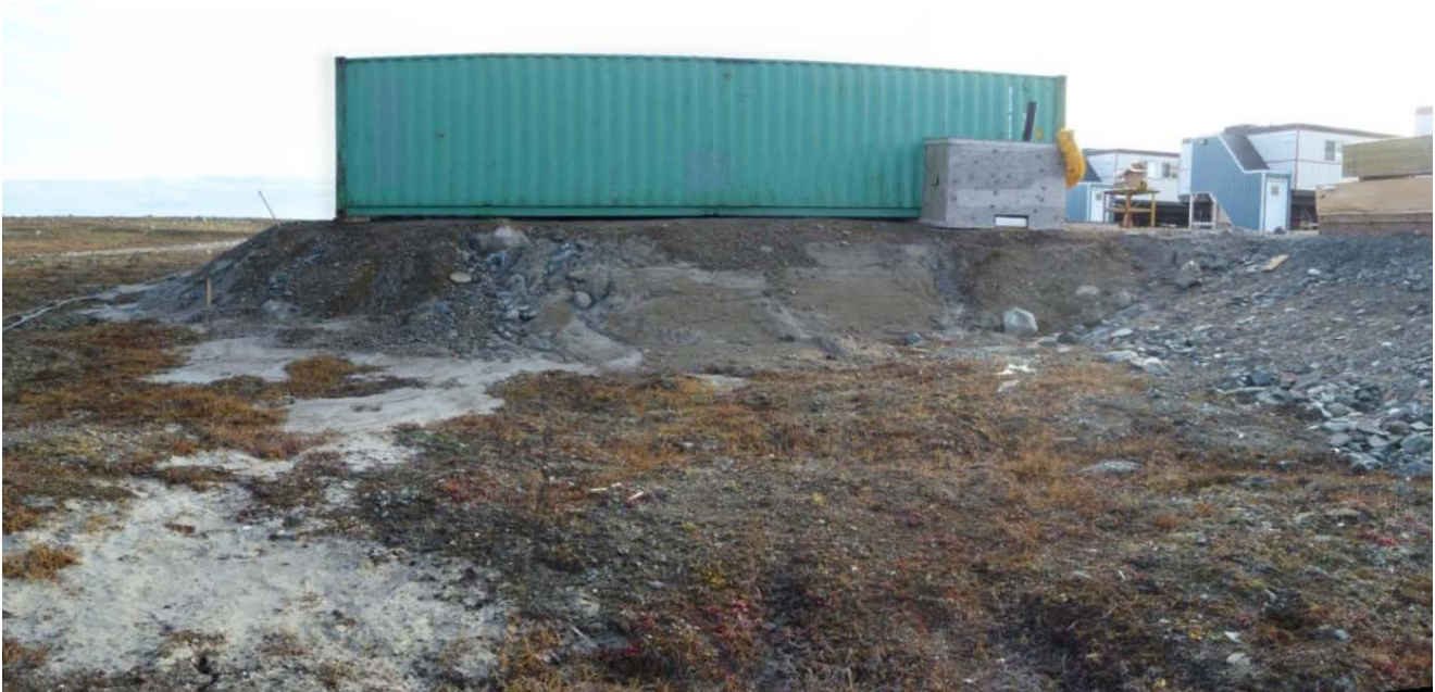
Photograph 4: Industrial Pad, Erosion of North Slope, Looking East (20 September 2017)
