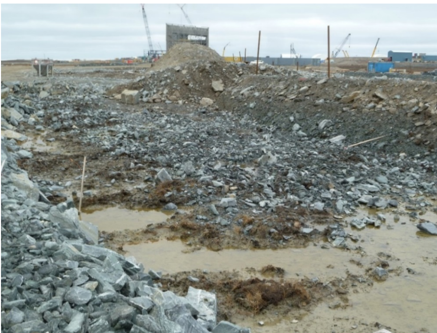
Photograph 47: Portal No. 2, Water Poned Adjacent to the West Side of the Portal Cut, Looking North. No Water Management (21 September 2017)
