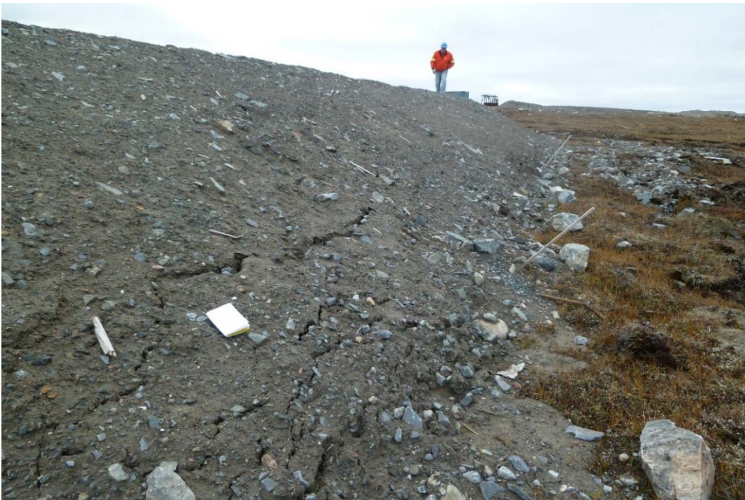
Photograph 64: Exploration Landfill, Cracking on Downstream Slope of North Berm, Looking West (19 September 2017)
