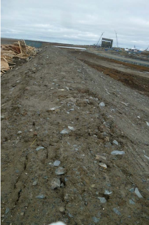
Photograph 67: Exploration Landfill, Crest of East Berm, Looking North. Cracking and some Erosion Visible (19 September 2017)
