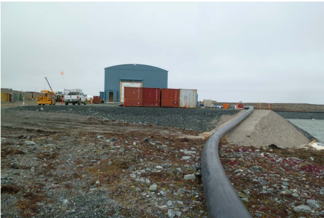
Photograph 25: Effluent Water Treatment Plant, South Slope of Pad, Looking North. Pipe Ramp Constructed with Sand that is Susceptible to Erosion (21 September 2017)
