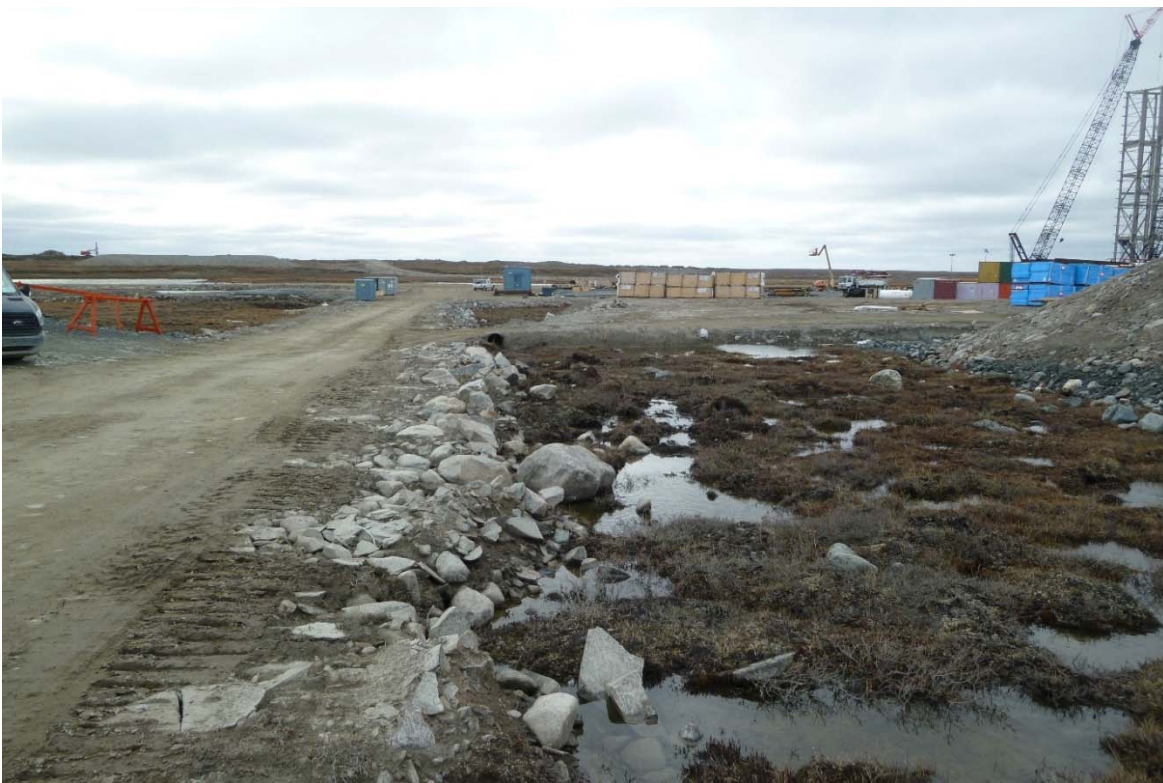
Photograph 12: Industrial Pad, Access Road at South End of Site, Culvert through Access is Exposed (21 September 2017)
