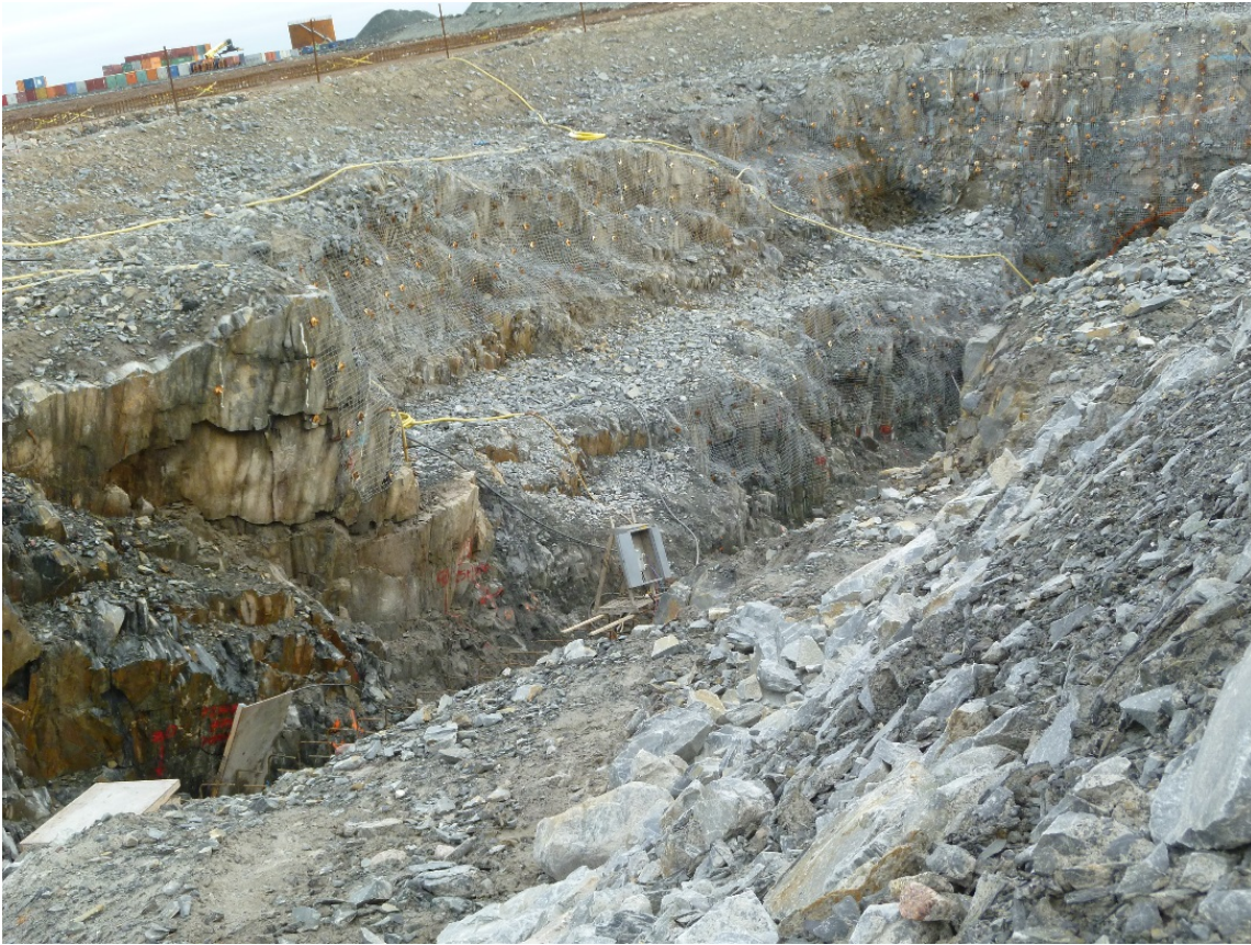
Photograph 44: Portal No. 2, East Rock Cut Face, Looking Southeast, and Some Evidence of Ravelling of Loose Rock onto the Rockfill Bench (21 September 2017)
