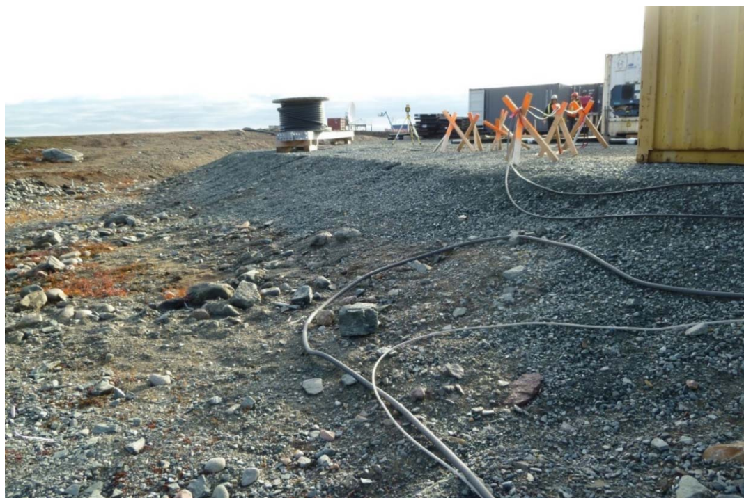
Photograph 6: Industrial Pad, East End of North Slope, Coarser Material, Less Erosion (20 September 2017)
