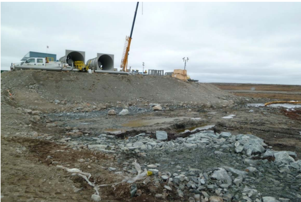
Photograph 56: Ventilation Intake Pad, West Slope, Looking East. Some Fine Grained Material used for Pad which may be Susceptible to Erosion (21 September 2017)
