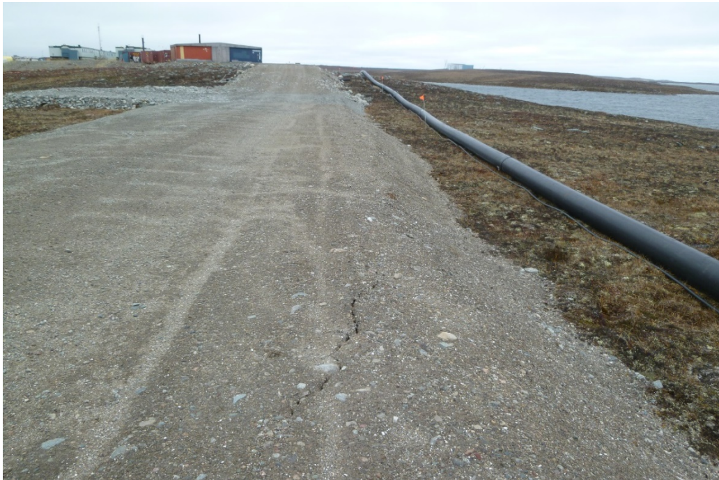
Photograph 16: Exploration Camp Diffuser Access Road, Some Cracking along Slope, Looking Northwest (21 September 2017)
