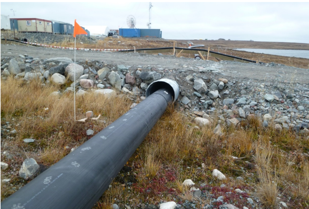
Photograph 12: Exploration Camp Fresh Water Intake Access, Culvert for Pipe Crossing (21 September 2017)
