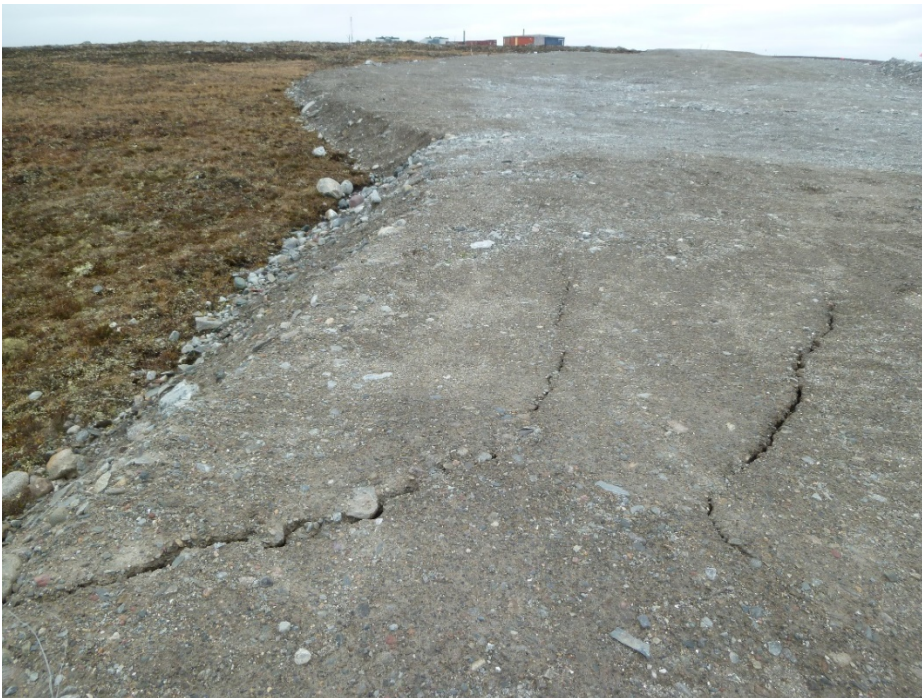
Photograph 18: Exploration Camp Diffuser Access Road, cracking near Southeast end near Meliadine Lake (21 September 2017)
