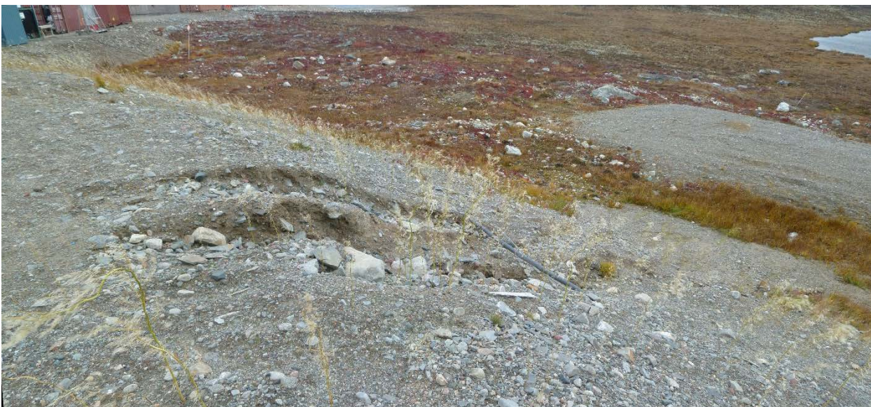
Photograph 4: Exploration Camp Pad, Erosion on South Slope (21 September 2017)
