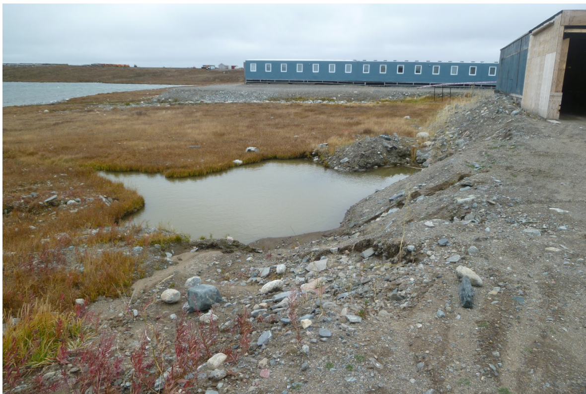
Photograph 5: Exploration Camp Pad, Localized Ponding and Erosion on South Slope (21 September 2017)
