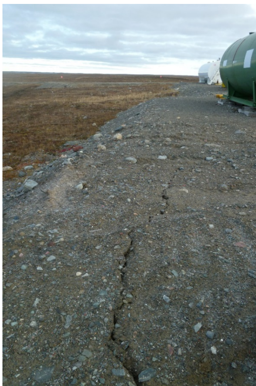
Photograph 30: Exploration Fuel Storage Pad, Cracking along Crest of East Slope, Looking South (19 September 2017)
