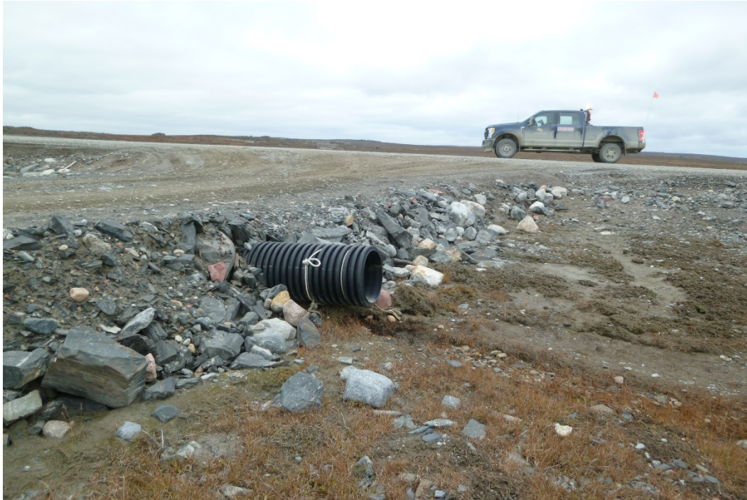
Photograph 3: Downstream End of Culvert through Access Road to B12 Quarry at KM14.7 (20 September 2017)
