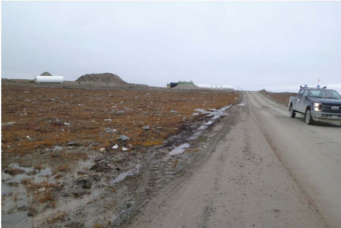
Photograph 27: Exploration Camp Access Road, Water Ponded Along East Edge of Road between Fuel Storage and Intersection with Main Road (21 September 2017)
