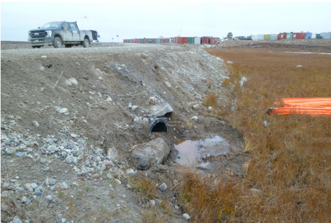
Photograph 26: Exploration Camp Access Road, Downstream end of Culver near Fuel Storage, Partially Blocked (21 September 2017)
