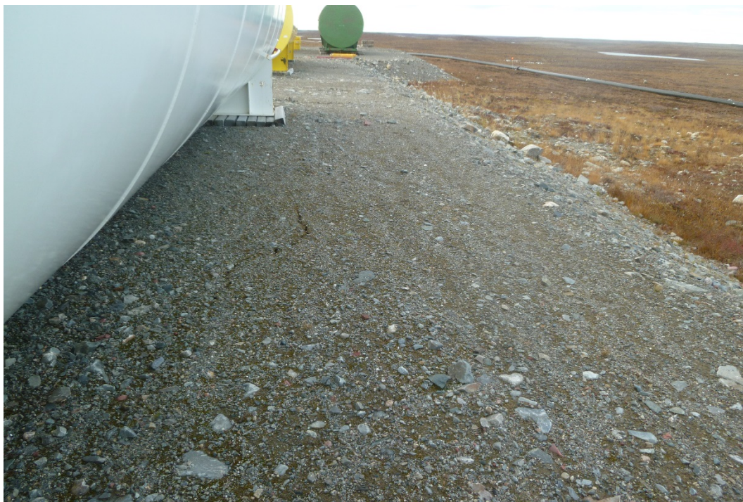
Photograph 31: Exploration Fuel Storage Pad, Minor Cracking near Crest of East Slope, Looking North (19 September 2017)
