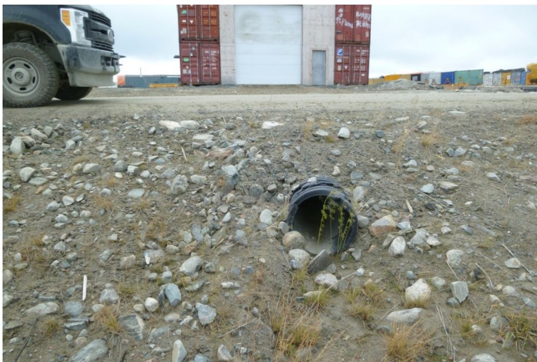
Photograph 22: Exploration Camp Access Road, Downstream end of Culvert near Camp (22 September 2017)
