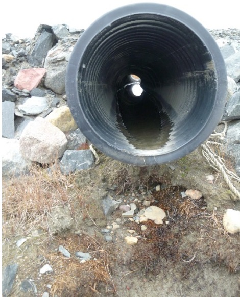
Photograph 2: View through Culvert Under Access Road to B12 Quarry at KM14.7, Some Dents, No Flow, Small Amount of Ponded Water Within Culvert (20 September 2017)
