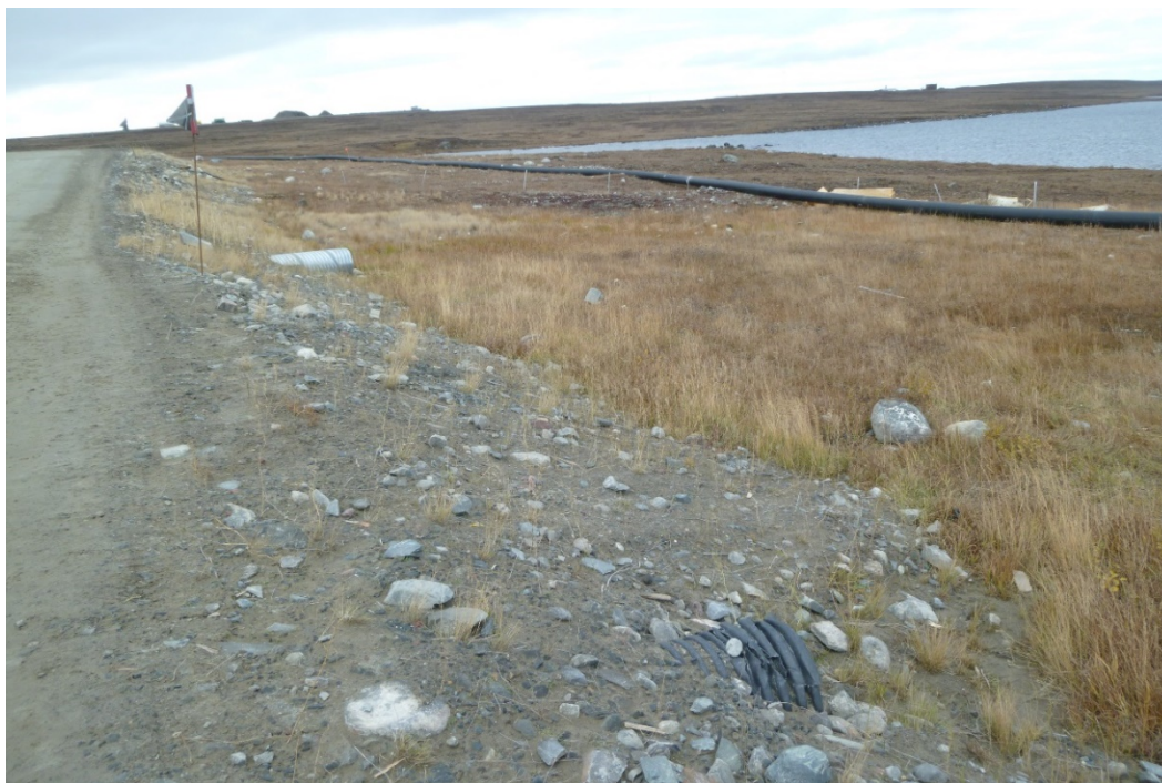
Photograph 21: Exploration Camp Access Road, Downstream ends of Culverts near Camp (black corrugated plastic and corrugated steel) (22 September 2017)
