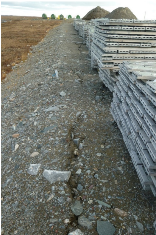
Photograph 40: Core Storage Pad, Cracking on Crest of East Slope, Looking South (19 September 2017)
