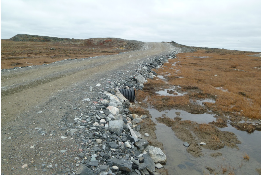
Photograph 1: At KM14.7, Access Road to B12 Quarry. Upstream End of 500 mm \varnothing Corrugated HDPE Culvert. Some Ponding Against Quarry Access Road and AWAR below Inlet of Culvert (20 September 2017)
