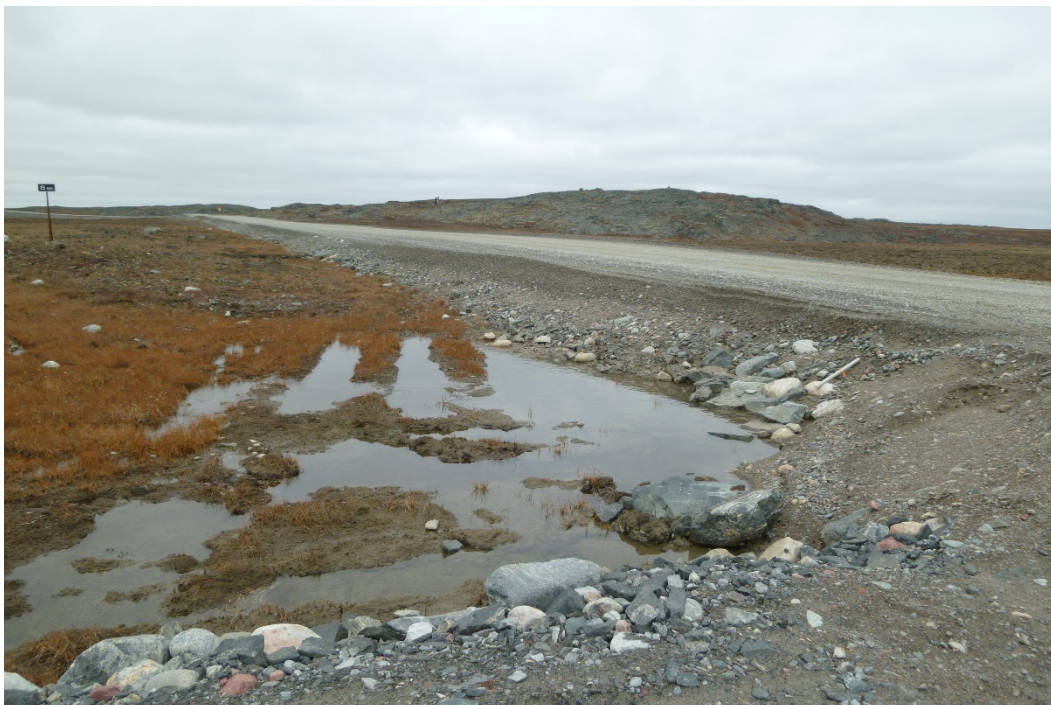
Photograph 4: Water Pooled Adjacent to AWAR and Access Road to B12 Quarry at KM14.7. Looking at AWAR from Quarry Access Road. (20 September 2017)
