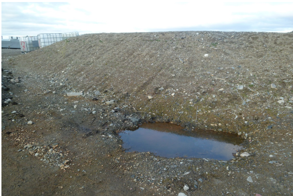
Photograph 34: Exploration Camp Landfarm, Small Pond of Water at Toe of Northeast Corner, Possible Seepage (19 September 2017)
