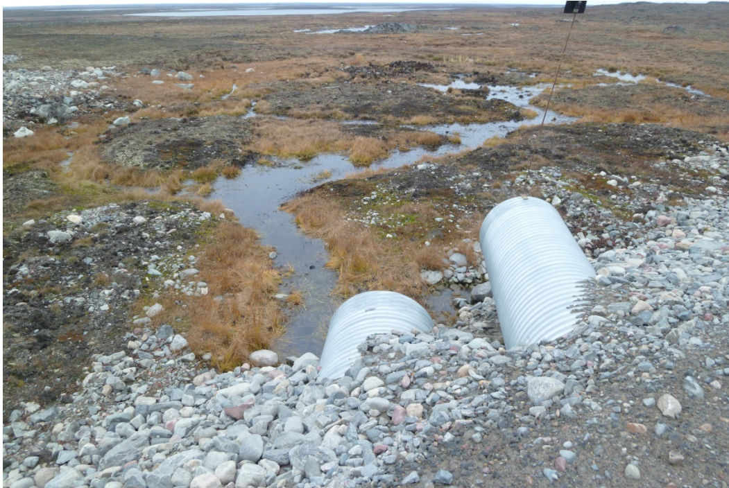
Photograph 13: Downstream View of Two CSP Culverts at KM 18.1 (20 September 2017)
