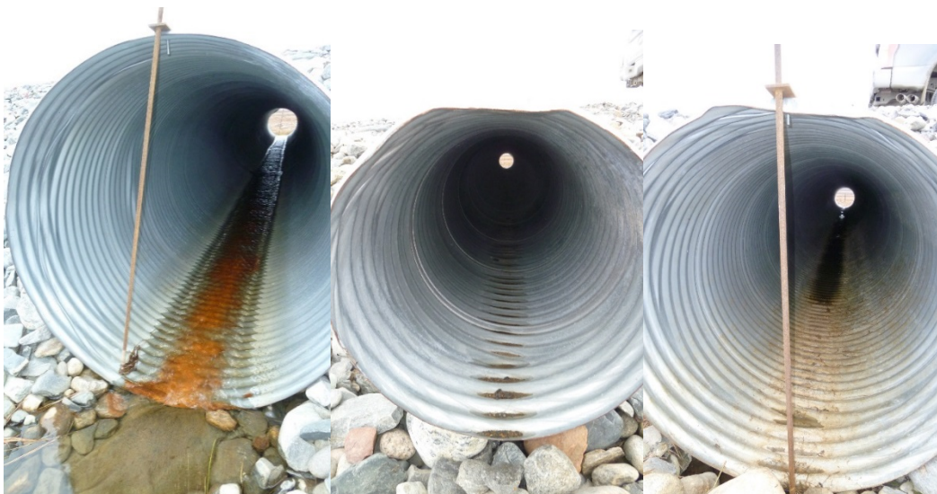
Photograph 6, 1 and 8: 3 CSP culverts at KM 16.3 from Upstream Looking Downstream. Good Condition, some Clear Flow in 1300 mm Ø Culvert. Good condition and no Flow for the 700 mm Ø (middle) and 1000 mm Ø (right) Culverts. (20 September 2017)
