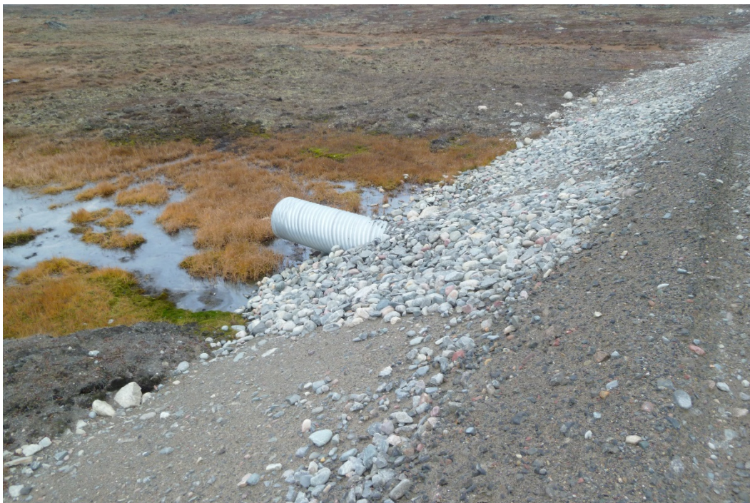
Photograph 18: Downstream End of 600 mm Ø CSP Culvert at KM18.15 (20 September 2017)
