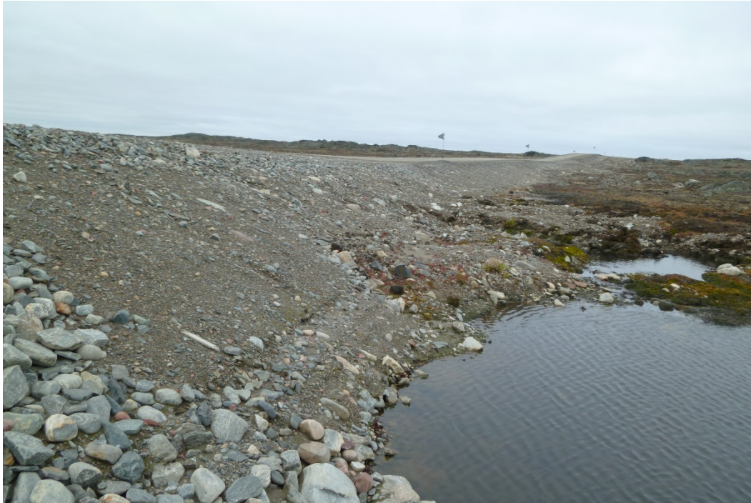
Photograph 17: View of The Road Embankment North of Upstream End Of 600 Mm Ø CSP Culvert at KM18.15. Some Erosion Observed on Embankment (20 September 2017)
