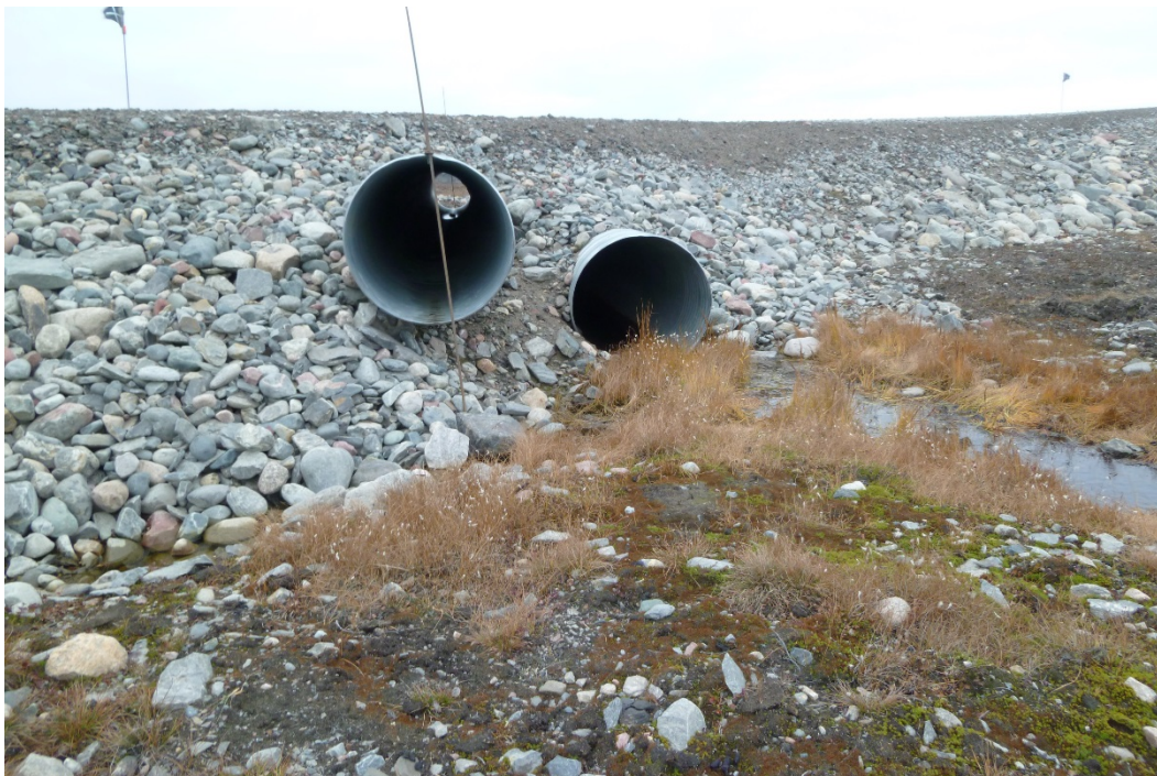
Photograph 14: Downstream Ends of the Two CSP Culverts at KM 18.1 (20 September 2017)
