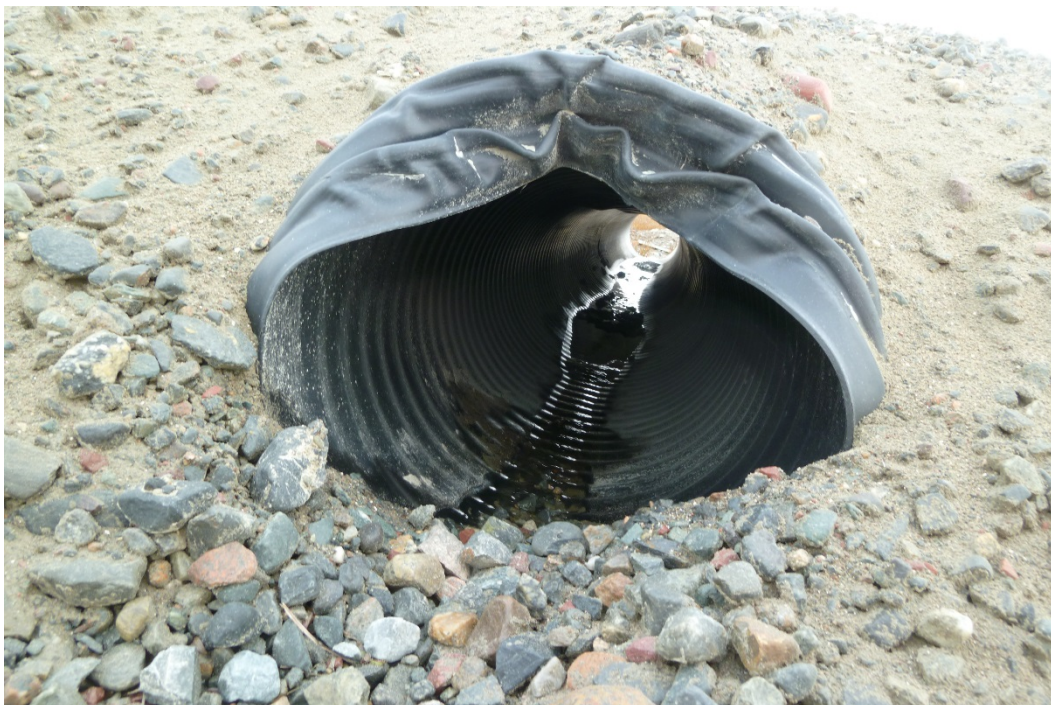
Photograph 30: Looking at the Inlet of the Culvert from Upstream to Downstream, 600 mm Ø HDPE, at KM25.8 (22 September 2017)
