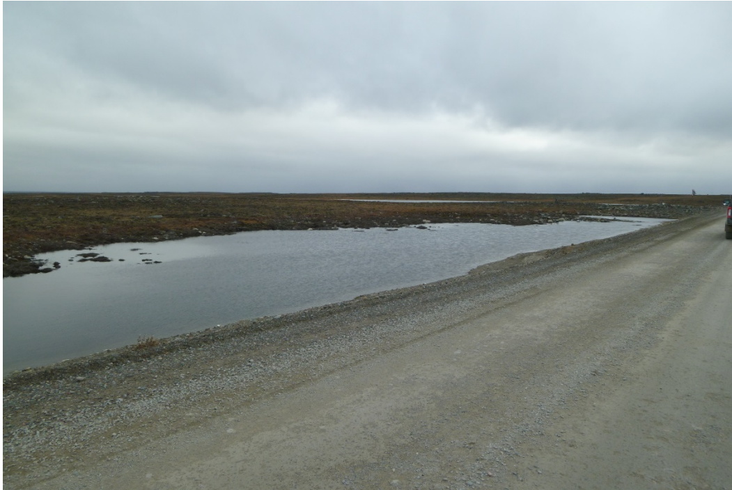
Photograph 27: Ponded Water on East Side of the Road Near KM22.7 (22 September 2017)
