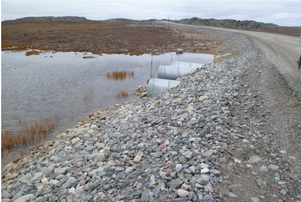
Photograph 5: KM16.3, Upstream Ends of 3 CSP Culverts from Front to Back of Photo: 1000 mm, 700 mm, and 1300 mm Ø Looking South (20 September 2017)
