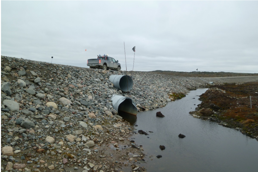
Photograph 11: View of Upstream Ends of Two CSP Culverts at KM18.1, Upper is 900 mm Ø and the Lower is 1000 mm Ø, Looking North to Single 600 mm Ø CSP at KM18.15 in Background of Photo. Cover Over Upper (900 mm Ø) Culvert is Thin on Upstream Side (20 September 2017)
