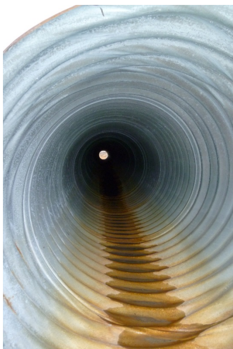
Photograph 16: View through 600 mm Ø CSP Culvert at KM18.15 from Upstream end (20 September 2017)
