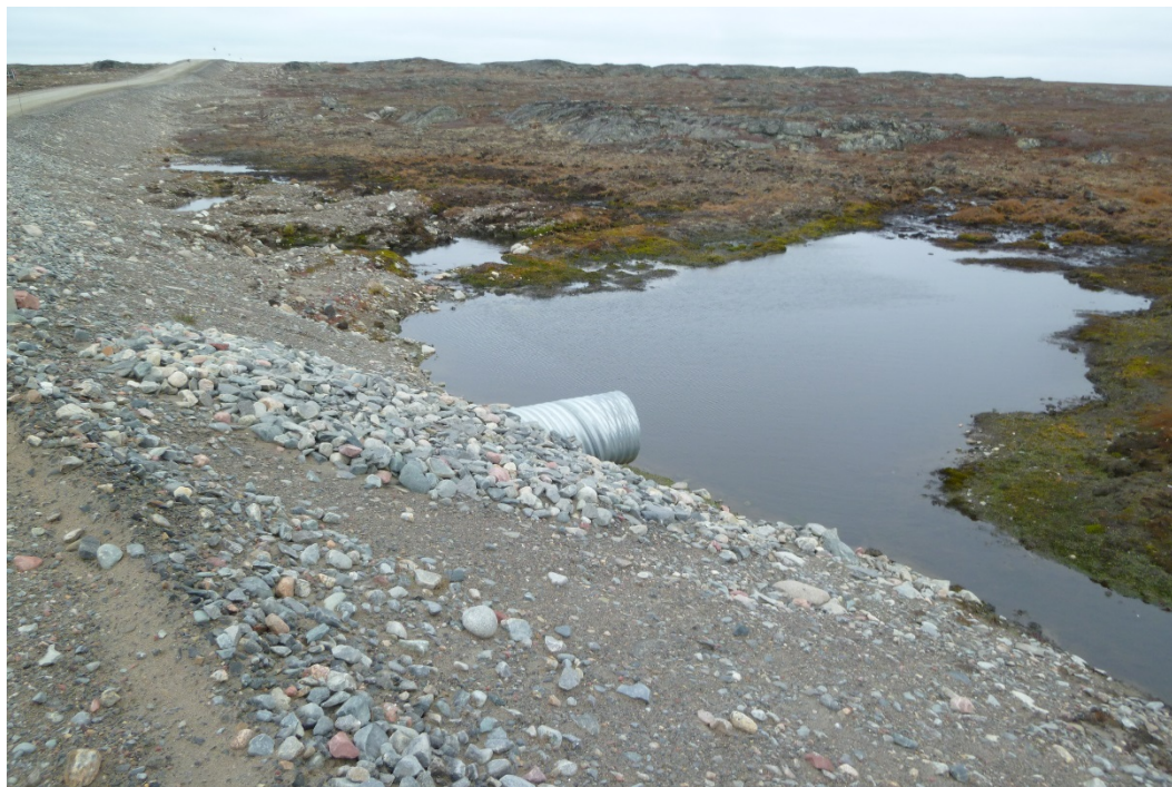
Photograph 15: Upstream End of 600 mm Ø CSP Culvert at KM18.15 (20 September 2017)
