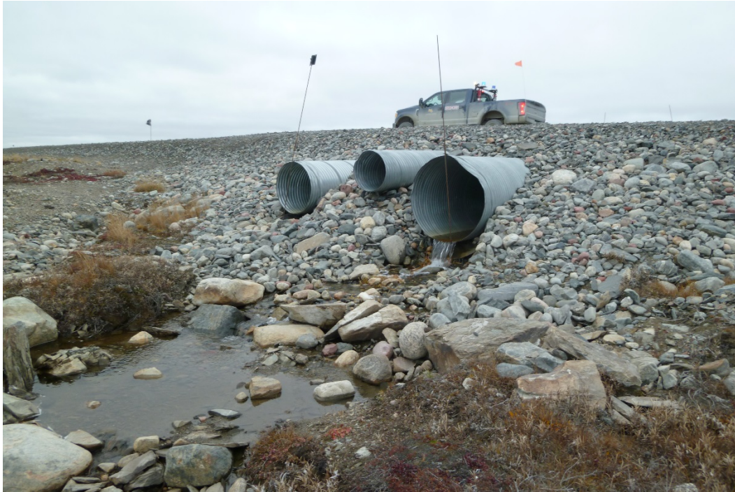
Photograph 9: Downstream Ends of Three CSP Culverts at KM16.3. Small Flow in 1300 Ø Culvert, Minor Deformation of End of Culvert. Small Erosion Visible at Outlet (20 September 2017)
