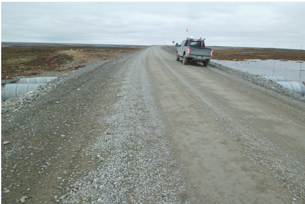
Photograph 10: Road Over 3 CSP Culverts, at KM16.3 Looking North (20 September 2017)
