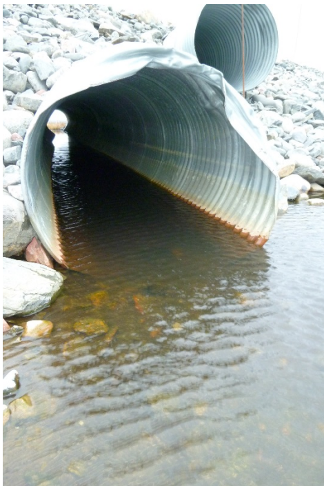
Photograph 12: View Through 1000 mm Ø CSP Culvert at KM18.1 From Upstream Side. Some Damage to Inlet of Culvert (20 September 2017)
