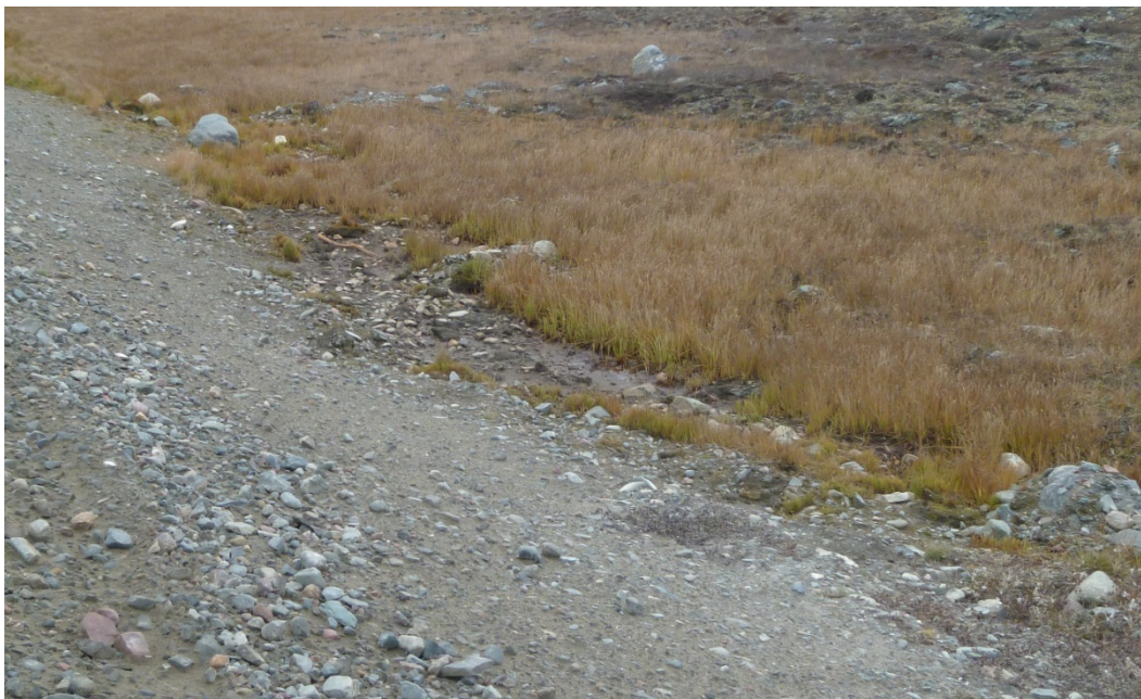
Photograph 28: Wet Ground on West side of Road Indicating Possible Seepage through Road Near KM22.7 (22 September 2017)
