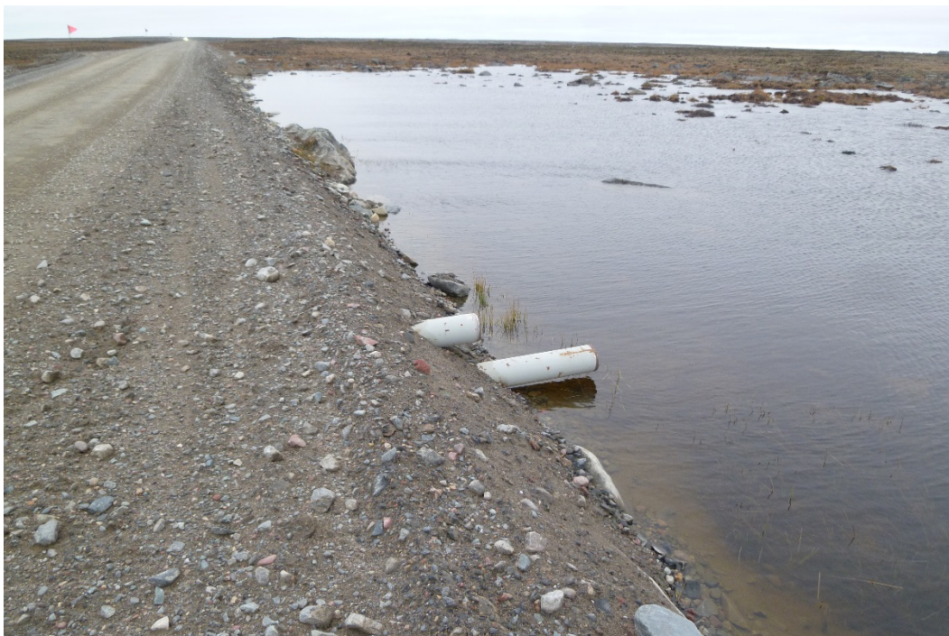
Photograph 24: KM22.3, There are Two Steel Pipes Vertically Offset, 160 Mm Ø. Looking at Upstream Ends. Inlets are Elevated, Could Be Installed at a Lower Elevation to Reduce Poned Water Along Road (20 September 2017)
