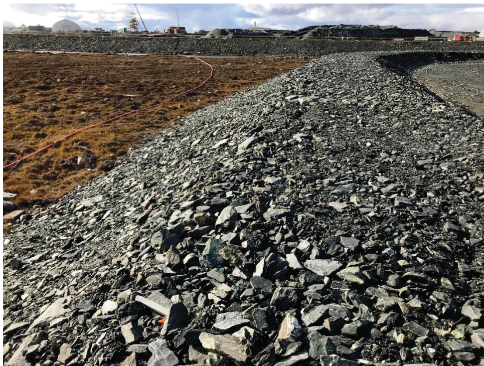
Photograph 47: Saline Pond, Southwest Perimeter Berm Looking Northwest, Cracking Along Downstream Crest. This Cracking was not Observed in 2017 (12 September 2018)
