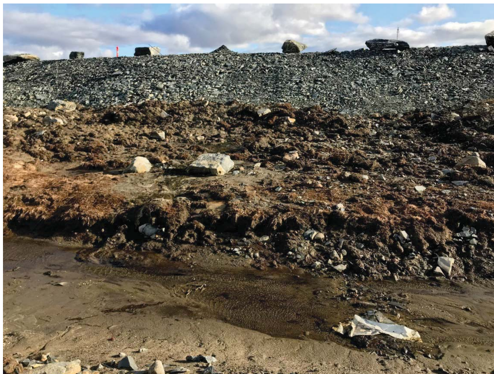
Photograph 15: DP1-B, Clear Seepage Visible from Dike Toe near Station 0+190. Less Seepage at This Location than in 2017 (12 September 2018)
