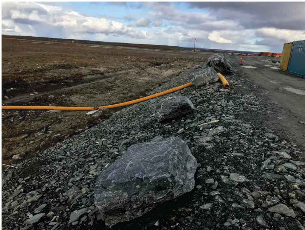
Photograph 11: DP1-B, Downstream Slope, Looking East. Orange Delineator on Crest Marks Thermistor Location (12 September 2018)
