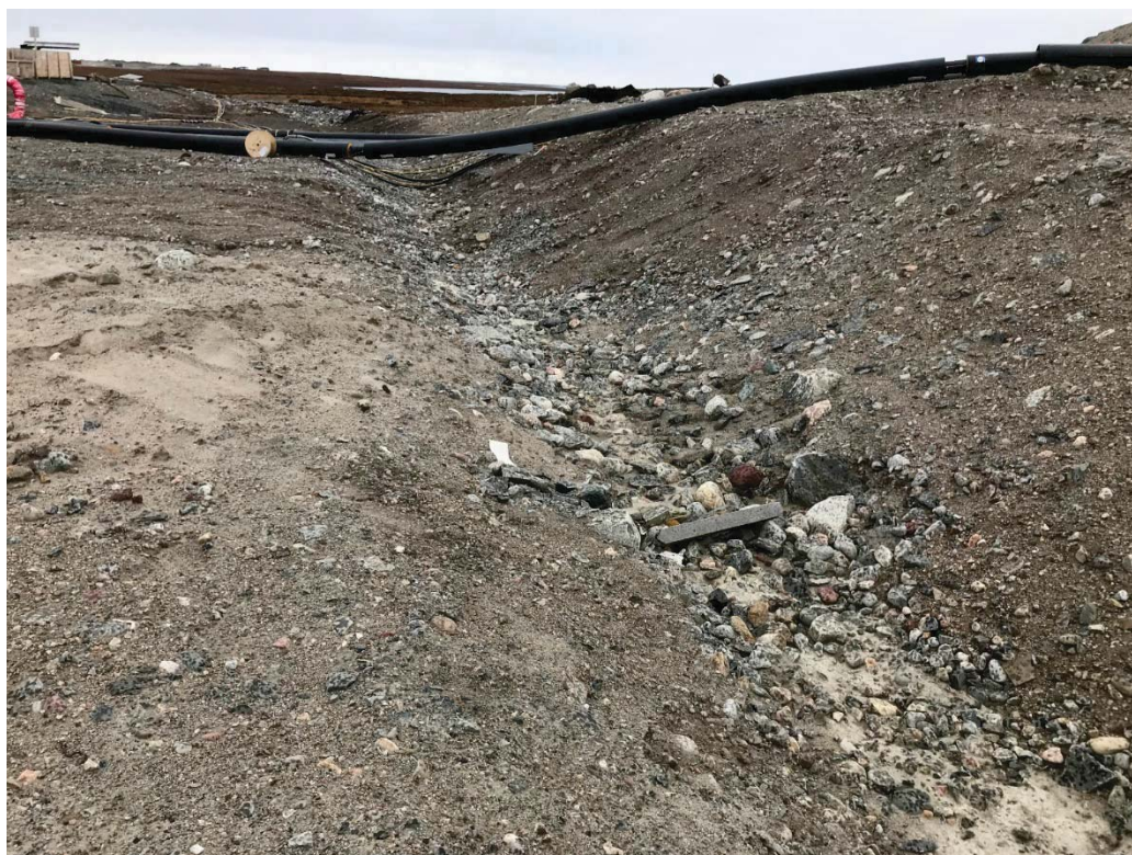
Photograph 57: Channel 2, Unlined Extension of East End of Channel 2, Looking Northwest (11 September 2018)
