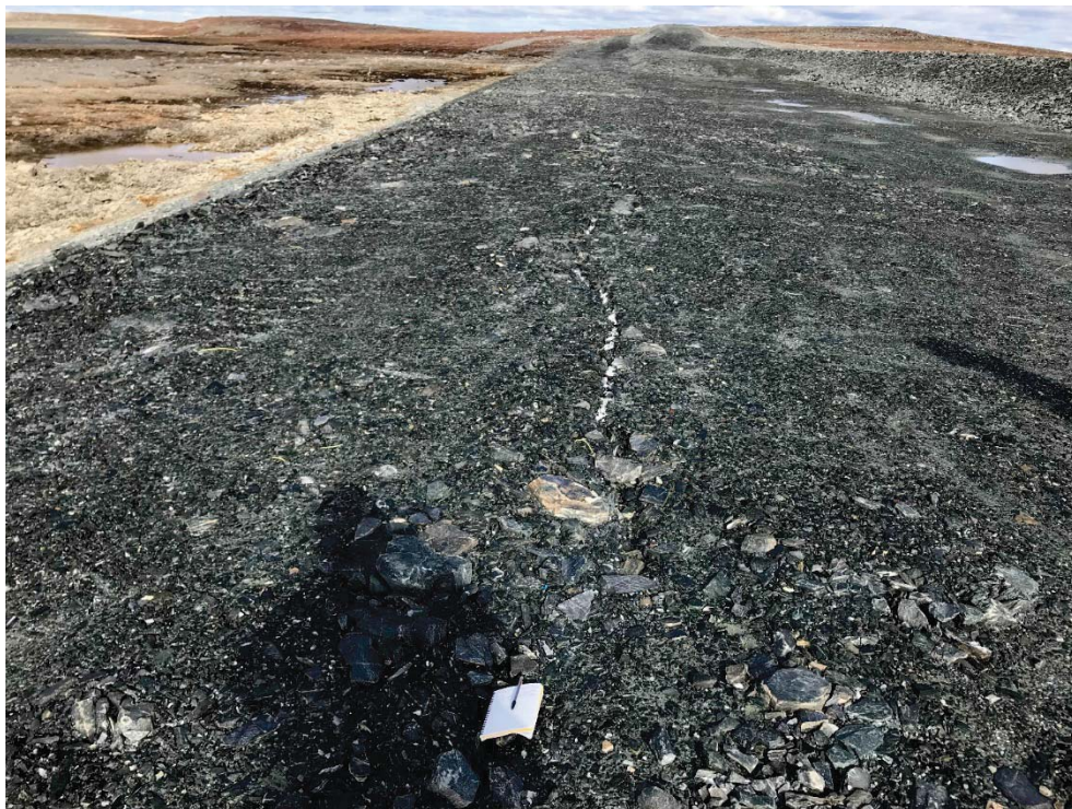
Photograph 9: D-CP1, Cracking on Upstream Bench Crest Near Station 1+450, Looking North. Similar Condition to 2017 (12 September 2018)
