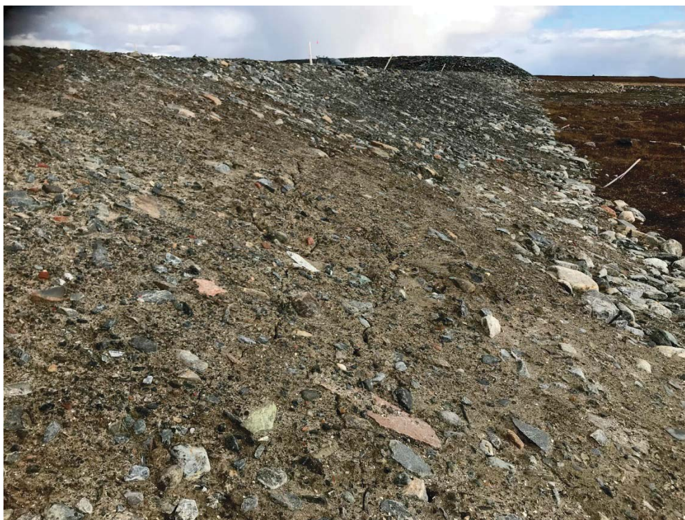
Photograph 77: Berm 3, Downstream Slope, Some Cracking Near Station 0+280, Looking North. Cracking was not Observed in 2017 (12 September 2018)
