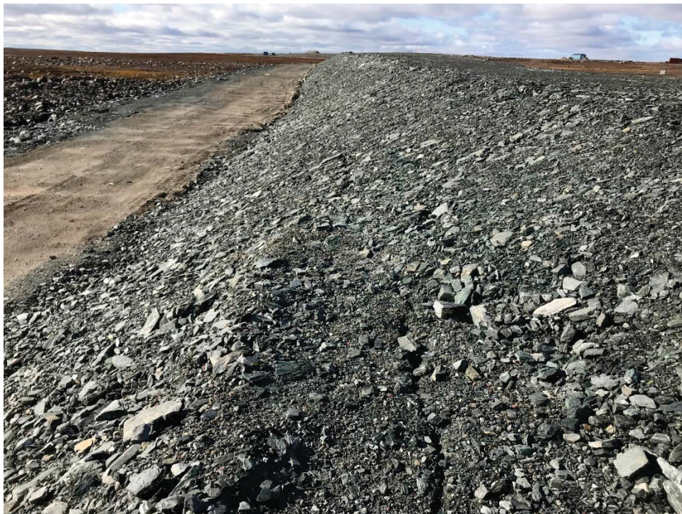
Photograph 41: D-CP5, Cracking in Downstream Slope Looking Southwest Near Station 1+175. This Cracking was not Observed in 2017 (12 September 2018)
