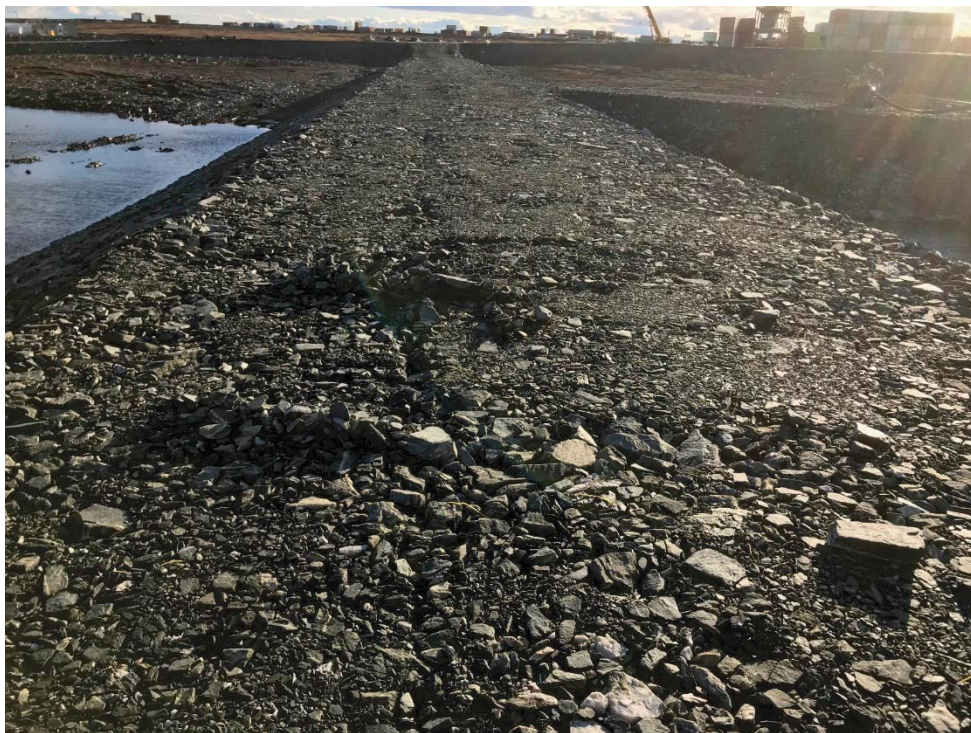
Photograph 4: DP1-A, Cracking Observed on Crest, Similar Condition to 2017 (12 September 2018)
