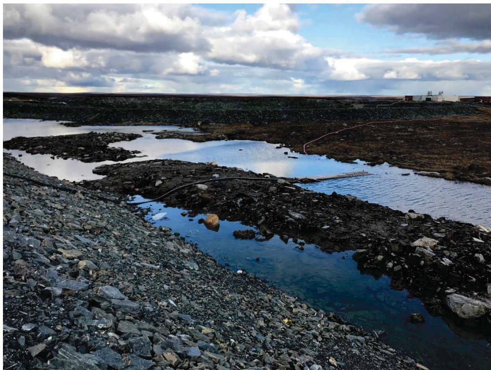
Photograph 35: View Northeast of the Saline Pond from near Station 0+150 of DP3-A. Clear Seepage Water Poned in Downstream Collection Channel and Along Dike Toe. More Poned Water than in 2017 (12 September 2018)
