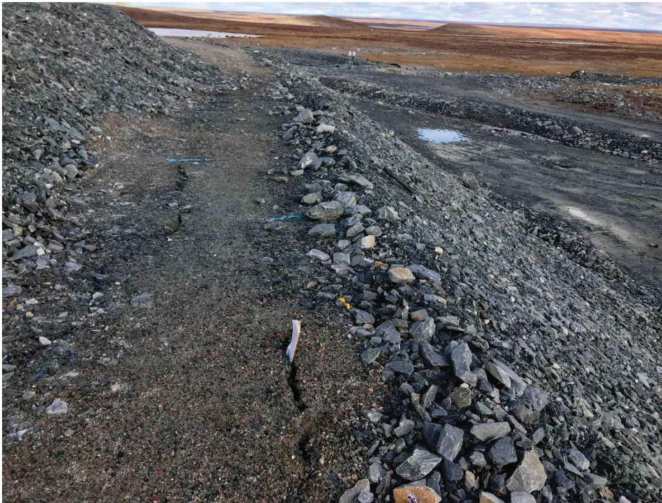
Photograph 19: D-CP1, Cracking on Downstream Bench Near Station 1+145, Looking Northeast. Cracks are Wider and Deeper Than in 2017 (12 September 2018)
