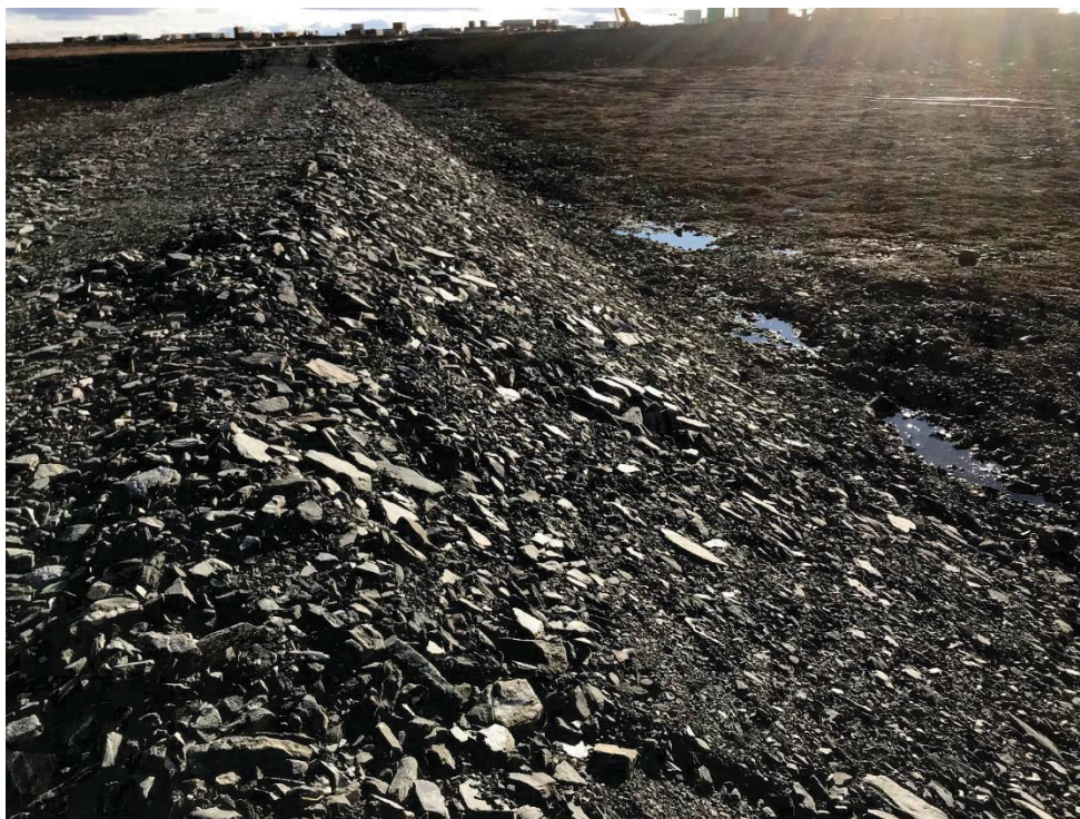
Photograph 3: DP1-A, North Slope Looking Southwest, Minor Slumping that was not observed during 2017 inspection (12 September 2018)
