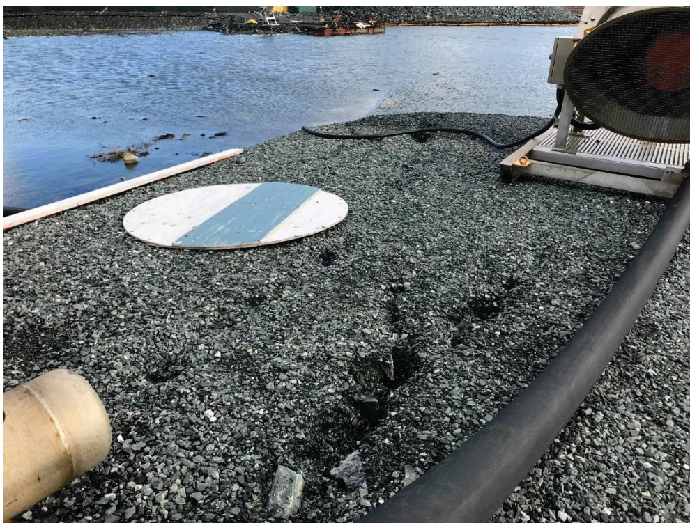
Photograph 12: DP1-B, Cracking on Crest of Jetty 2 has Increased Slightly from 2017. No cracking observed at Jetty 3 or Jetty 4 during inspection (12 September 2018)
