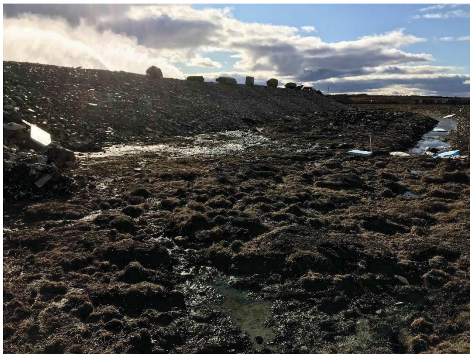
Photograph 13: DP1-B, Downstream Slope near Station 0+300, Looking West. Minor Seepage from Downstream Toe, Similar to 2017, Entering Collection Channel to Right of Photograph (12 September 2018)
