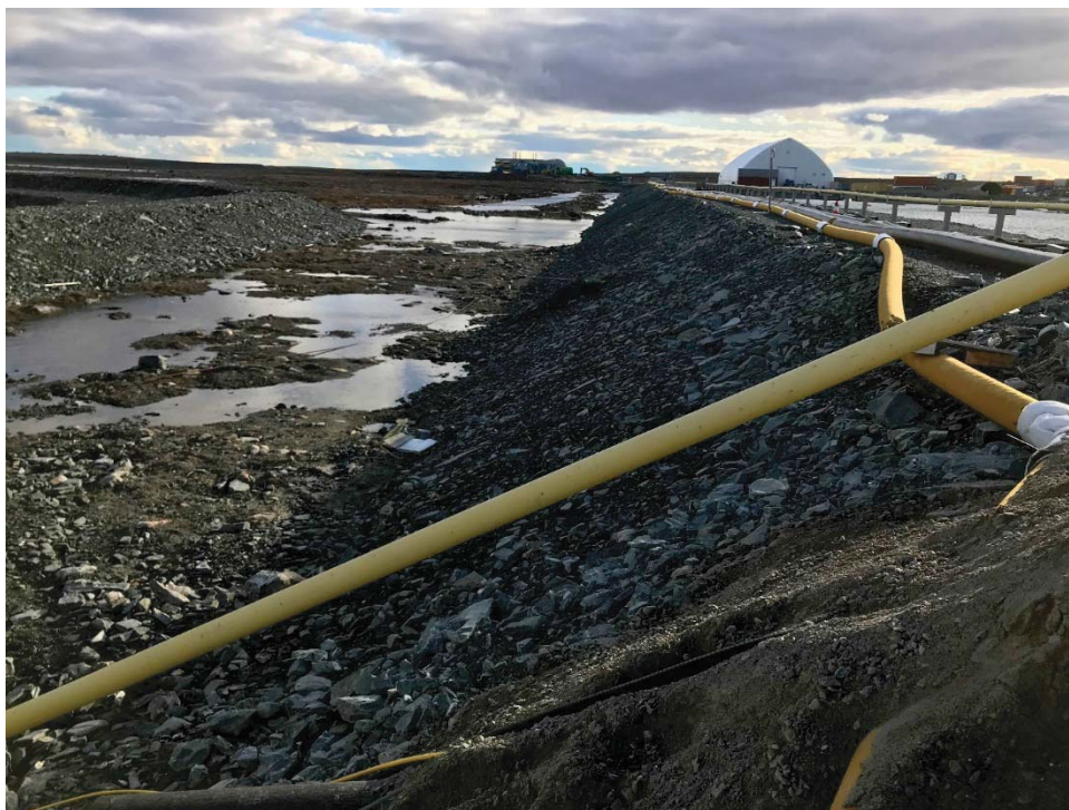
Photograph 30: DP3-A, Downstream Slope and Seepage Collection Channel, Looking Southwest near Station 0+300. More Water Pooled Downstream than in 2017 (12 September 2018)
