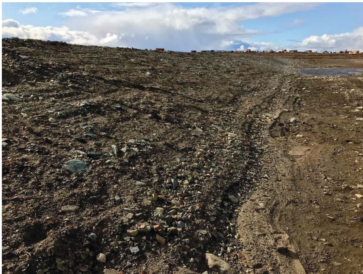
Photograph 78: Berm 3, Upstream Slope, Erosion at Toe and Along Slope from Previous High Water Mark, Near Station 0+230, Looking Northwest (12 September 2018)
