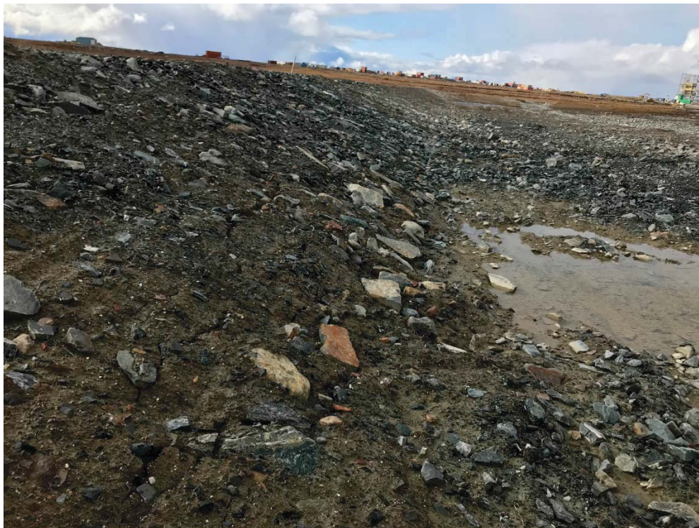
Photograph 76: Berm 3, Upstream Slope, Some Cracking Near Station 0+280, Looking North. This Cracking was Not Observed in 2017 (12 September 2018)
