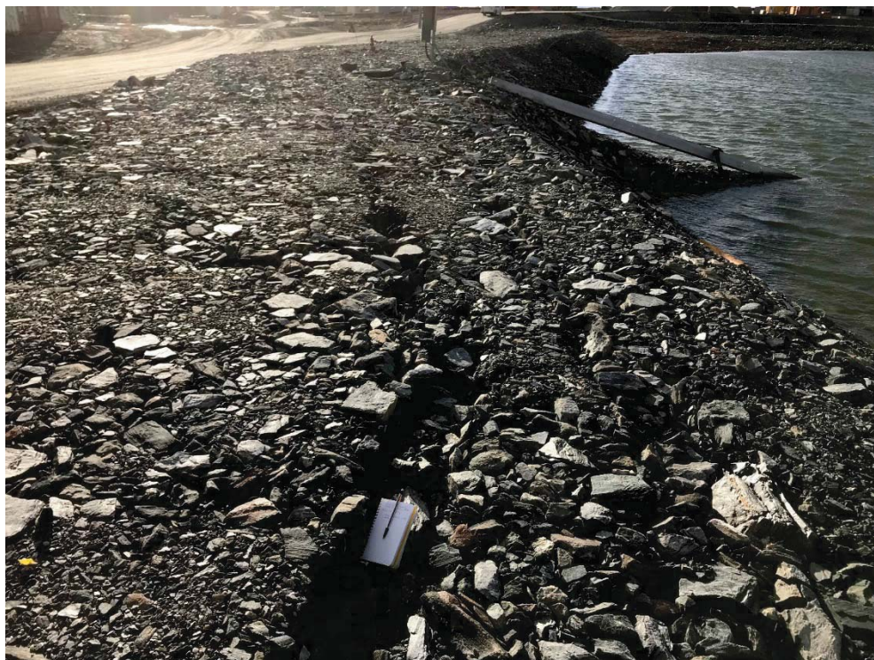
Photograph 27: DP2-A, Cracking near Station 0+100, looking West. (12 September 2018)
