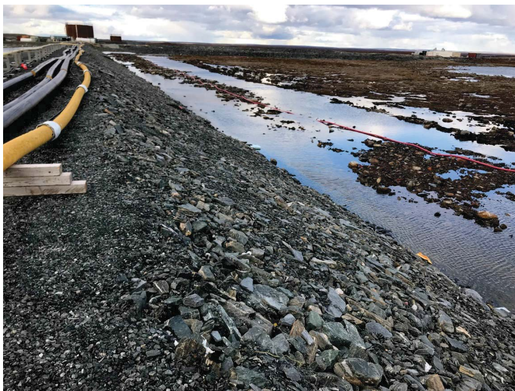
Photograph 36: DP3-A Downstream Slope and Seepage Collection Channel, looking Northeast near Station 0+40. More Poned Water Downstream than in 2017 (12 September 2018)
