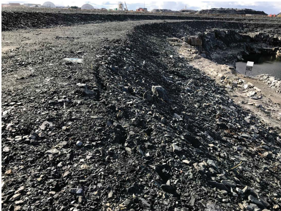
Photograph 48: Saline Pond, Southeast Perimeter Berm Cracking in Upstream Crest, Looking Northwest. This Cracking was not Observed in 2017 (12 September 2018)
