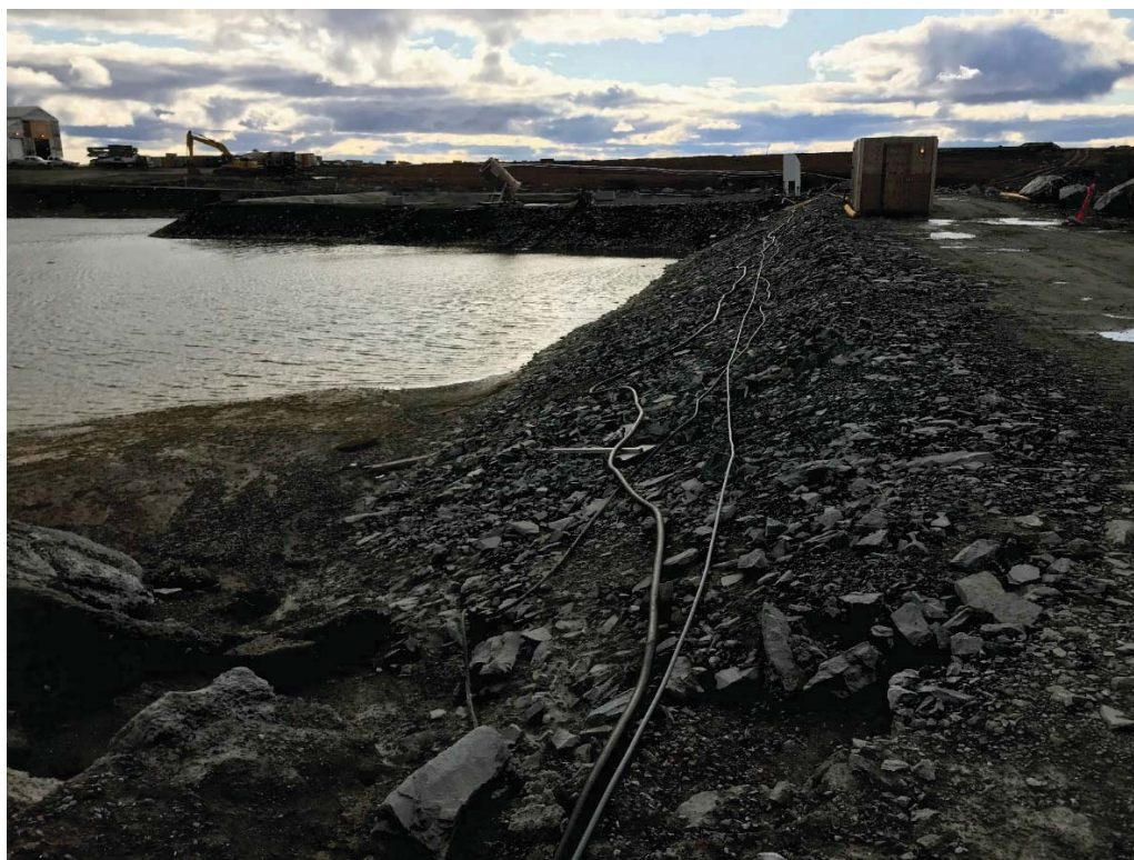
Photograph 10: DP1-B, Upstream Slope from Jetty 2 Looking East toward Snow Melt Management Pond, Minor Erosion on Slope (12 September 2018)
