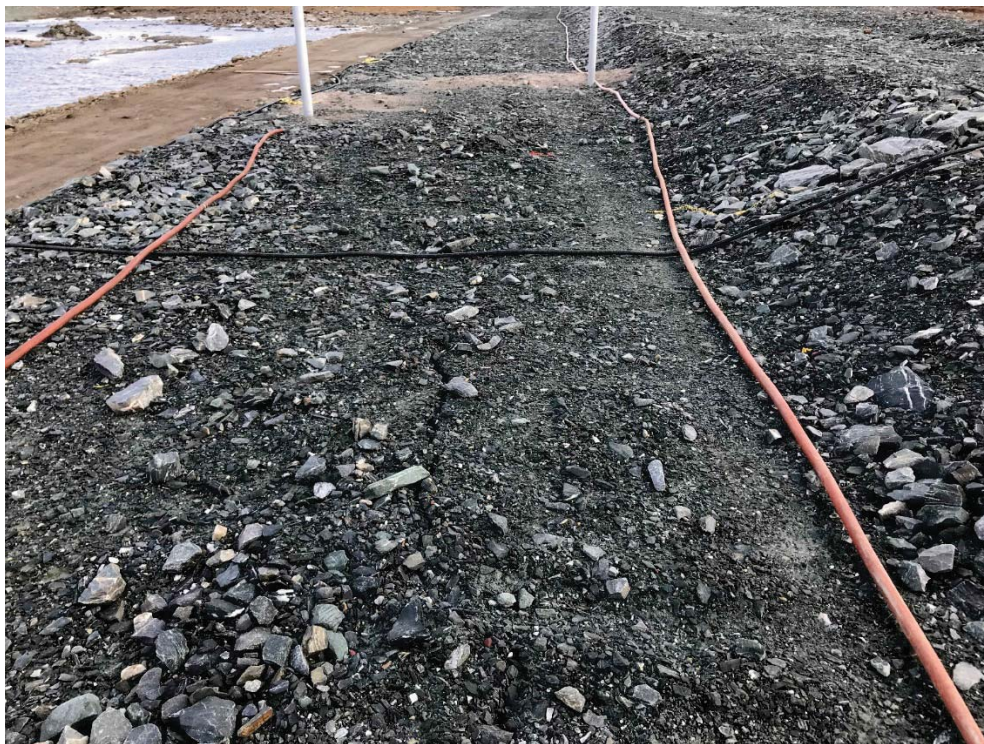
Photograph 34: D-CP5, Cracking on Upstream Bench Looking Northeast Near Station 1+180. This Cracking was not Observed in 2017 (12 September 2018)
