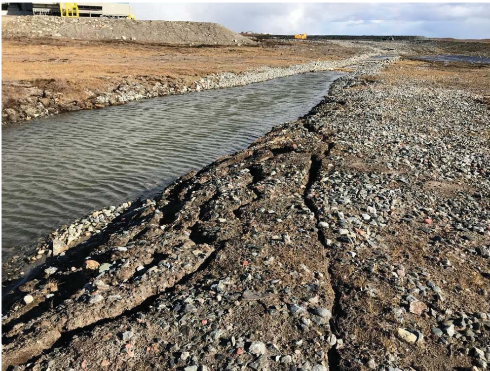
Photograph 71: Channel 5, Water Poned in Channel and Cracking Along South Slope of Trench Near Station 0+050, Looking Southwest. This Cracking was Not Observed in 2017 but Access to This Area was Limited due to Water Levels and Saturated Conditions in the Tundra (12 September 2018)
