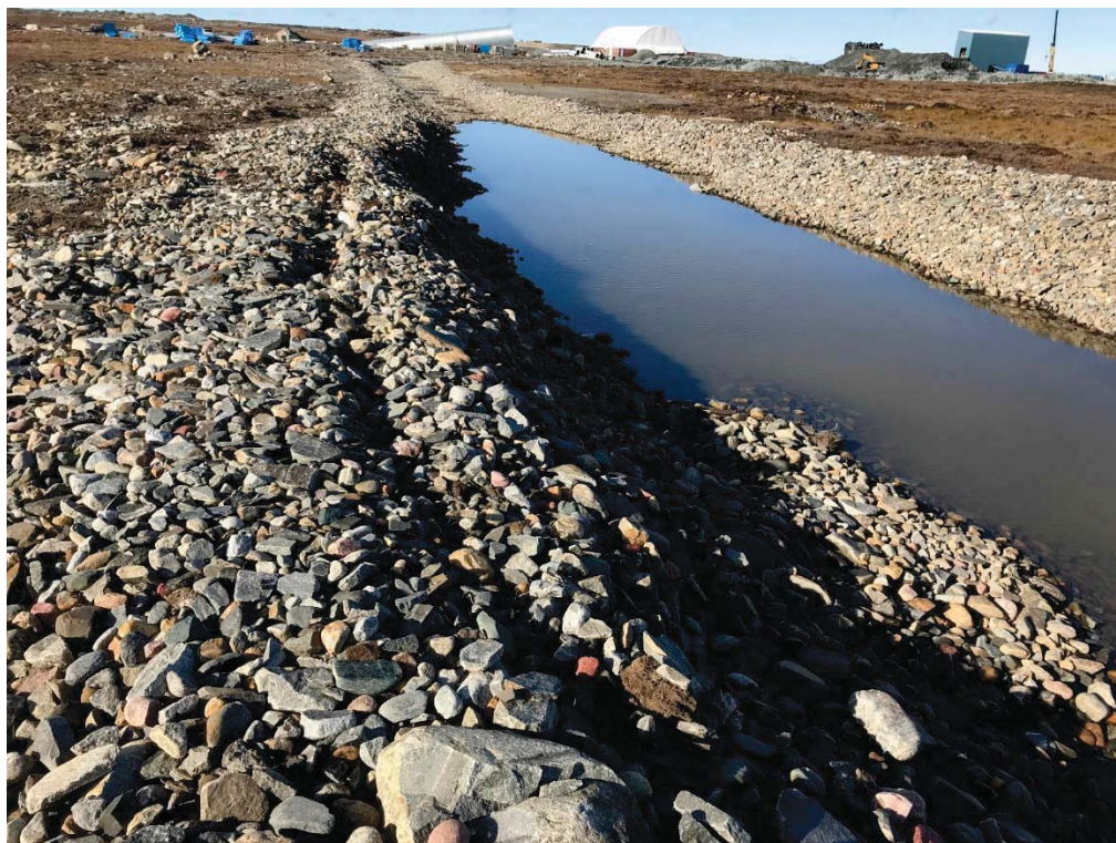
Photograph 52: Channel 1, Small Slump and Crack along the South Slope Crest About 30 m West from Outlet of Channel (13 September 2018)
