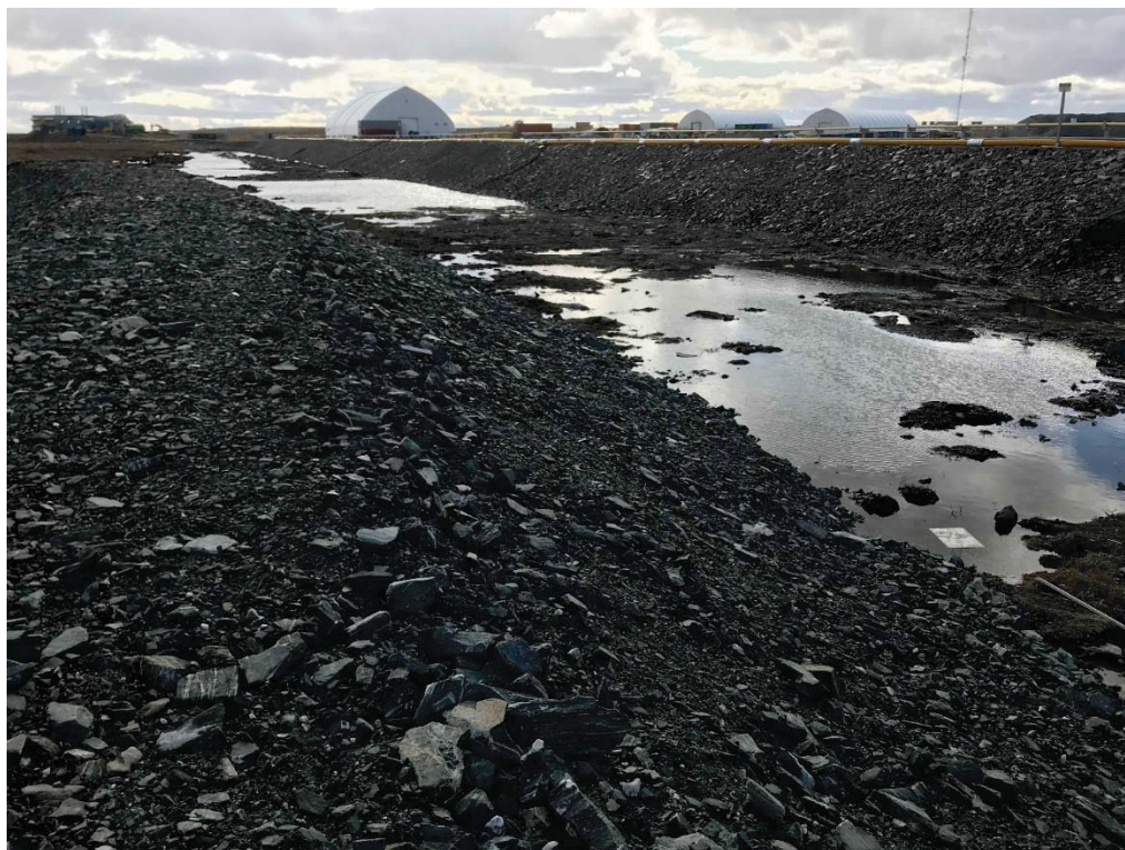
Photograph 50: Saline Pond, Downstream Slope of the Northwest Perimeter Berm and Water Ponded Between Saline Pond and DP3-A (12 September 2018)
