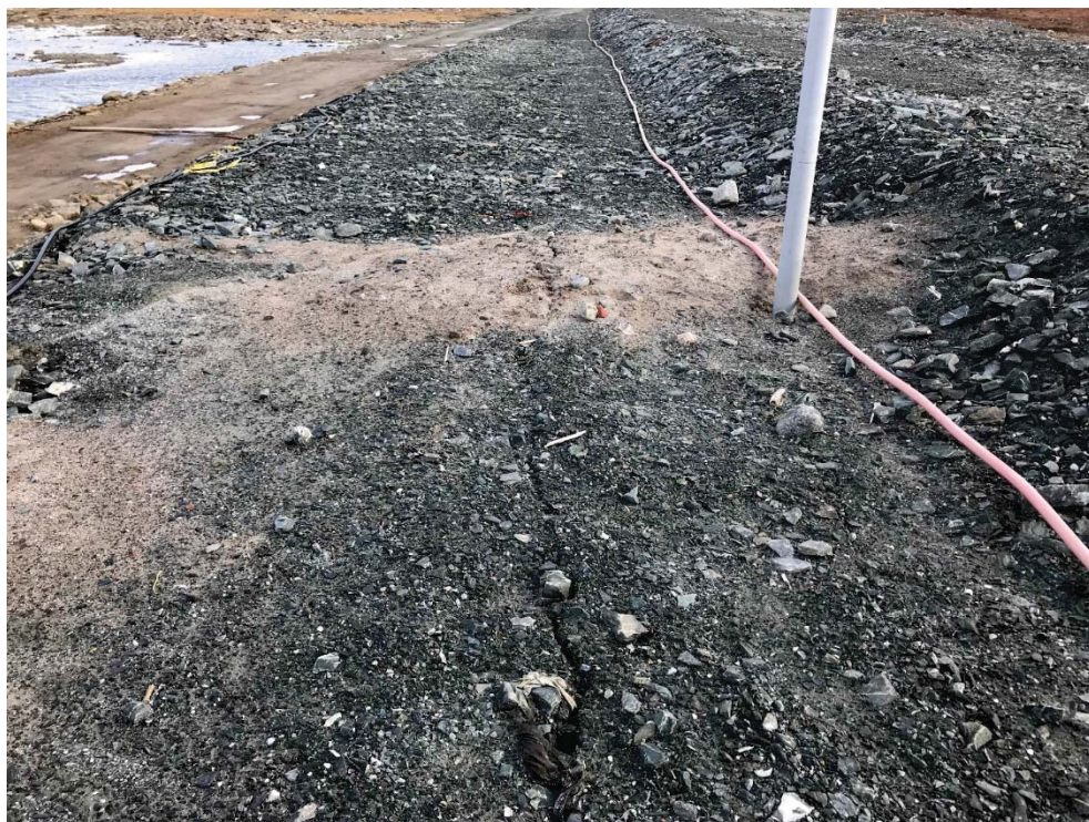
Photograph 35: D-CP5, Cracking on Upstream Bench Looking Northeast Near Station 1+185. This Cracking was not Observed in 2017 (12 September 2018)
