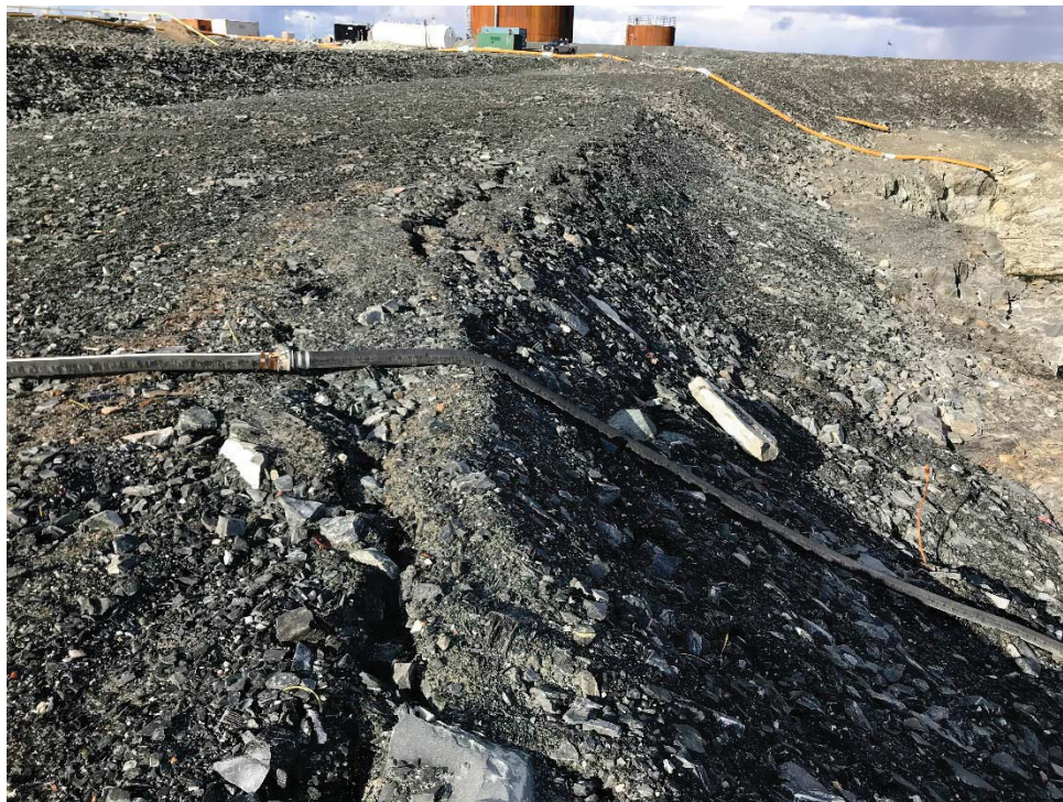
Photograph 46: Saline Pond, Cracking in Northwest Perimeter Berm Looking Southeast. Cracking and Slumping have Increased Slightly from 2017 (12 September 2018)
