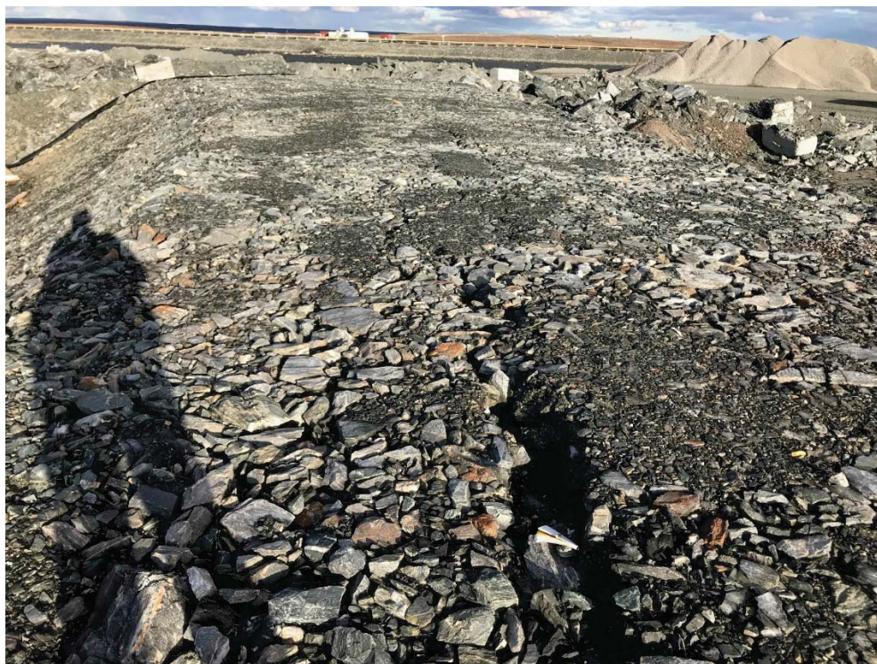
Photograph 28: DP2-A, Cracking near Station 0+100, looking East. The Length of the Cracking in This Area of the Dike was Similar to 2017, but the Cracks were Wider and Deeper (12 September 2018)
