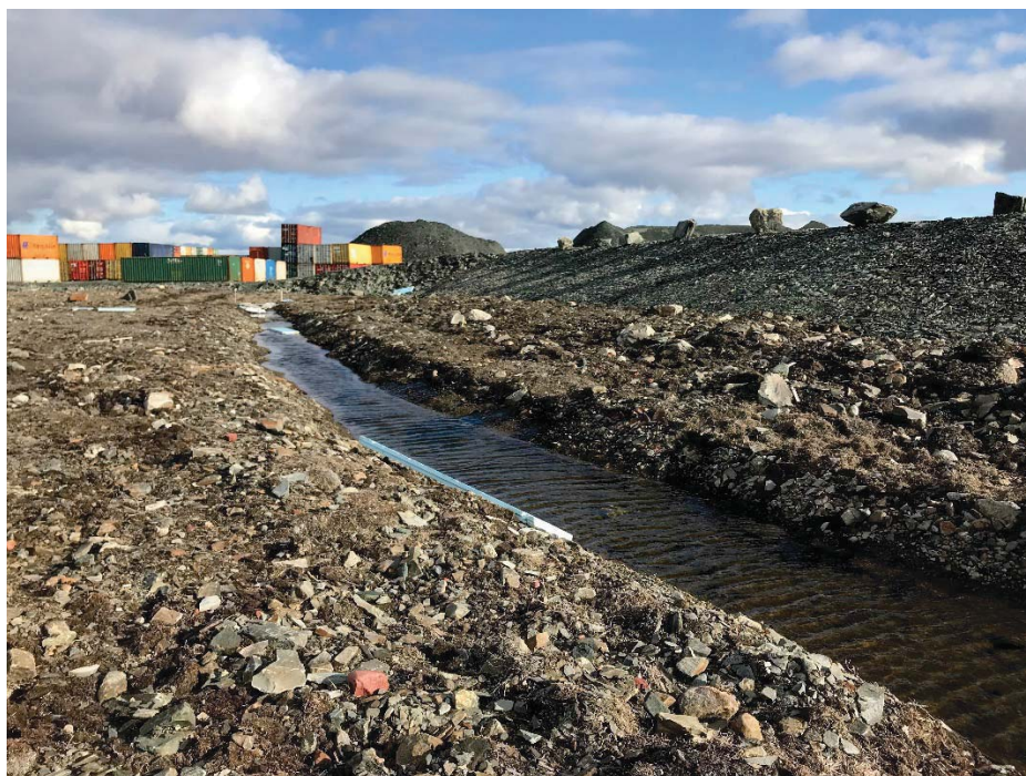
Photograph 14: DP1-B, Run-off and Seepage Collection Channel Downstream of Dike, Looking East. Seepage in Channel was Clear and at a Similar Level to 2017 (12 September 2018)
