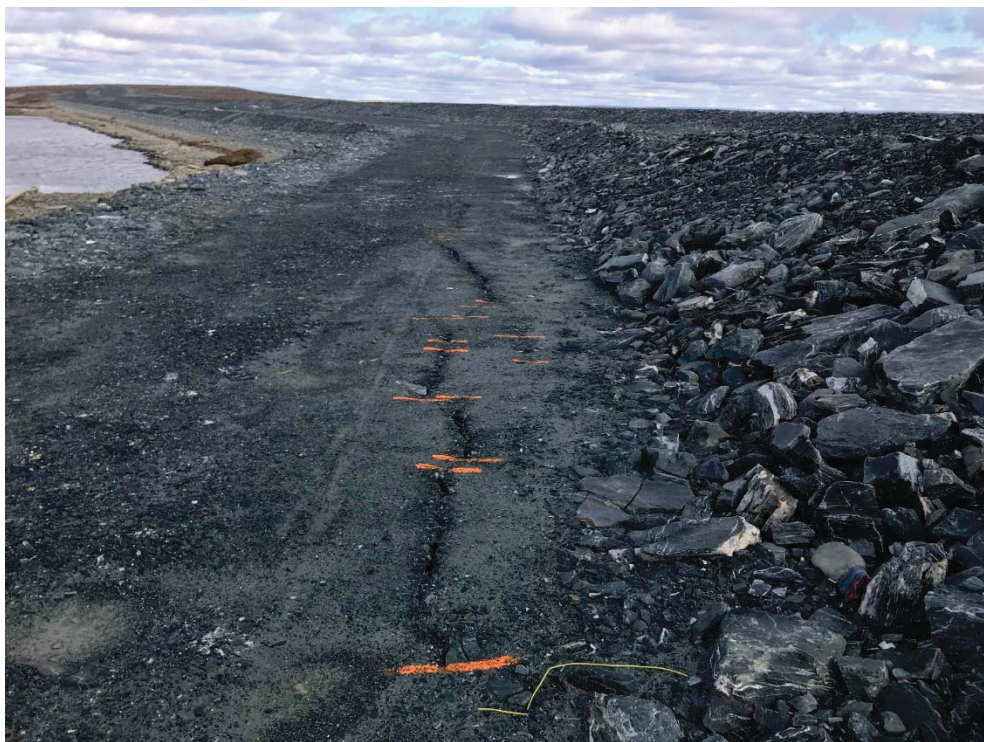
Photograph 4: D-CP1, Cracking on Upstream Bench Crest Near Station 1+150, Looking Northeast. Length of Cracking had Increased Slightly from 2017 Observations and Minor Increase in the Widths of the Cracks (12 September 2018)
