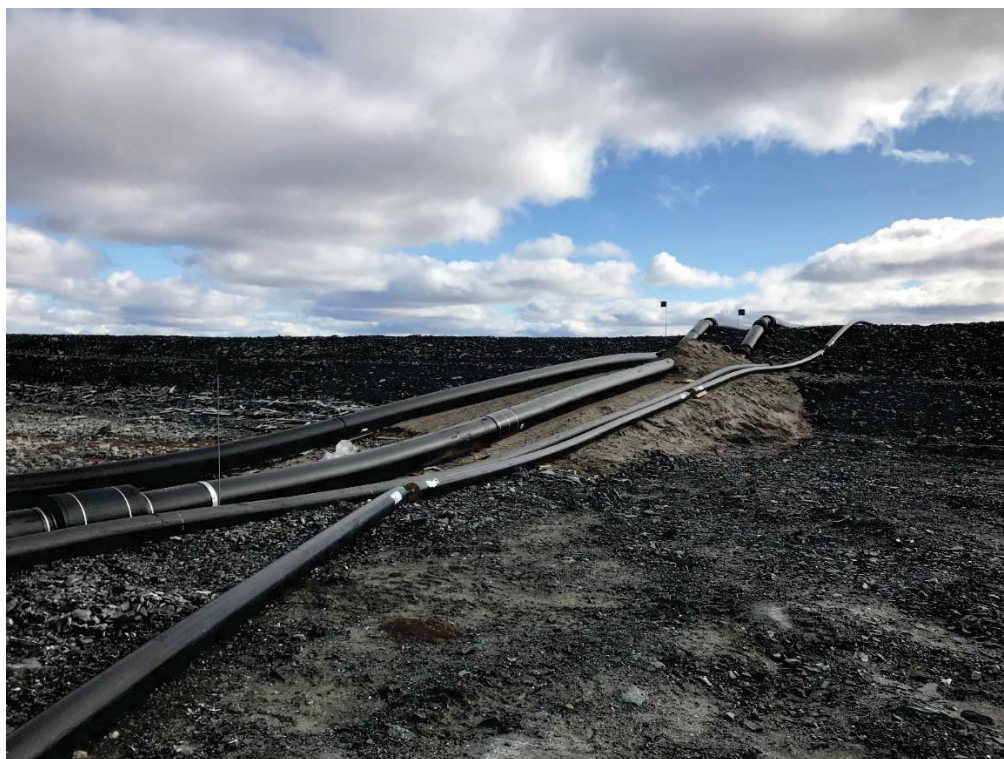
Photograph 2: D-CP1, Water Pipeline Ramp Upstream of Dike Near Station 1+140, Looking South. Some Minor Erosion Observed that was not Observed in 2017 (12 September 2018)
