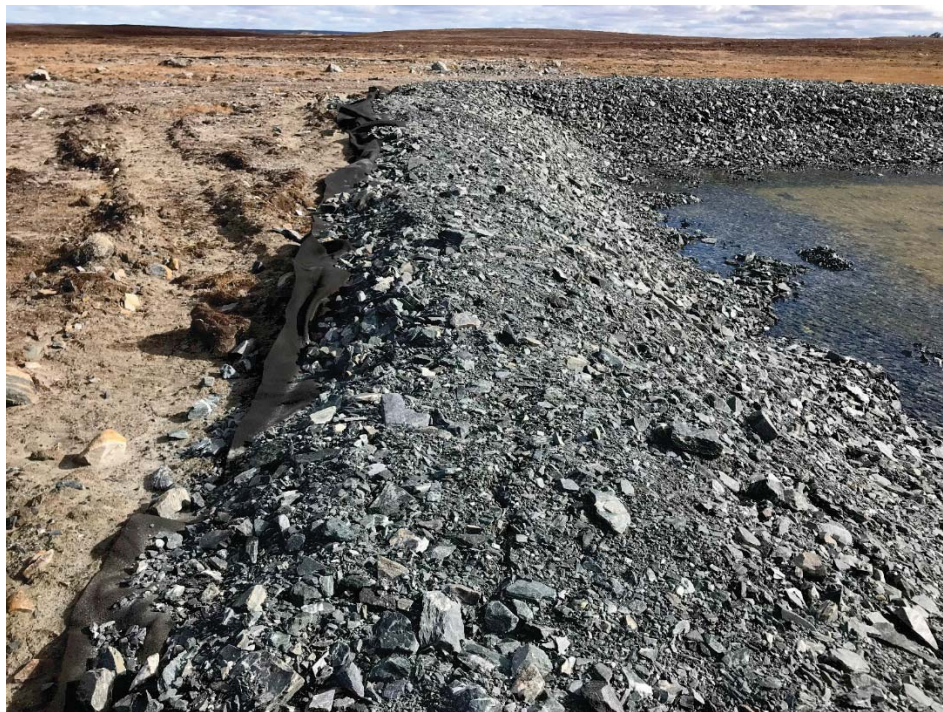
Photograph 26: D-CP1, Cracking/Slumping in North Side of Downstream Sump, Looking East. Similar Condition to 2017 (12 September 2018)
