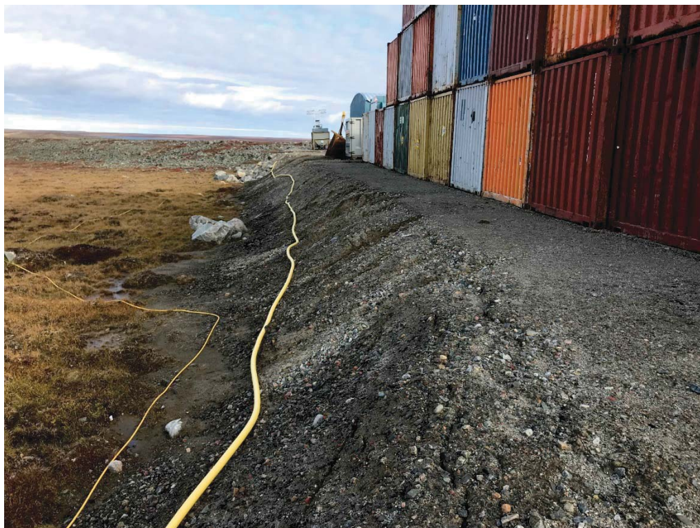
Photograph 53: Emulsion Plant Pad, Erosion and Cracking on East Slope, Looking North. (14 September 2018)
