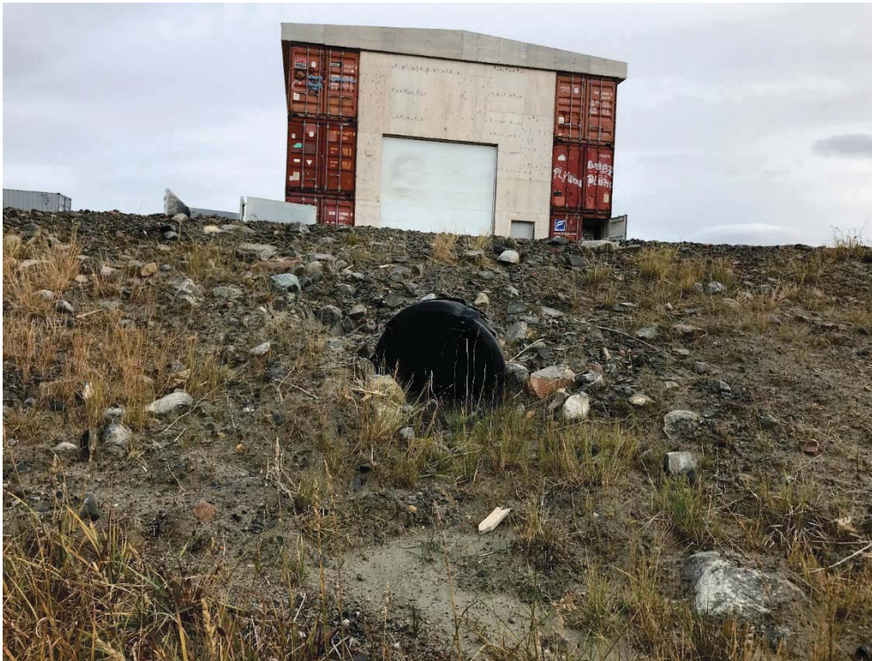
Photograph 23: Exploration Camp Access Road, Downstream End of Culvert on North Side of Camp, not exposed on upstream (10 September 2018)
