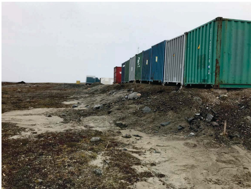
Photograph 41: Erosion of North Slope of Main Camp/Industrial Pad, Looking East. (11 September 2018)
