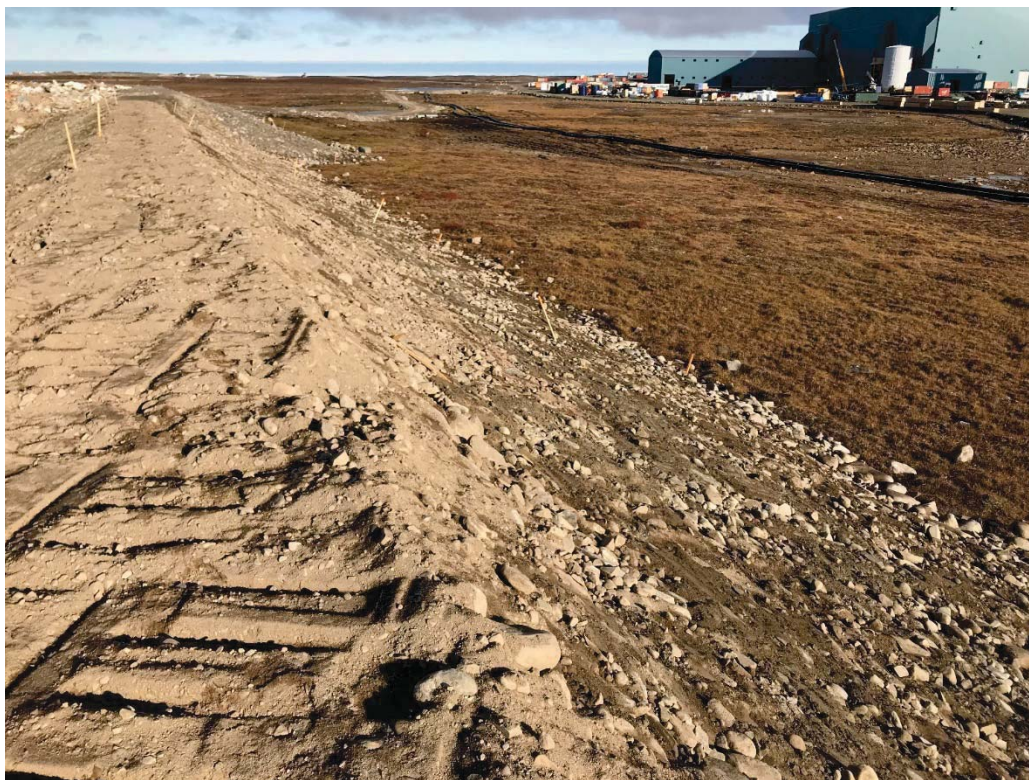
Photograph 34: Operations Landfill Expansion, Northeast Slope from the Southeast Corner of the New Landfill Expansion. Slopes of New Expansion are Steeper than Original Landfill Slopes (13 September 2018)
