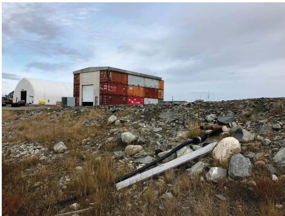
Photograph 26: Exploration Camp Access Road, Downstream Ends of Steel Pipes on Northwest Side of Camp, not exposed on upstream (10 September 2018)
