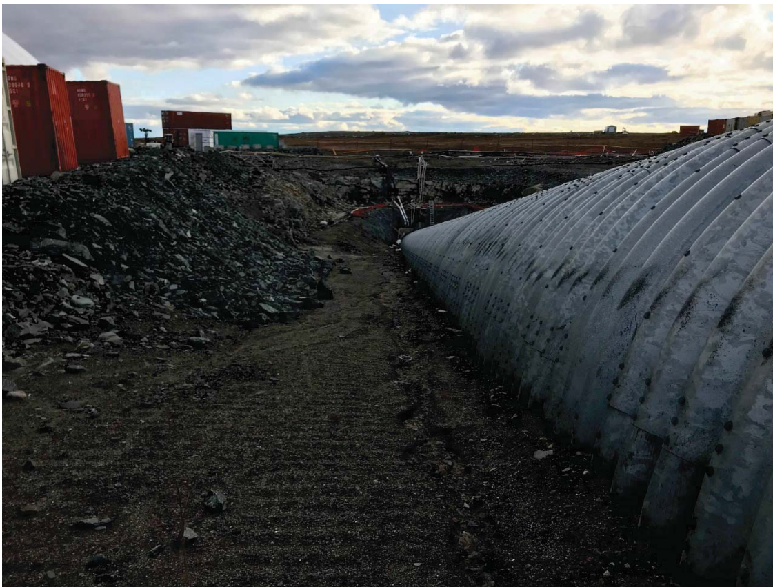
Photograph 12: Portal No. 1, View Down East Side, Looking South. Minor Erosion on Surface of Backfill (12 September 2018)
