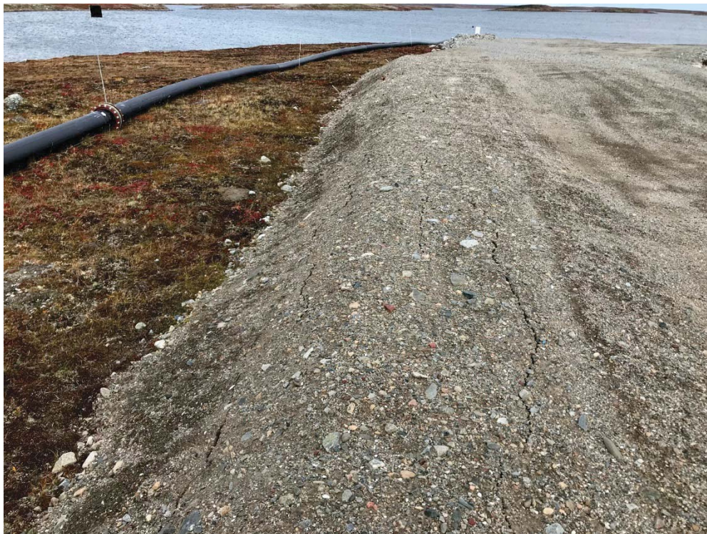
Photograph 19: Exploration Camp Diffuser Access Road, Minor Cracking on North Side of Road, Looking East (10 September 2018)
