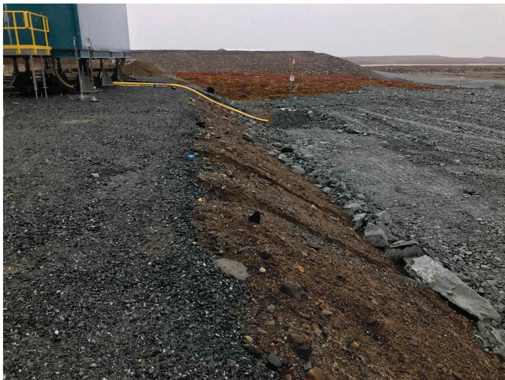
Photograph 47: South Slope of Incinerator Pad, Erosion of Esker Material on Slope, Crushed Material Placed as Pad Surface, Looking East. Placement of Rockfill for Construction of Ore Storage Pad 2 In Progress to South. (11 September 2018)
