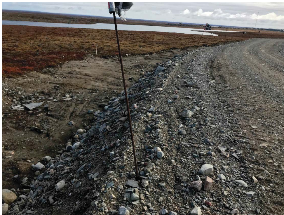
Photograph 21: Emulsion Plant Access Road, Looking Southeast from Near Dino Access Gate, Some Minor Cracking in Road Crest (14 September 2018)
