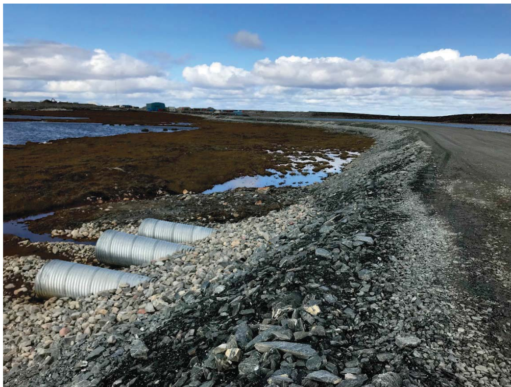
Photograph 8: Culvert #3, Upstream Ends of Culverts, Looking North. Service Road on Right (12 September 2018)
