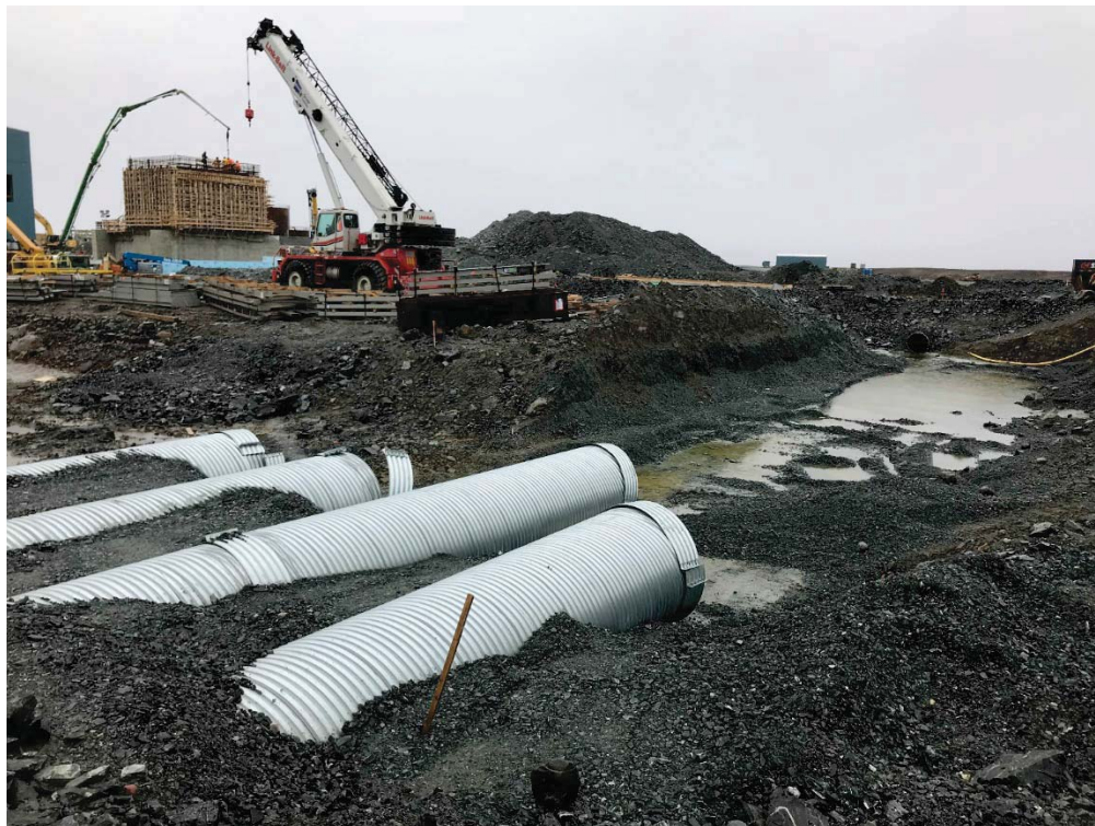
Photograph 7: Culvert #2, Downstream Ends of Culverts, Looking Southeast. Temporary Culvert in background. Culvert #2 to be Extended and Will Connect with Channel #1 (12 September 2018)
