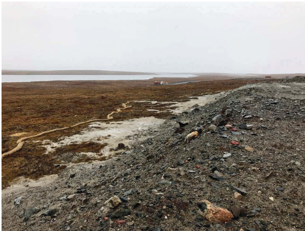
Photograph 29: Wesmeg Borrow, Erosion Along Western Toe, Looking North (11 September 2018)
