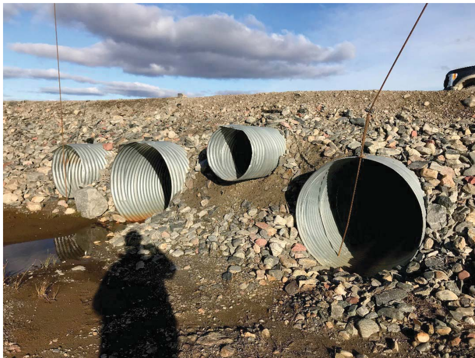
Photograph 48: Upstream ends of four CSP culverts at KM12.1. From left to right the diameters are 900 mm, 1300 mm, 700 mm, 1300 mm. Small dent in inlet of uppermost culvert (13 September 2018)
