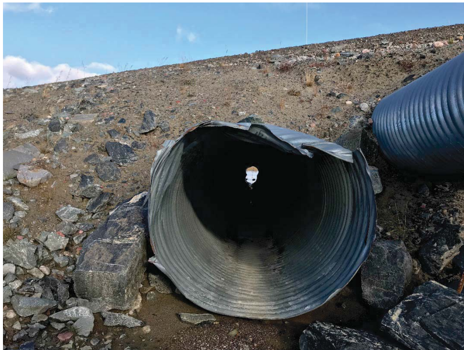
Photograph 19: Damaged upstream end of 900 mm culvert at KM7.4, similar to what was observed in 2017. It appears the damage may have been caused by boulders that rolled down the slope (13 September 2018)
