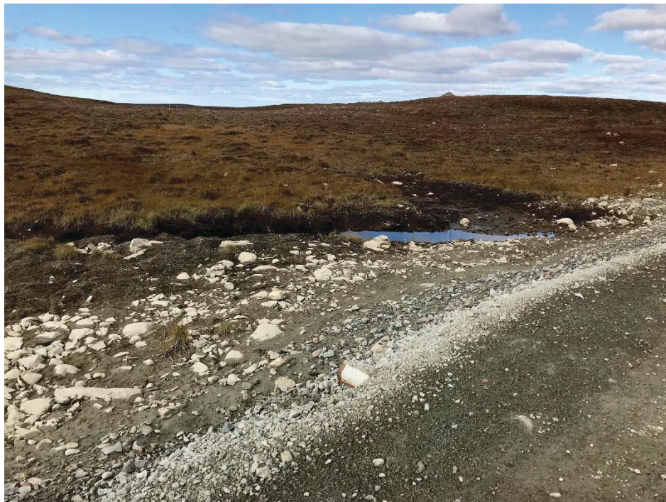
Photograph 103: At KM26.8, water ponded on west side of road north of culverts. Water is not against road, but should be monitored during higher water levels to assess if larger culverts needed. (14 September 2018).
