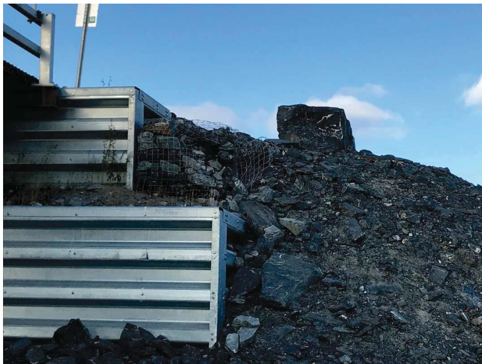
Photograph 41: M-5 Bridge at KM10.5, photo of damaged gabion on the downstream side of the Left (north) Abutment that should be replaced. (13 September 2018)
