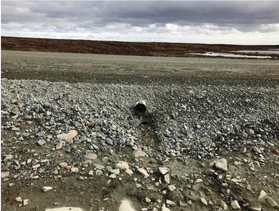
Photograph 101: At KM26.8, upstream ends of two vertically offset 160mm Ø steel pipes. The inlet of the lower pipe has been covered during placement of new road fill, should be extended. (14 September 2018).
