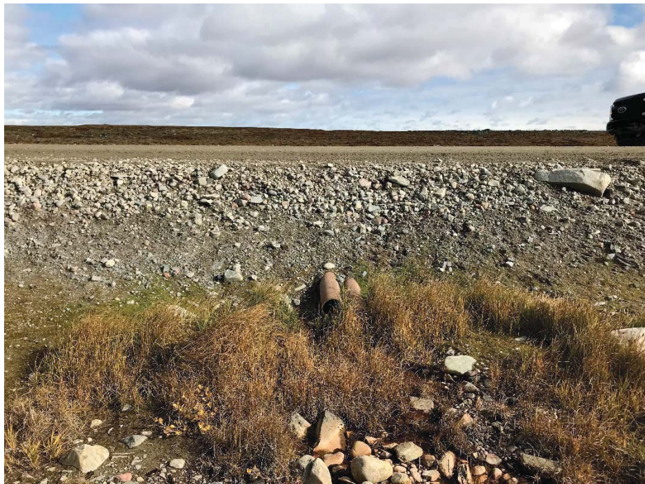
Photograph 83: Downstream ends of two 170 mm Ø steel pipes at KM21.7 (14 September 2018)
