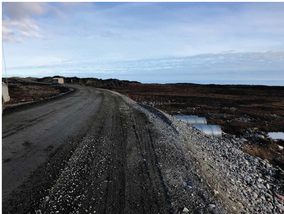
Photograph 64: AWAR surface over downstream ends of 3 CSP culverts at KM 16.3 (13 September 2018)
