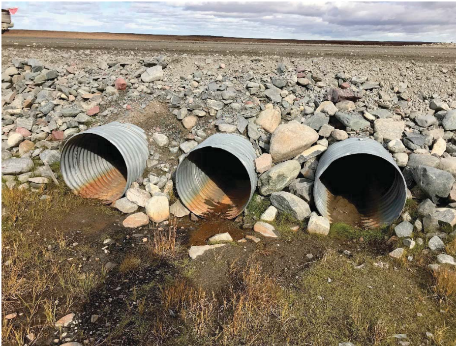
Photograph 96: Upstream ends of three 700mm Ø CSP culverts at KM26.5. Minor sediment buildup in the bottom of the culverts shouldn't substantially influence flows, monitor. (14 September 2018)
