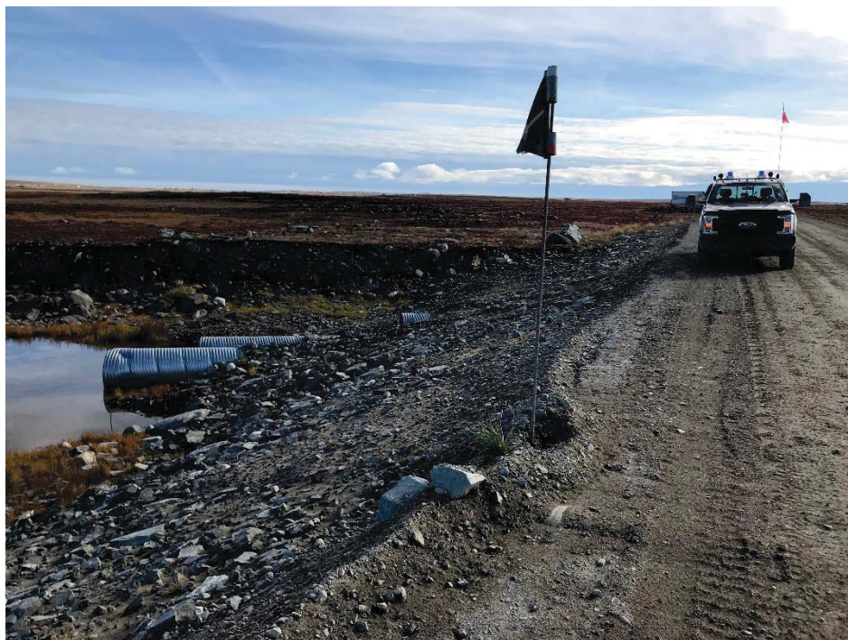
Photograph 20: Downstream embankment and road over 3 CSP culverts at KM7.4, looking south (13 September 2018)
