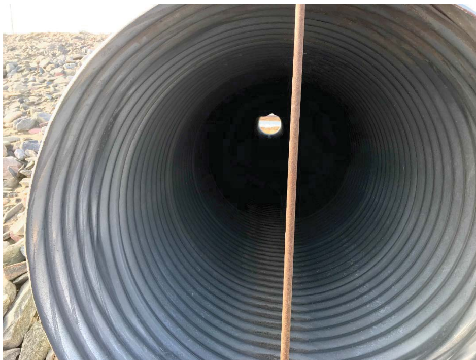
Photograph 33: View through lower CSP culvert at KM9.1 from downstream to upstream. No observable change in deformation of culvert when compared to 2017 inspection (13 September 2018)
