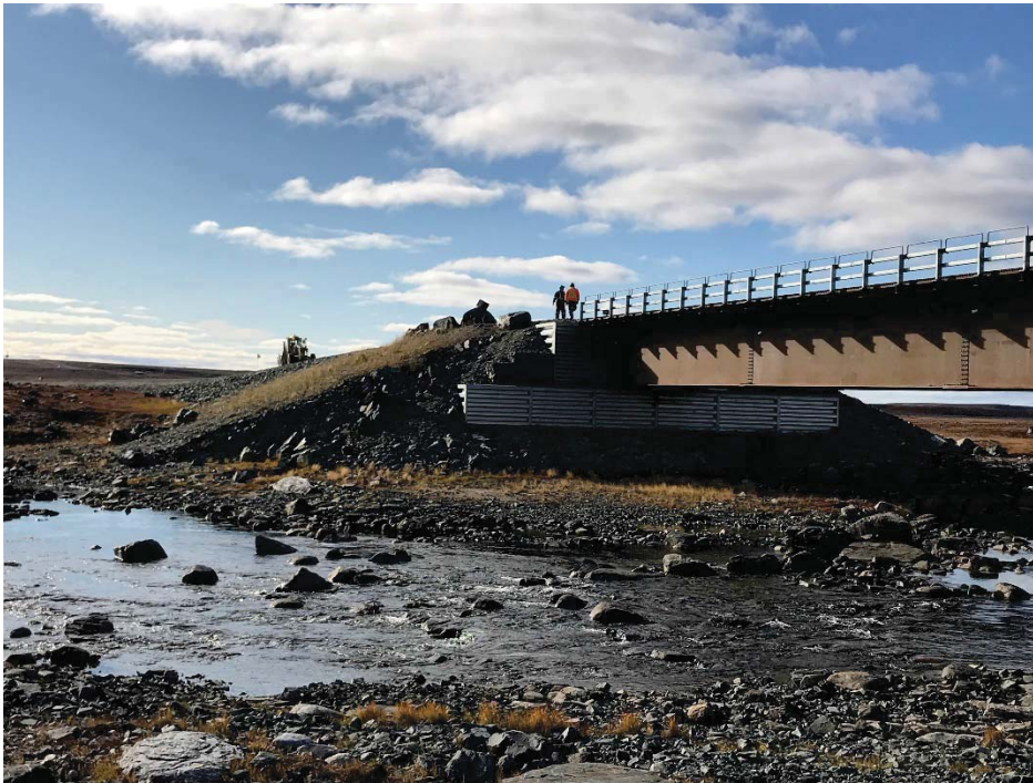
Photograph 29: Meliadine River Bridge at KM8.0 view of Right (southwest) Abutment, photo taken from the Left (northeast) Abutment. Finer grained material on abutment was observed in 2017; grass has grown on this material since 2017, no substantial erosion observed. Continue to monitor. (13 September 2018)
