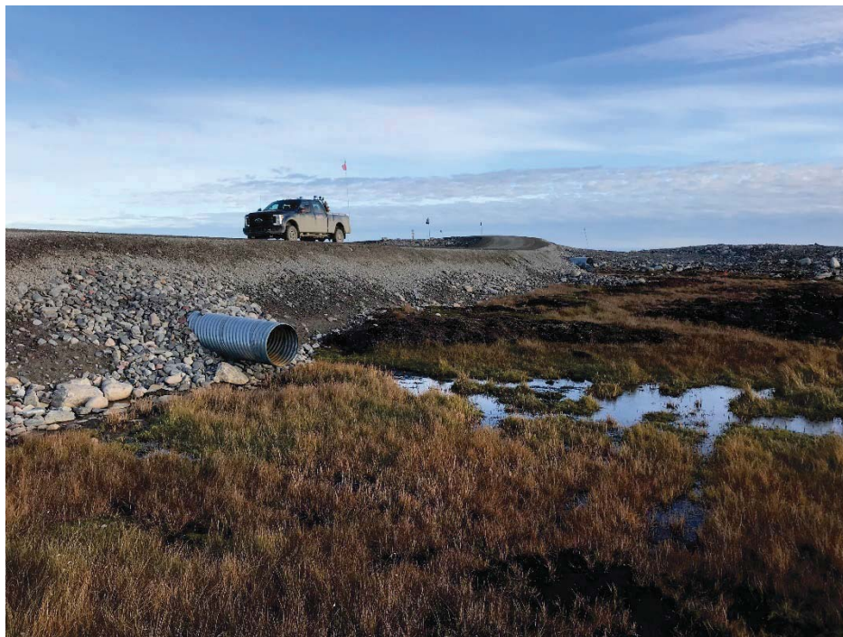
Photograph 72: Downstream end of 600 mm Ø CSP culvert at KM18.15 and view of AWAR slope, looking south (13 September 2018)
