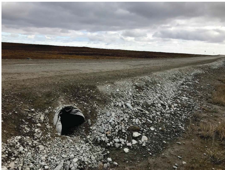
Photograph 91: Damaged upstream end of corrugated 600 mm Ø HDPE culvert at KM25.8. Inlet is partially blocked and should be cleaned out. (14 September 2018)
