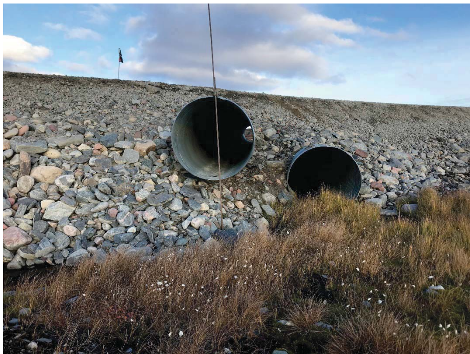
Photograph 69: Downstream ends of two CSP culverts at KM 18.1 (13 September 2018)
