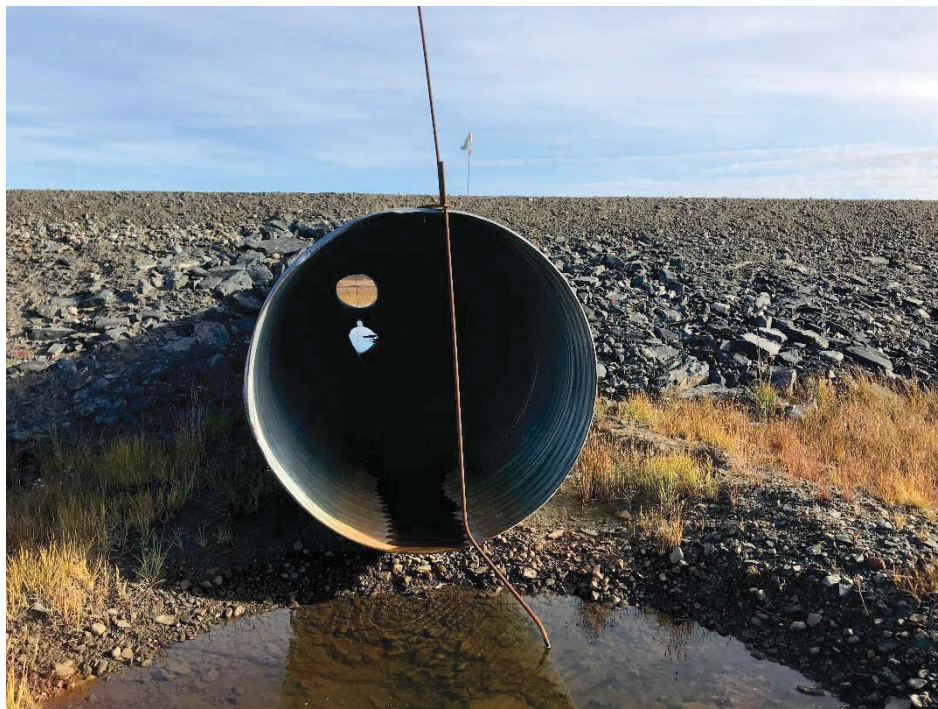
Photograph 38: View through 1300 mm Diameter CSP Culvert at KM9.5 from the downstream end. Slight deformation of culvert under the road (13 September 2018)
