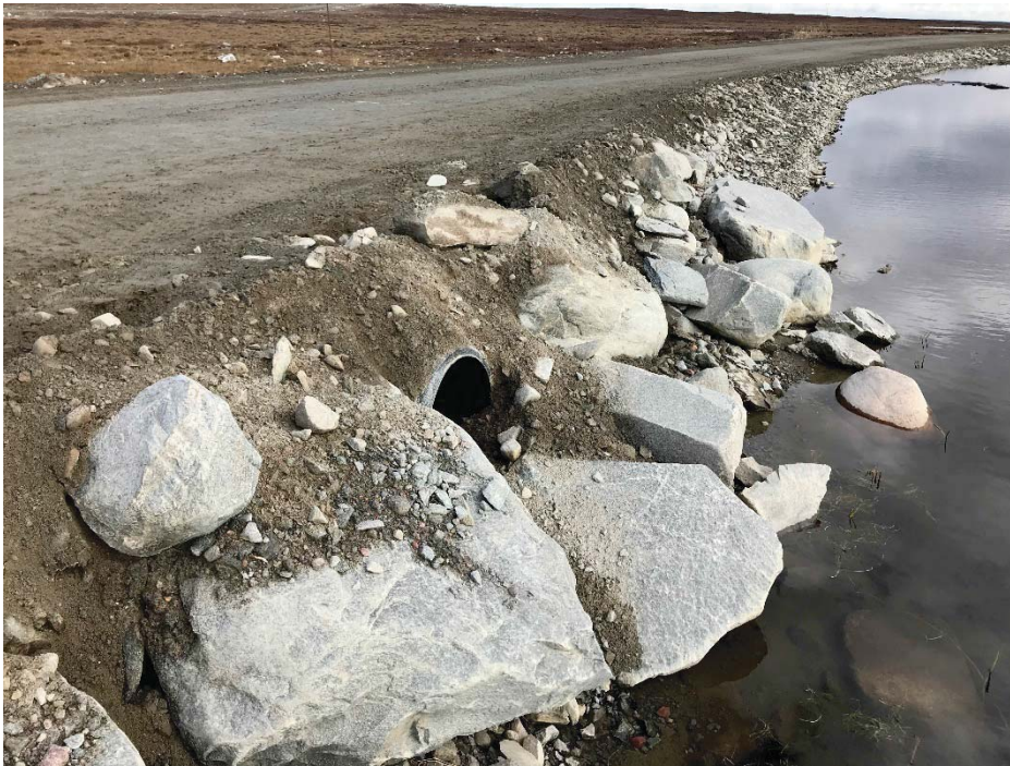
Photograph 111: At KM29.6, upstream end of single 500 mm Ø corrugated HDPE culvert. Inlet to the culvert is partially blocked by riprap and road fill and is elevated above ponded water at this location. Remove riprap, clean out culvert and recommend lowering invert. (14 September 2018).
