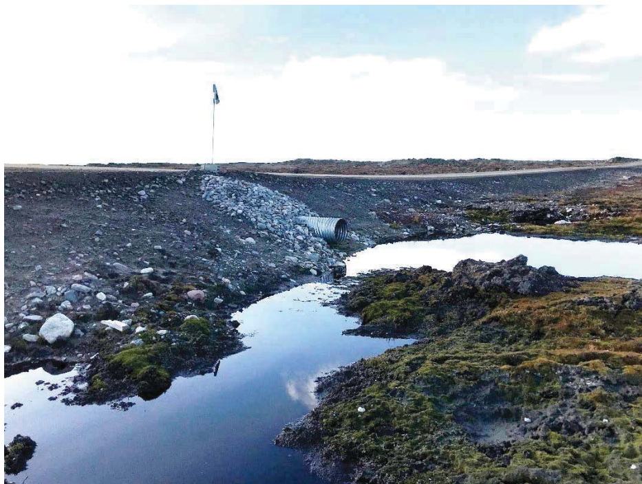
Photograph 71: Upstream end of a 600 mm Ø CSP Culvert at KM18.15. Water ponding below inlet. (13 September 2018)
