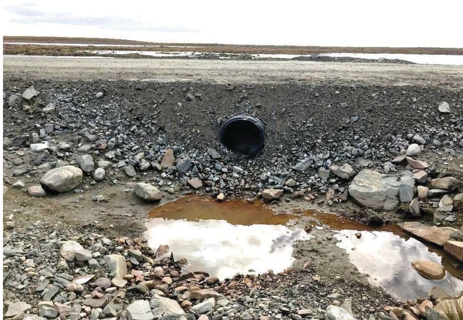
Photograph 113: Downstream end of 500 mm Ø corrugated HDPE culvert at KM29.6 (14 September 2018).
