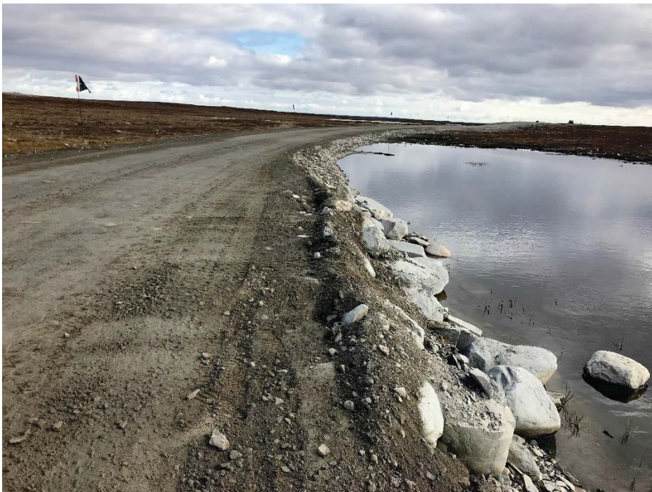
Photograph 112: View of water ponded upstream of 500mm Ø corrugated HDPE culvert at KM29.6 (14 September 2018).
