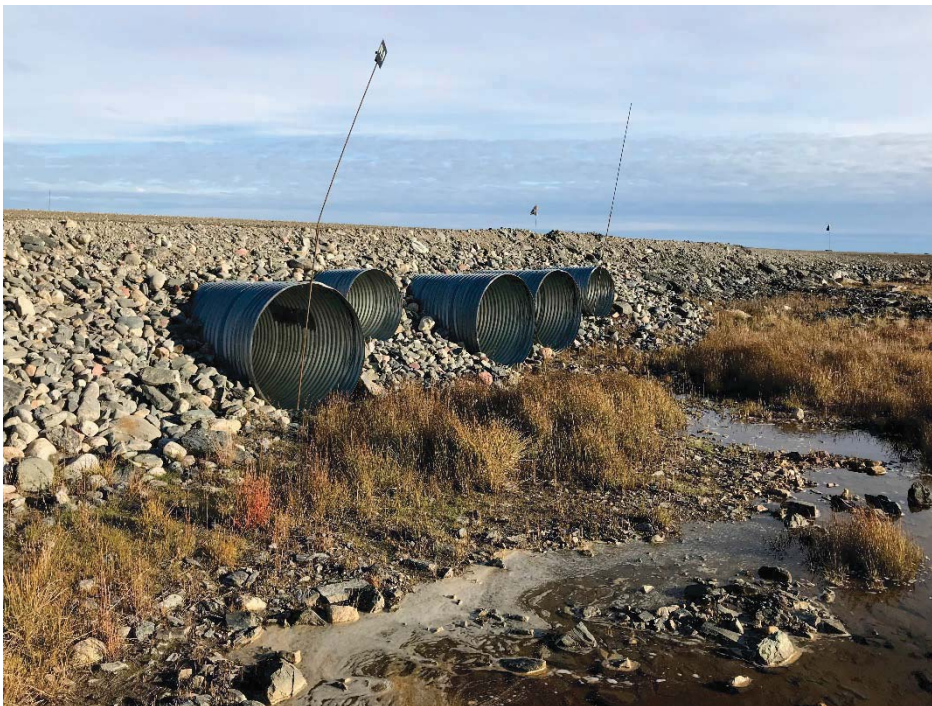
Photograph 56: Downstream ends of 5 CSP culverts at KM13.5 (13 September 2018)
