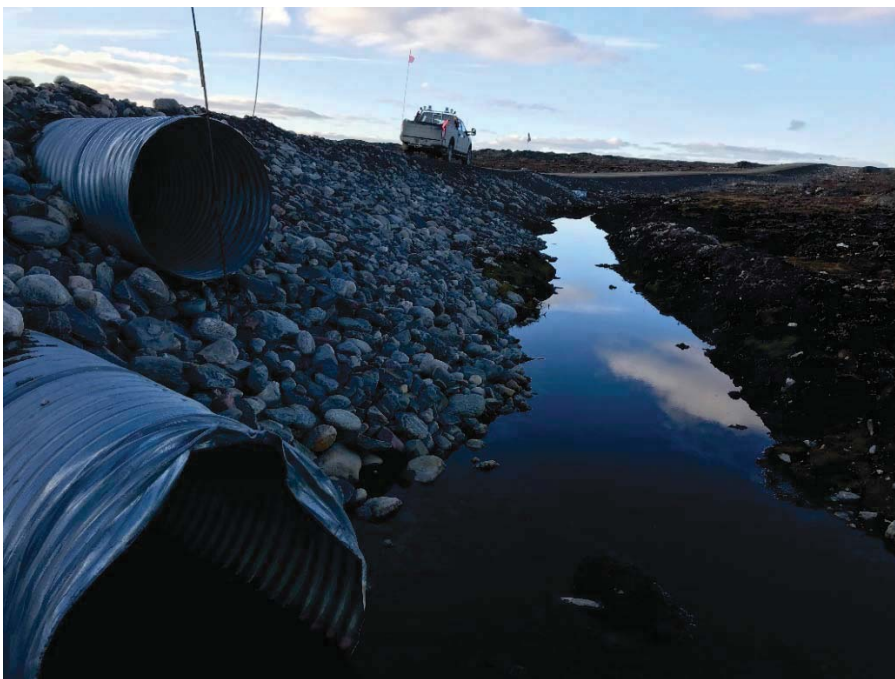
Photograph 68: Damage to the inlet of the lower (1000 mm Ø) CSP culvert at KM18.1. View north along the AWAR road embankment, slope looks good, but water ponded along road. Culvert at KM18.15 visible in background (13 September 2018)
