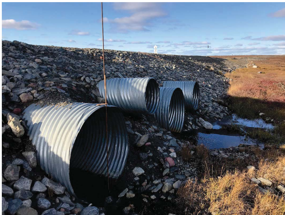
Photograph 50: Downstream ends of four CSP culverts at KM12.1, looking north along the embankment (13 September 2018)
