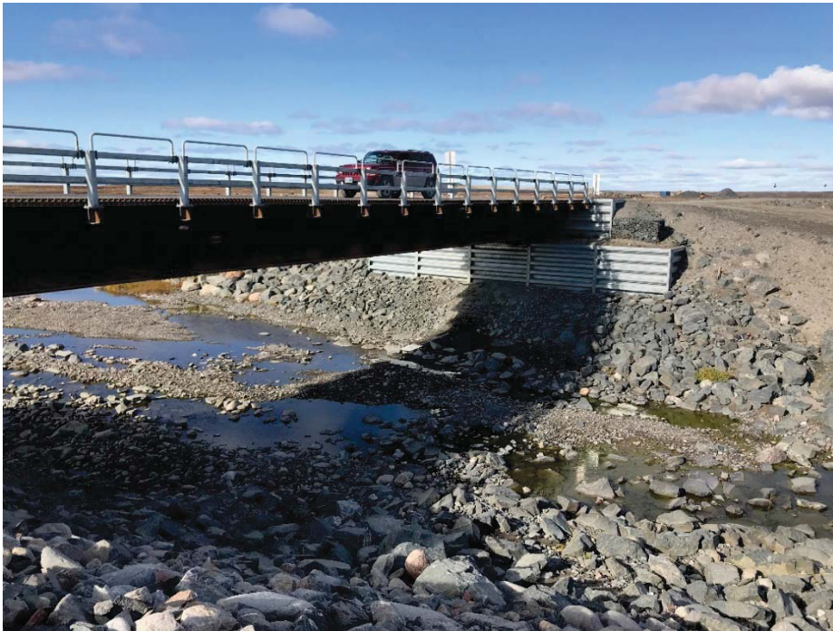
Photograph 5: Char River Bridge, downstream side of left (north) abutment, taken from the downstream side of the right (south) abutment. Finer grained material observed over coarse rockfill. (13 September 2018)
