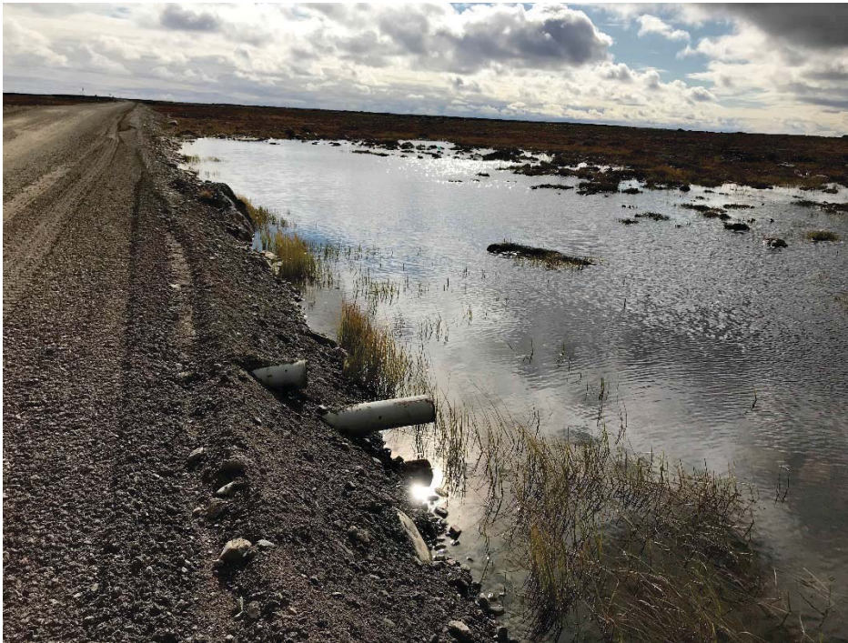
Photograph 85: At KM22.3, upstream ends of two 160 mm Ø steel pipes that are vertically offset. Water is ponded on the upstream side (14 September 2018)
