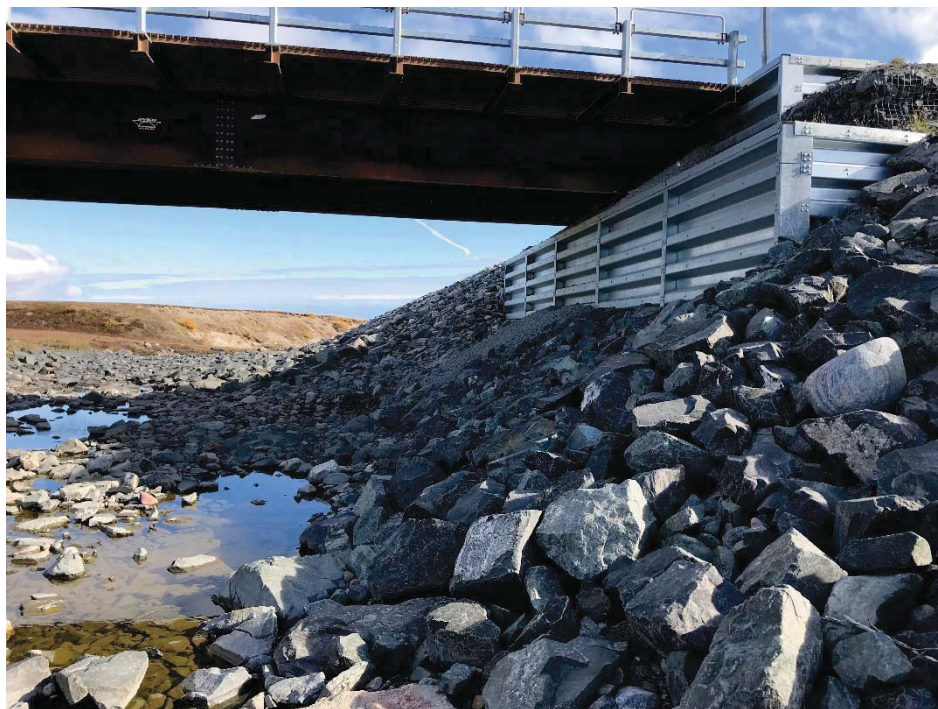
Photograph 3: Char River Bridge, right (south) abutment armouring, from the upstream side (13 September 2018)
