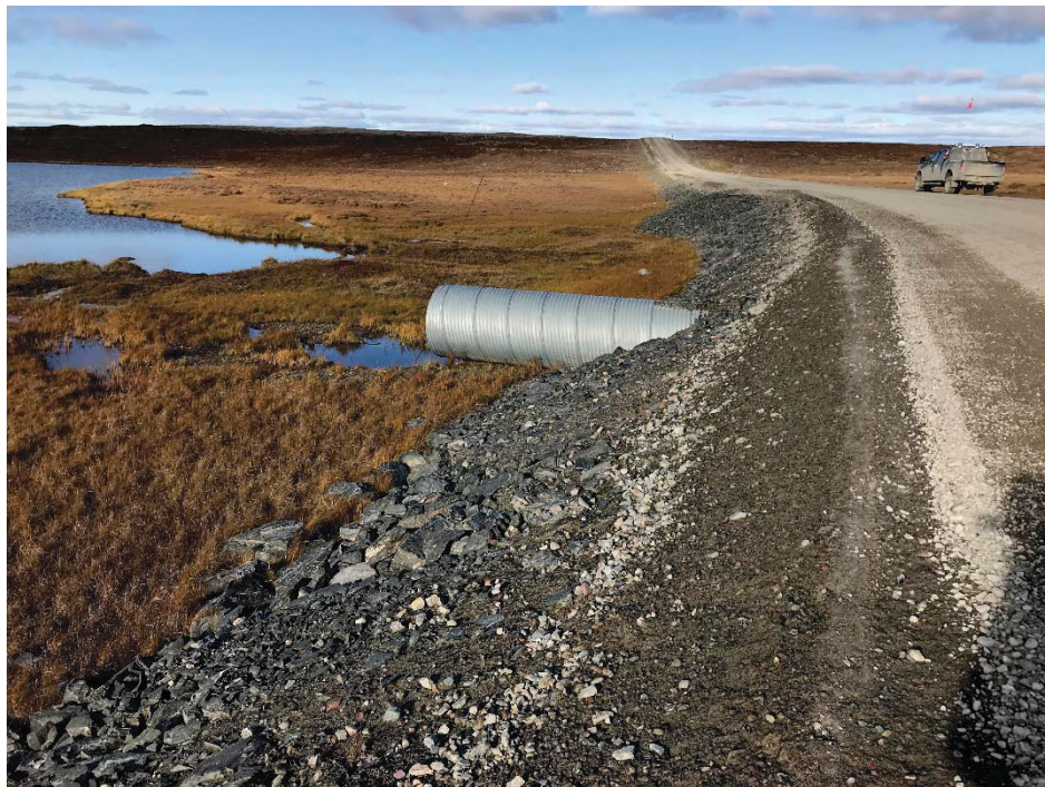
Photograph 37: Downstream end of a single 1300 mm CSP culvert at KM9.5 (13 September 2018)
