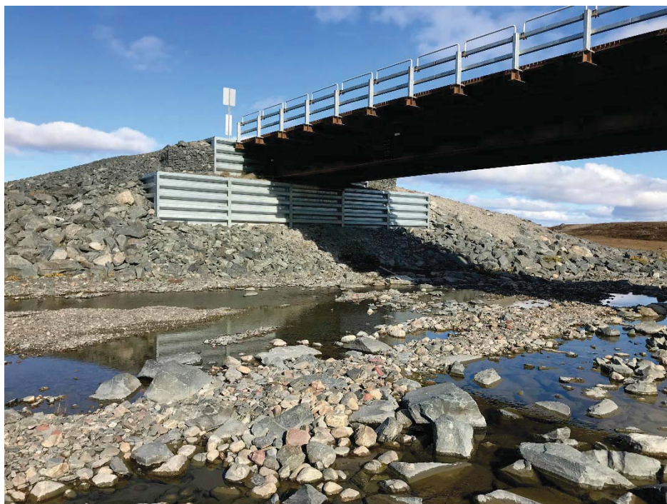
Photograph 2: Char River Bridge, Left (north) Abutment Armouring from the Upstream Side of the Right (south) Abutment (13 September 2018)
