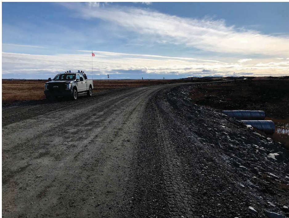
Photograph 12: Upstream embankment and road over 3 CSP culverts at KM7.1 (13 September 2018)
