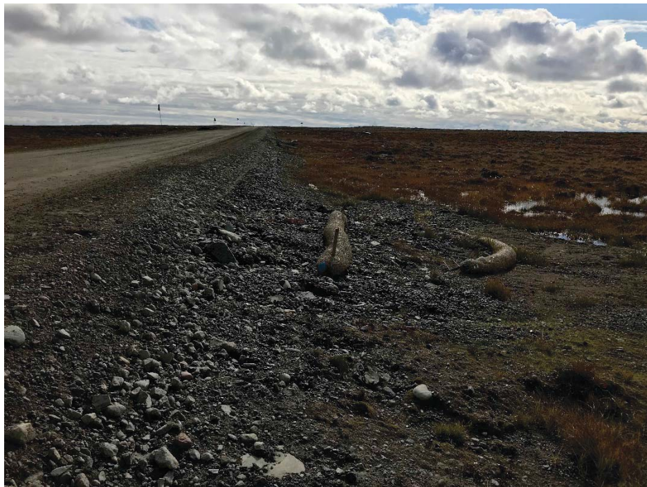
Photograph 84: Straw logs placed on west side of the road, south of the steel pipes at KM21.7 (14 September 2018)
