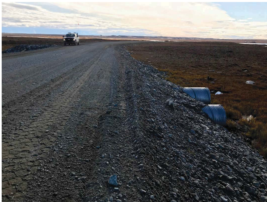
Photograph 34: Upstream embankment and road surface over two CSP culverts at KM9.1, looking southwest (13 September 2018)
