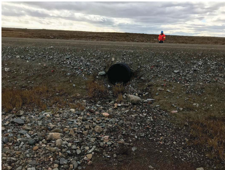
Photograph 92: Downstream end of corrugated 600 mm Ø HDPE culvert at KM25.8 (14 September 2018)
