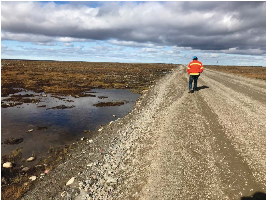
Photograph 78: At KM21.2 where water is ponding on the west side of the AWAR, looking north (14 September 2018)
