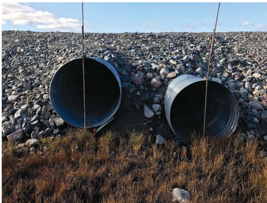
Photograph 32: Downstream ends of two 1000 mm \varnothing CSP culverts at KM9.1, (13 September 2018)
