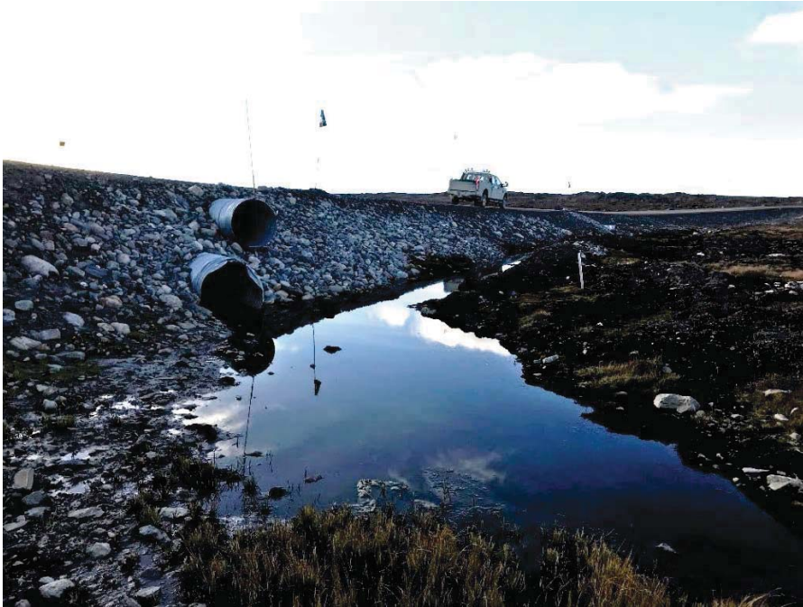
Photograph 67: At KM18.1, upstream ends of two CSP culverts. Upper culvert is 900 mm Ø and the lower is 1000 mm Ø. Cover over upper (900 mm Ø) culvert is thin on upstream side (13 September 2018)
