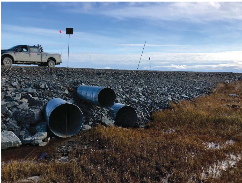
Photograph 14: Upstream ends of 3 CSP culverts at KM7.1 (13 September 2018)
