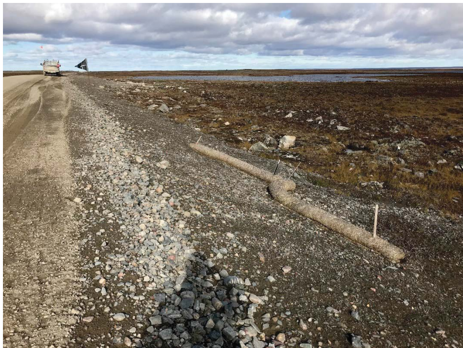
Photograph 80: At KM21.5, a straw log on east side of the road. Water reportedly flows over the road during spring freshet at this location. (14 September 2018)
