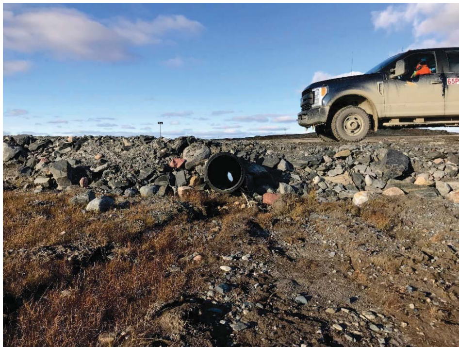
Photograph 60: View through culvert under B12 Quarry access road at KM14.7 of AWAR, no flow, small amount of ponded water within culvert (13 September 2018)
