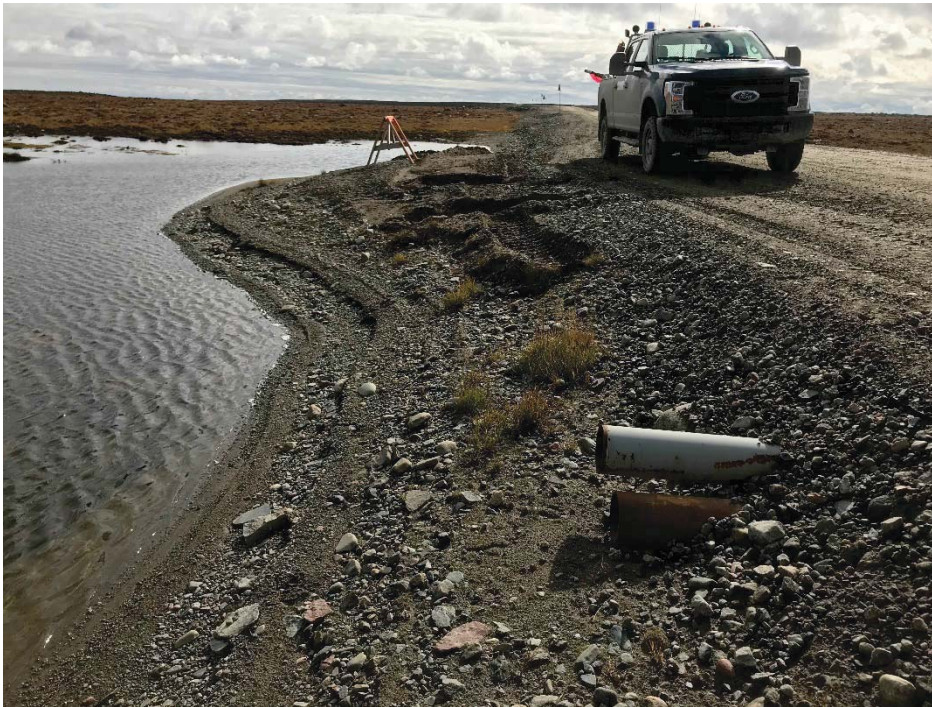
Photograph 81: At KM21.7, view of the upstream ends of two steel pipes, each with an outside diameter of 170 mm. Water is ponded year-round at this location. Mine personnel reported that during freshet it was necessary to excavate the road at this location to let the water drain (14 September 2018)
