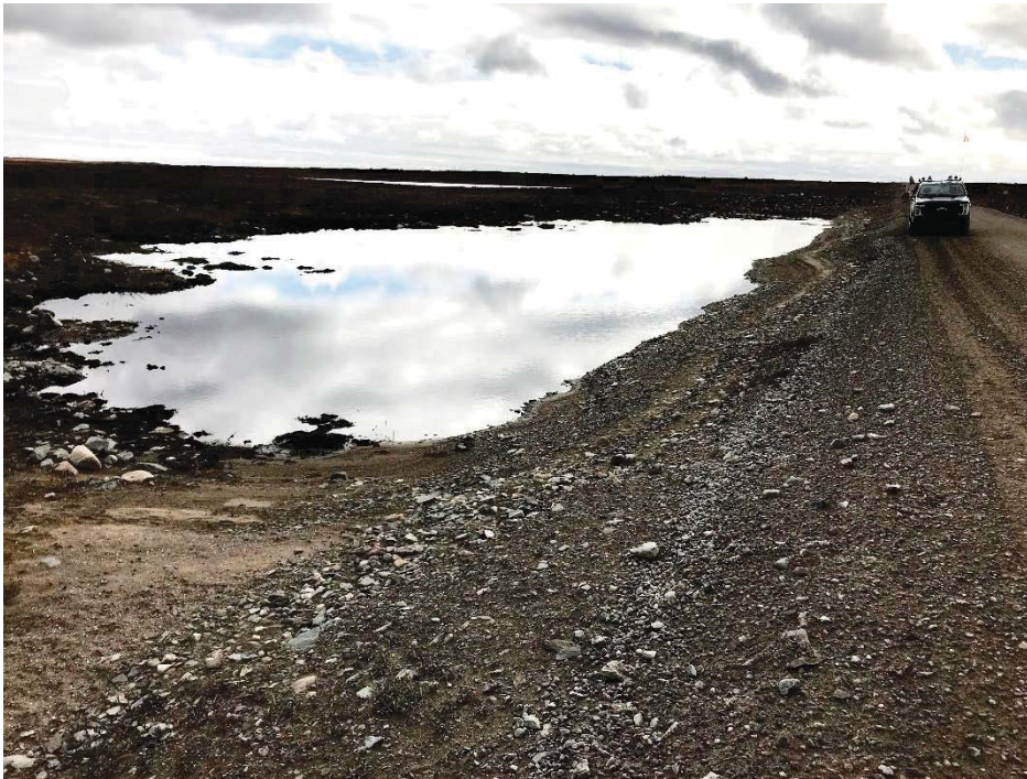
Photograph 89: Ponded water on the east side of the AWAR near KM22.7. No culvert at this location (14 September 2018)
