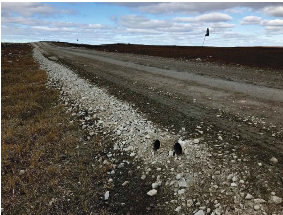
Photograph 94: Upstream ends of two 160 mm Ø steel pipes at KM26.2. The lower pipe is bent upwards and should be replaced. The inlets are elevated close to road surface and nearly covered by road fill, consider lowering and extending (14 September 2018)
