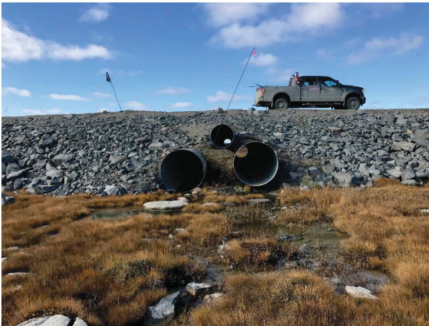
Photograph 6: At KM6.2, Downstream ends of 3 CSP culverts. Lower two culverts are 1300 mm \varnothing , upper culvert is 700 mm \varnothing . All are in good condition. Small erosion between culverts, consider adding armouring (13 September 2018)
