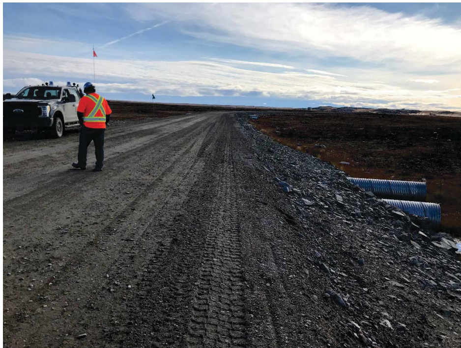
Photograph 15: Upstream embankment and road over 3 CSP culverts at KM7.1, looking south (13 September 2018)
