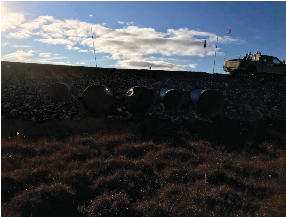
Photograph 55: At KM13.5, upstream ends of 5 CSP Culverts (3×1300 mm \varnothing ; 2×900mm \varnothing ). The 900 mm culverts are vertically elevated. Minor deformation of the culverts under the road (13 September 2018)
