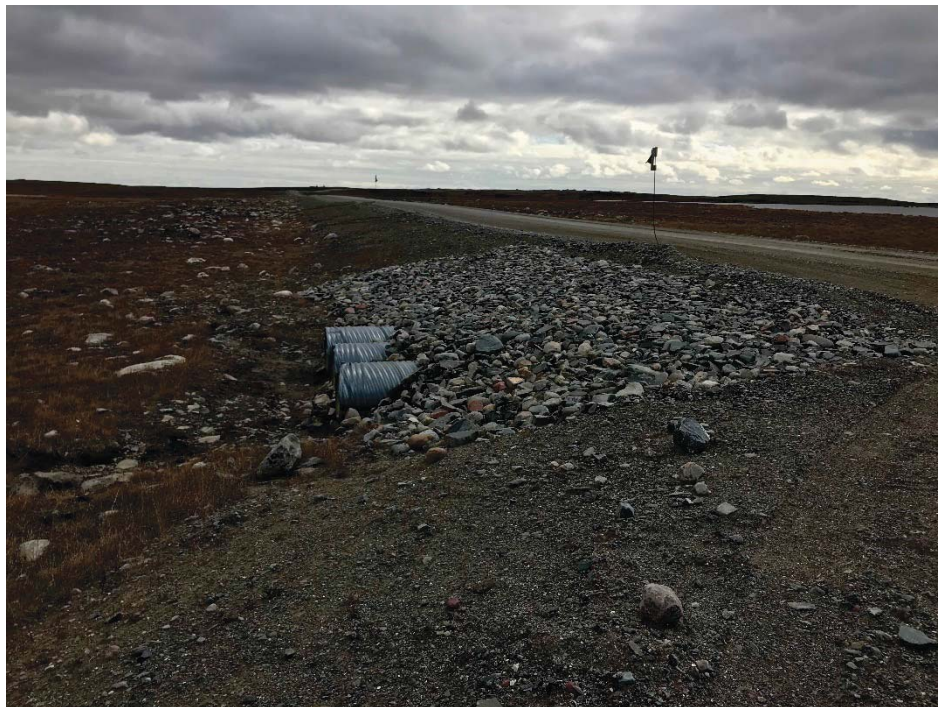
Photograph 97: Downstream ends of three CSP culverts at KM26.5. Riprap and embankments are in good condition (14 September 2018).
