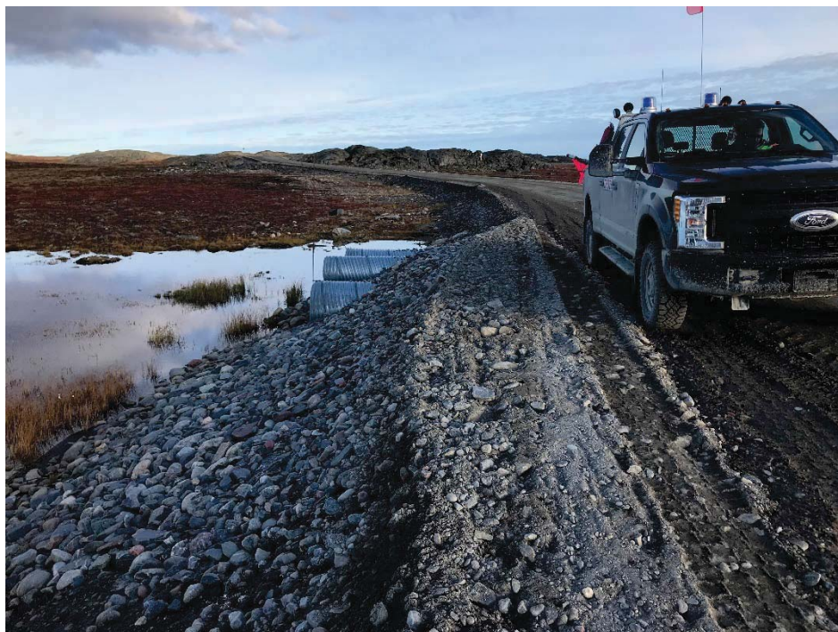
Photograph 63: At KM16.3, upstream ends of 3 CSP culverts, looking south (13 September 2018)
