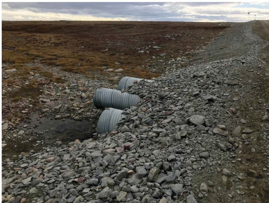
Photograph 106: Downstream ends of three CSP culverts at KM27.1. From left to right, 1000 mm, 700 mm, and 900 mm ø. (14 September 2018)
