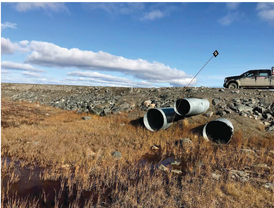
Photograph 10: Upstream ends of 3 CSP culverts at KM7.0. Minor damage to the upper and lower right culverts. Some exposed sand around the culvert inlets, additional armoring should be considered (13 September 2018)
