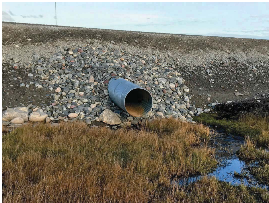
Photograph 73: Closer view of downstream end of 600 mm Ø CSP culvert at KM18.15 (13 September 2018)
