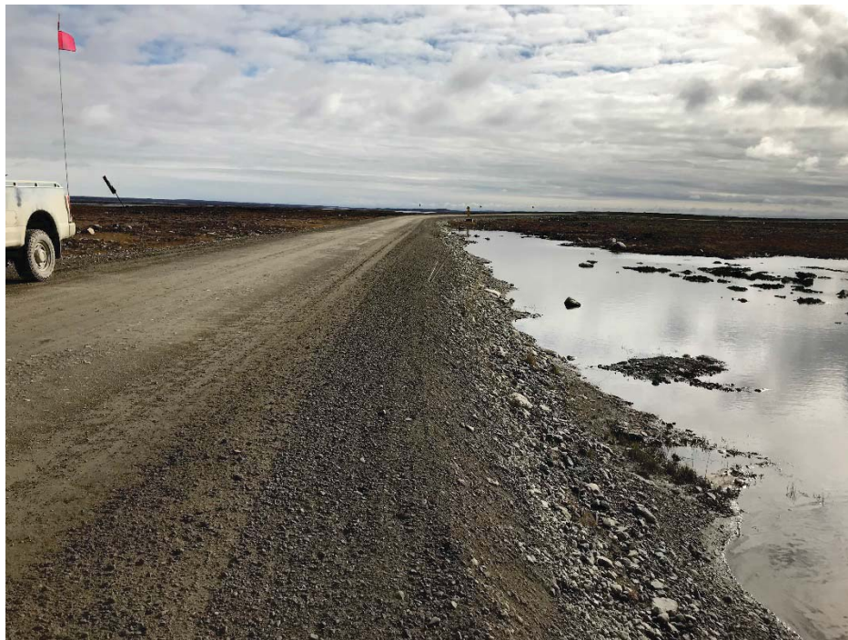
Photograph 76: Water ponding on the west side of the road at KM19.5, looking south. Installation of a culvert should be considered (14 September 2018)
