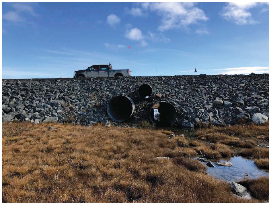
Photograph 7: Upstream to downstream view of 3 CSP culverts at KM6.2 (13 September 2018)
