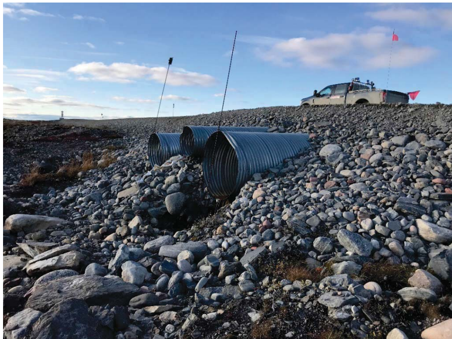
Photograph 65: Downstream ends of three CSP culverts at KM16.3. Diameters of the culverts from left to right are: 1000 mm, 700 mm, and 1300 mm Ø. Small flow in 1300 Ø culvert and minor deformation. Some erosion visible at outlet of 1300 mm culvert (13 September 2018)
