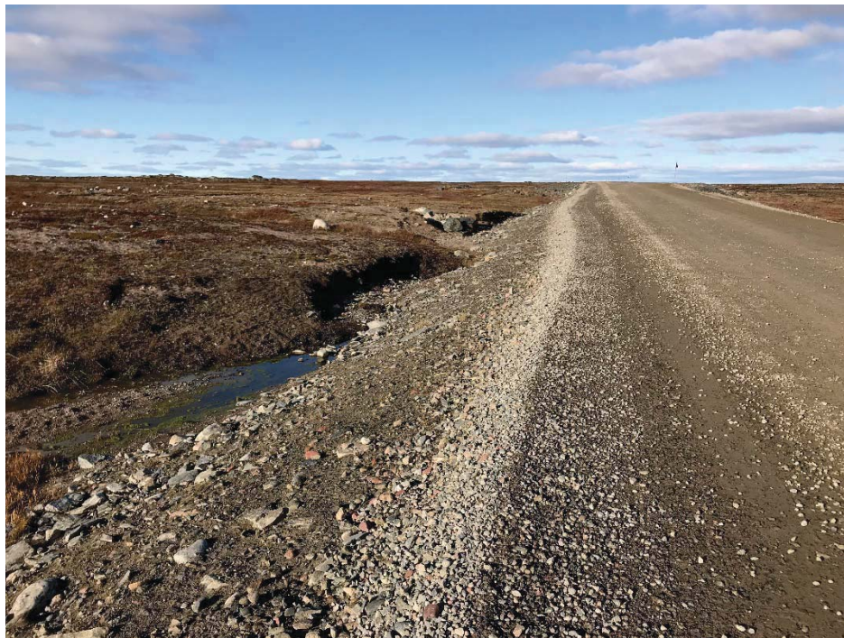
Photograph 53: West side of AWAR at KM12.6 where water flows along the side of the road and seeps under the road from west to east (13 September 2018)
