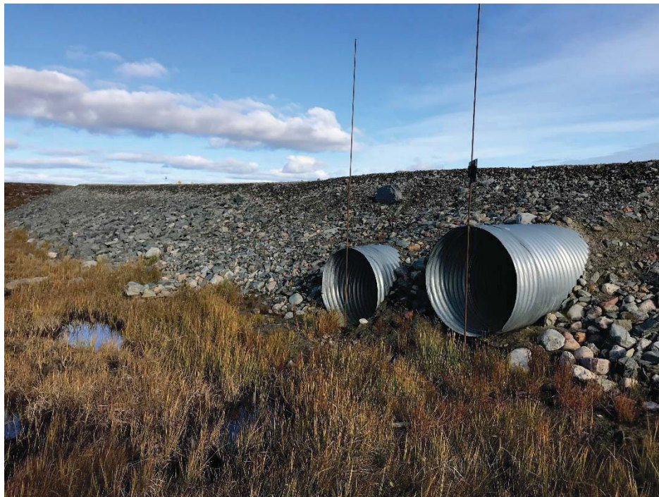
Photograph 31: At KM9.1, upstream ends of two 1000 mm \varnothing CSP culverts (13 September 2018)
