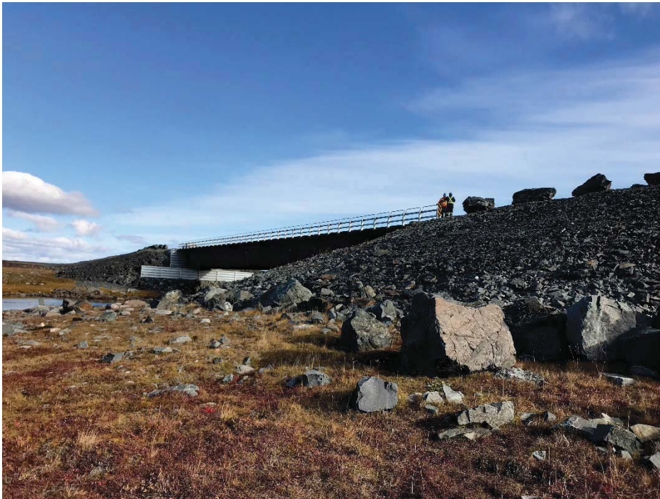
Photograph 28: Meliadine River Bridge at KM8.0. Embankment for the Right (southwest) Abutment, from the upstream side. The far abutment in the photo is the Left (northeast) Abutment. Riprap is in good condition (13 September 2018)
