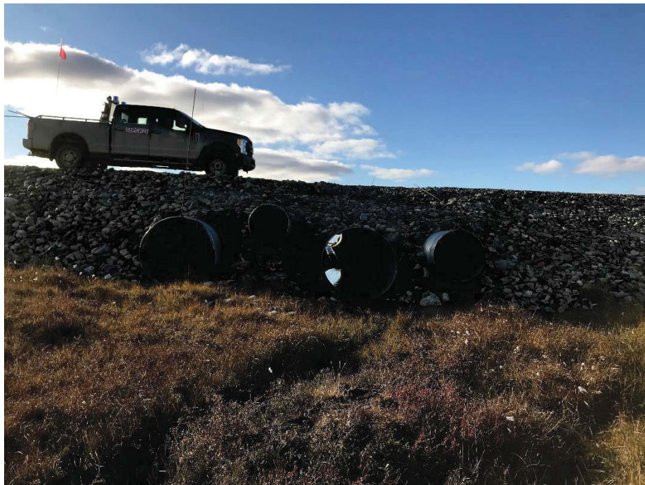
Photograph 49: Downstream ends of four CSP culverts at KM12.1. Small flow observed through the lowest culvert (second from right in the photograph). Visible deformation of the culverts under the road (13 September 2018)
