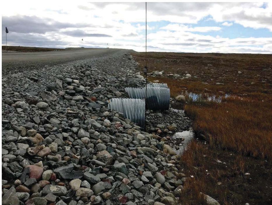
Photograph 105: At KM 27.1, upstream ends of three CSP culverts. Some minor sloughing of riprap observed around culvert inlets. (14 September 2018)
