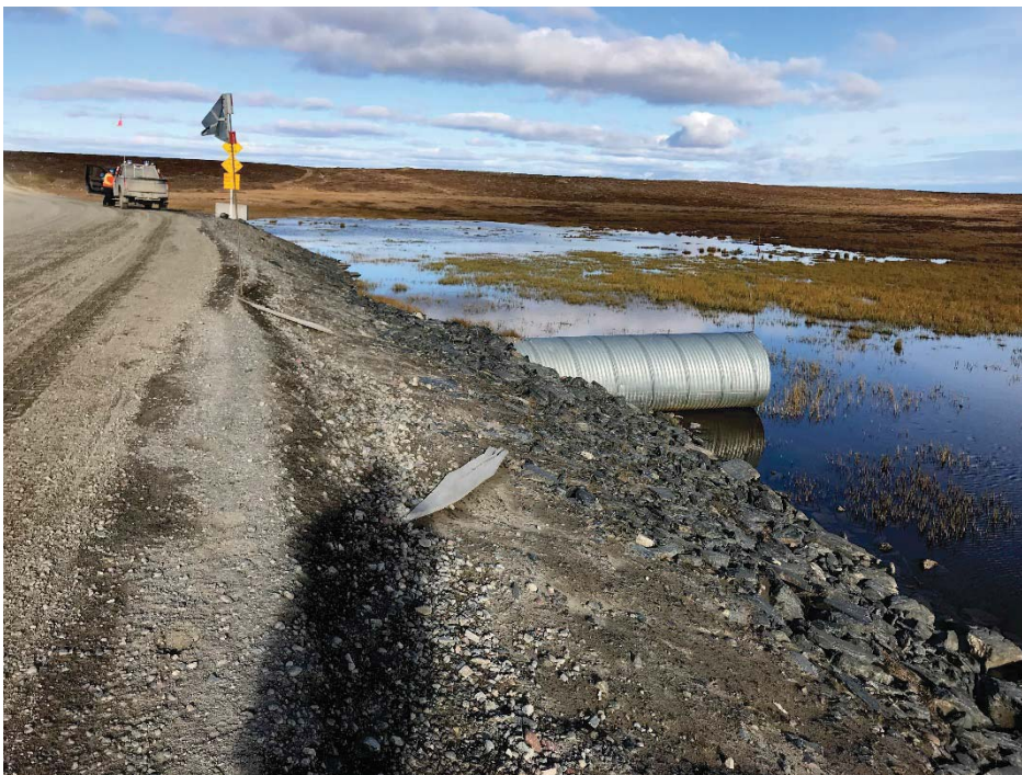
Photograph 36: At KM9.5, upstream end of a single 1300 mm ø CSP. Culvert inlet is elevated, allowing water to pond upstream. (13 September 2018)
