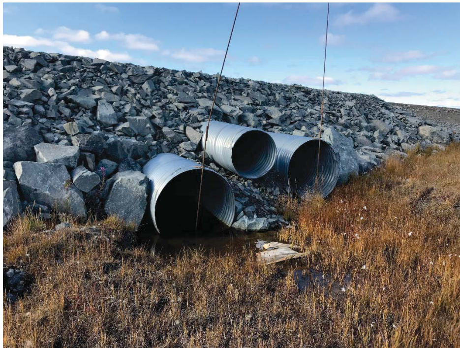
Photograph 13: At KM7.1, downstream ends of 3 CSP culverts. Lower two culverts are 1000 mm \varnothing , upper culvert is 700 mm \varnothing . All are in good condition. Small flow through lower culvert at time of inspection. Riprap in good condition (13 September 2018)
