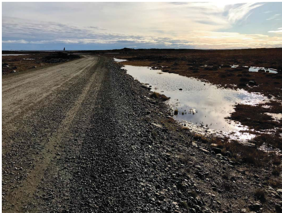
Photograph 54: AWAR KM 12.6, ponded water on the east side of the road where it is seeping out of the road fills (13 September 2018)
