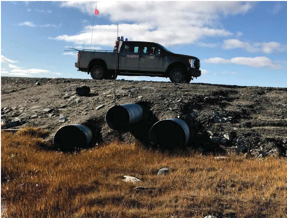
Photograph 9: At KM7.0, downstream ends of 3 CSP culverts. Lower two culverts are 1000 mm \varnothing , upper culvert is 700 mm \varnothing . All are in good condition. Water ponded in lower culvert at the time of inspection (13 September 2018)
