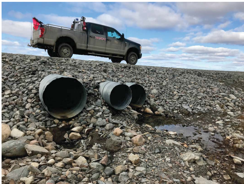
Photograph 107: Downstream outlets of three CSP culverts at KM27.1, some minor erosion/deposition evident under outlets. Monitor and add rip-rap if further erosion occurs. (14 September 2018).
