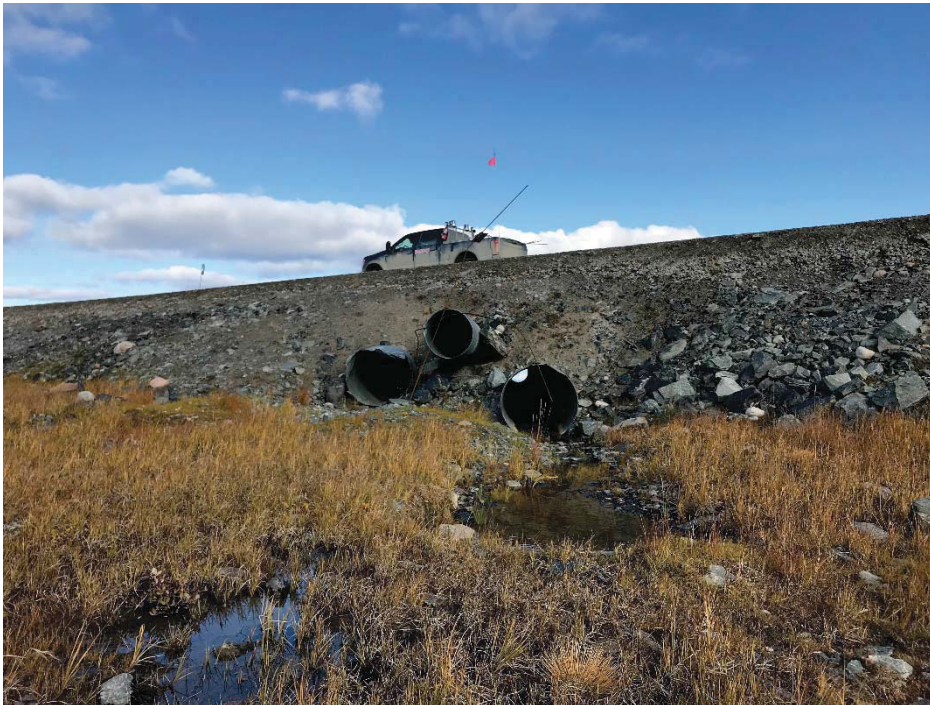
Photograph 17: At KM7.4, upstream ends of 3 CSP culverts. Lower two culverts are 900 mm \varnothing (left) and 1000 mm \varnothing (right), and the upper culvert is 700 mm \varnothing . Inlet of the 900 mm has been damaged, (13 September 2018)
