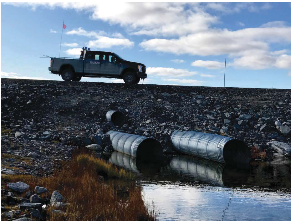
Photograph 18: Downstream ends of 3 CSP culverts at KM7.4 (13 September 2018). Consider extending the upper culvert to reduce erosion of the embankment.
