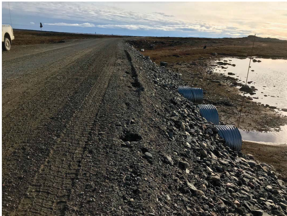
Photograph 51: Upstream ends of four CSP culverts at KM12.1 looking south along the embankment (13 September 2018)
