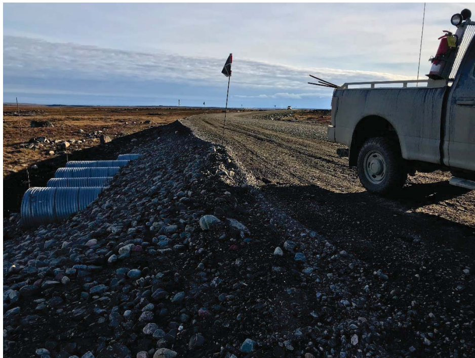
Photograph 57: View of the embankment and road over upstream ends of 5 CSP culverts at KM13.5 looking south (13 September 2018)
