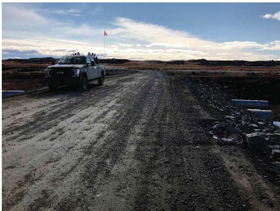
Photograph 8: Road over 3 CSP culverts at KM6.2 (13 September 2018)
