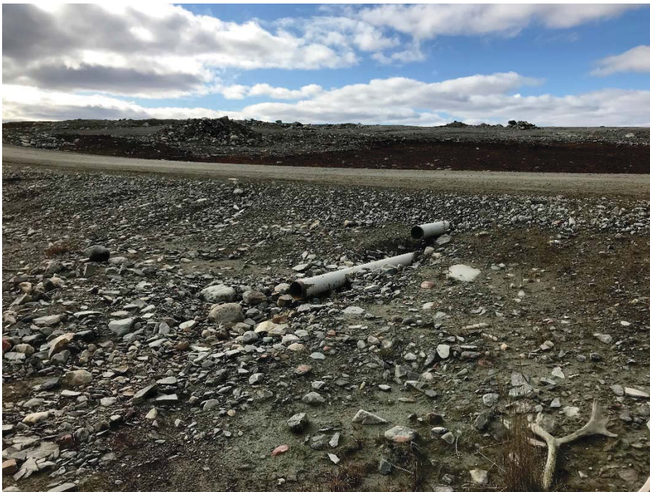
Photograph 102: Downstream ends of two 160mm Ø steel pipes at KM26.8. Some minor erosion of the road embankment evident beneath the outlets of both pipes (14 September 2018).
