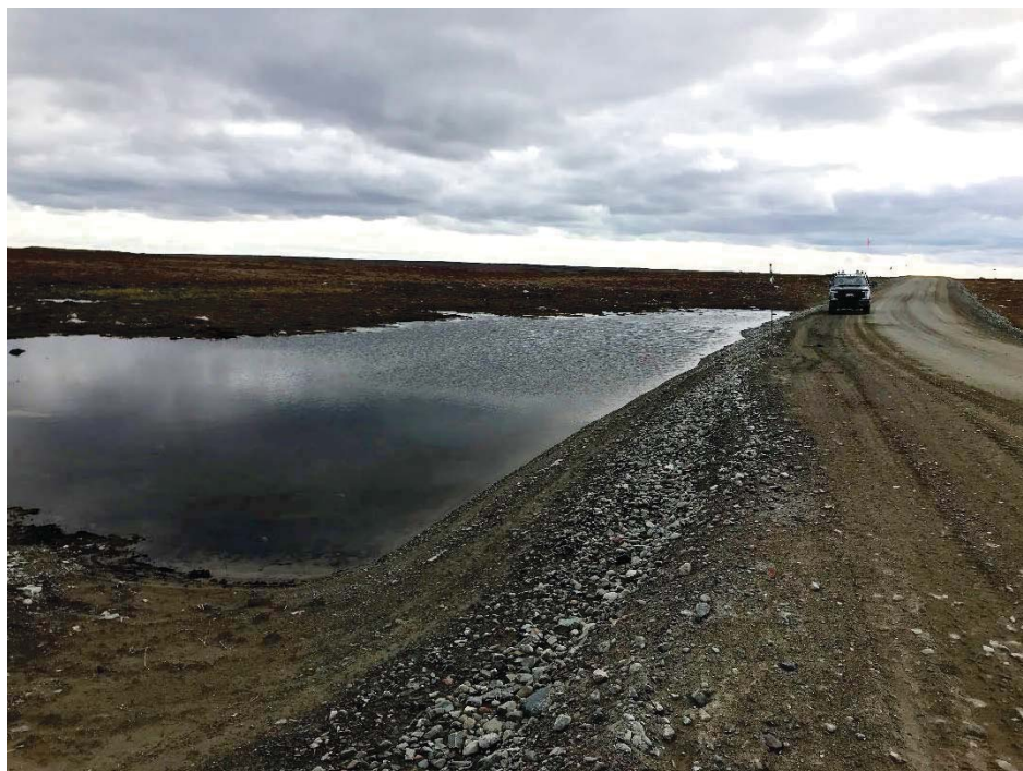
Photograph 109: At KM28.7 where water is ponding on the east side of the AWAR. Mine personnel report that water flowed over the road in the spring. Consider installing a culvert at this location (14 September 2018).
