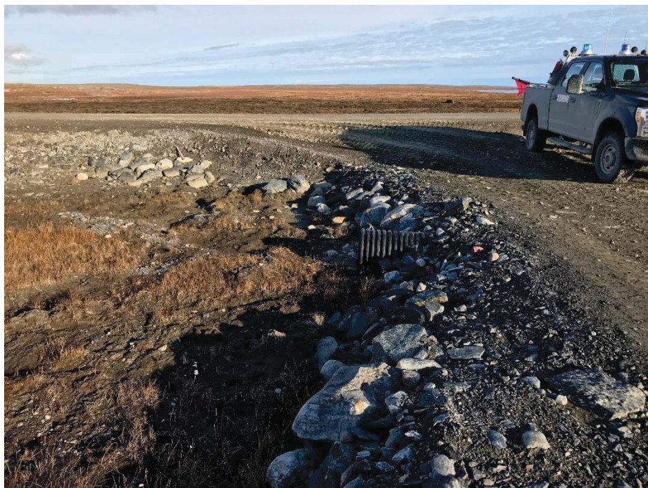
Photograph 61: Upstream end of culvert through B12 Quarry access road at KM14.7 of AWAR (13 September 2018)
