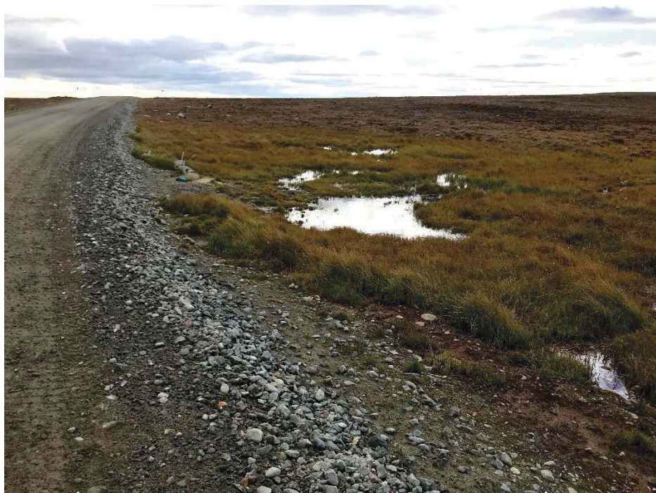
Photograph 110: Wet ground and some ponded water on the west side of the AWAR at KM28.7 (14 September 2018).
