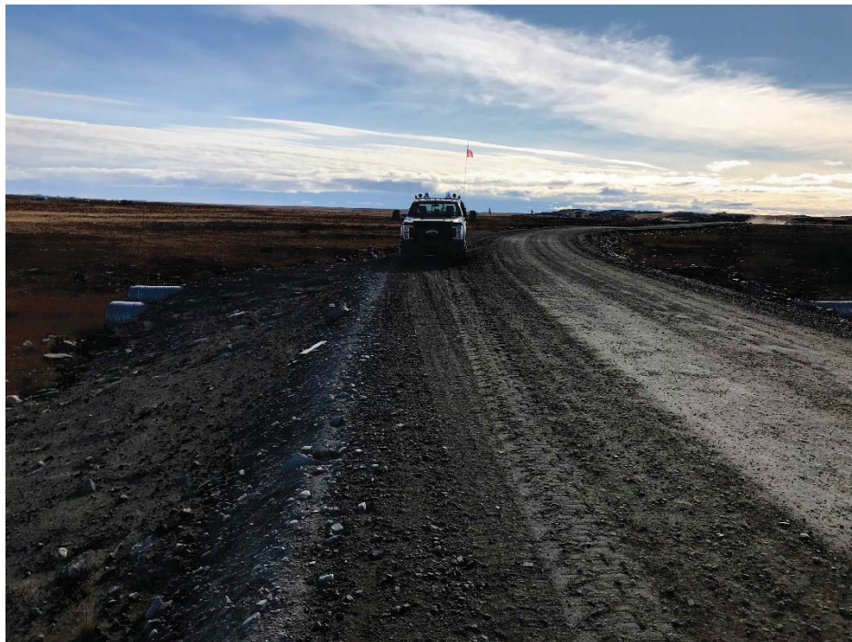
Photograph 11: Downstream embankment and road over 3 CSP culverts at KM7.0 (13 September 2018)
