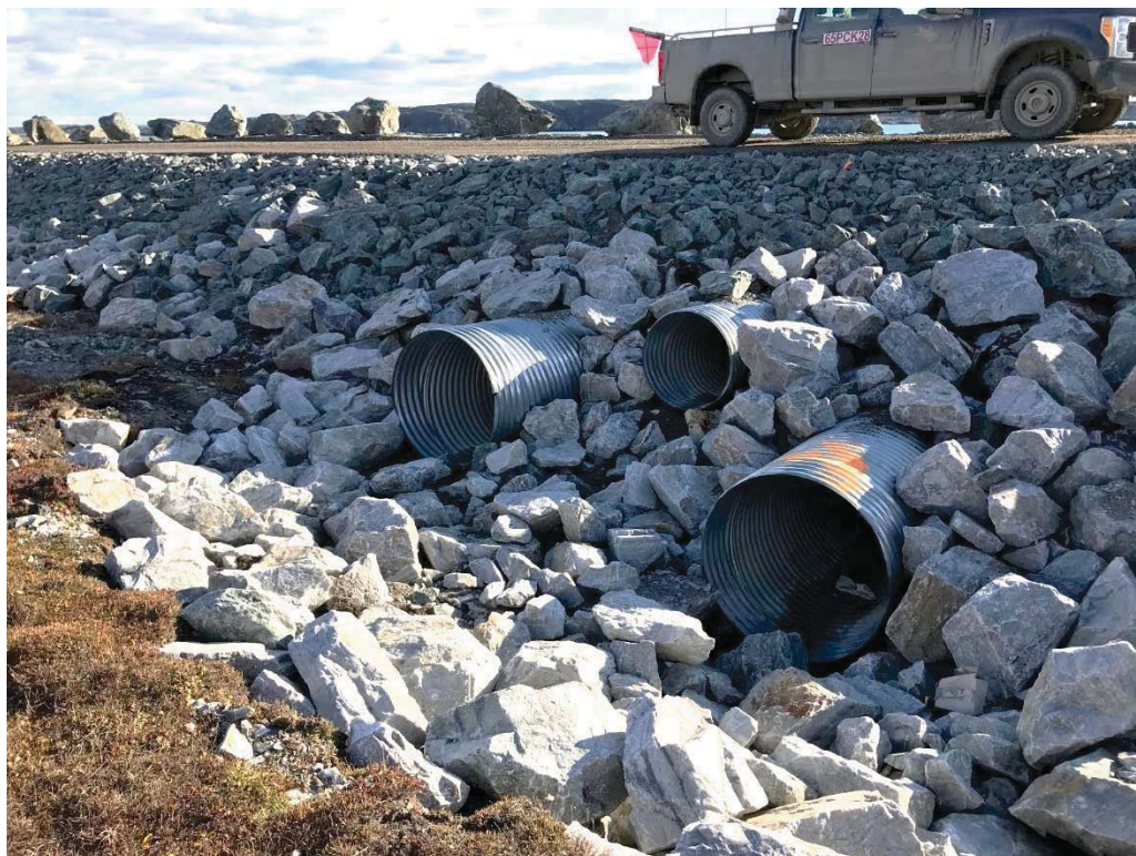
Photograph 15: Inlets for Culvert C03, Looking South (14 September 2018)
