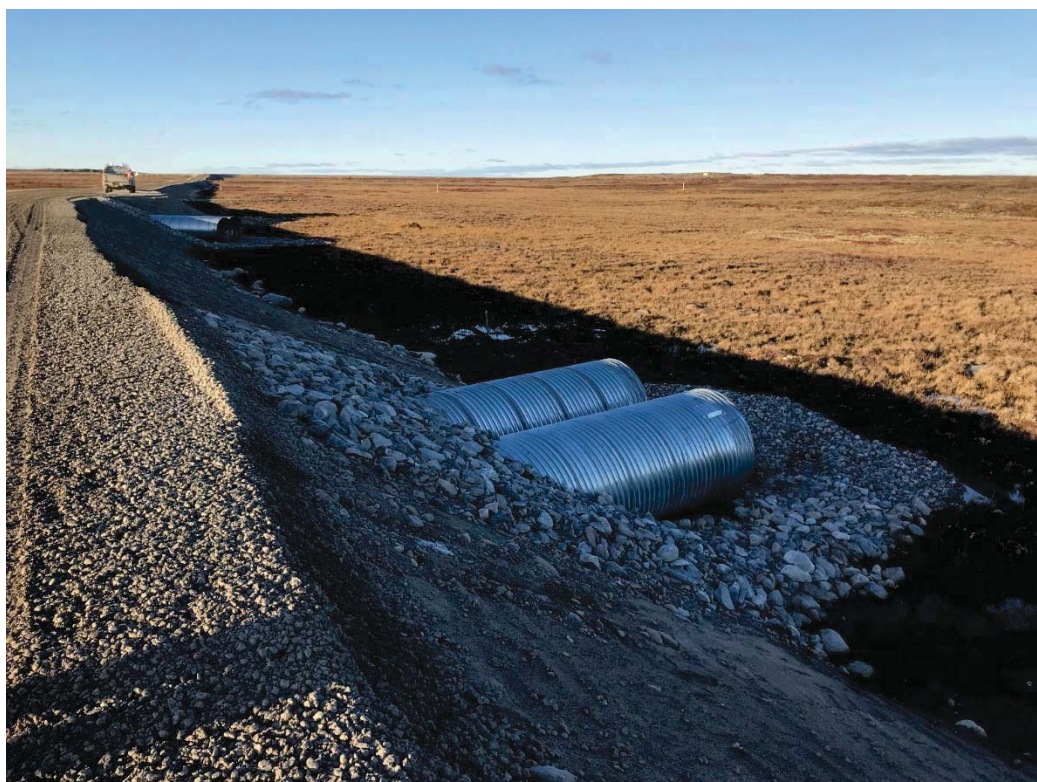
Photograph 44: Culvert 12a Outlet, Looking North (14 September 2018)
