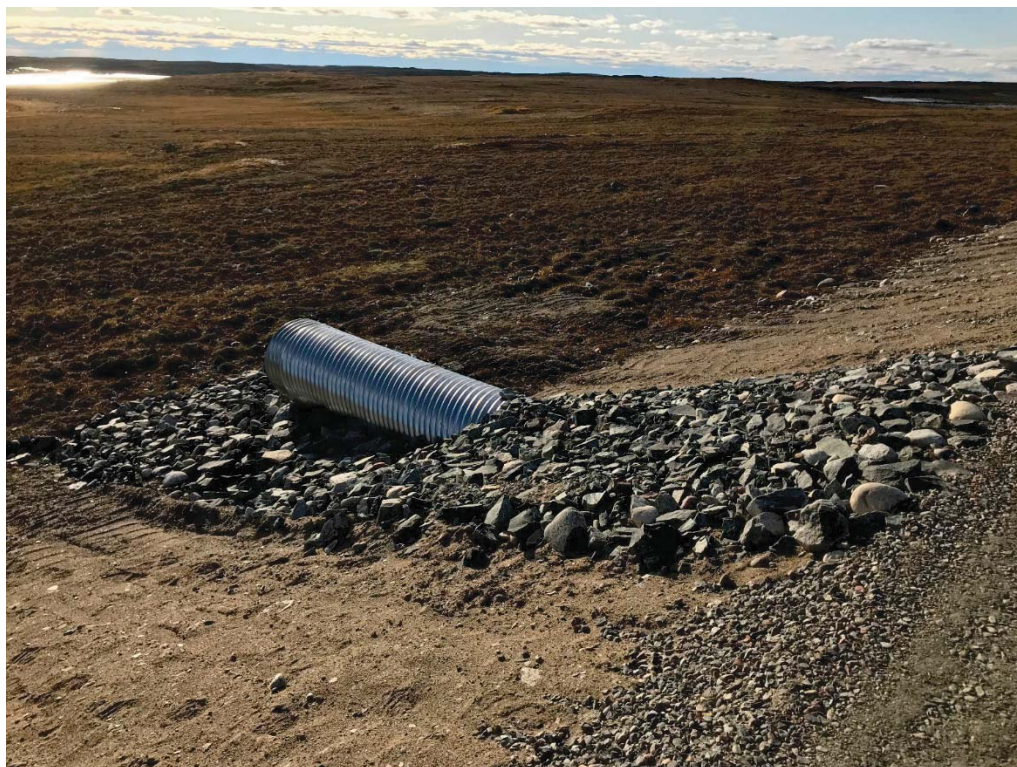
Photograph 25: Outlet for Culvert C06-1, Looking West (14 September 2018)
