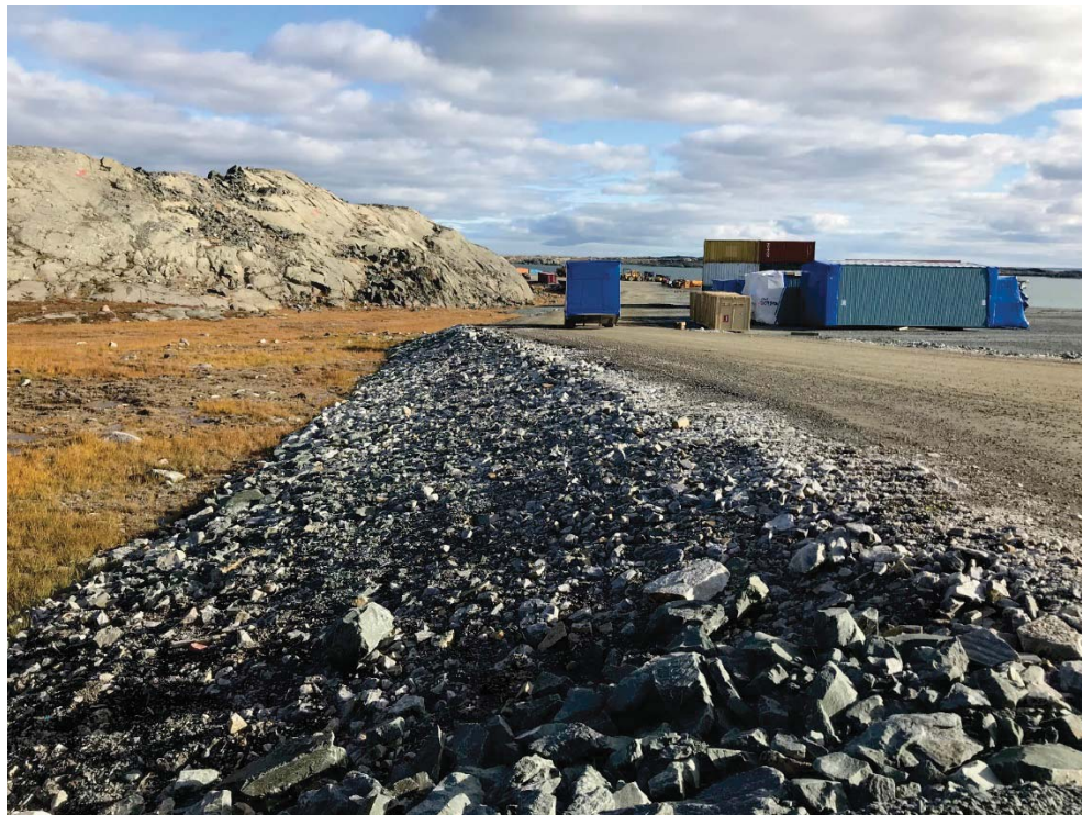
Photograph 5: Itivia Fuel and Laydown Area, Pad Slope on North Boundary of Facility, Looking East (14 September 2018).
