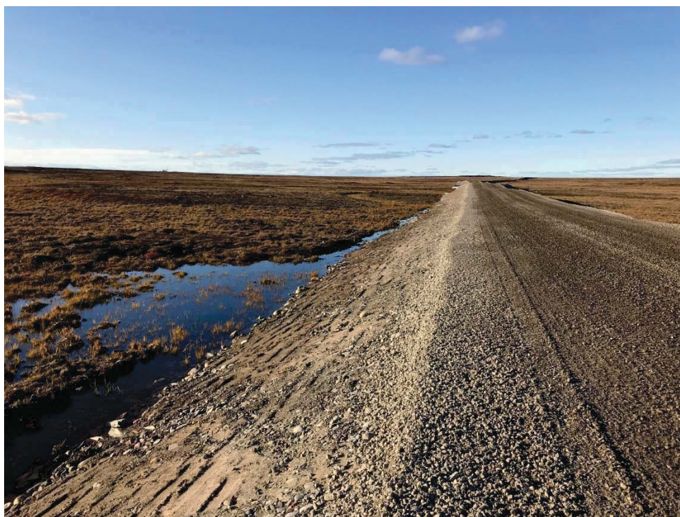
Photograph 38: Small Pond at KM 4.6 with Channel along Road Embankment Toe back to C11b, Looking North (14 September 2018)
