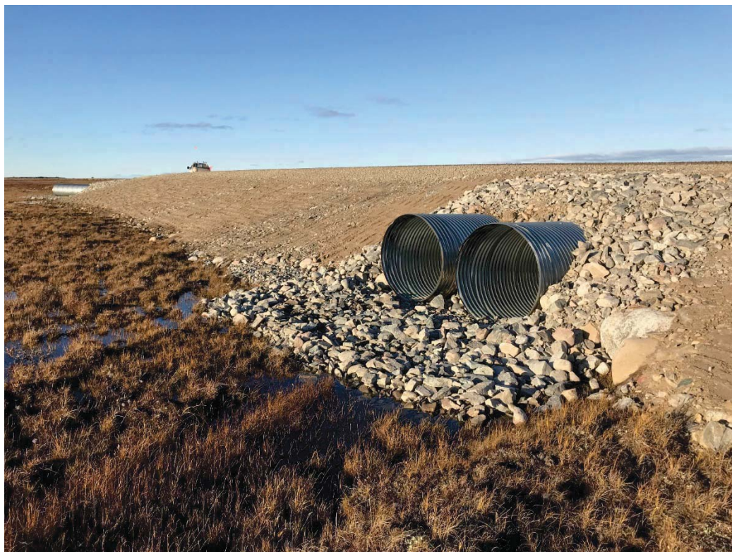
Photograph 43: Culvert 12a Inlet, Looking North (14 September 2018)
