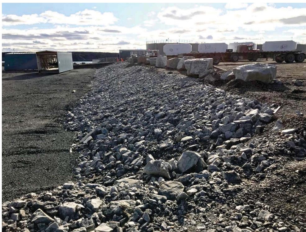
Photograph 6: Itivia Fuel and Laydown Area, Interior Slope, Looking South (14 September 2018).
