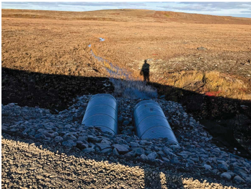
Photograph 41: Inlets and Upstream Drainage Channel for Culvert C11c, Looking East (14 September 2018)
