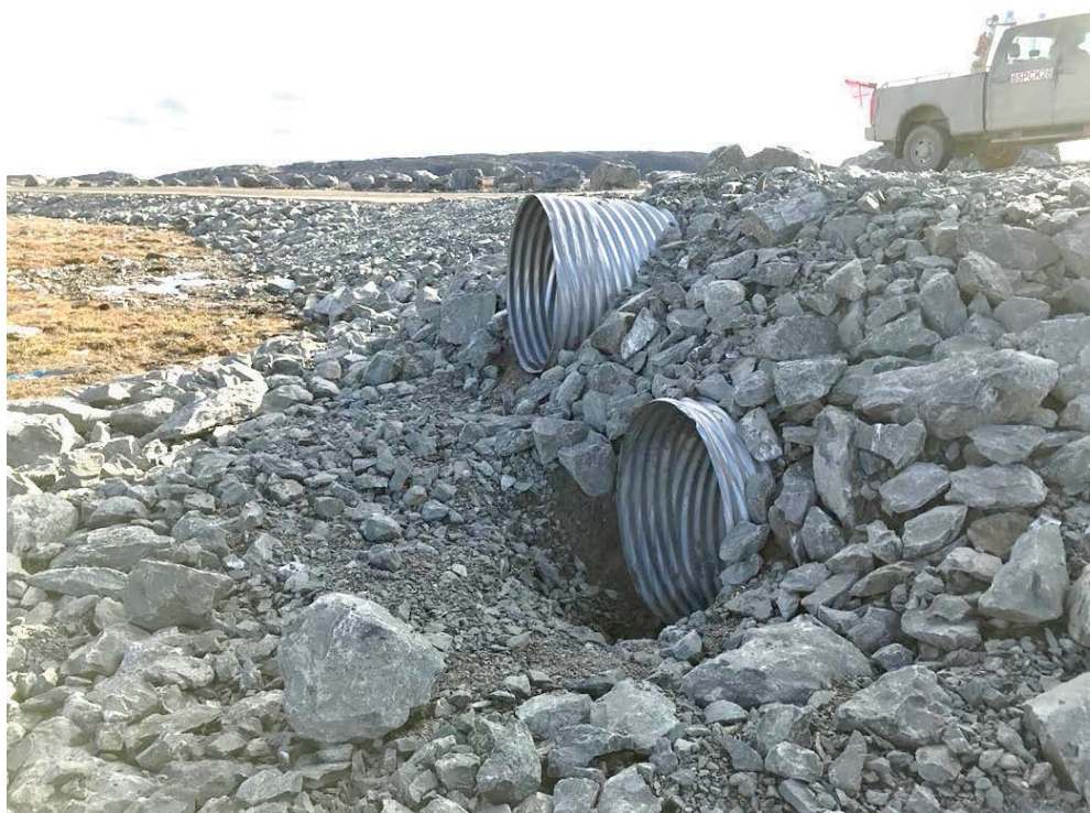
Photograph 12: Inlets of Culvert C01, Looking East (14 September 2018)
