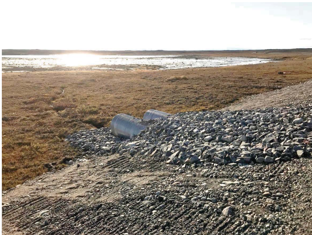
Photograph 31: Road Embankment and Outlets for Culvert C09, Looking West (14 September 2018)
