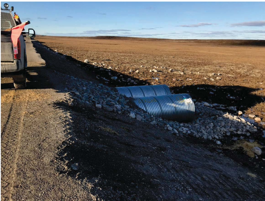
Photograph 36: Outlets of Culvert C11a, Looking North (14 September 2018)
