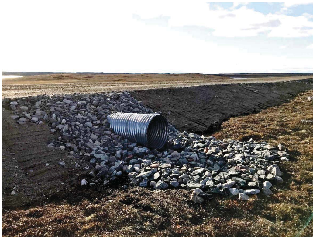
Photograph 24: Inlet for Culvert C06-1, Looking West (14 September 2018)
