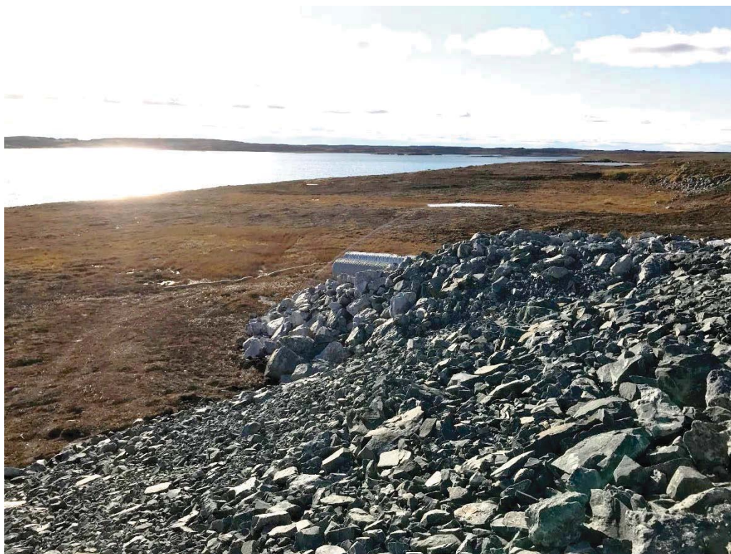
Photograph 16: Road Embankment and outlets for Culvert C03, Looking West (14 September 2018)
