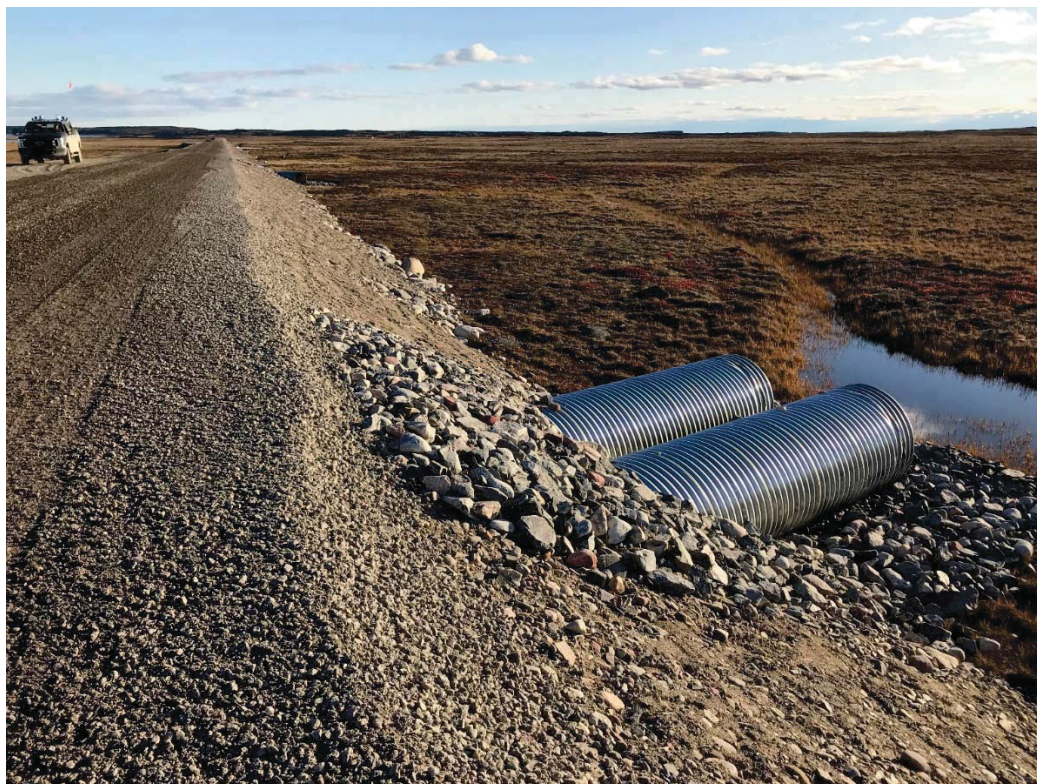
Photograph 42: Outlets and Downstream Drainage for Culvert 11c, Looking South (14 September 2018)
