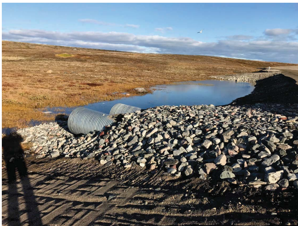
Photograph 30: Ponded Water to the East of Inlet for Culvert C09, Looking East (14 September 2018)
