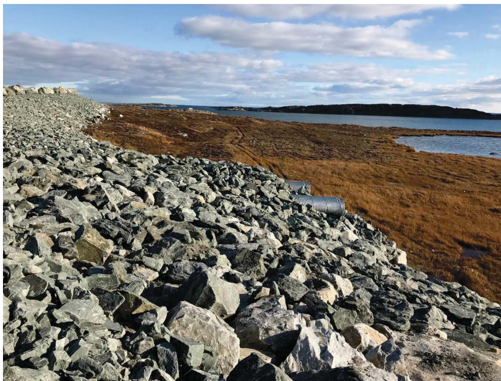
Photograph 18: Road Embankment and outlets for Culvert C04, Looking Southeast (14 September 2018)
