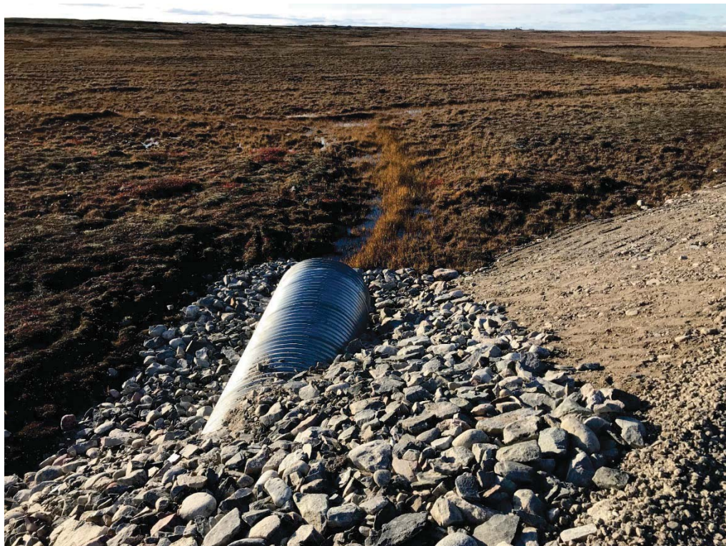
Photograph 39: Upstream Natural Drainage Path and Culvert C11b-1 Inlet, Looking West (14 September 2018)
