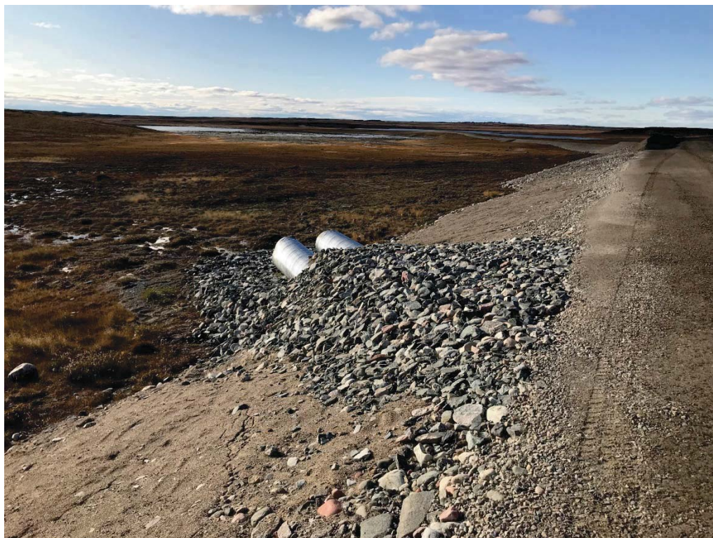
Photograph 27: Outlets of Culvert C07a, Looking West (14 September 2018)
