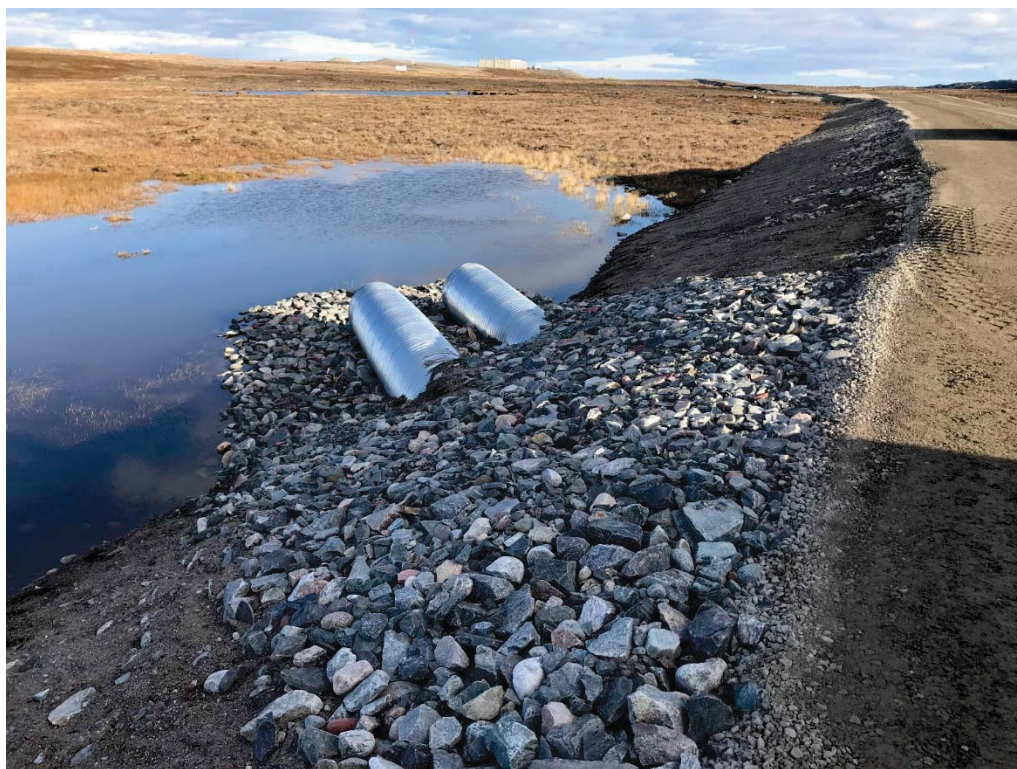
Photograph 26: Inlets and Upstream Poned Water at Culvert C07a, Looking East (14 September 2018)
