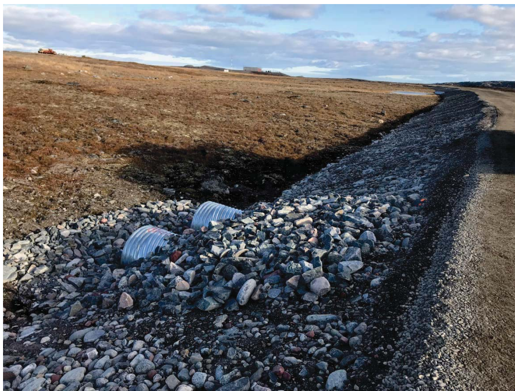
Photograph 28: Inlets of Culvert C07b, Looking East (14 September 2018)
