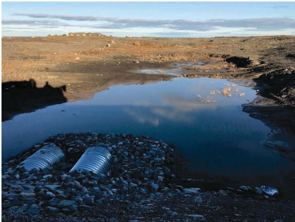
Photograph 47: Culvert 13 Inlets, Ponded Water Upstream and Below the Culvert Inverts, Looking East (14 September 2018)
