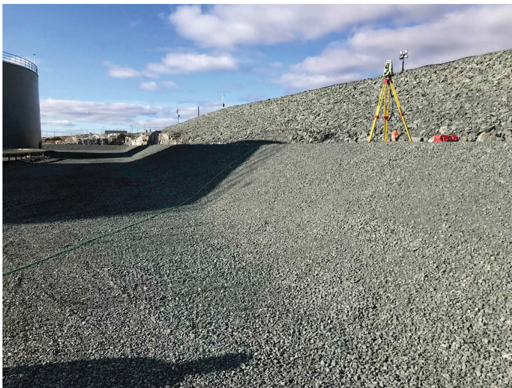
Photograph 8: Itivia Fuel and Laydown Area, Interior North Slope of Fuel Storage Facility, Looking West. (14 September 2018).
