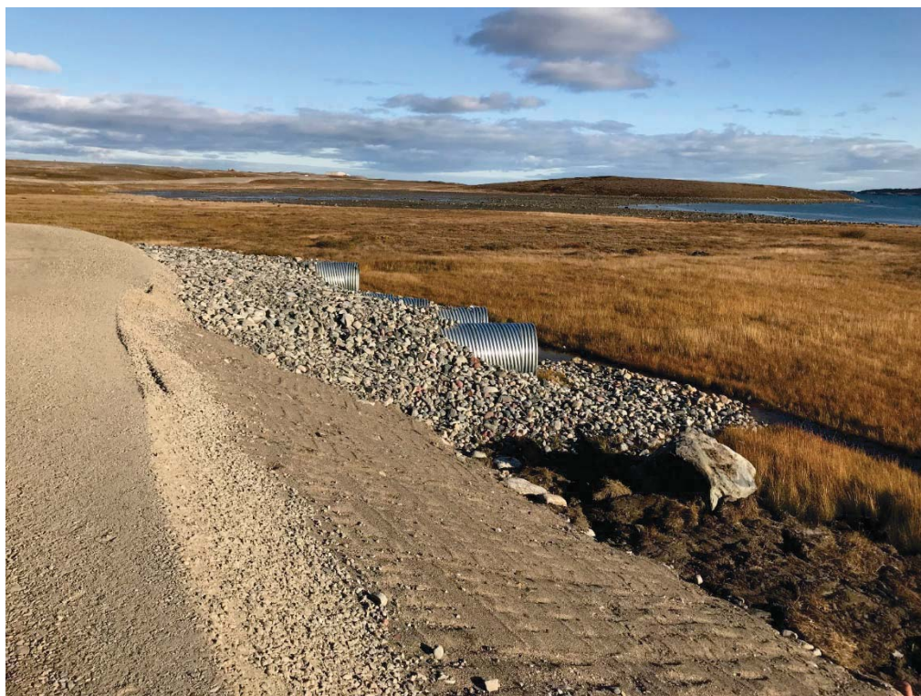
Photograph 34: Outlets for Culvert C10, Looking Southeast (14 September 2018)
