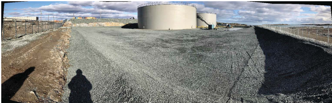
Photograph 7: Itivia Fuel and Laydown Area, Overview of Interior of Fuel Storage Area, Looking Northeast from Southwest Corner. (14 September 2018).
