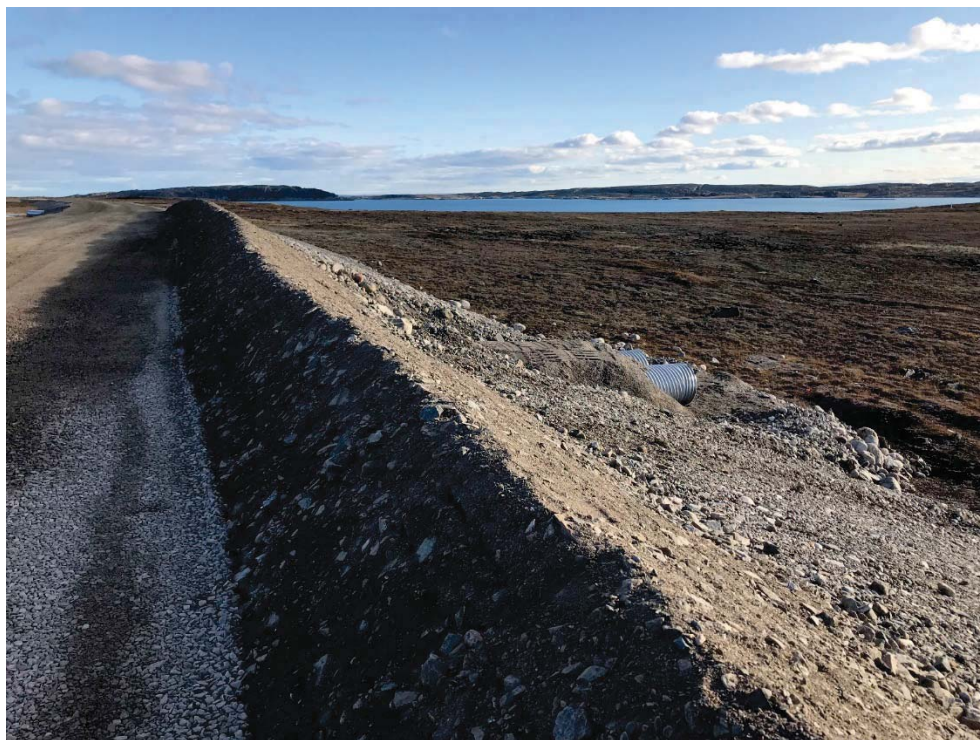
Photograph 29: Safety Berm and Embankment Slope over Culvert C07b Outlets, Looking Southeast (14 September 2018)
