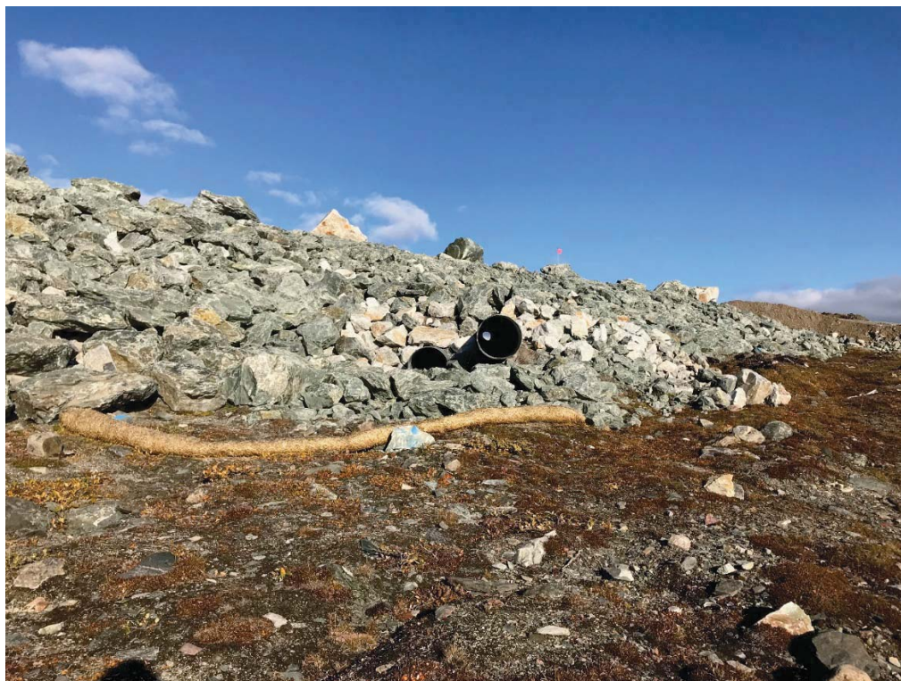
Photograph 13: Outlets for Culvert C02, Looking Northeast (14 September 2018)
