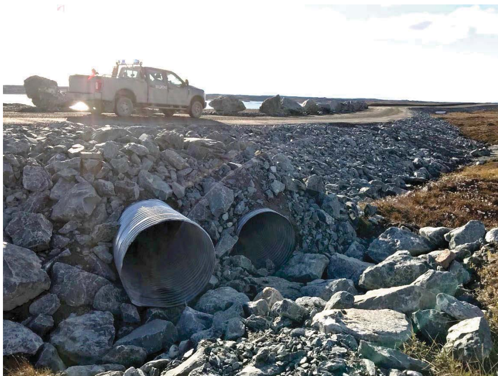
Photograph 17: Inlets for Culvert C04, Looking West (14 September 2018)
