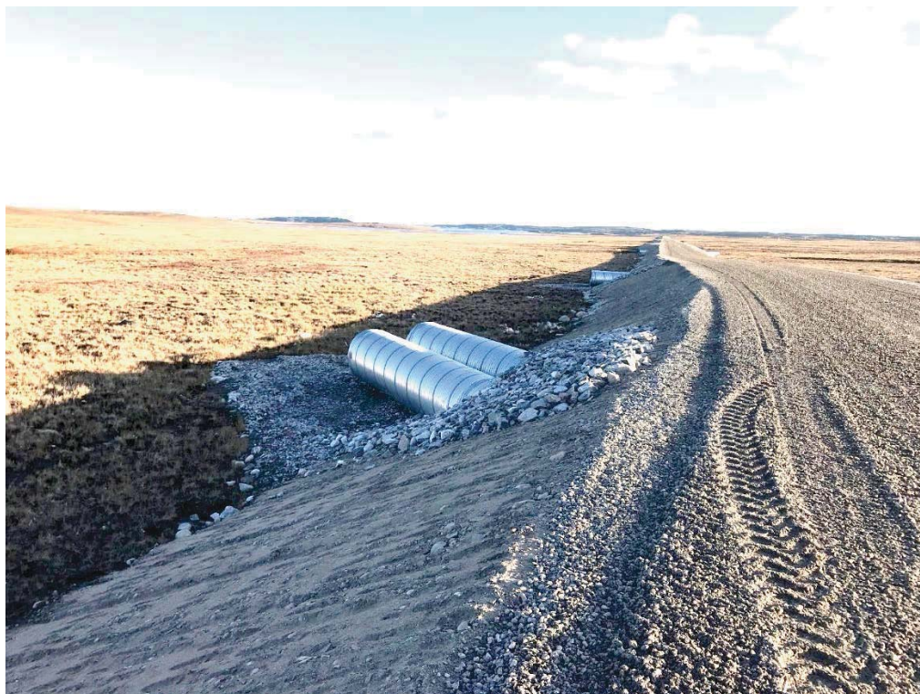
Photograph 45: Culvert 12b Inlets, Looking Southeast (14 September 2018)
