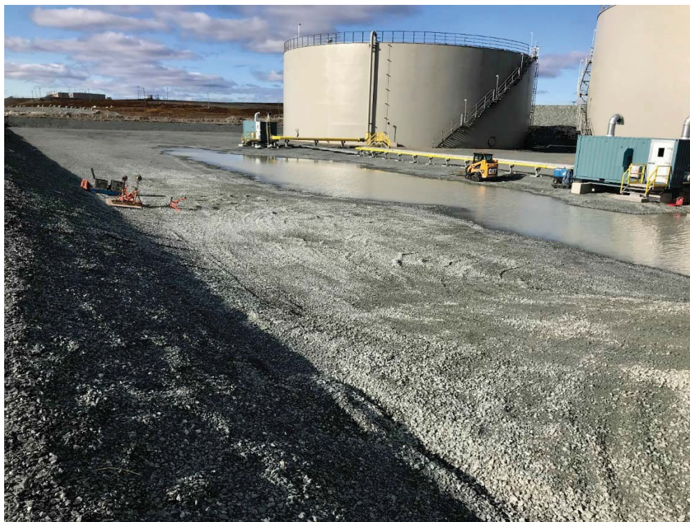
Photograph 11: Itivia Fuel and Laydown Area, Water Poned on South Side of Tanks, actively being pumped at time of inspection, Looking Northwest. (14 September 2018).
