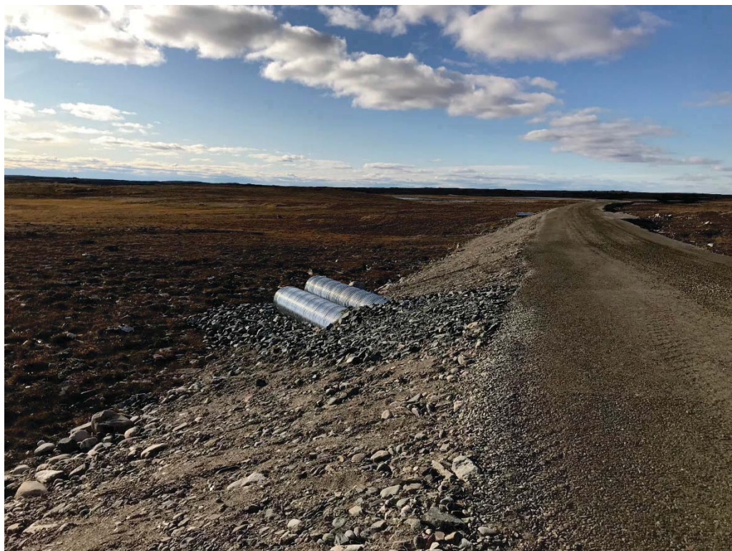
Photograph 23: Outlets of Culvert C06 and Road Embankment, Looking Northwest (14 September 2018)
