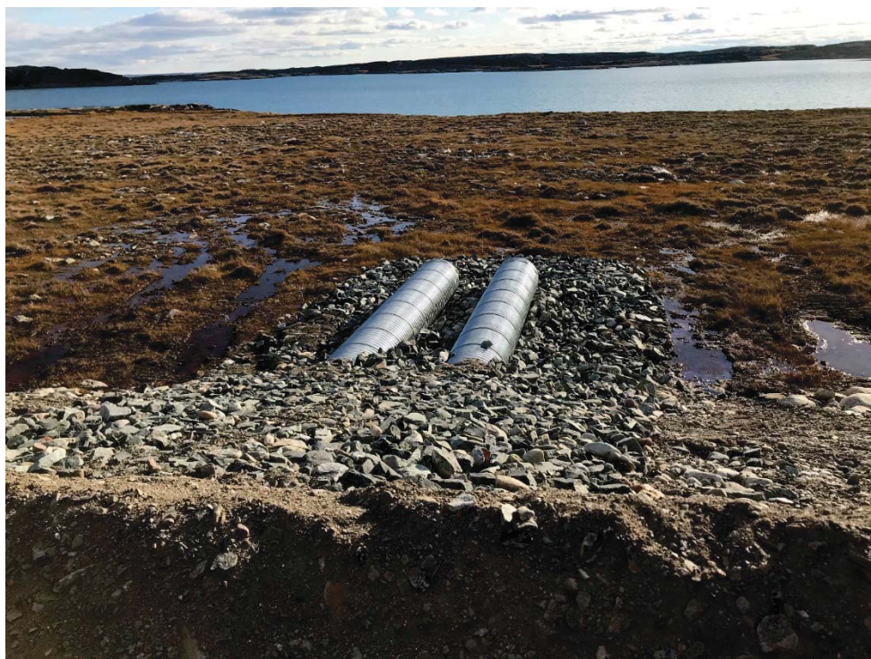
Photograph 20: Outlets for Culvert C05, Looking Southwest (14 September 2018)
