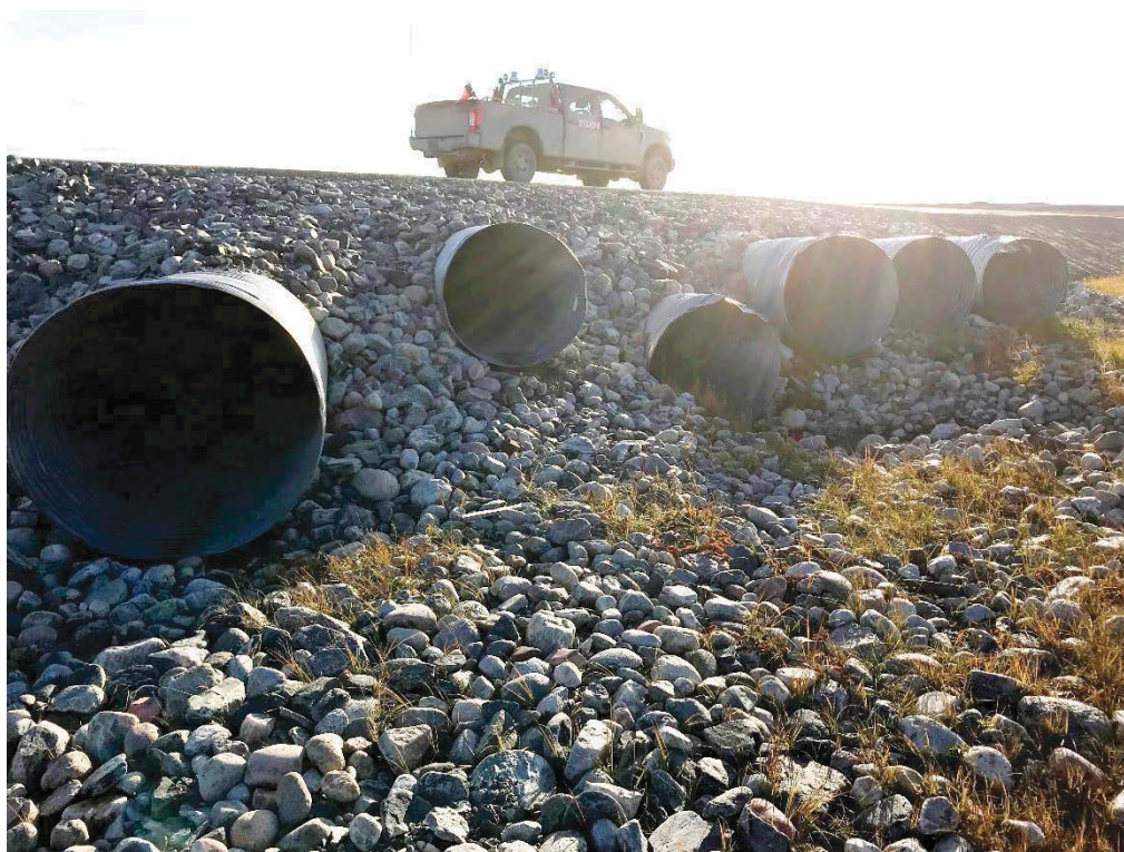
Photograph 33: Inlets for Culvert C10, Looking South (14 September 2018)
