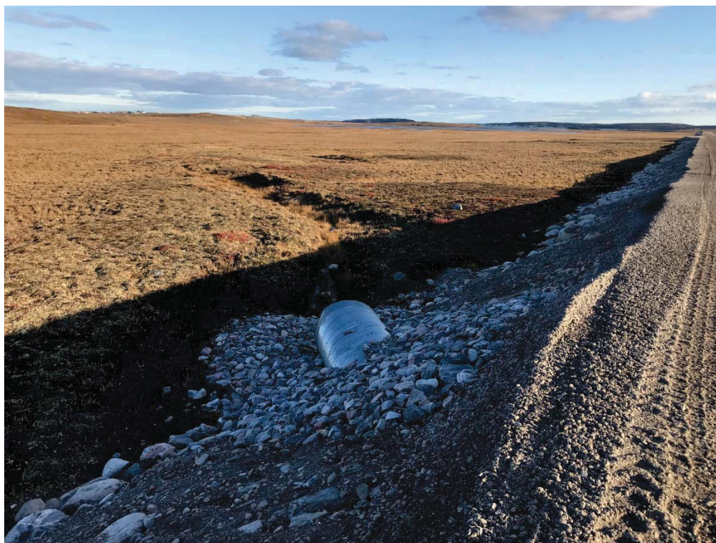
Photograph 40: Culvert C11b-1 Outlet and Downstream Drainage Channel, Looking Southeast (14 September 2018)
