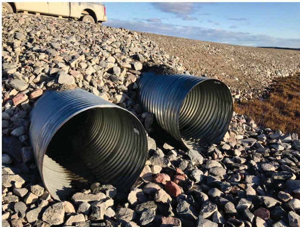
Photograph 37: Inlets of Culvert C11b. Flow through Left Culvert, Looking East. Minor Amount of Riprap in Front of Culvert Should be Removed. (14 September 2018)
