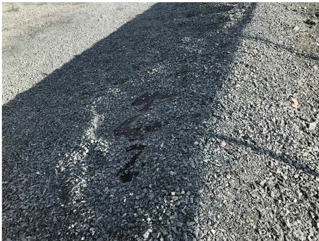
Photograph 9: Itivia Fuel and Laydown Area, Liner Exposed on Interior Slope of South Berm. (14 September 2018).
