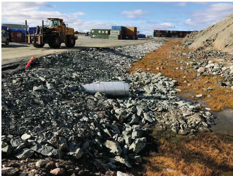
Photograph 1: Inlets of Culverts at Entrance to Itivia Fuel and Laydown Area, Looking Southwest (14 September 2018).
