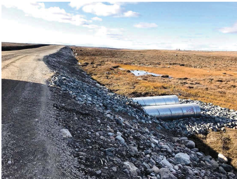
Photograph 19: Road Embankment and Inlets for Culvert C05, Looking Northwest (14 September 2018)
