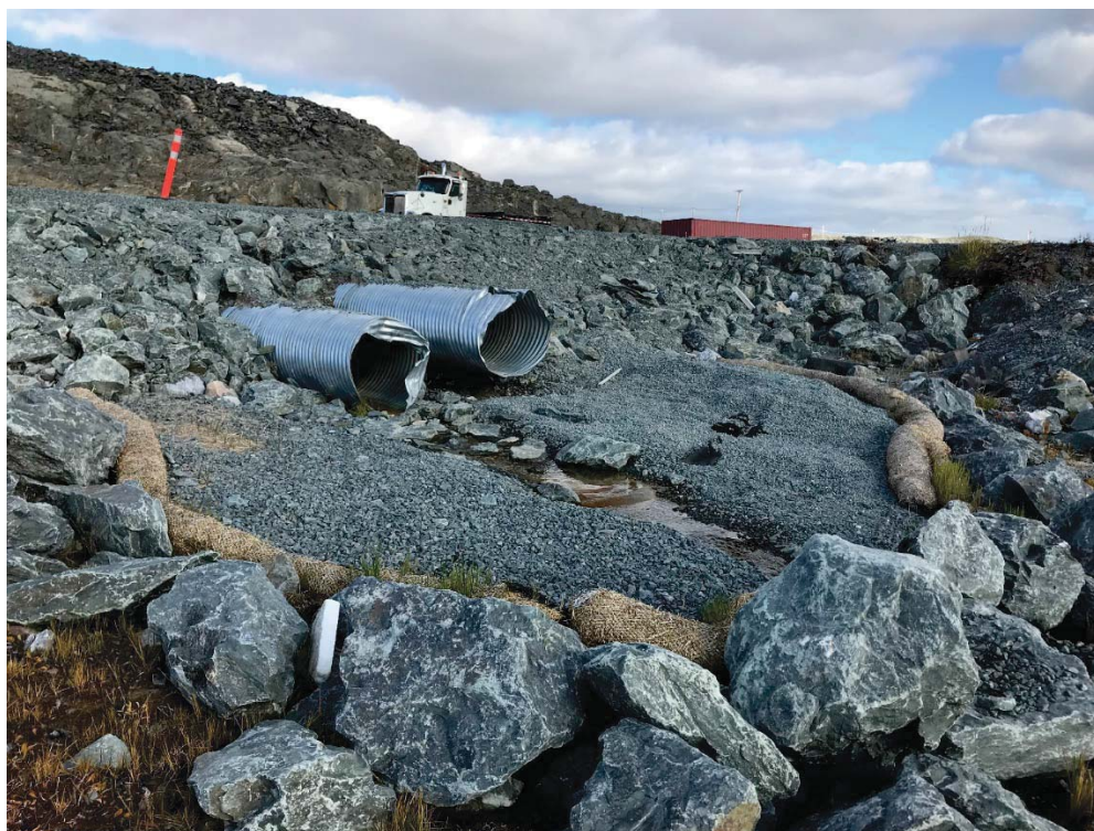
Photograph 2: Outlets of Culverts at Entrance to Itivia Fuel and Laydown Area, Looking North (14 September 2018).
