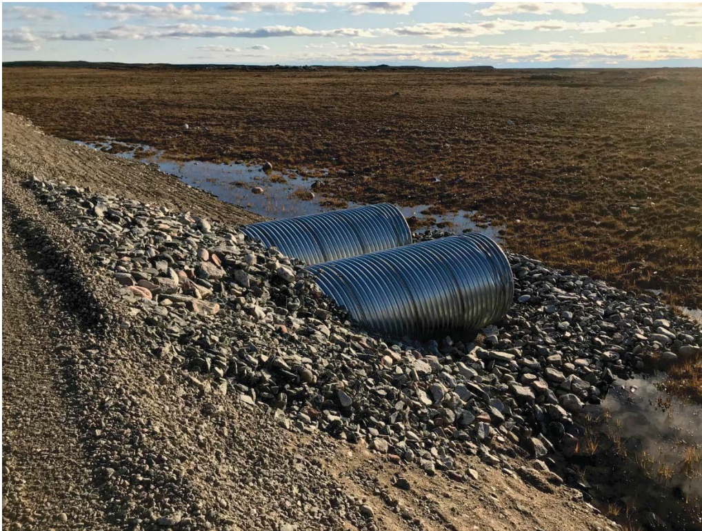
Photograph 35: Inlets of Culvert C11a, Looking Southwest (14 September 2018)
