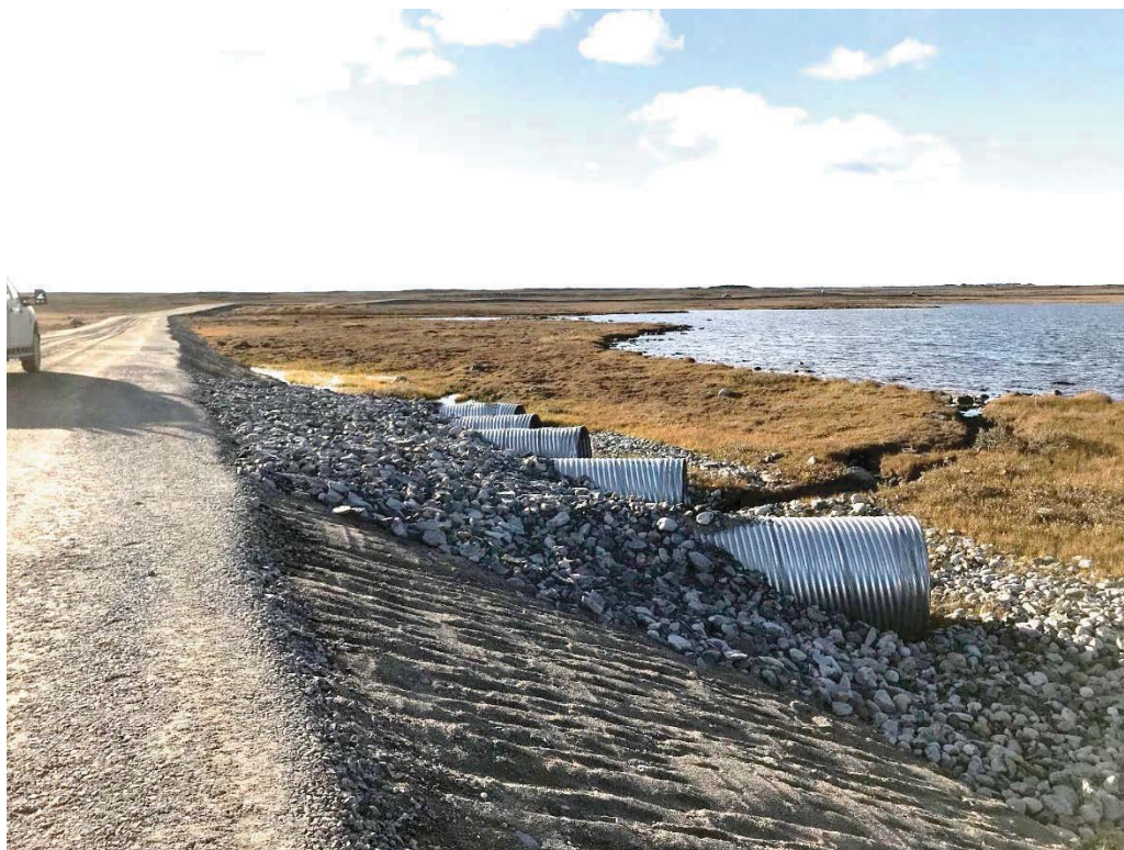
Photograph 32: Inlets for Culvert C10, Looking East (14 September 2018)
