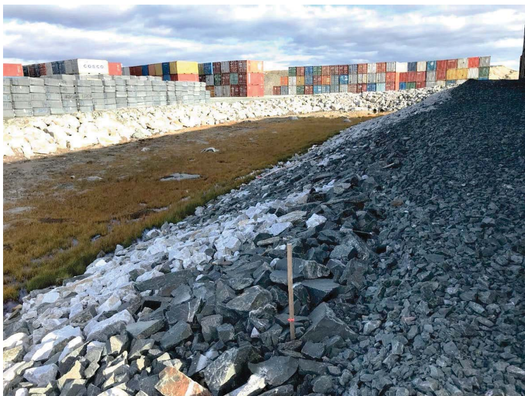
Photograph 4: Itivia Fuel and Laydown Area, Pad Slopes on West End of Facility, Looking North (14 September 2018).
