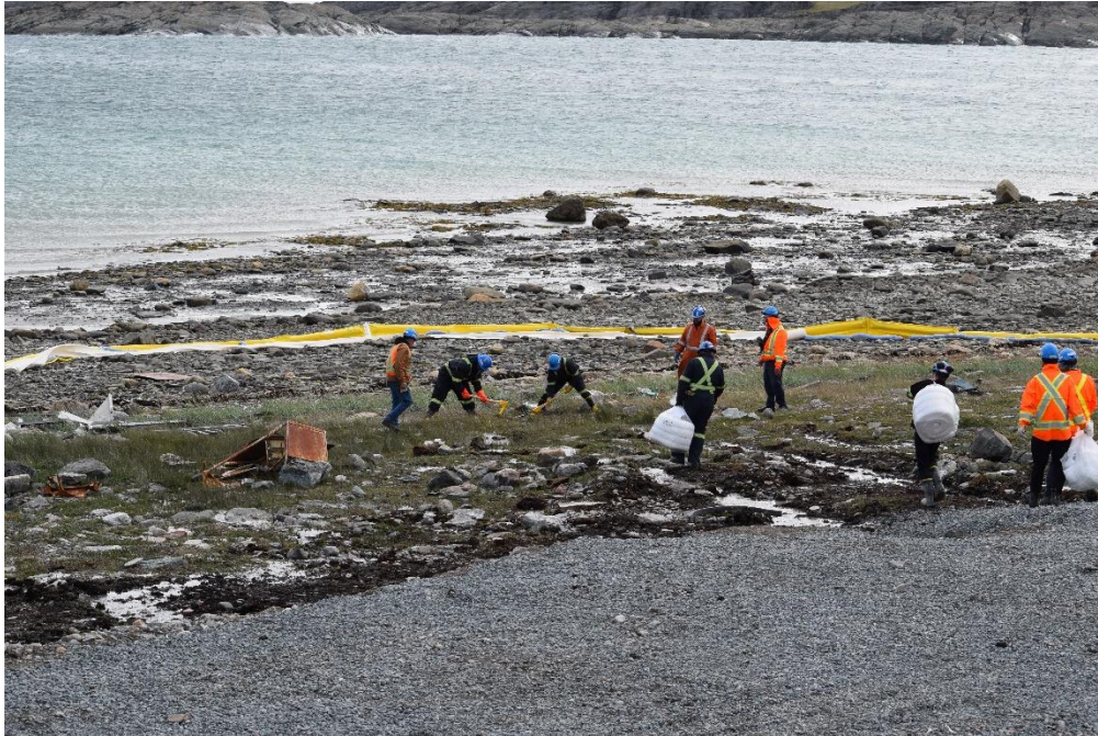
16:04 – Absorbent padding was placed on top of spill where visible product was observed behind marine barrier (wind blowing toward shore)
