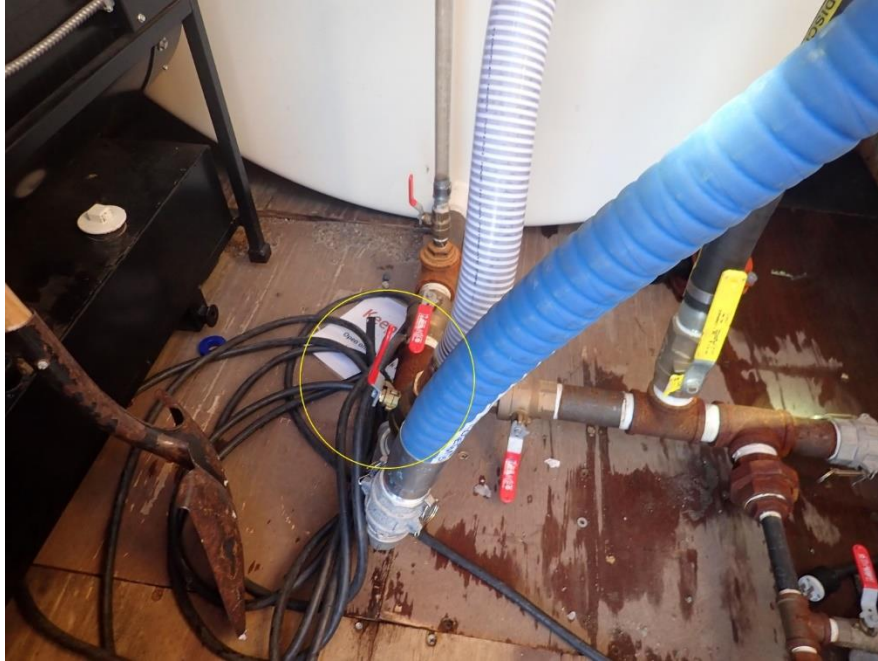
Picture 2: Release valve left open causing the spill.
