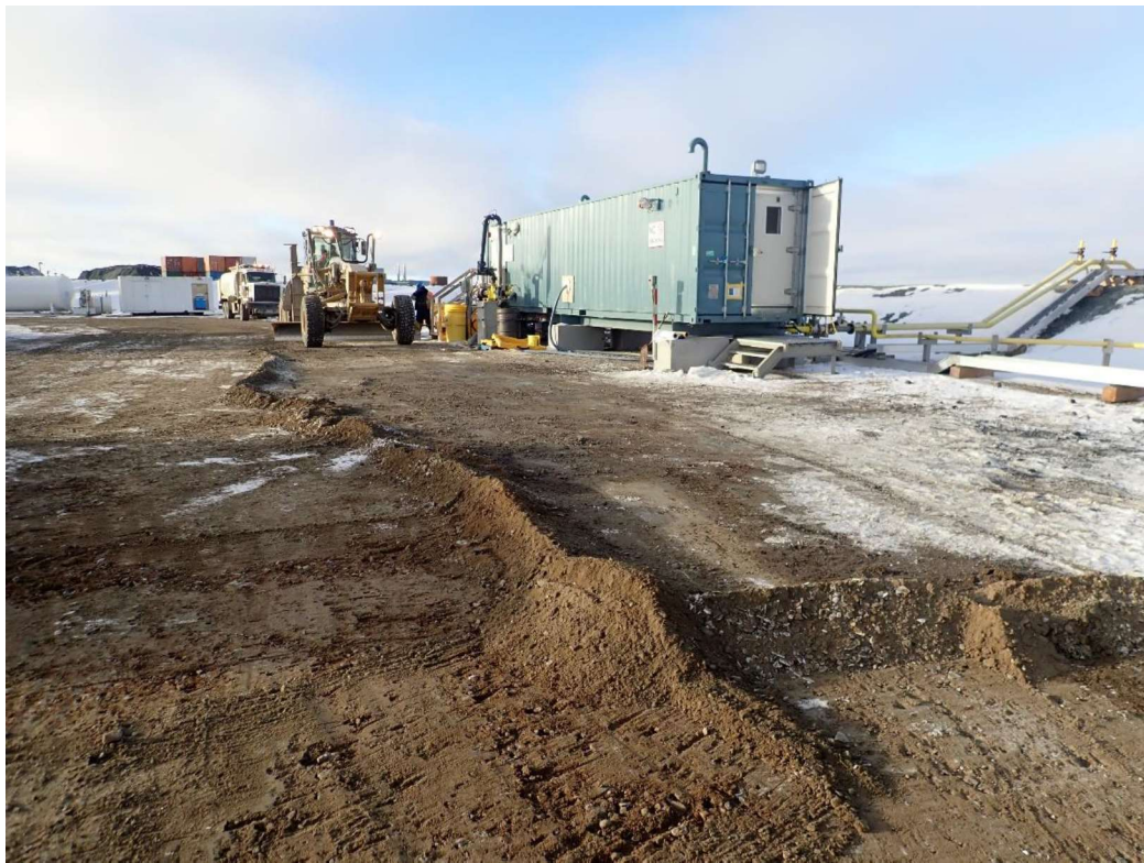
Photo 2: Scrapping of the surface material
