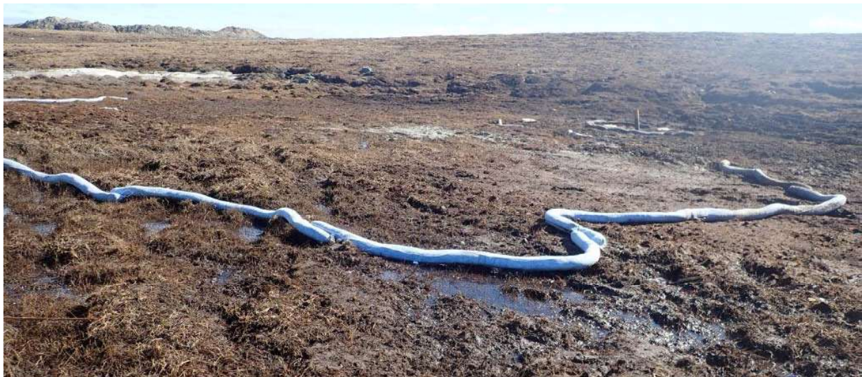
Figure 1: Booms placed downstream of spill location.
