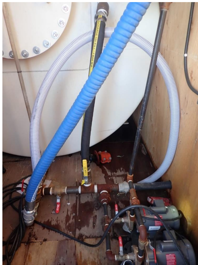
Picture 3: Discharge hose connected to retention tank release valve.
