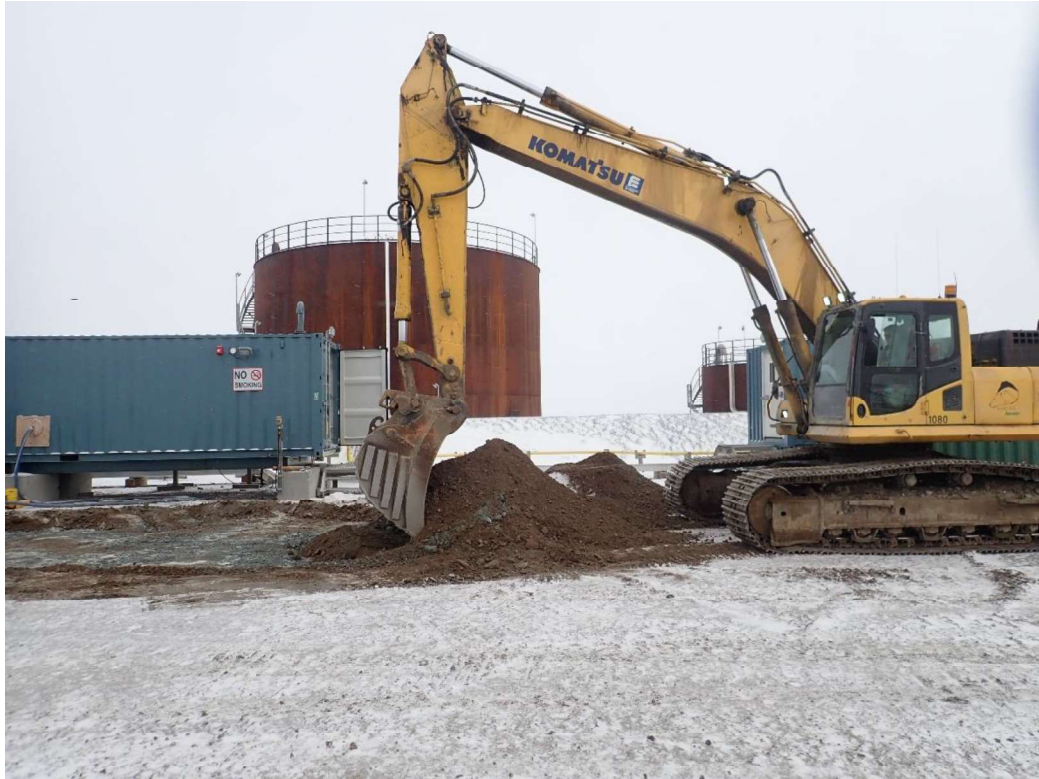
Photo 3: Excavation of the contaminated material
