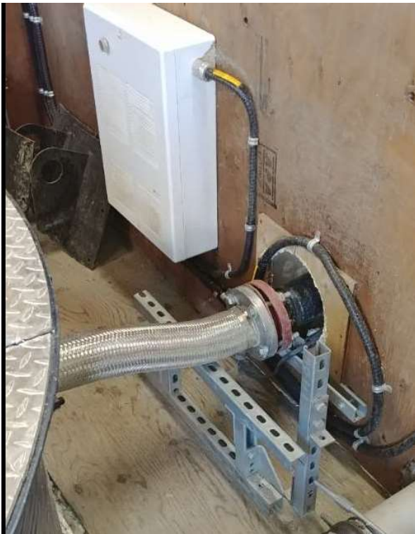
Figure 1: Newly installed flexible hose.
