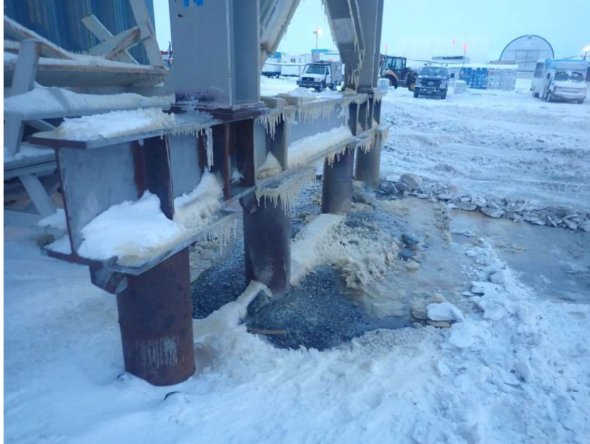
Figure 1: Water from boiler recirculation system flowing to ground.
