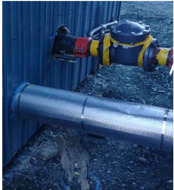
Figure 2: Insulated piping outside the MSB sewage lift station.
