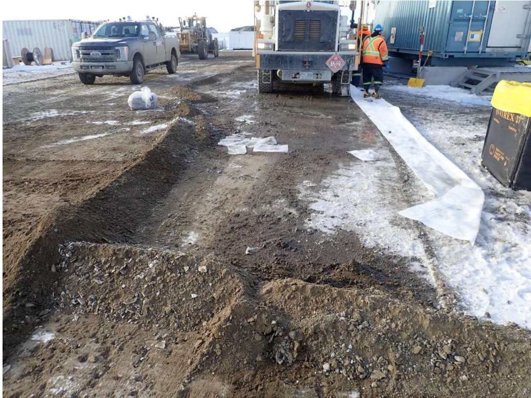
Photo 1: Contain the spill with berm and absorbent pads
