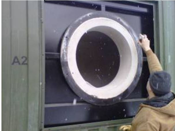
Gasket adhesive spray being applied
