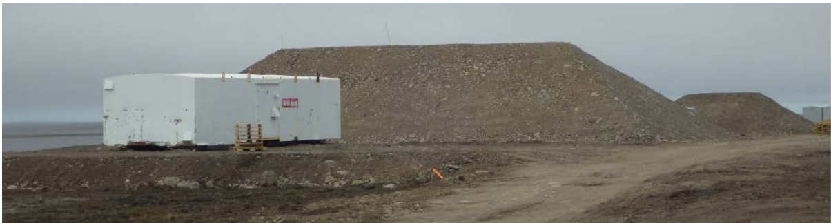
Figure 3-4 Surface Explosive Magazines and Berms
