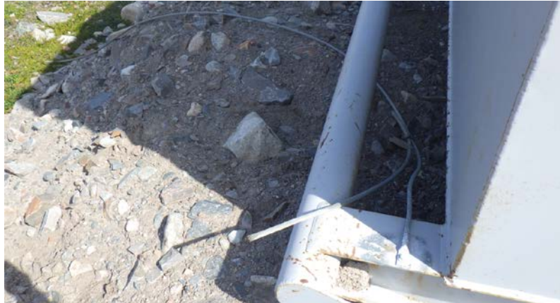
Figure 3-5 Surface Explosive Magazines – Grounding
