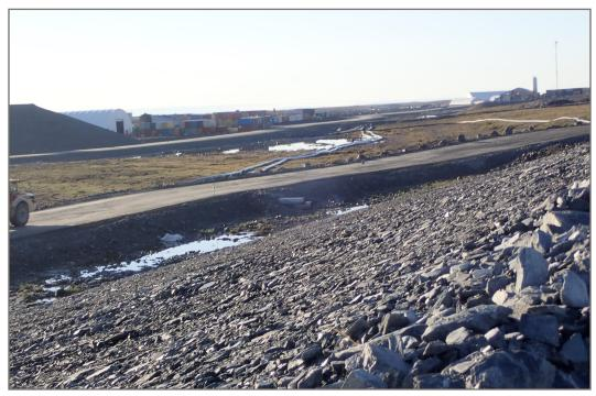
Photo 12: TSF - Rockfill covered TSF slope
