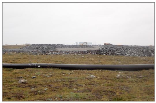
Photo 4: WRSF3—Initial lifts of waste rock in WRSF3
