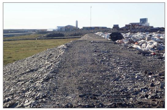
Photo 2: Landfill—East berm, waste close to crest.
