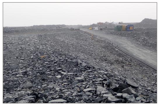
Photo 14: SP4—Rockfill covered overburden slope.
