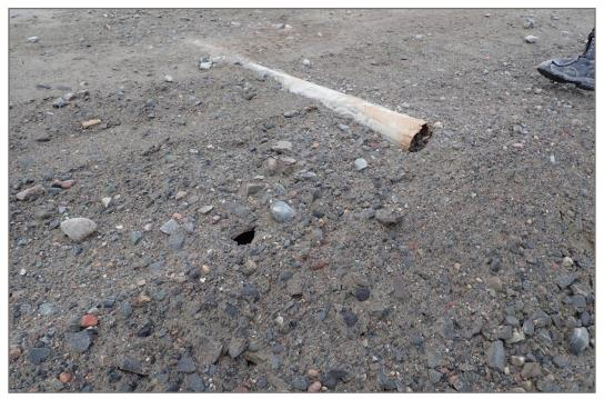
Photo 33: Culvert 26.2, Both inlets blocked with road fill.
