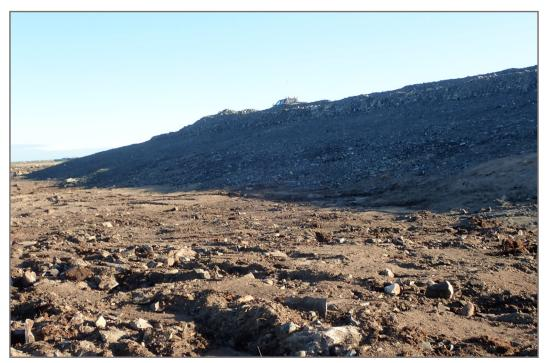
Photo 13: TSF - Rockfill covered TSF slope above CP3.
