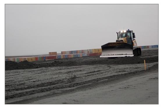
**Photo 8:** TSF - Spreading tailings, prior to compaction.
