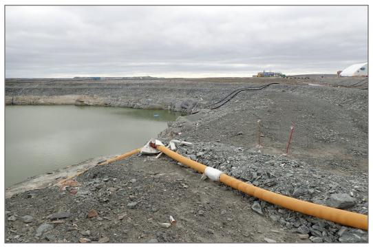
**Photo 3:** SP1 Saline Pond - discharge line into pond.
