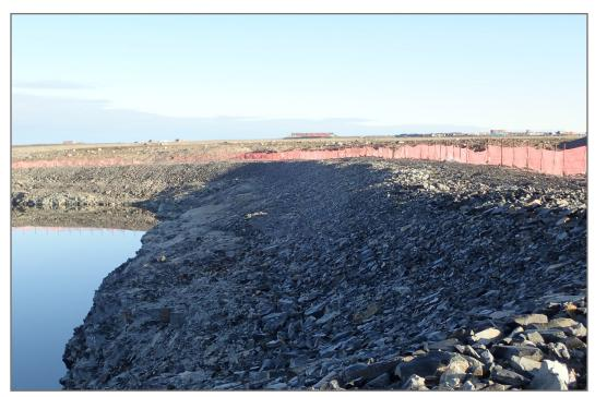
Photo 9: Pond CP3 - Rockfill covered overburden slope.
