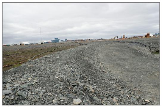
Photo 4: SP1 Saline Pond - thermal berm at crest.
