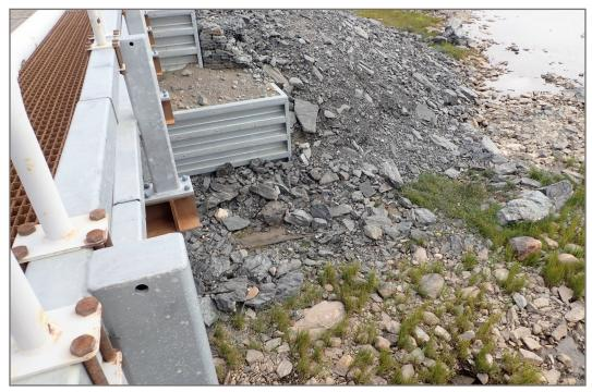
Photo 20: M-5 Bridge—Geotextile exposed at north abutment .
