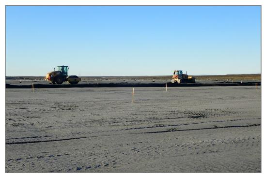
**Photo 3:** TSF - Placing and compacting tailings.
