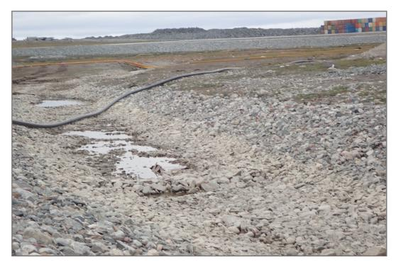
Photo 20: Channel 5—Settlement and ponding
