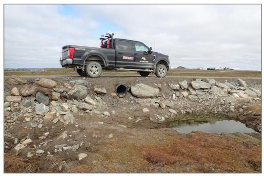
**Photo 38:** Culvert 29.6 - HDPE Culvert, inlet collapse approximately 25%.
