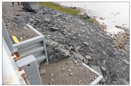
Photo 19: M-5 Bridge—Gabion North Abutment
