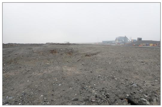
Photo 2: WRSF1 - Winter placed till—relatively wet, and settling.
