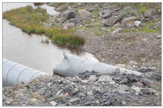
Photo 8: Culvert km 7.4—Damage to culvert inlet
