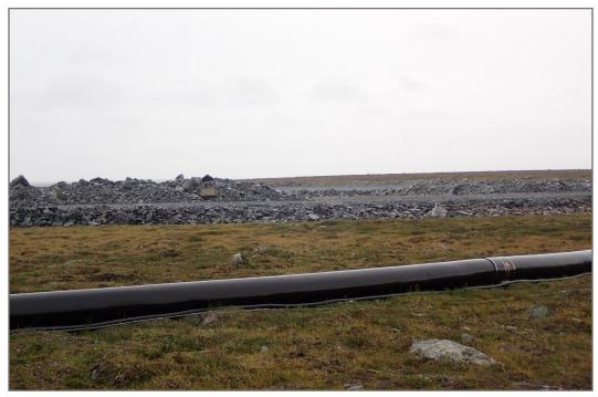
Photo 5: WRSF3—Initial lifts of waste rock in WRSF3
