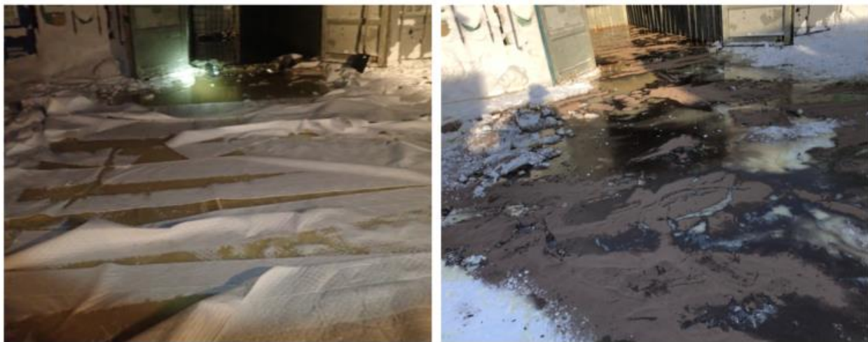
Figure 3: Initial clean up response, absorbing and slowing the spread of the oil.
