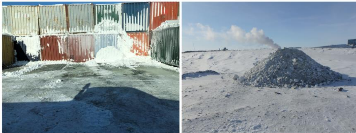
Figure 4: Initial clean-up of the area after sea-cans removed and loader began removing material (Left). Contaminated material brought to the landfarm (Right).
