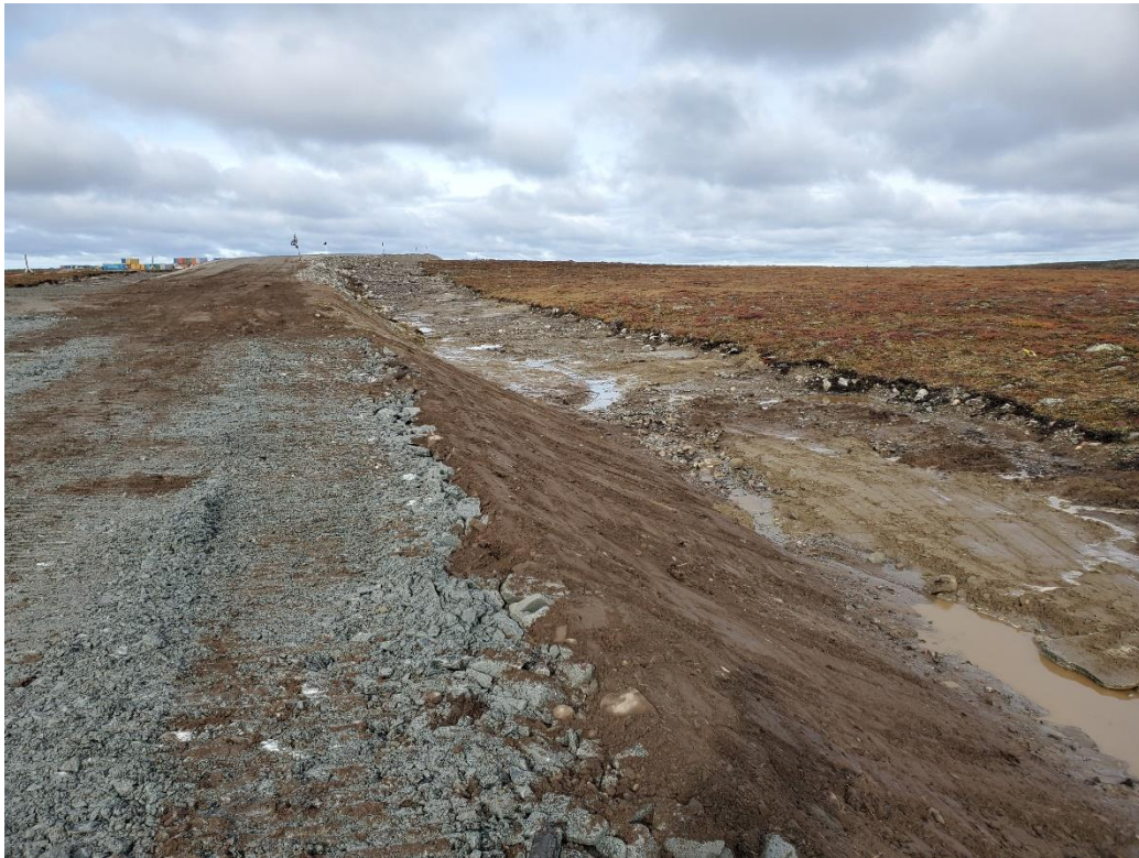
Figure 5: Road widened, and drainage channel restored.
