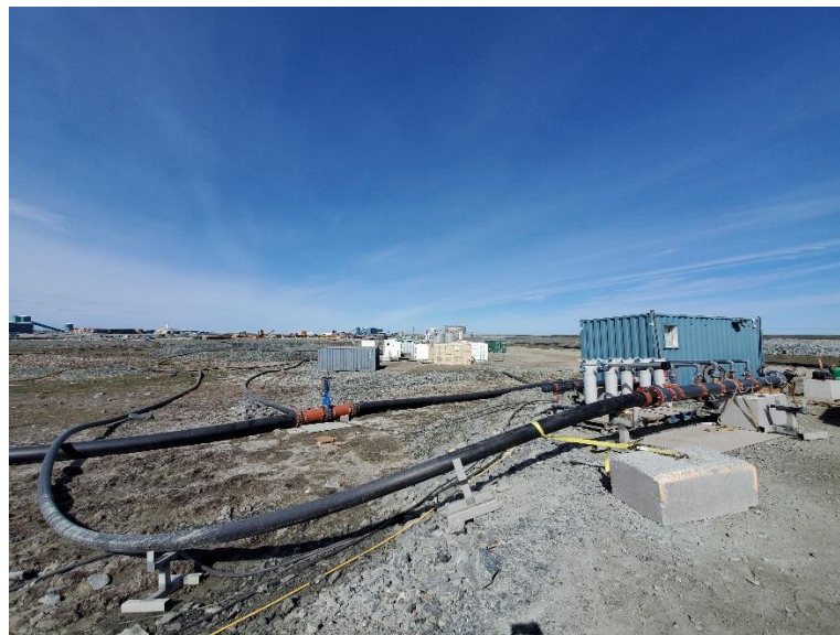
Figure 3: Piping replaced from SP3 to loading station.
