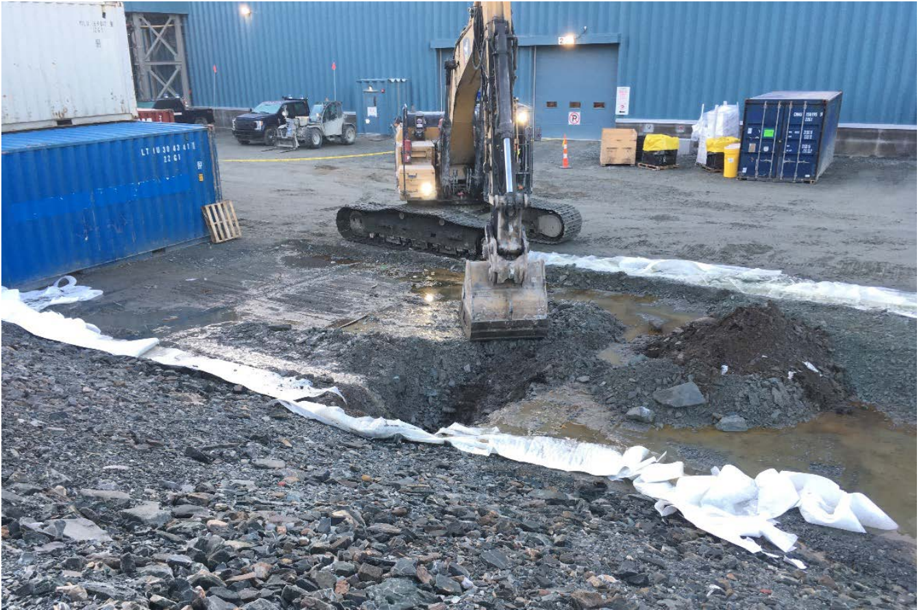
Figure 9: Digging Containment Trenches
