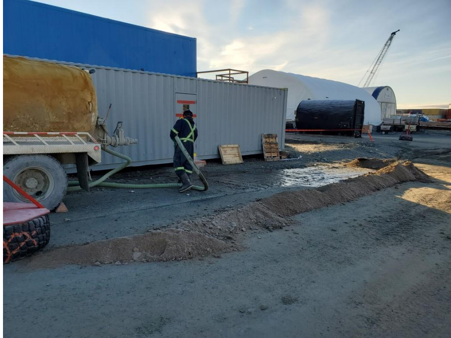
Figure 2: Soil berm deployed to isolate the spill. Vacuum truck used to removed spill material.
