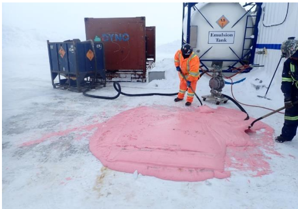
Figure 4: Spilled emulsion being pumped to emulsion bin.
