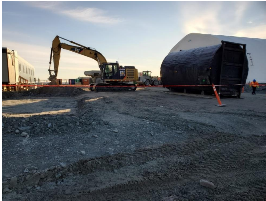
Figure 4: Construction of pad for addition of new equalizing tank.
