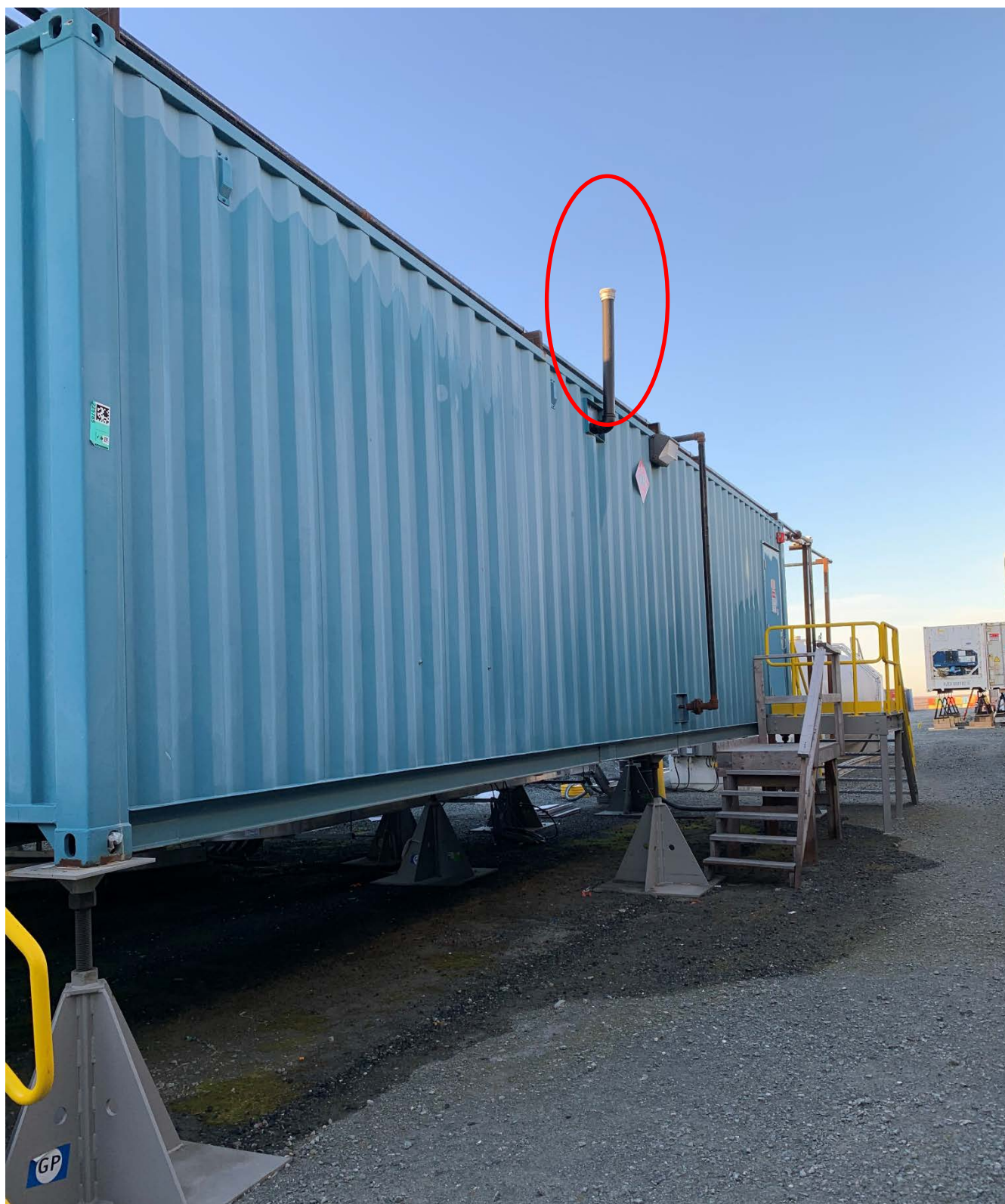
Figure 11: CCEG Daily Tanks Vent Missing Piping to Main Camp Complex Tank
