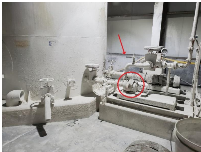
Figure 2: Calcium Hydroxide solution sprayed from the ruptured seal (circled) and seeped out between the cladding and concrete (arrow).
