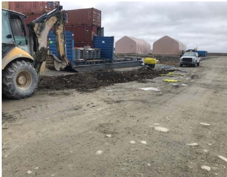
Figure 3: Contaminated gravel being removed from Jet A spill area.
