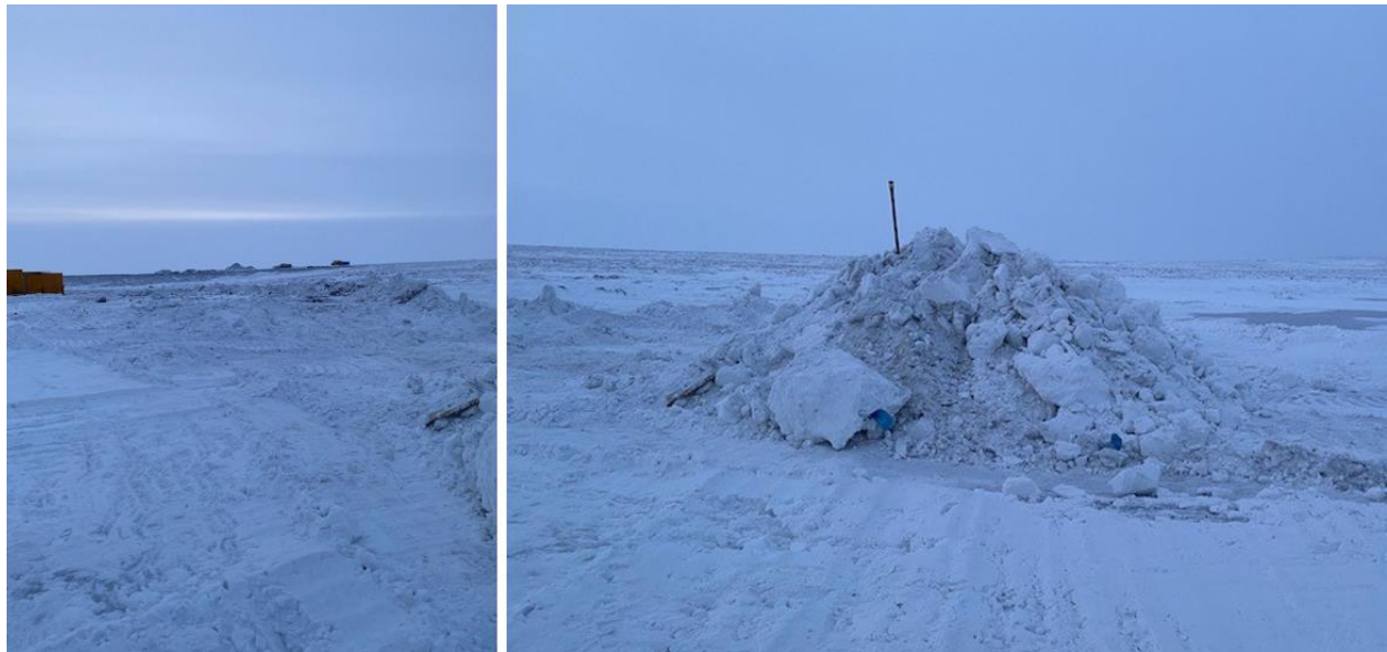
Figure 4: All contaminated snow and ice was scraped into a pile and brought to the snow cell.
