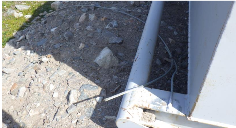
Figure 3-5 Surface Explosive Magazines – Grounding
