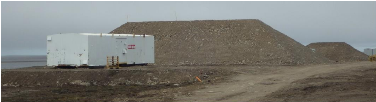
Figure 3-4 Surface Explosive Magazines and Berms
