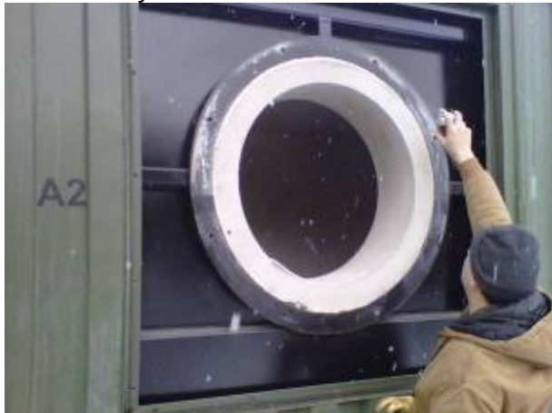
Gasket adhesive spray being applied
