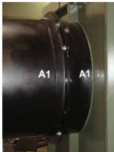
Correctly Installed Breech on Primary Chamber
