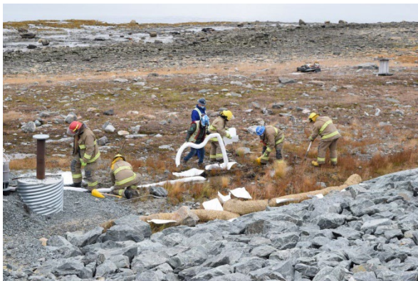
Photo 4: Deploying absorbent booms and sediment control logs
