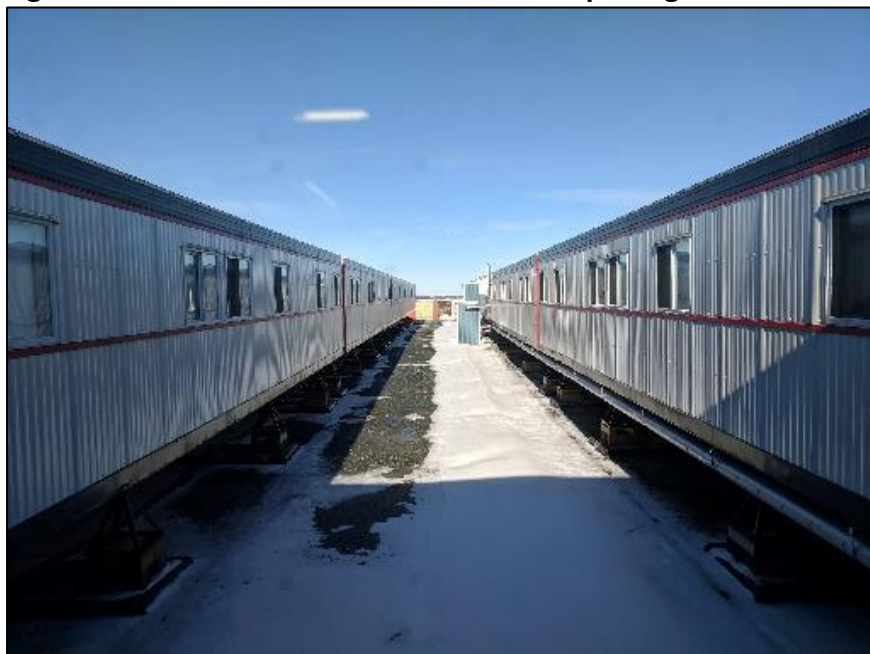
Figure 5: Snow Removal from Between Camp Wings
