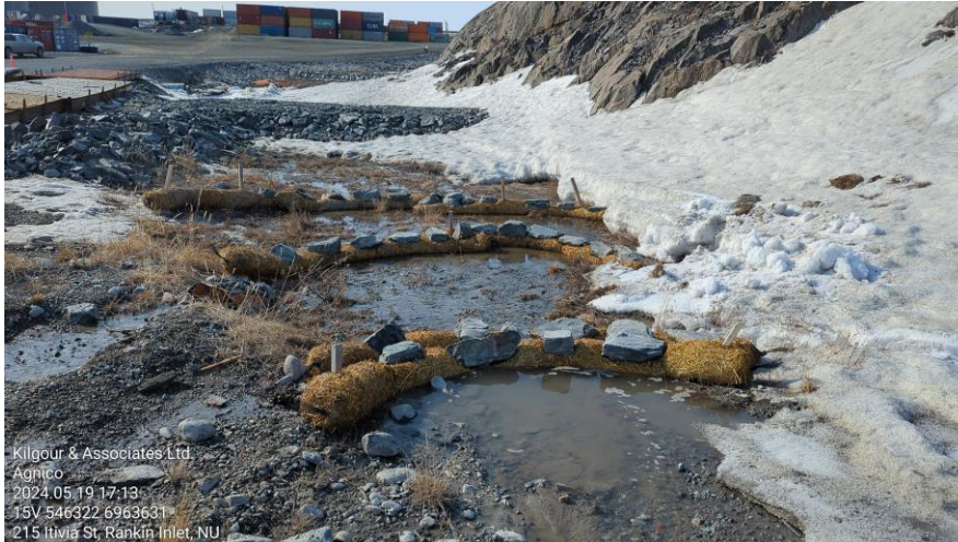
Photo 4. Straw logs placed between Itivia Upstream West and Itivia Culvert to mitigate the sediment loading.
