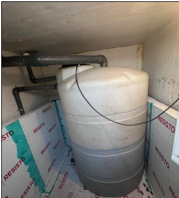
Photo 4: New sewage tank installed.
