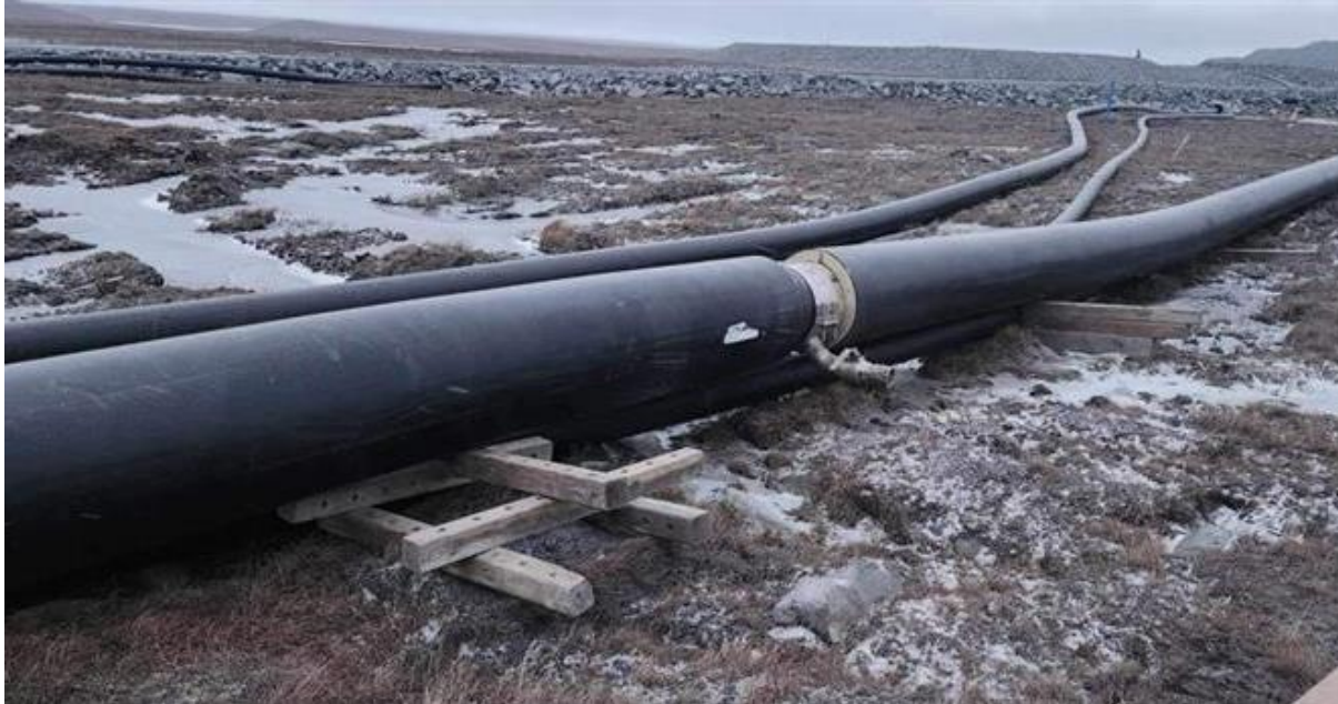
Photo 3: Repair leak and cribbing at the area of the treated water release.
