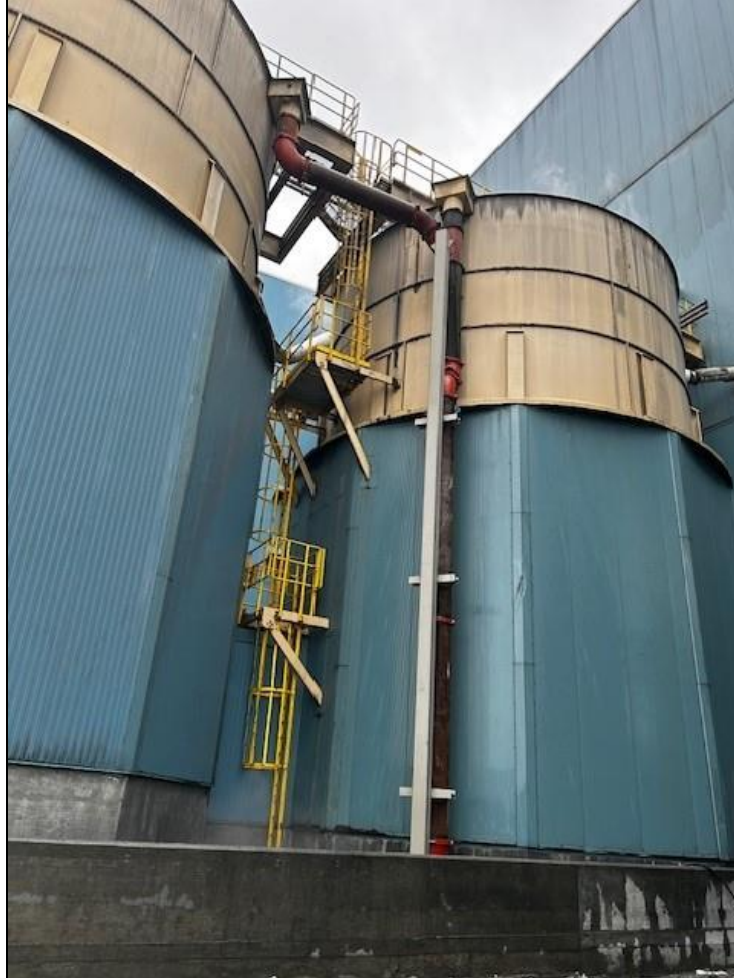
Photo 5: Completed corrective action of extending the secondary overflow collection pipe to discharge directly into the containment berm wall.
