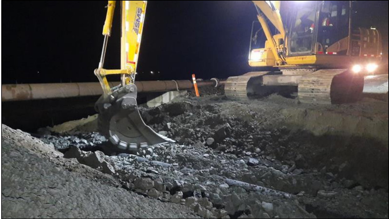
Photo 1: Trench being excavated for installation of temporary HDPE drainage pipe.
