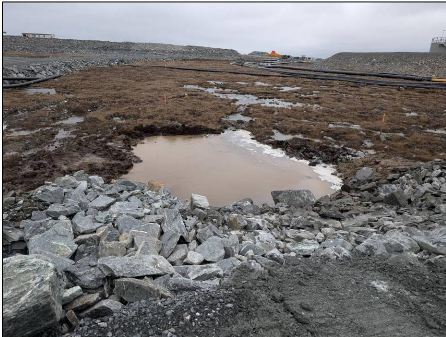
Photo 2: Sump excavated to collect the treated water.
