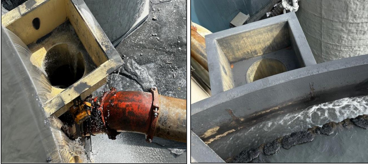
Photo 2: Secondary overflow collection pipe was ineffective in capturing overflow as the tank wall blocked the flow of water into the collection pipe. Photos of both tanks are shown prior to corrective actions being implemented.
