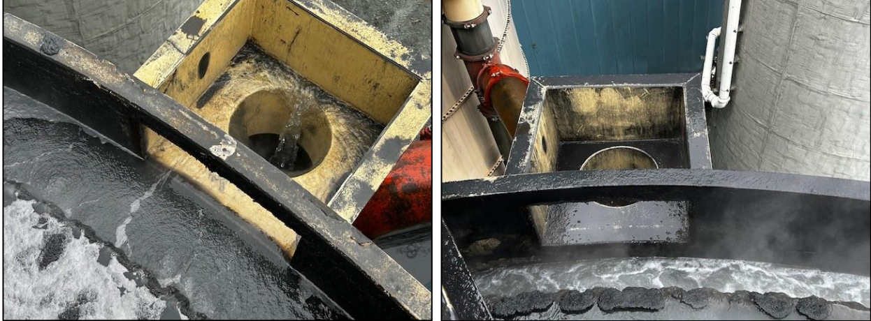
Photo 4: Completed corrective action of cutting-away the tank wall to allow overflow to enter the secondary overflow collection pipe from both tanks.
