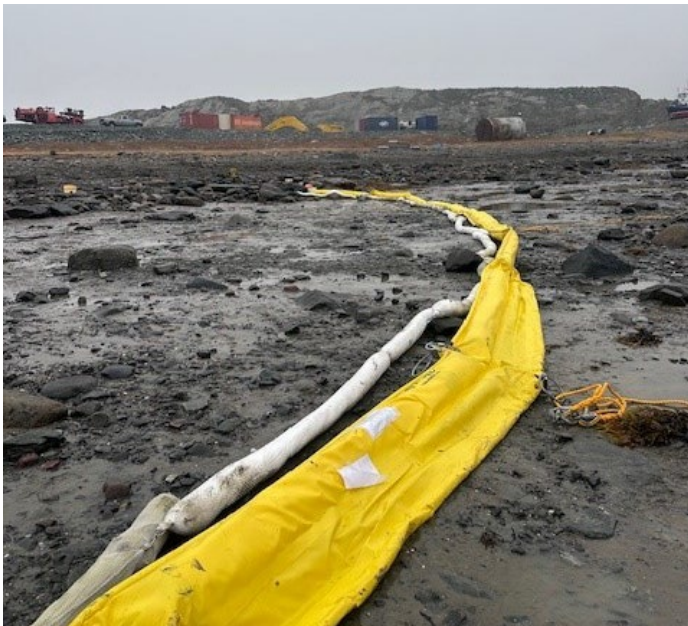
Photo 4: Marine booms installed along shore (in a real scenario these would be deployed in water)
