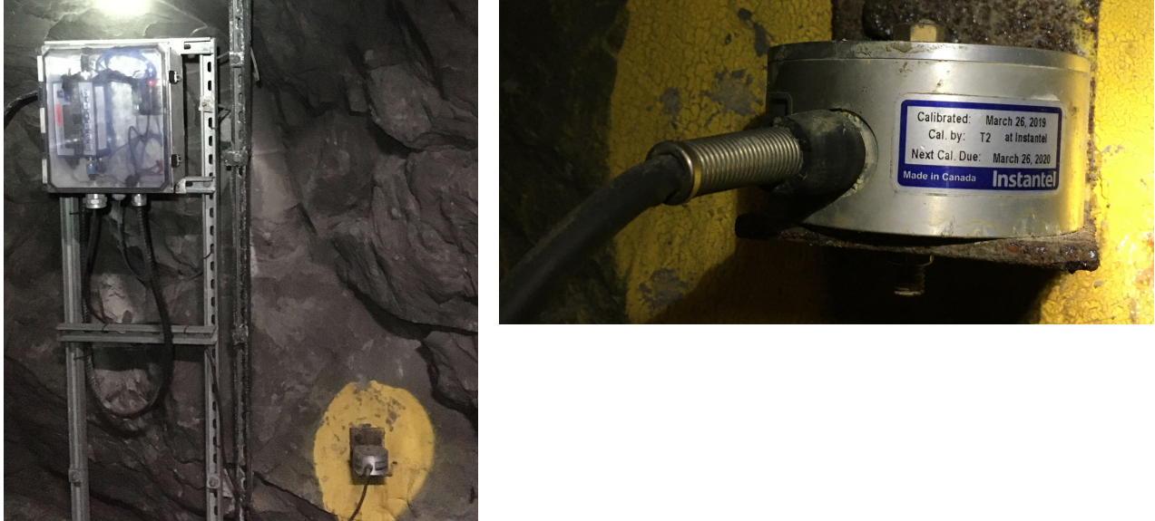
Figure 3. Previous Underground Installation (L75) shown as an example – (Date:2019)
