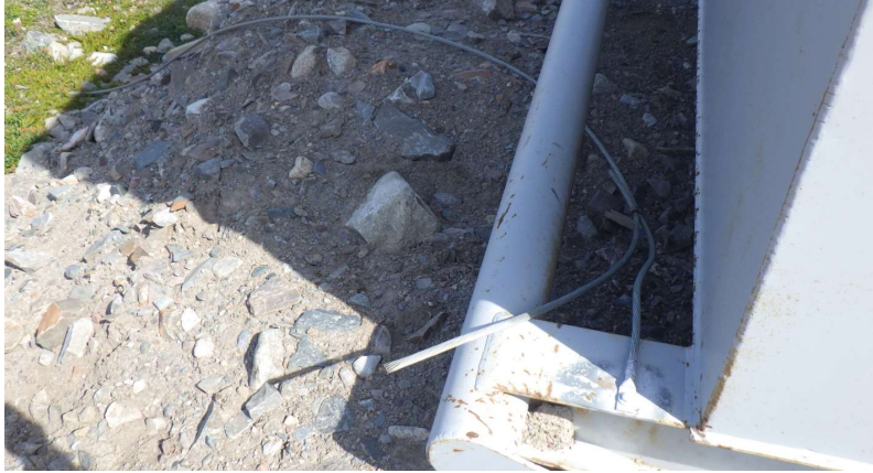
Figure 3-5 Surface Explosive Magazines – Grounding
