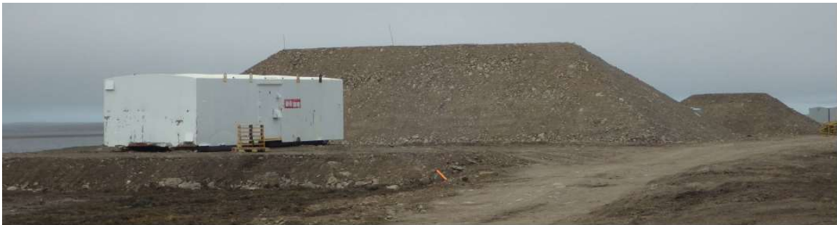
Figure 3-4 Surface Explosive Magazines and Berms
