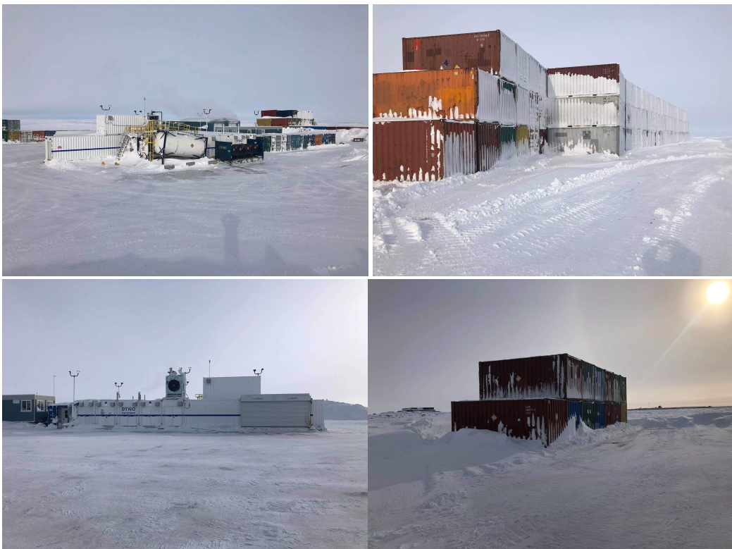
Figure 2-2 Modular Emulsion Plant and Ammonium Nitrate Storage Pad
